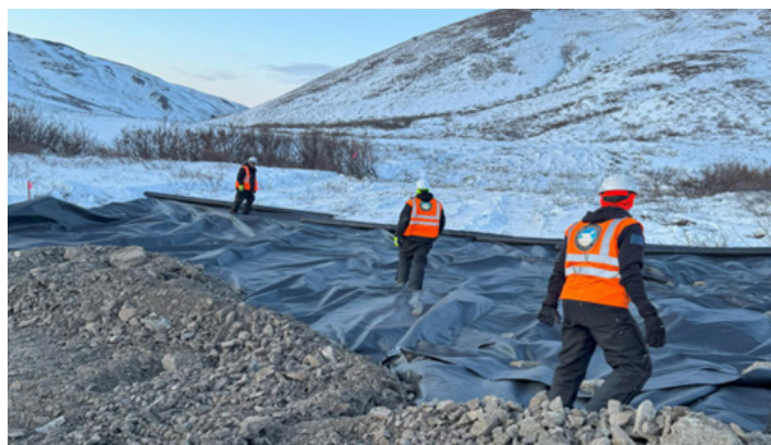
Staking the road alignment, preparing the ground for protective textile fabric. (Photo: Station 10 on Jan. 6)
