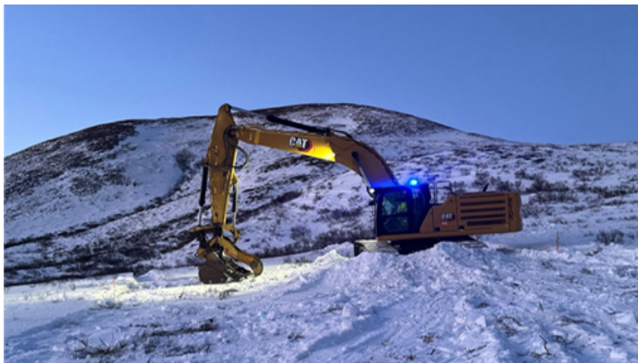
Carefully removing snow along the surveyed road alignment, while minimizing the disturbance to the surrounding tundra. (Photo: Station 18 on Jan. 6)
