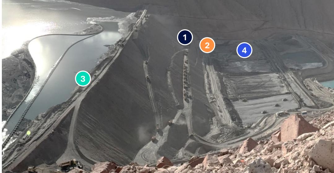
November 2025 – QB Site Visit
