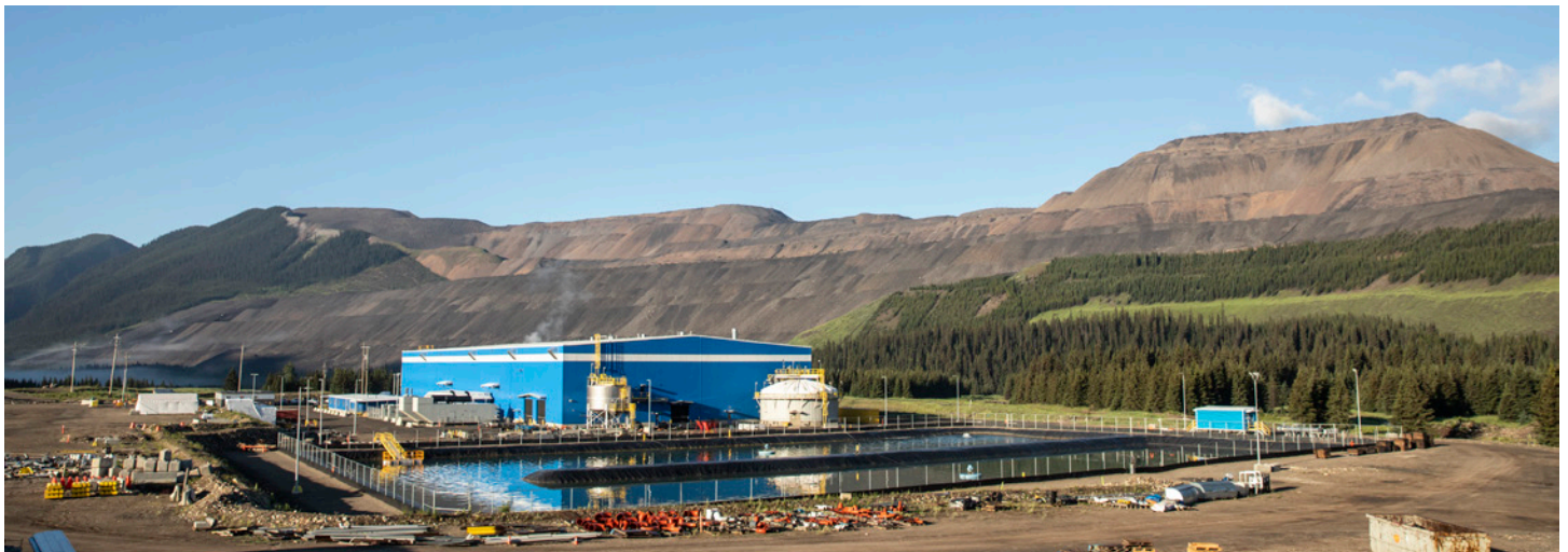
Image: View of the Fording River Operations South Active Water Treatment Facility
