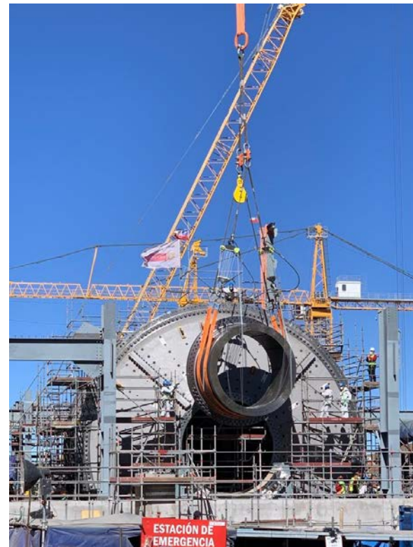
SAG #1 trunnion installation, August 2020
