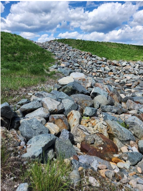
Photo II.26 Siliceous TSF Spillway
