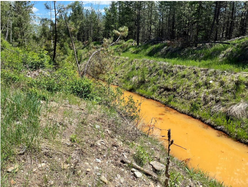
Photo II.24 Seepage downstream of No. 2 Siliceous Dike
