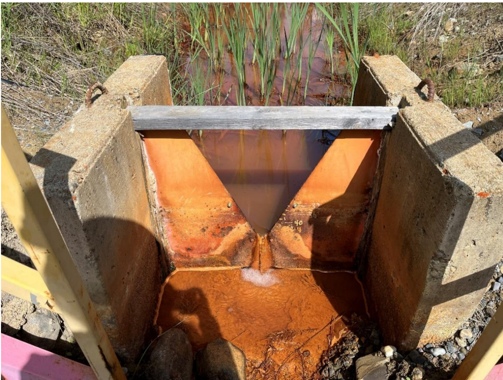
Photo II.16 Weir #4 worn notch
