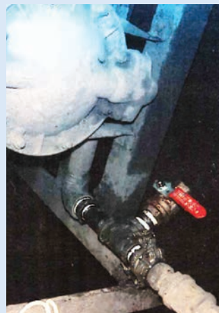
Transfer pump drain for freeze protection. Great job Marquay!
