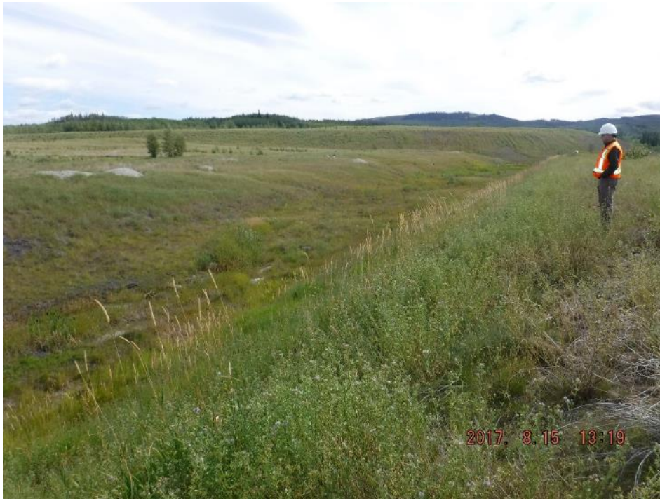
Photo I-52 From dam crest looking northwest at the spillway low flow channel and downstream slope – no obstruction or sign of distress (PTD-2017-42)
