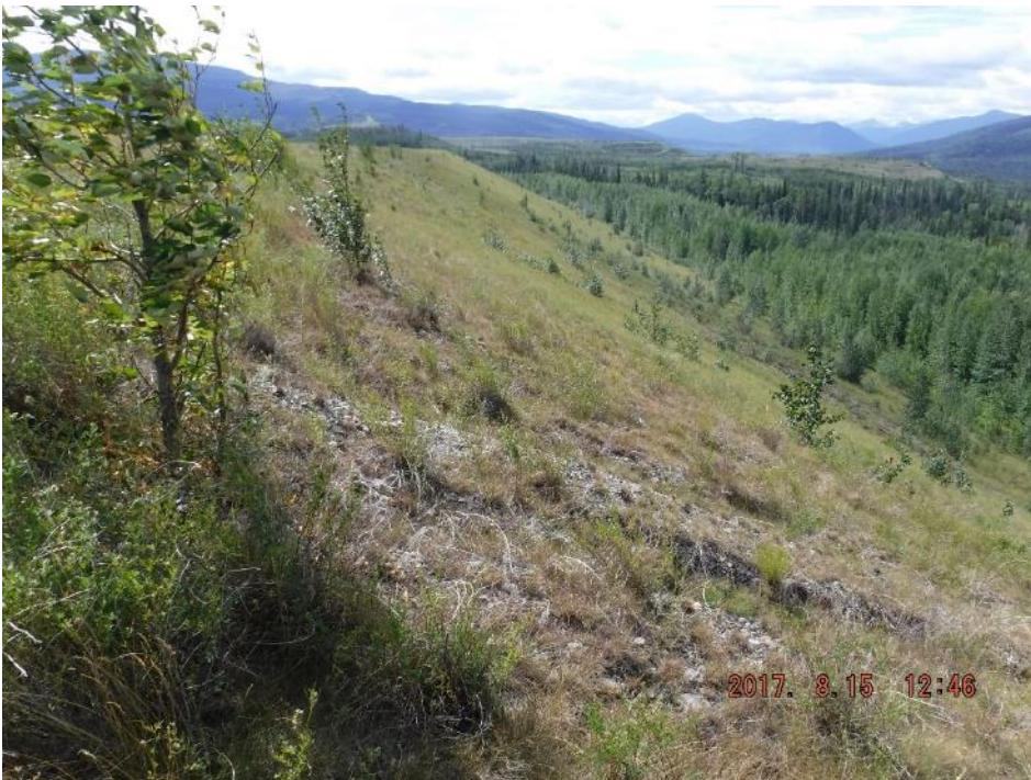
Photo I-42 Overview of the downstream slope from the dam crest near Sta. 1+200 – looking southwest. No sign of distress, significant movement or erosion (PTD-2017-34)
