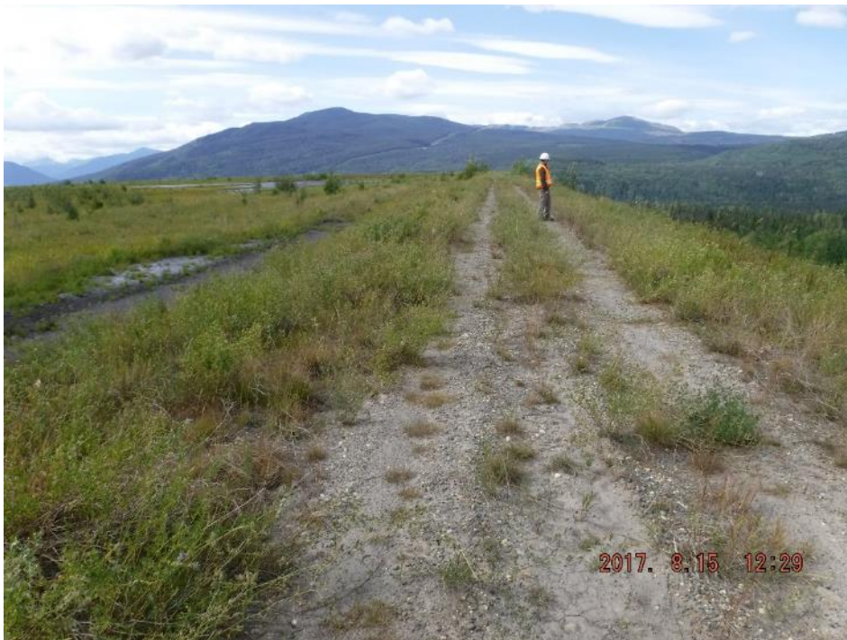
Photo I-40 PTD crest – no sign of distress. Tailings surface is approximately 2 m lower than dam crest level (PTD-2017-32)
