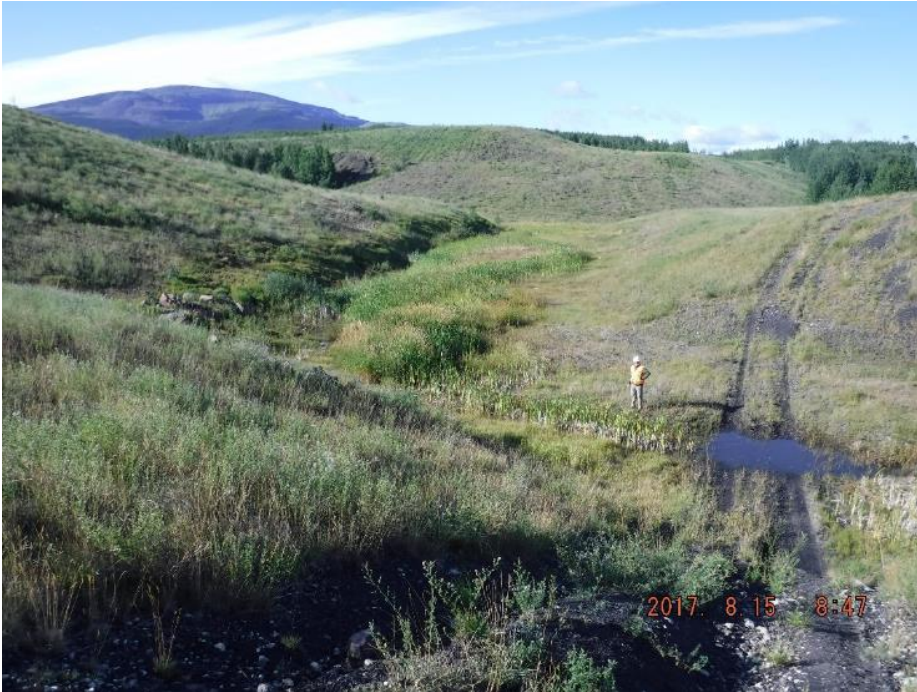
Photo I-5 Spillway channel – viewed from inside the PTD impoundment looking northwest along the channel. Channel is well vegetated but no obstruction observed; (PTD-2017-03)
