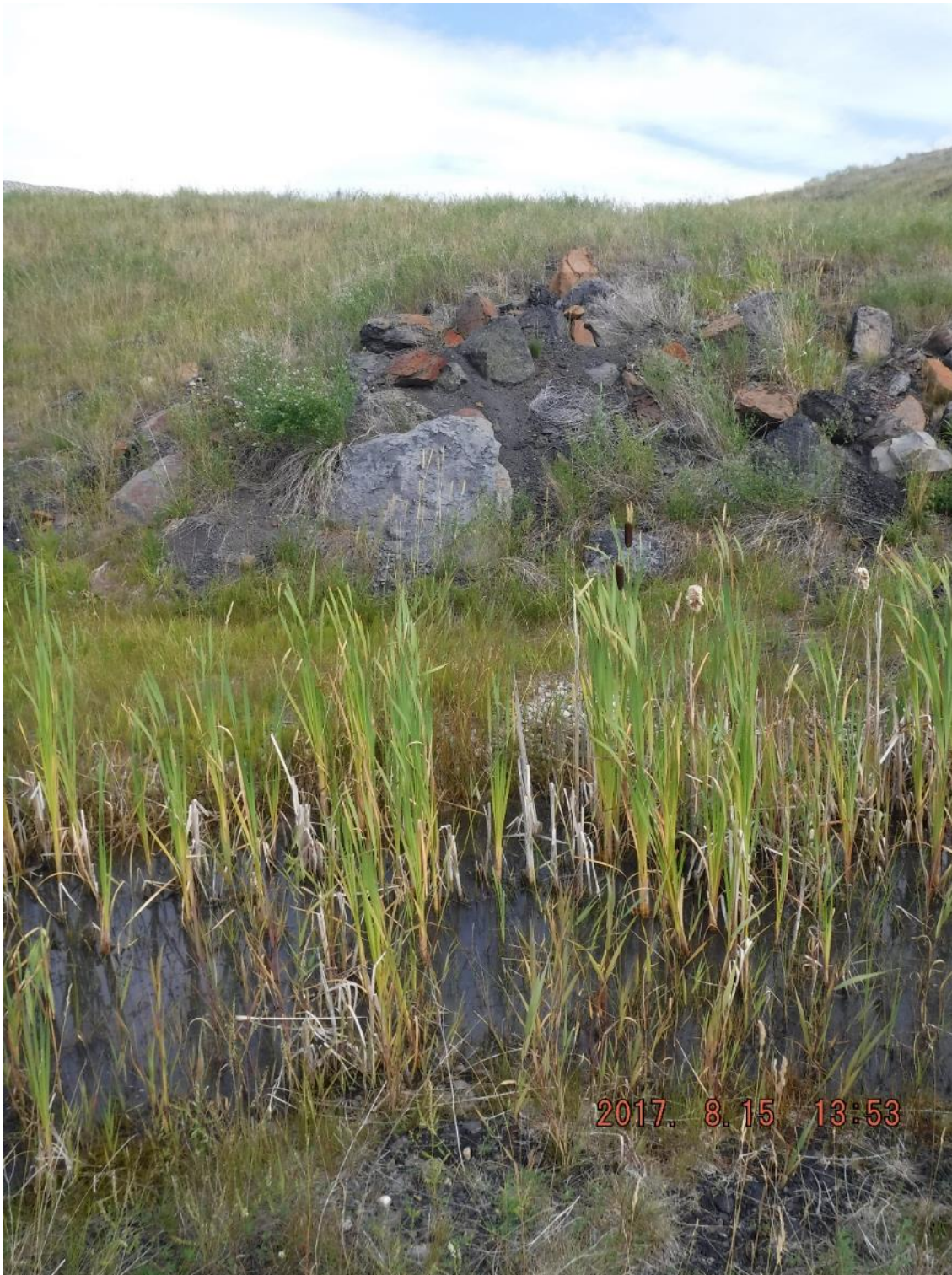
Photo I-53 Standing inside the spillway channel looking north at deteriorating riprap and ponded area inside local depressions inside the channel (PTD-2017-43)
