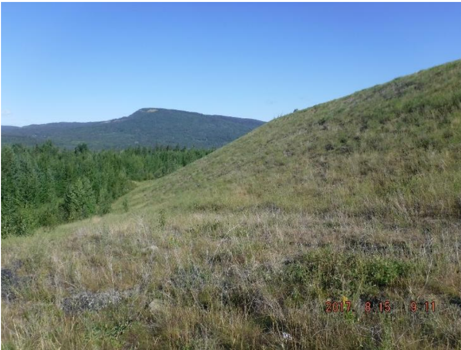
Photo I-12 PTD downstream slope - looking northeast. No sign of distress (PTD-2017-09)
