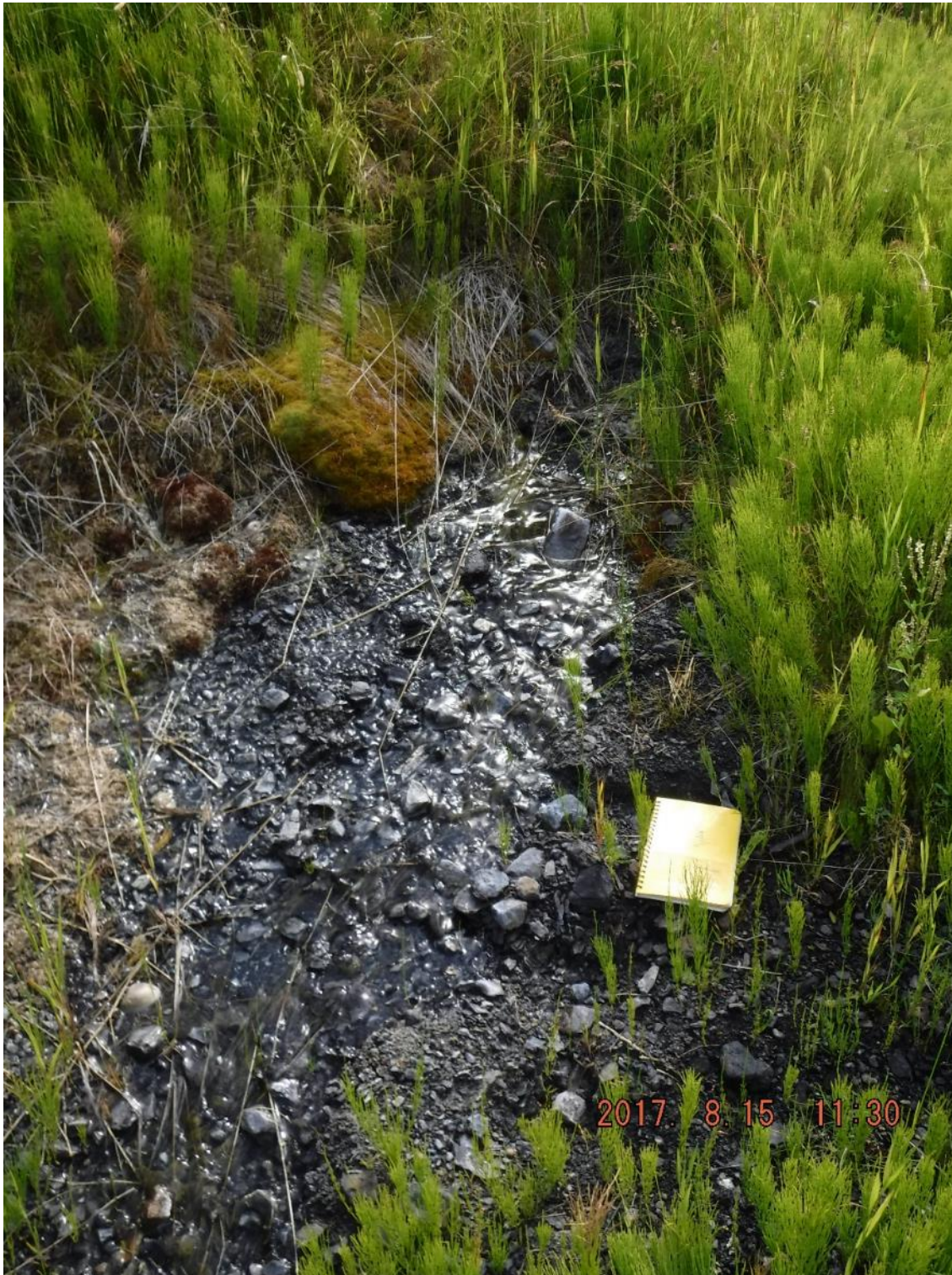
Photo I-30 Flow noted coming from finger drain – flow was estimated 3 to 5 L/min (PTD-2017-23)
