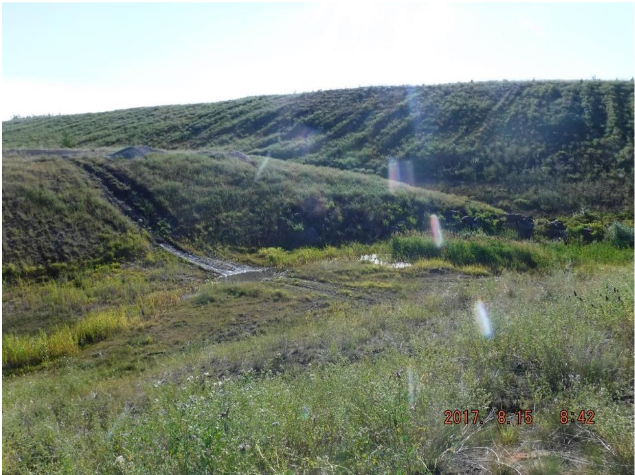
Photo I-1 Spillway channel - looking east towards the spillway channel's 90° bend – minor vegetation, but no obstruction (PTD-2017-01)
