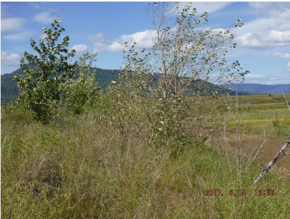
Photo I-50 Large trees on the upstream slope of the PTD (PTD-2017-41)
