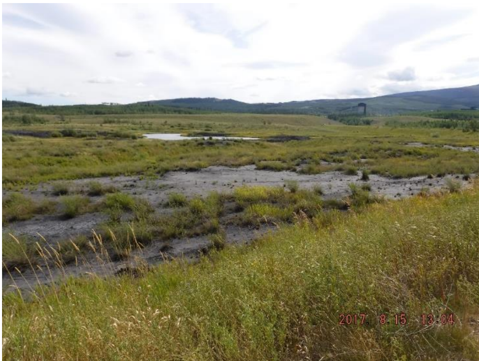
Photo I-46 From dam crest near Sta. 0+600 looking at the ponded area and the tailings beach; no sign of sinkholes or distress (PTD-2017-38)
