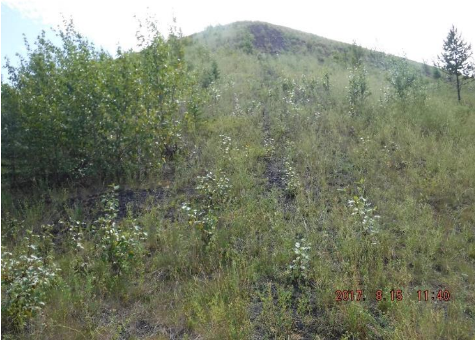
Photo I-32 Overview of PTD northwest corner - steep scarp near downstream slope ramp – inactive due to the amount of vegetation growth on scarp (PTD-2017-25)
