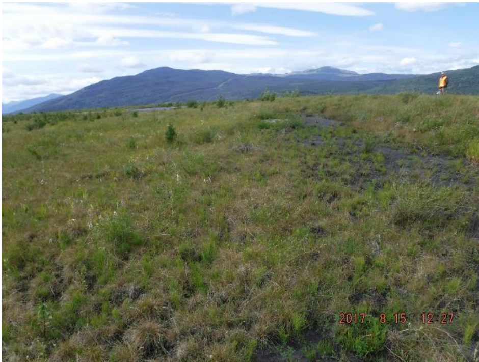
Photo I-39 Upstream Slope and Tailings beach – no sinkholes or sign of distress (PTD-2017-31)
