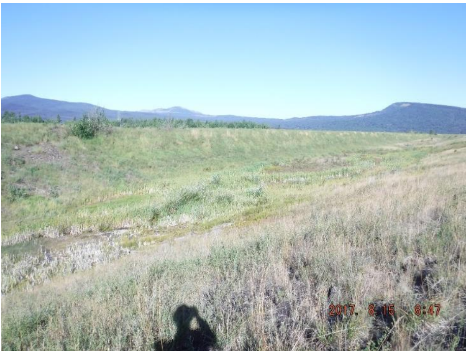
Photo I-5 Spillway channel – viewed from inside the PTD impoundment looking northwest along the channel. Channel is well vegetated but no obstruction observed; (PTD-2017-03)
