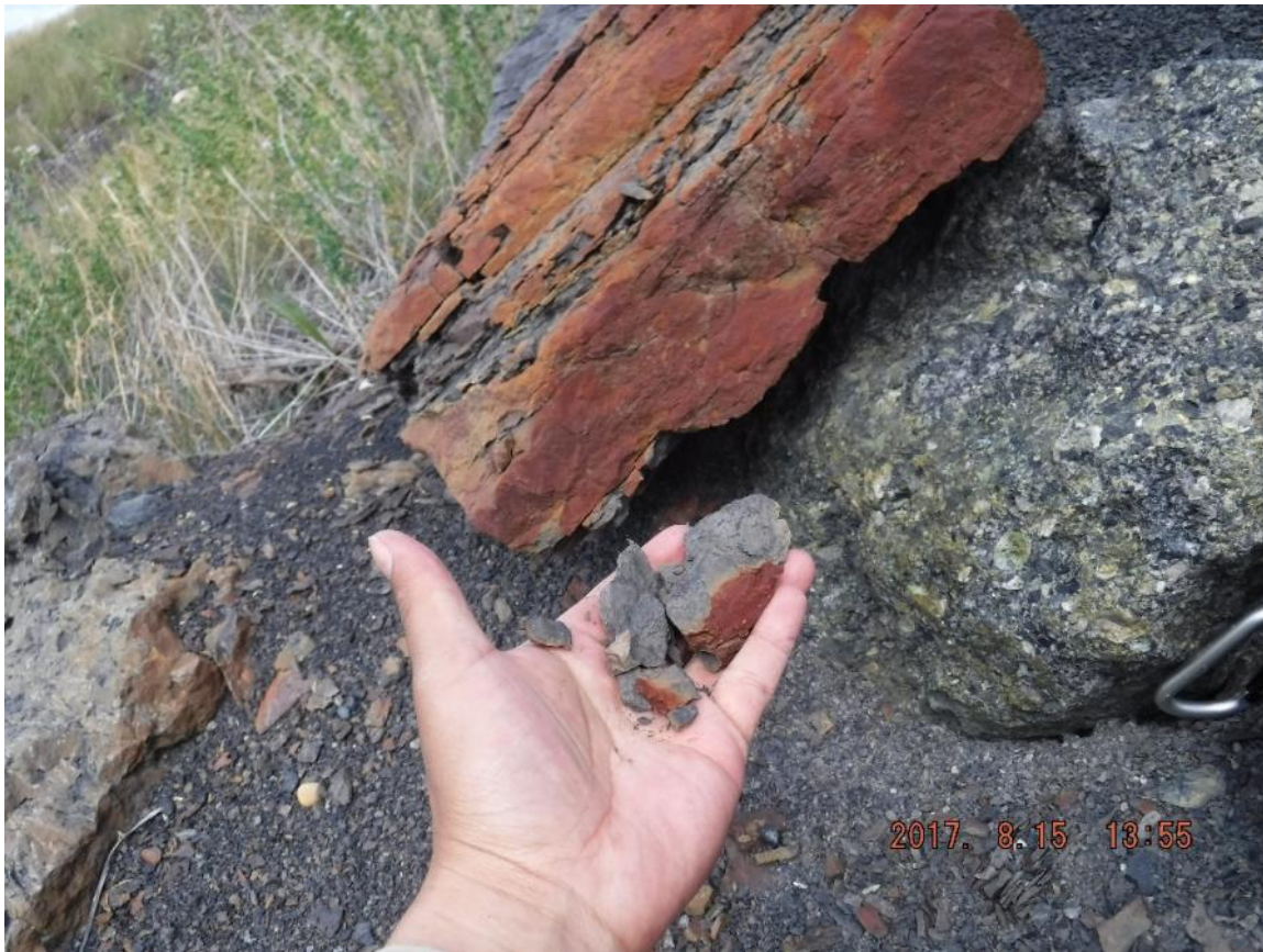
Photo I-56 Closeup of the deteriorating riprap (PTD-2017-44)
