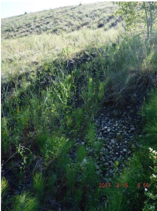
Photo I-17 Finger drain at the PTD toe – <1 L/min flow (PTD-2017-13)
