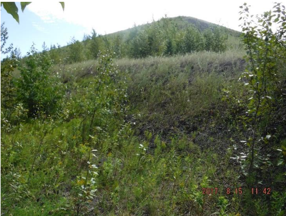
Photo I-32 Overview of PTD northwest corner - steep scarp near downstream slope ramp – inactive due to the amount of vegetation growth on scarp (PTD-2017-25)
