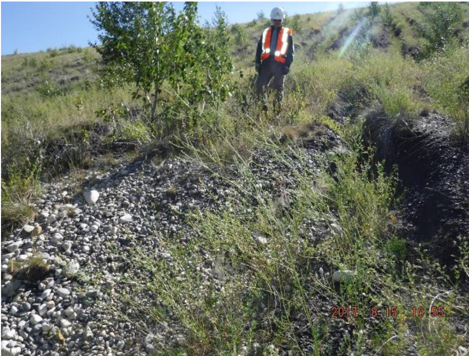
Photo I-27 Closeup of small flow (<1 L/min) downstream of the finger drain outlet (PTD-2017-21)
