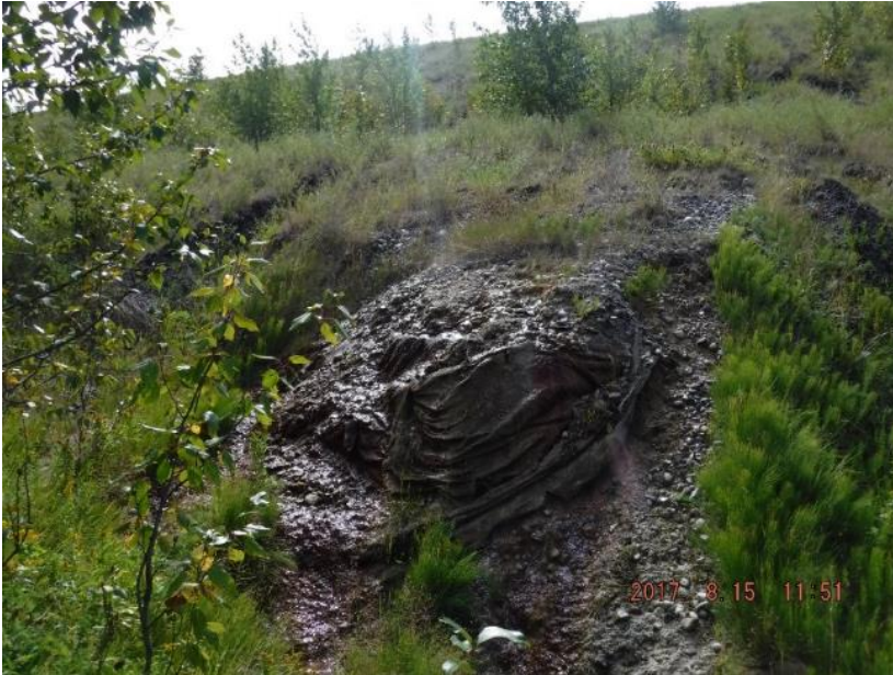
Photo I-33 Finger drain with geotextile – red (oxidized iron) precipitate observed (PTD-2017-26)
