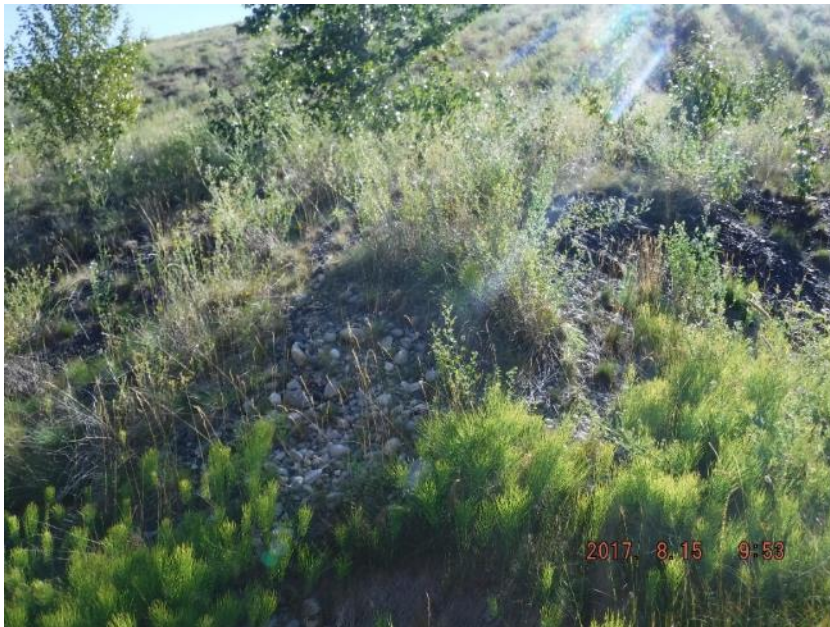
Photo I-16 Finger drain at the PTD toe – <1 L/min flow (PTD-2017-12)
