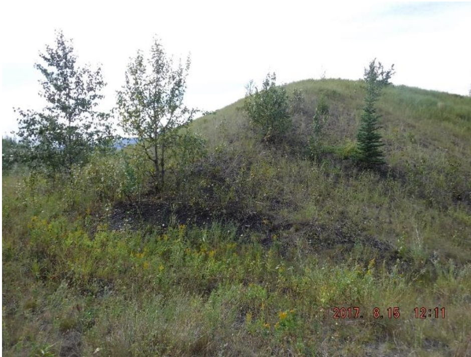
Photo I-35 PTD northeast corner's downstream slope – no sign of distress (PTD-2017-27)
