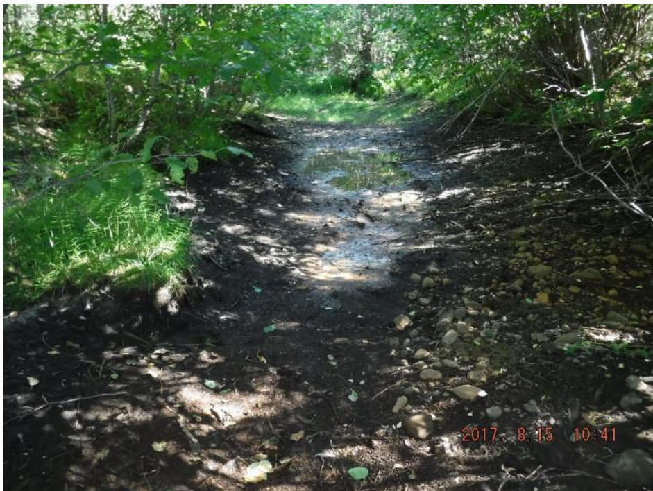
Photo I-25 Outlet channel of the Sedimentation Pond – ponded area appears to be smaller than previous year; no discharge noted (PTD-2017-20)
