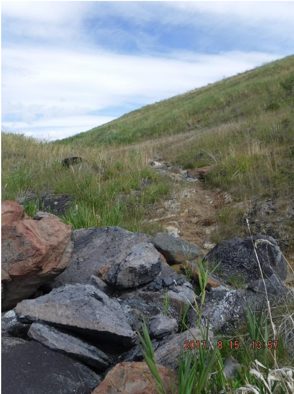
Photo I-55 Standing inside the spillway channel looking east at deteriorating riprap and a small channel behind the riprap with flow of <2 L/min (PTD-2017-44)
