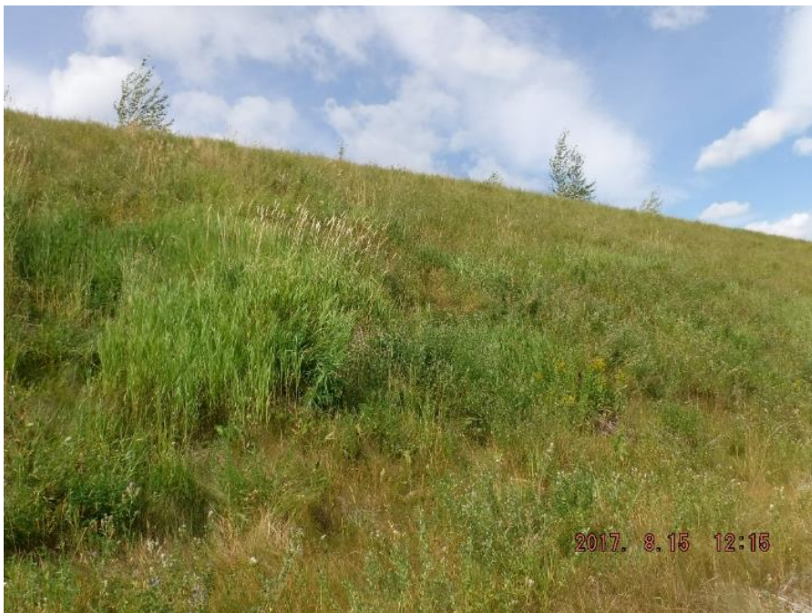
Photo I-36 Change in vegetation type observed at approximately Sta. 2+200. Vegetation is thick lush green, likely indication of increased moisture in this part of the dam (PTD-2017-28)
