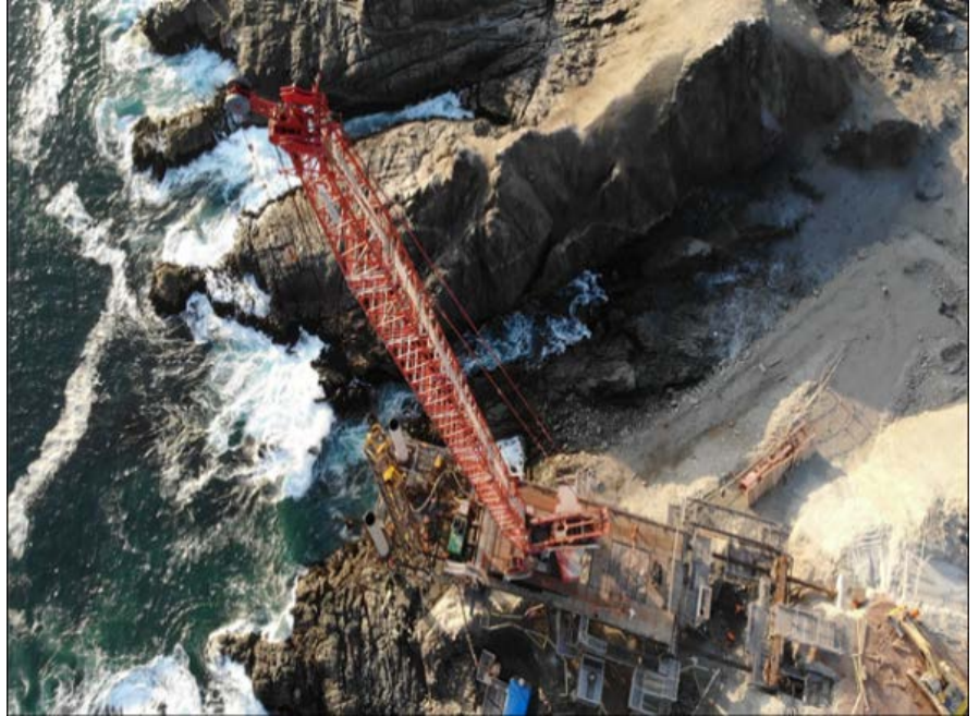
QB2 restarted port marine works.
