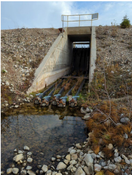
Photo I-23 Polishing Pond Spillway – looking south, spillway outlet, syphons not active, clear flow downstream at the spillway outlet (Location 23)
