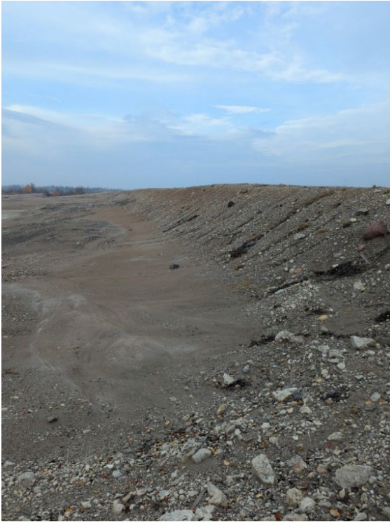
Photo I-4 South Dyke – looking southeast, ponds at the downstream toe drier than typical (Location 4)
