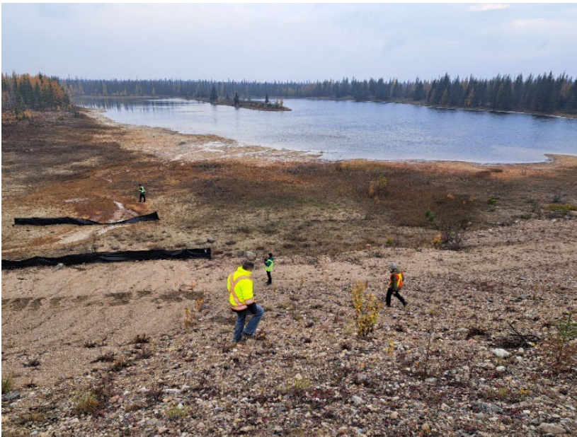
Photo I-11 West Dyke – looking south, downstream slope and coconut matting installed October 2022 (Location 11)
