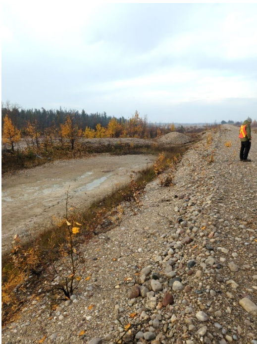
Photo I-2 South Dyke – looking southwest, South Dyke toe, dry where typically have ponded water (Location 2)
