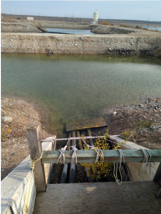
Photo I-23 Polishing Pond Spillway – looking south, spillway outlet, syphons not active, clear flow downstream at the spillway outlet (Location 23)
