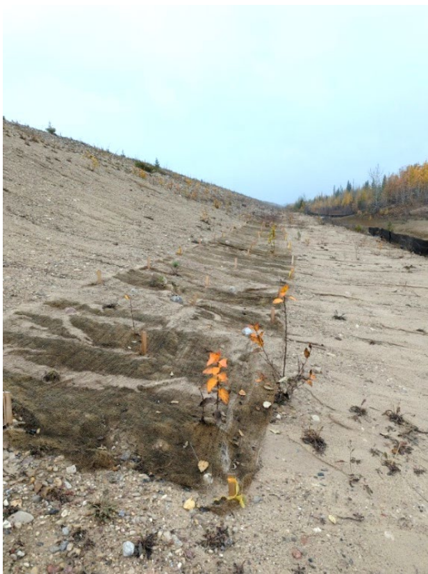
Photo I-11 West Dyke – looking south, downstream slope and coconut matting installed October 2022 (Location 11)
