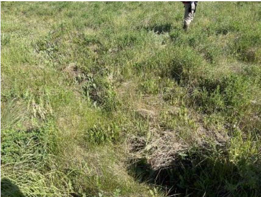
Photo II-2 Tailings Impoundment – Local depression on cover. No signs of erosion or standing water in low spot
