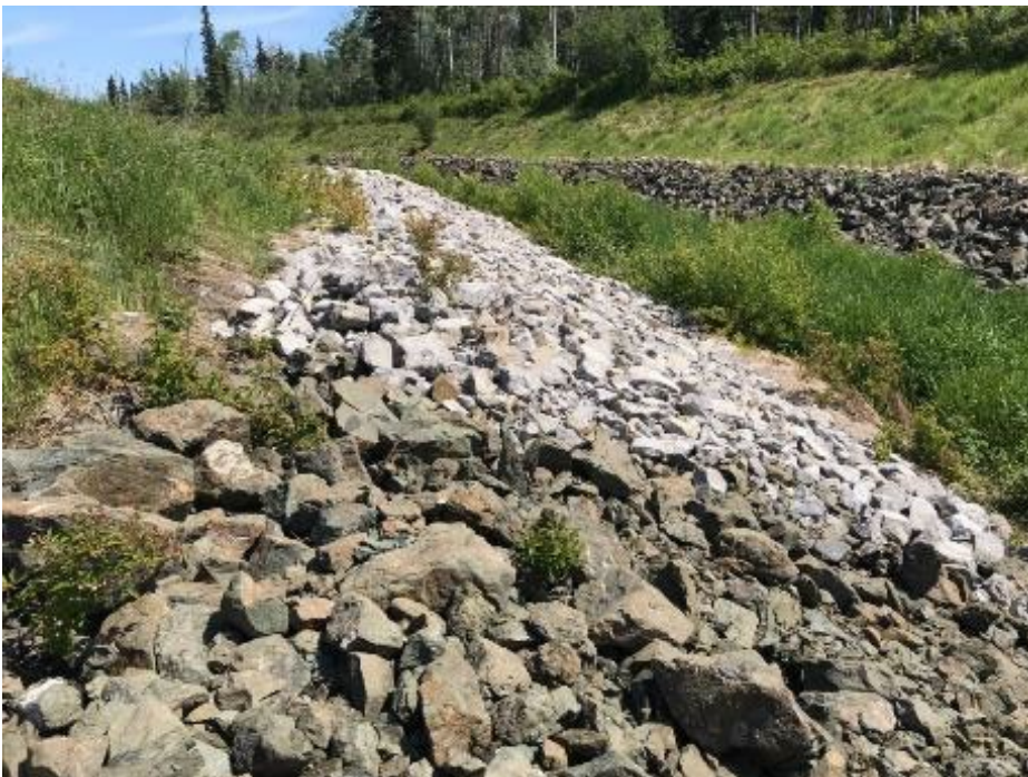
Photo II-36 Ed Creek Diversion Channel – Looking upstream from near second bend. Light coloured area of riprap was replaced in 2014 and is in good condition
