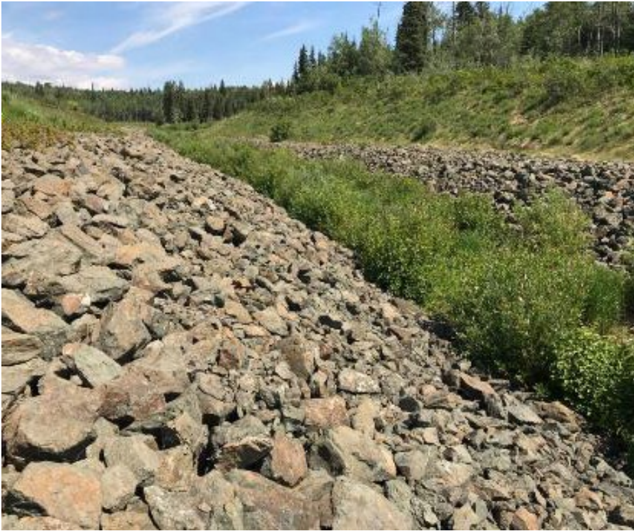
Photo II-36 Ed Creek Diversion Channel – Looking upstream from near second bend. Light coloured area of riprap was replaced in 2014 and is in good condition
