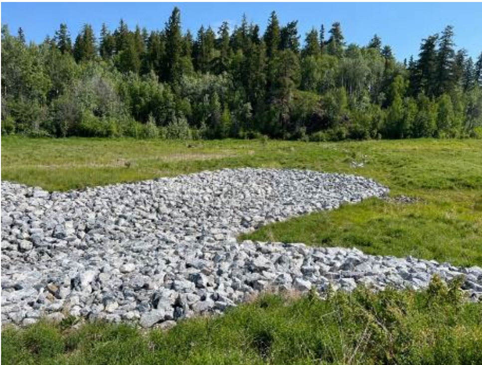
Photo II-18 Closure Spillway – Inlet apron
