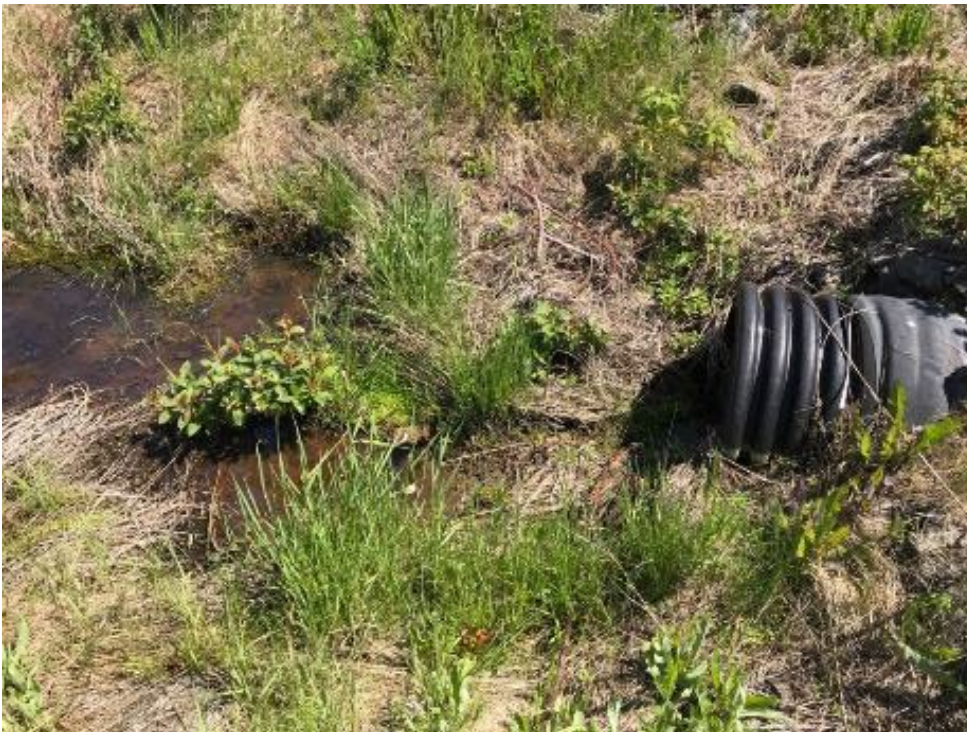
Photo II-42 Inlet of 460 mm culvert on north bank of Ed Creek Diversion Channel. Vegetation cleared near inlet in October 2022
