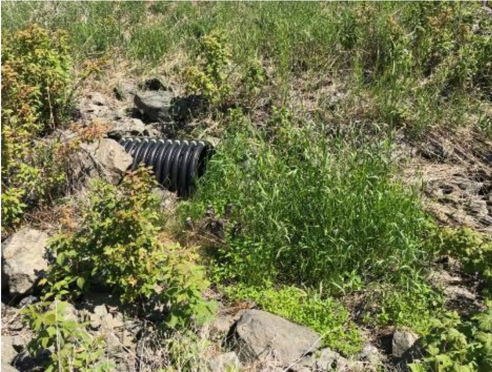
Photo II-42 Inlet of 460 mm culvert on north bank of Ed Creek Diversion Channel. Vegetation cleared near inlet in October 2022
