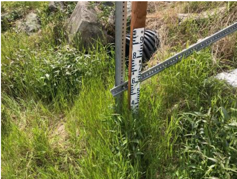
Photo II-26 Outlet Channel – Culvert inlet and flow monitoring station. Vegetation cleared in October 2022
