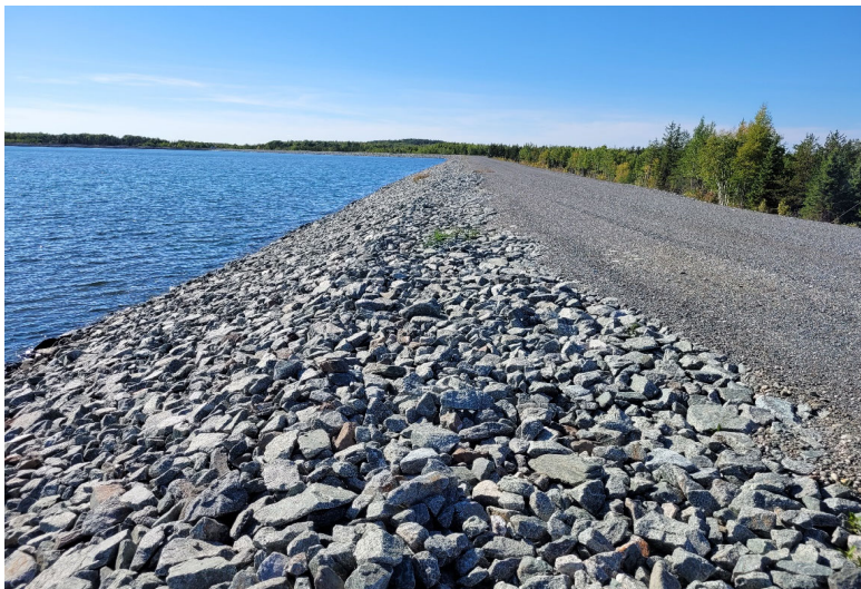
Photo 2 : Dams 1D – View of the upstream slope with riprap replaced. traffic gravel was placed on the crest.
