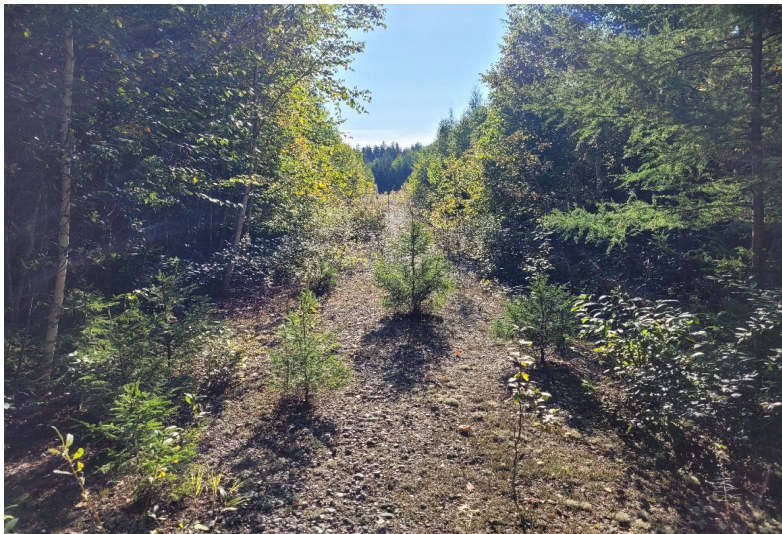
Photo 14 : Trees are continuing to encroach on the side slopes and crest of the Dam 4A embankment
