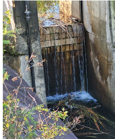
Photo 15 : Main spillway at Dam 4B - Significant debris observed during the 2022 inspection has been removed
