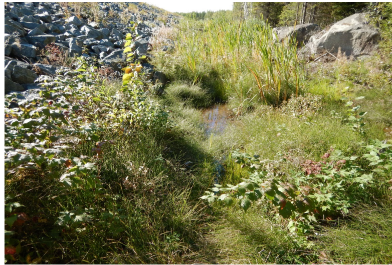
Photo 3 : Ponded water with little to now observable flow at toe of Dam 1C. Similar flows occur on Dams 1A and 1B.
