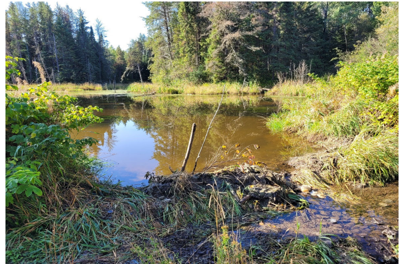
Photo 19 : Beaver activity historically observed at the toe of Dam 4B is not actively occurring. Continued monitoring is required.
