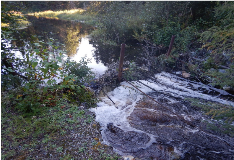
Photo 13 : Unnamed Creek to the west of Dam 2B. Access road fill has been breached due to beaver blockage of culverts immediately to the west.
