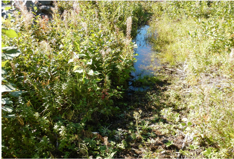
Photo 5 : Area of ponded water at the toe of Dam 1C, due to disturbance by tree removal equipment.
