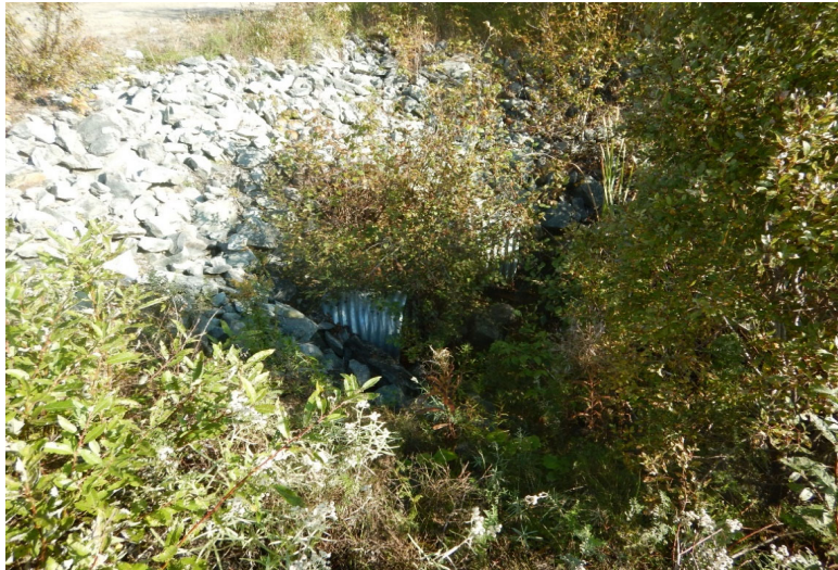
Photo 17 : Culverts at the final effluent point were clear although some limited vegetation is present upstream
