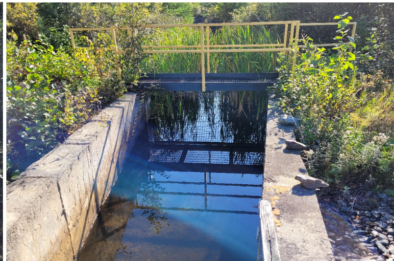
Photo 16 : outflow channel from the spillway to the Parshall flume contains significant vegetation
