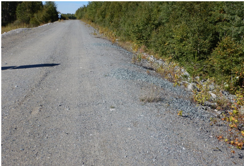
Photo 10 : Erosion features that have been infilled on the downstream shoulder of Dam 1E.
