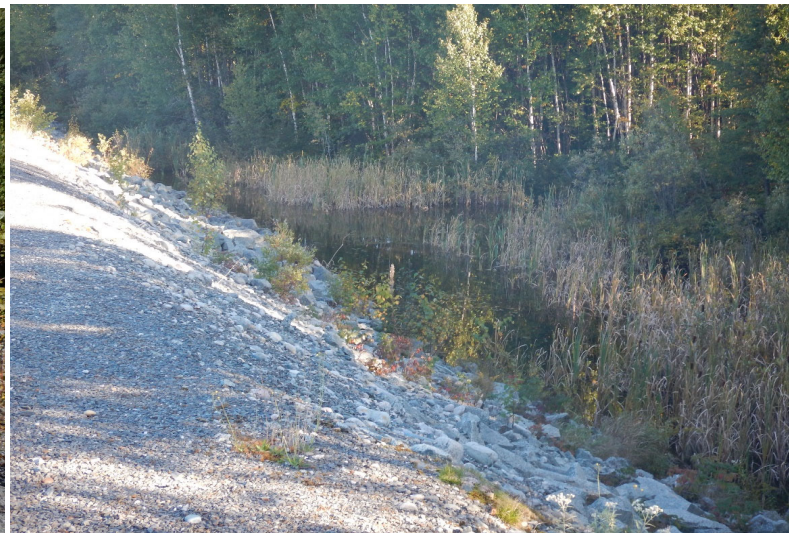
Photo 12 : Dam 2A - Stagnant water at toe of Dam 2B.
