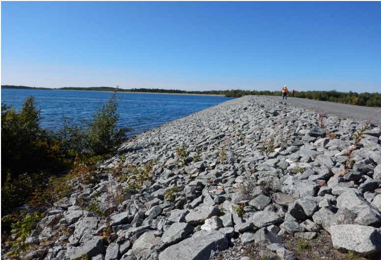
Photo 1 : Dams 1D – View of the upstream slope with riprap replaced.
