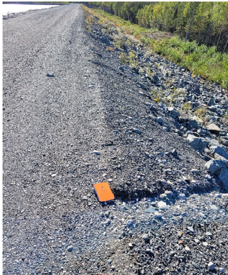
Photo 9 : Dam 1B - Minor crest erosion features will require maintenance in future.
