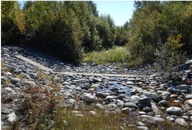
Photo 6 : Concrete weir of the second emergency spillway between Dams 1D and 1E at the TSF with approach channel in background. Good condition.
