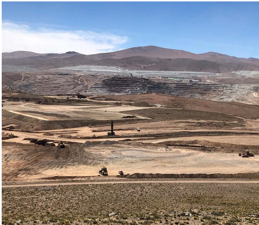
General view of the concentrator area, looking east. March 1, 2019.
