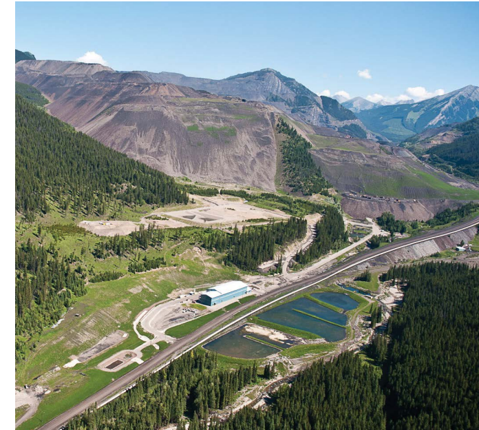
The West Line Creek Active Water Treatment Facility at Line Creek Operations.
