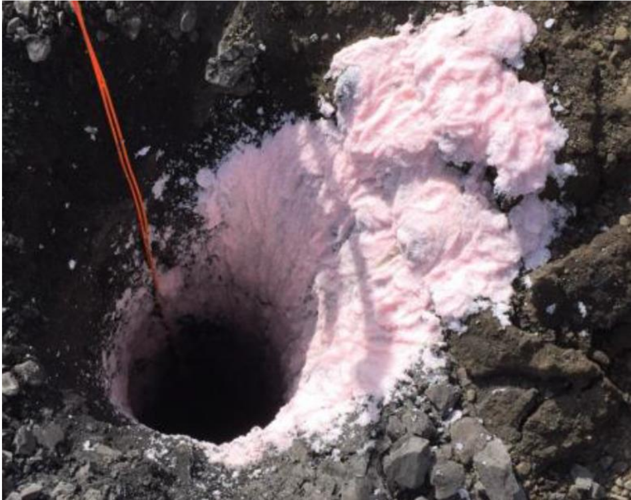
Figure 2-11 Augured Emulsion Blasting Product Stuck to the Sides of an Upper Section of a Drill Hole for Blasting
