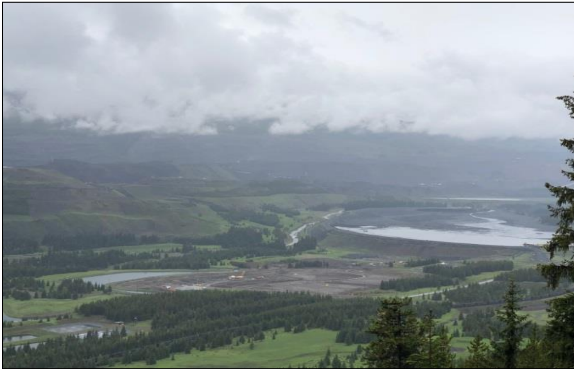
Figure 2-7 Fording River Operation South Active Water Treatment Facility Construction Site (June 2018)
