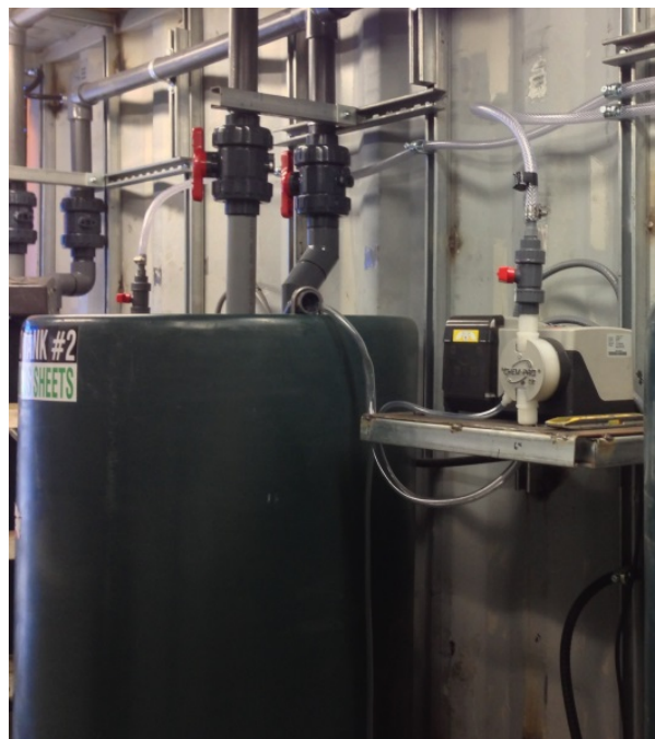
Figure 4.9 Antiscalant reagent tank and reagent pump
