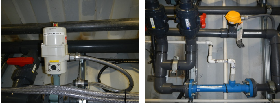
Figure 4.4 Process flow control valve (left); process flow meter and inline mixer (right)
