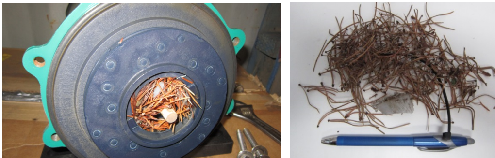
Figure 4.11 Blockages of the discharge pump impeller on August 28 (left) and September 6 (right)
