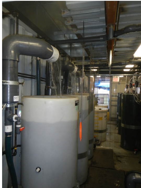
Figure 4.5 Cascades located in the process seacan
