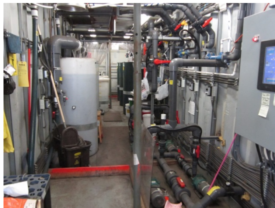
Figure 4.3 The interior of the process seacan
