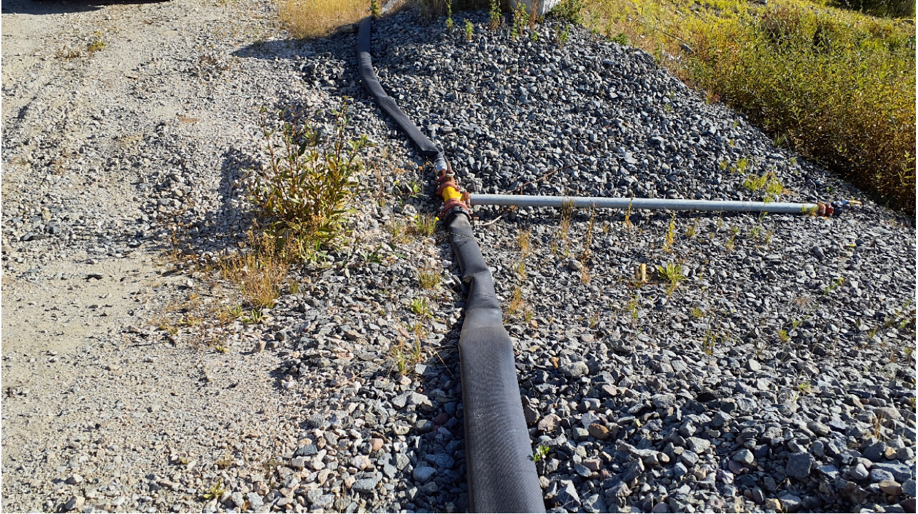
Photo I-C-4 View of spillway inlet. Pipeline is related to temporary diesel pump stationed on crest. (BTH-2023-15)
