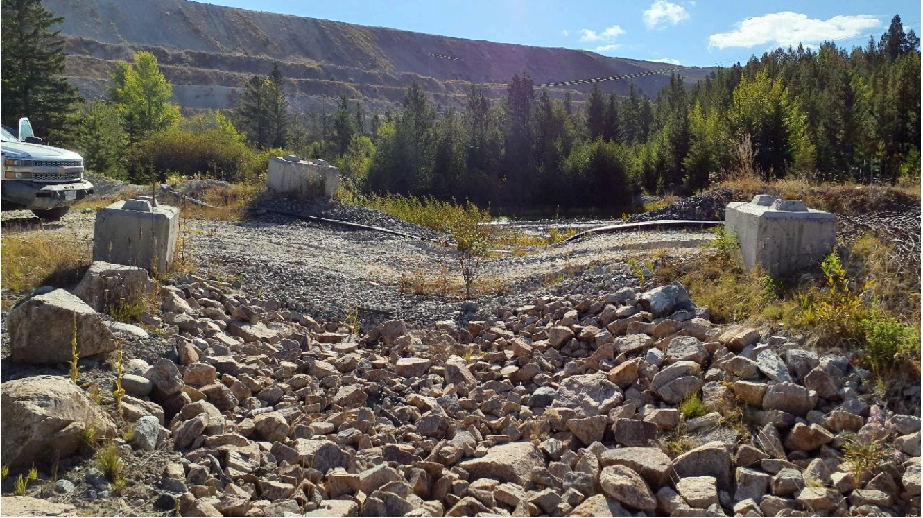
Photo I-C-5 Spillway channel and road crossing at right abutment. (BTH-2023-16)
