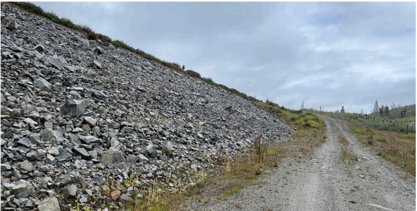
Photo I-B-3 Left abutment and downstream slope, looking north, with no observation of erosion scours or damage. (BTH-2023-07)
