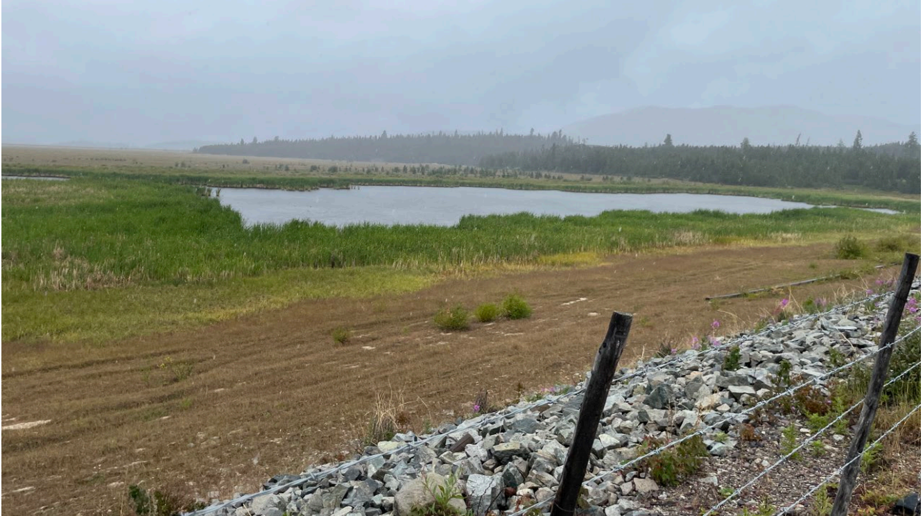
Photo I-B-9 Overview of upstream beach, looking towards dam. No sign of erosion or depression was observed. (BTH-2023-08)
