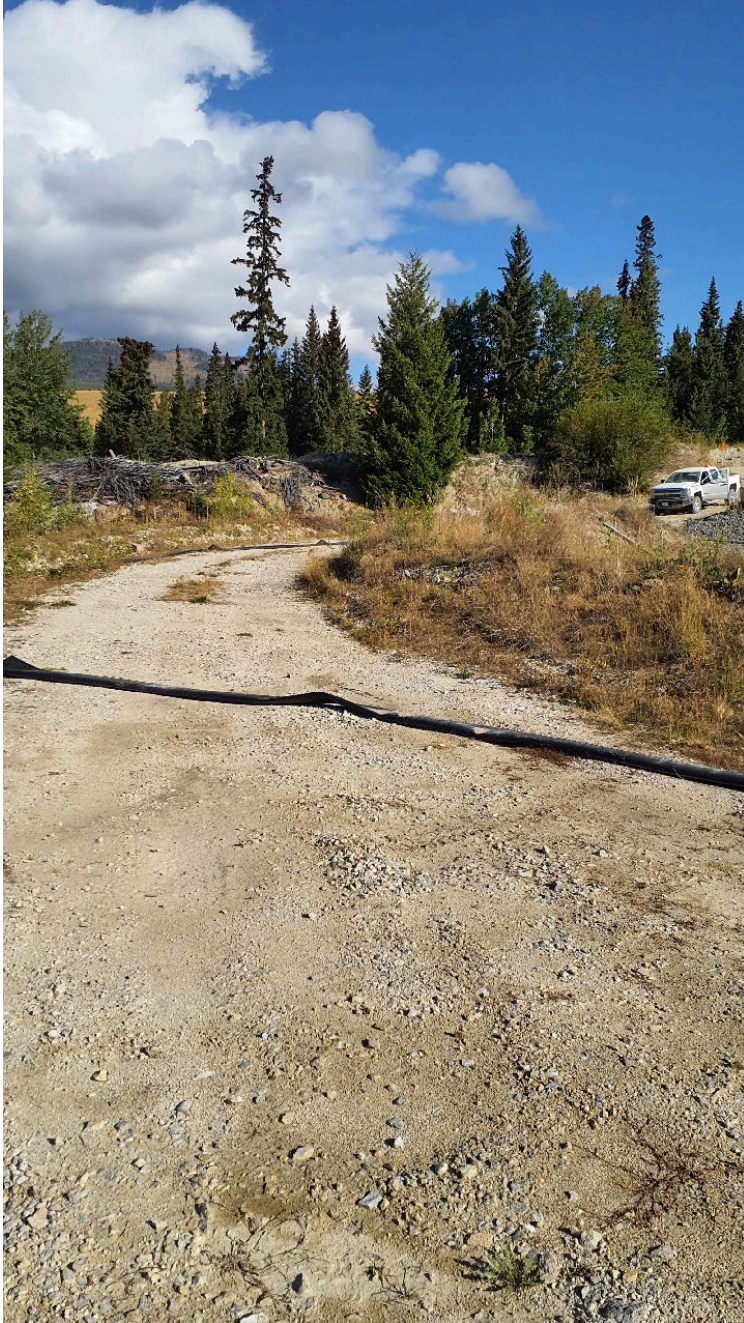
Photo I-C-2 R3 Seepage Pond dam crest, no cracking or no sign of distress was observed. (BTH-2023-13)
