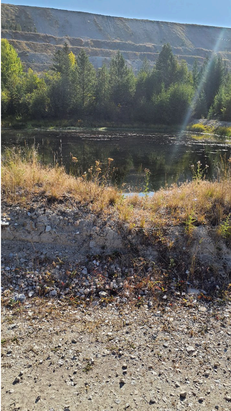
Photo I-C-7 Low point of the berm along upstream side of dam crest. KCB recommended the dam survey be checked to confirm this feature is captured and has been accounted for in the freeboard calculation. (BTH-2023-17)
