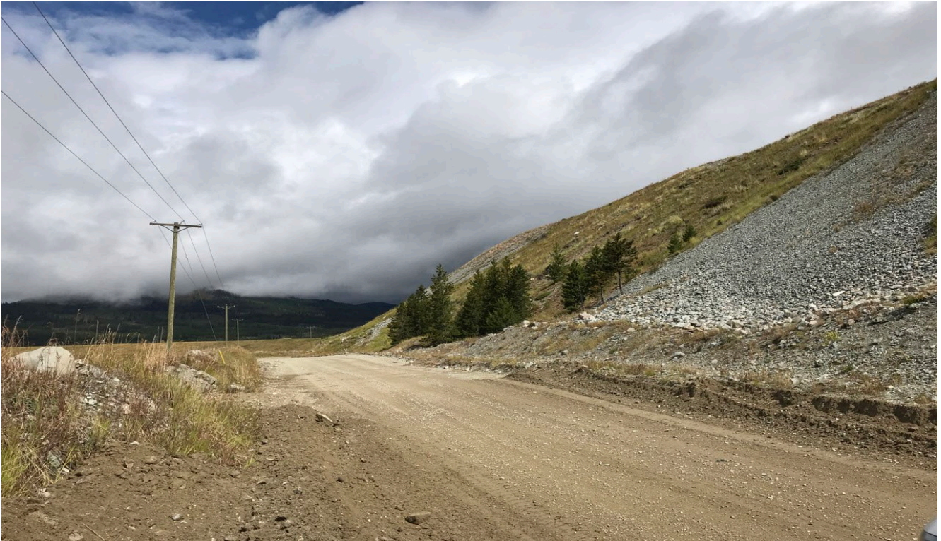
Photo I-A-7 Overview of downstream slope from mine road. Vegetation cover is well established. Previous erosion areas, covered by rockfill, are holding up well (BTH-2023-03)
