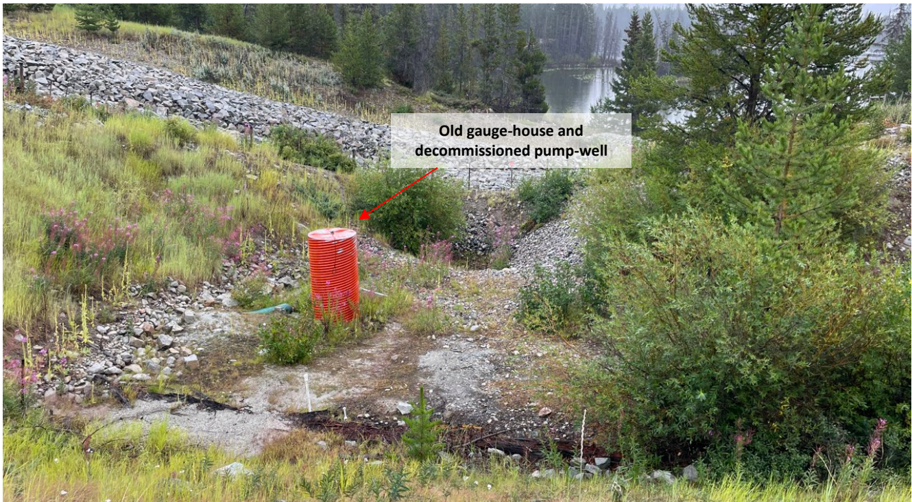
Photo I-B-6 Decommissioned pumping well and discharge point of underdrain. (BTH-2023-09)
