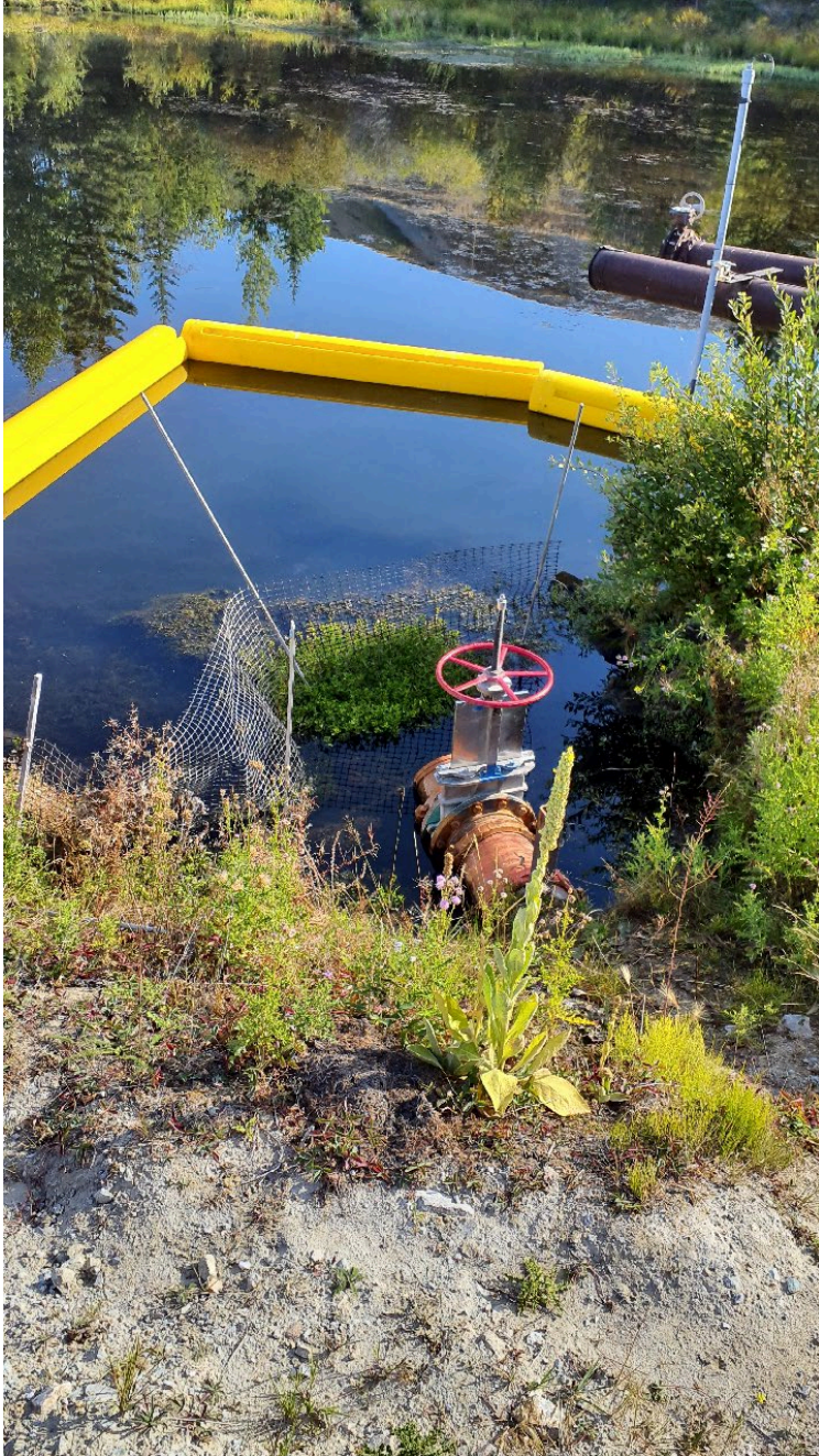
Photo I-C-3 View of outlet pipe, debris mesh and new debris boom. Clear water was flowing at the time of the site visit. (BTH-2023-14)
