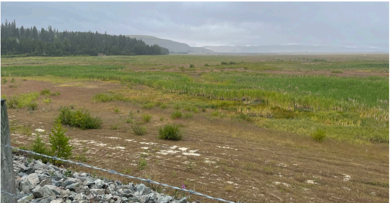
Photo I-B-9 Overview of upstream beach, looking towards dam. No sign of erosion or depression was observed. (BTH-2023-08)
