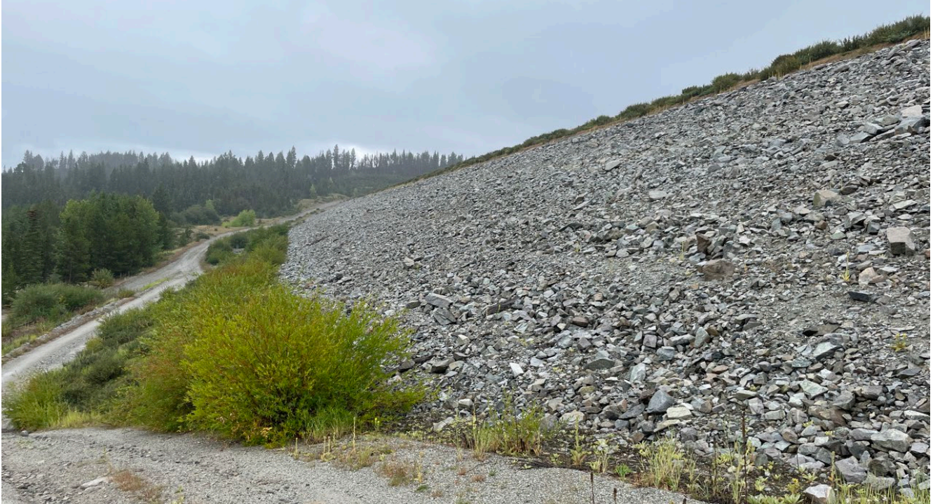
Photo I-B-4 Left abutment and downstream slope, looking south, with no observation of erosion scours or damage. (BTH-2023-07)
