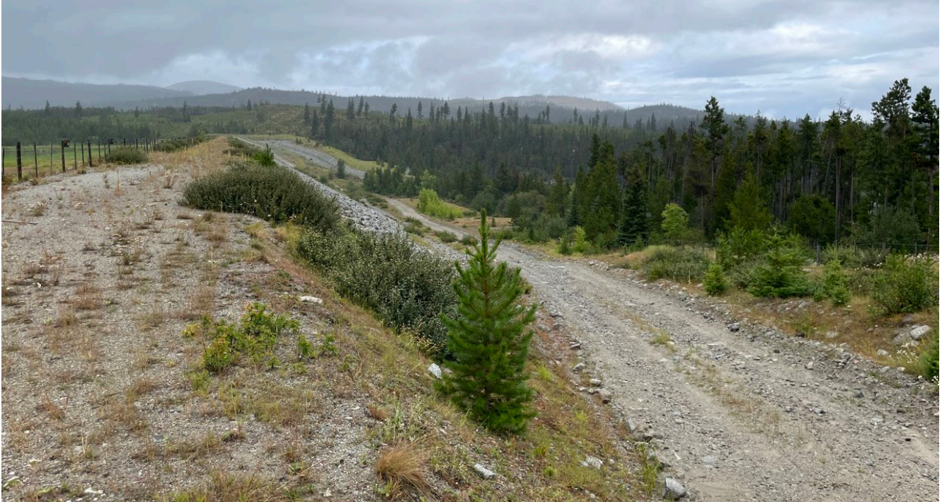
Photo I-B-3 Left abutment and downstream slope, looking north, with no observation of erosion scours or damage. (BTH-2023-07)
