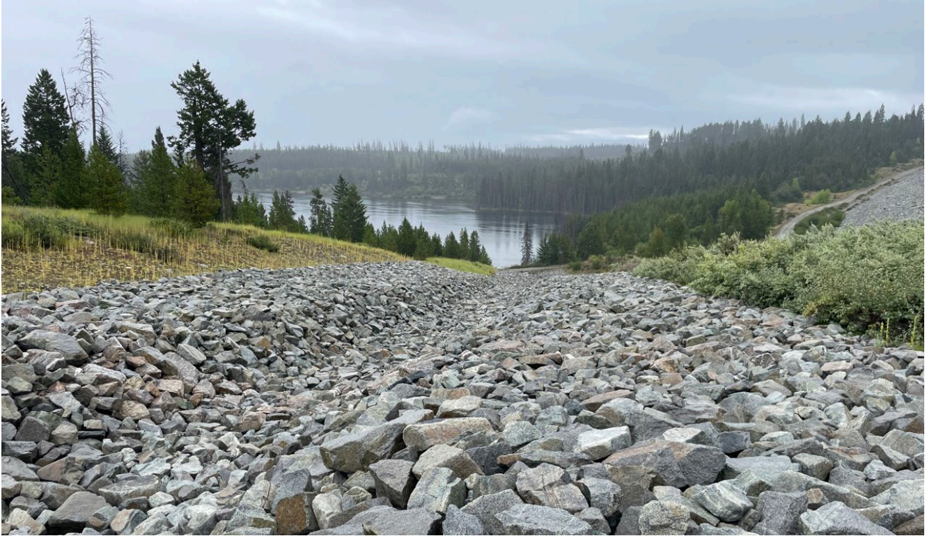
Photo I-B-15 Riprap lined portion of spillway channel looking towards Bose Lake. (BTH-2023-11)
