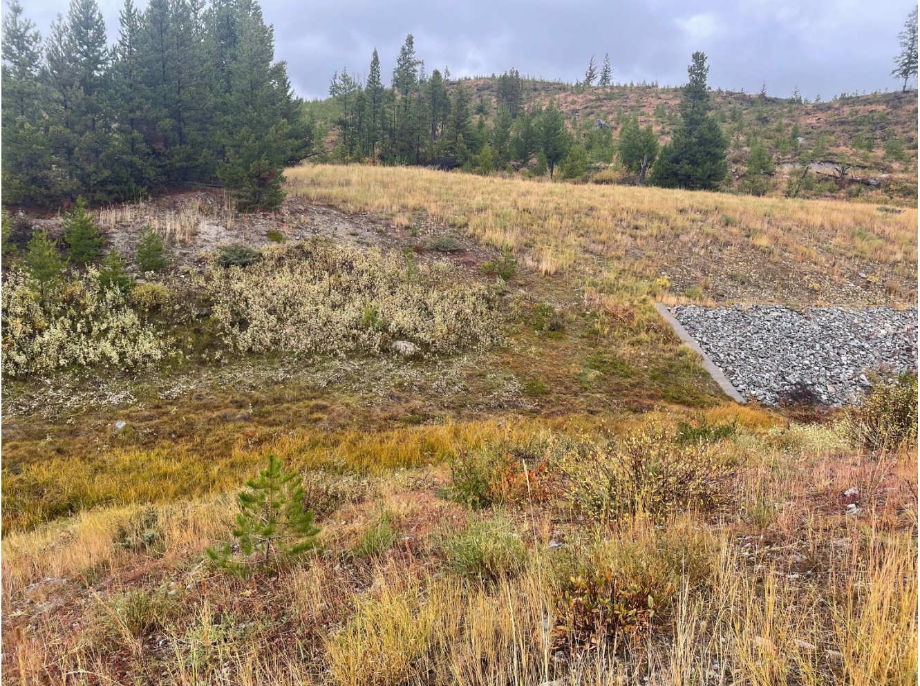
Photo I-B-14 Spillway channel between inlet and riprap-lined segment, after vegetation clearing was completed, photo provided by HVC after site visit.
