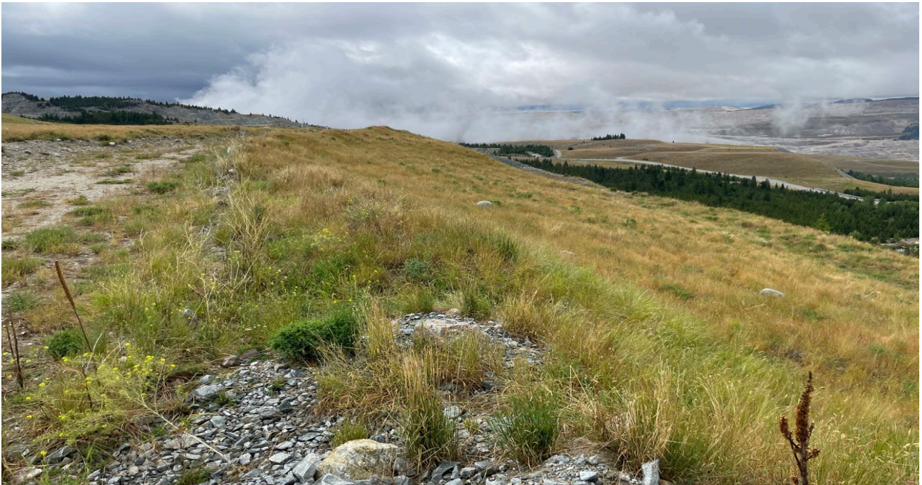
Photo I-A-6 Upper portion of downstream slope with reclamation cover. (BTH-2023-02)
