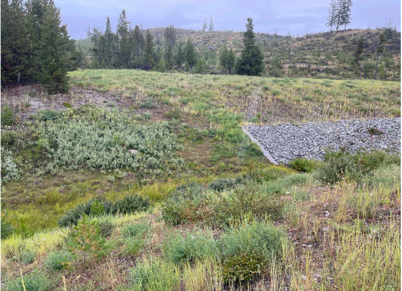
Photo I-B-13 Spillway channel at transition point between inlet and riprap-lined segment, looking towards north. (BTH-2023-10)
