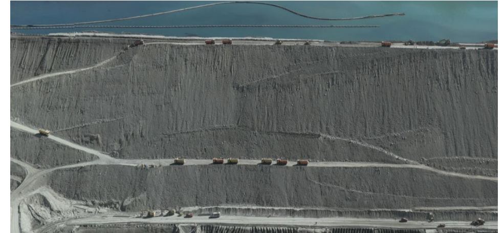
Rock bench 4 under construction, October 24, 2025
