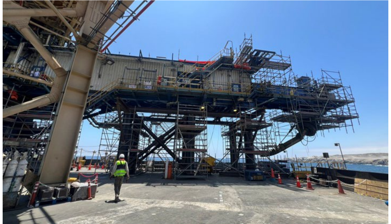
Boom structural support installation, October 24, 2025
