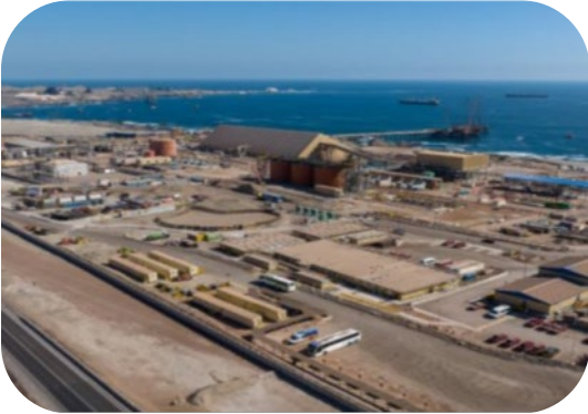
QB desalination plant
