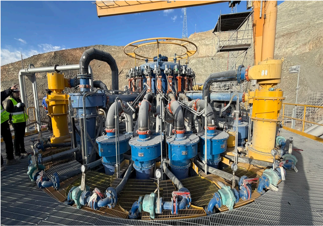
First cyclone battery refitted, October 24, 2025
