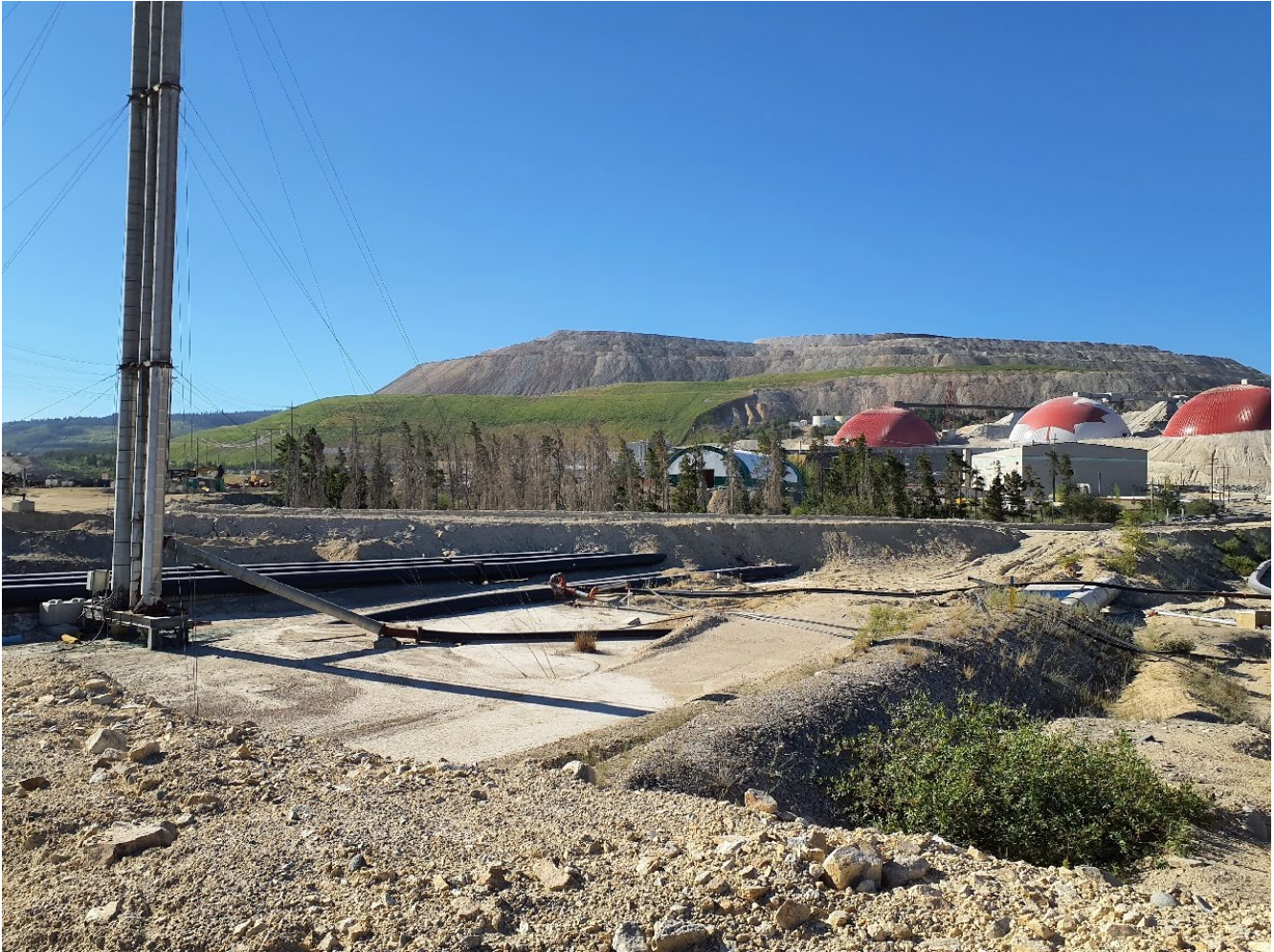
Photo I-4 7-Day Pond TSF impoundment. Structure within TSF impoundment is part of permanent dewatering-pump system. Pumping system was active at the time of the site visit (SDP-2022-04)
