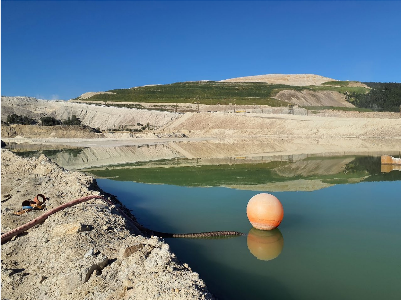
Photo I-5 7 Day Pond TSF impoundment view from north abutment. Poned water observed at the time of the site visit (SDP-2022-05)
