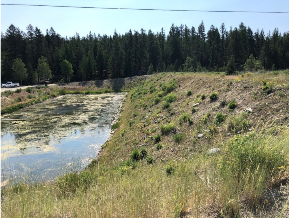
Photo II.32 Sludge Impoundment North Dike downstream slope
