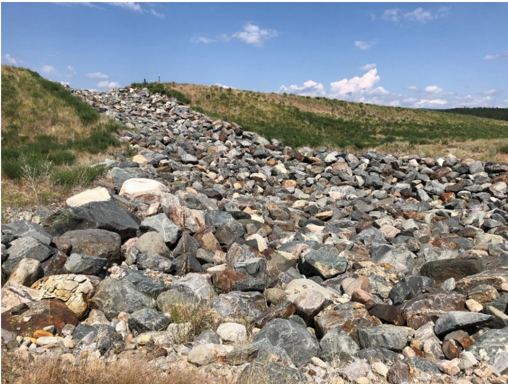
Photo II.26 Siliceous TSF Spillway
