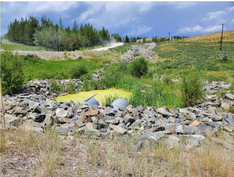
Photo II.20 Emergency Spillway Channel outlet to Cow Creek
