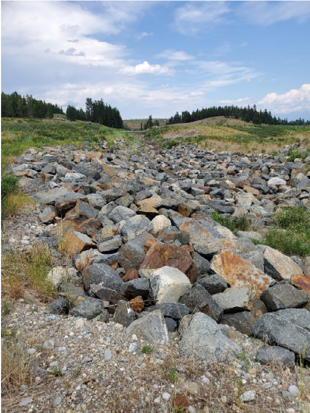
Photo II.20 Emergency Spillway Channel outlet to Cow Creek
