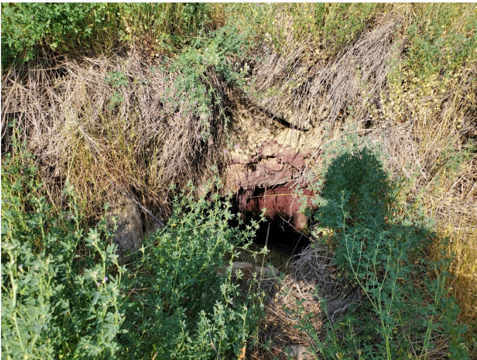
Photo II.36 Void from Collapse of Disused Pipe in Calcine
