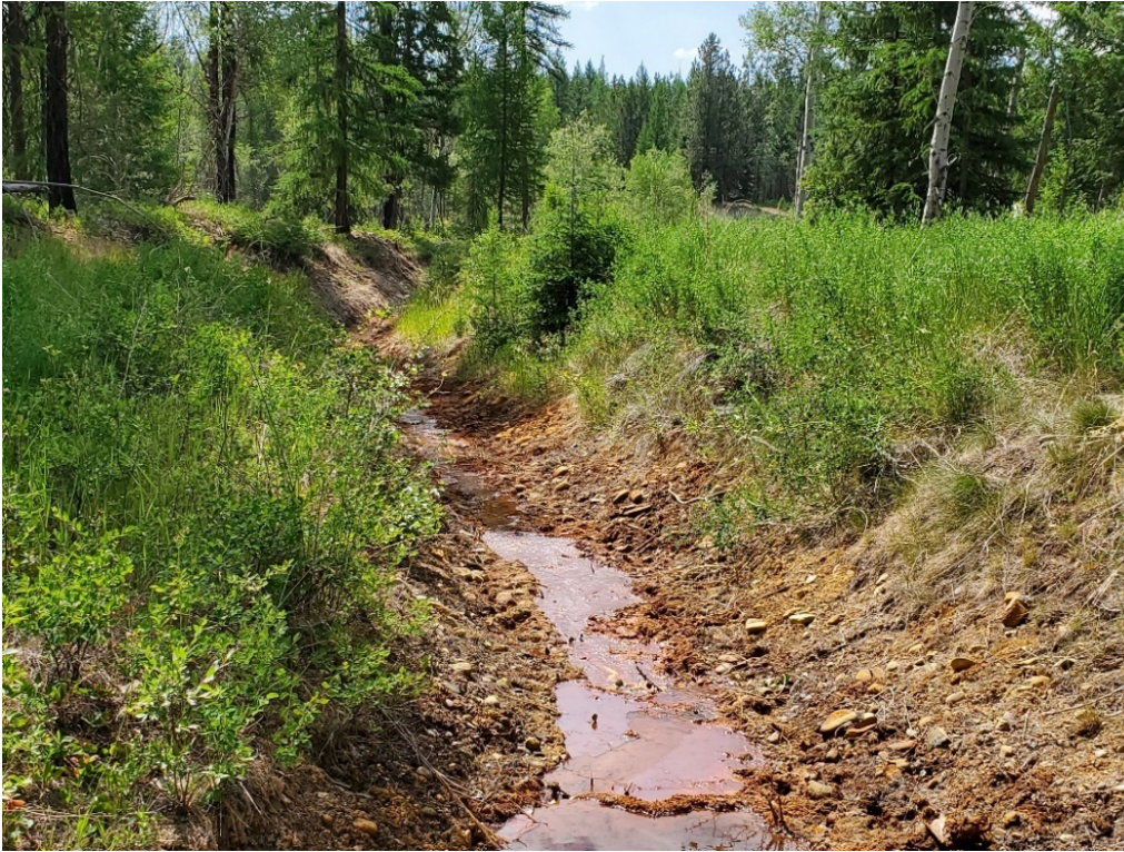
Photo II.26 Siliceous TSF Spillway
