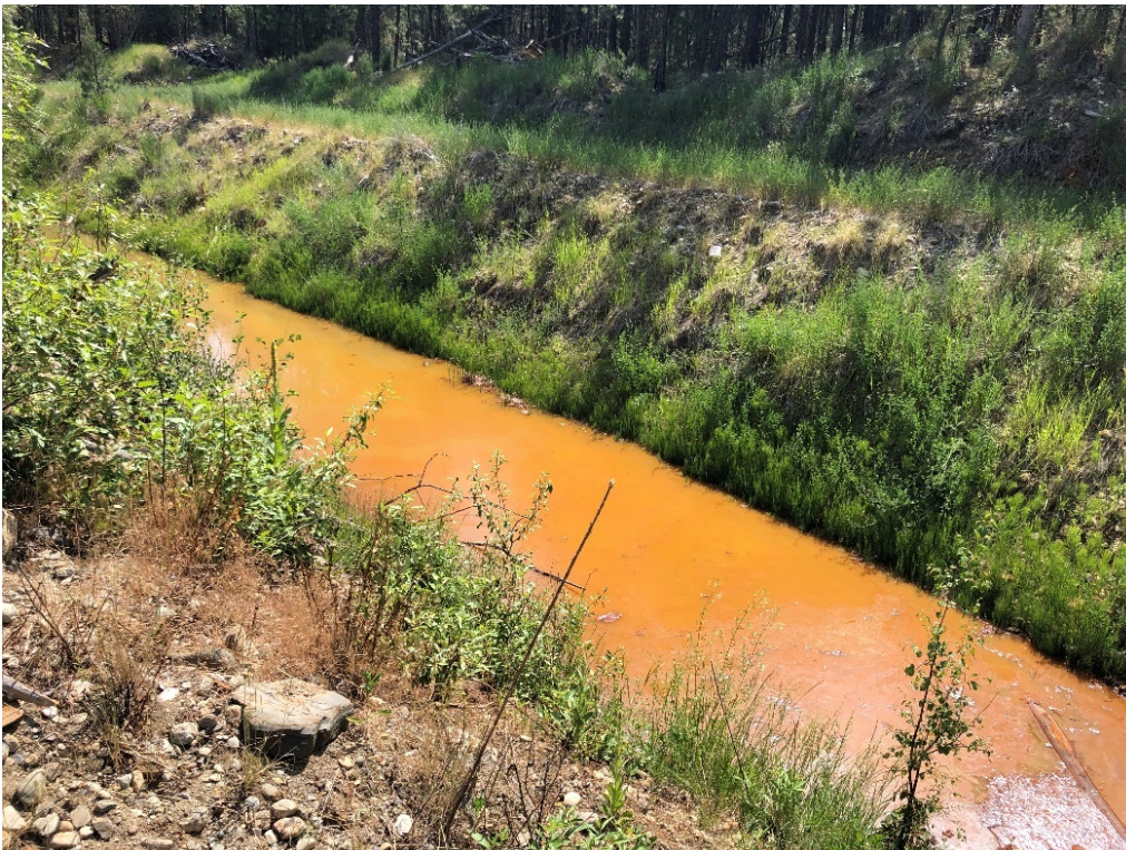
Photo II.24 Seepage downstream of No. 3 Siliceous Dike
