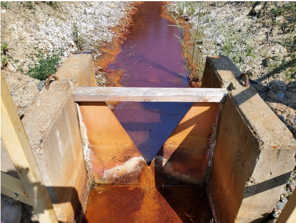
Photo II.16 Weir #4 worn notch
