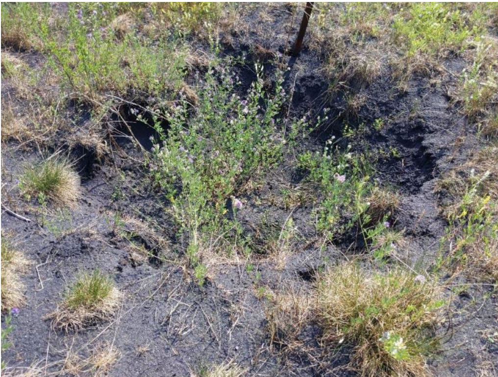
Photo I-9 Sinkhole on the tailings beach (SNTD-2021-06)
