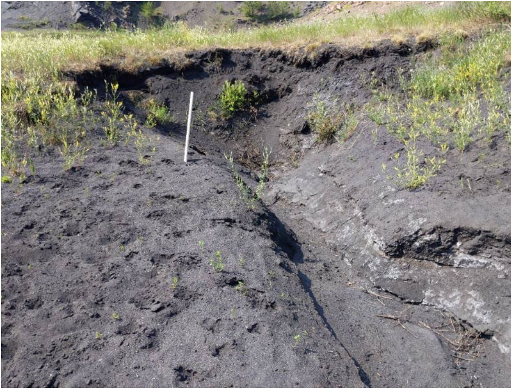
Photo I-9 Sinkhole on the tailings beach (SNTD-2021-06)
