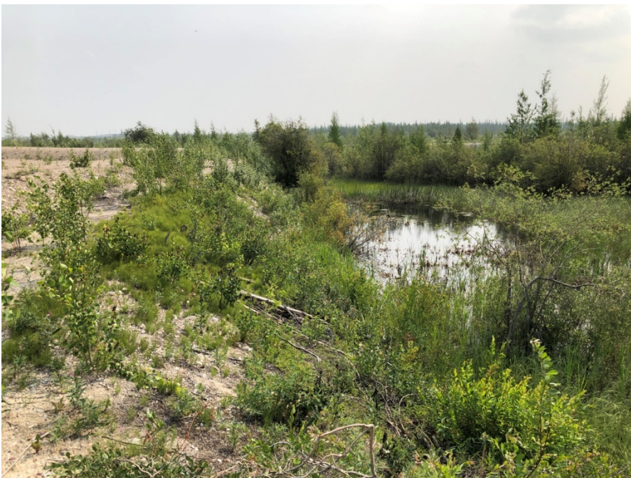
Photo II-10 South Dyke – looking southeast, standing water at downstream toe
