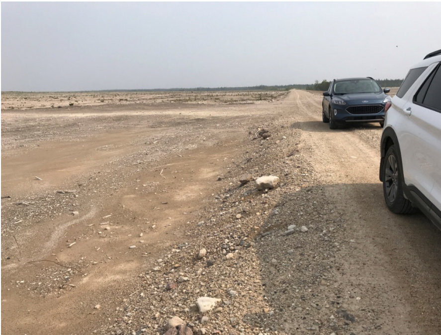
Photo II-6 South Dyke – looking northeast, minor rills on downstream slope
