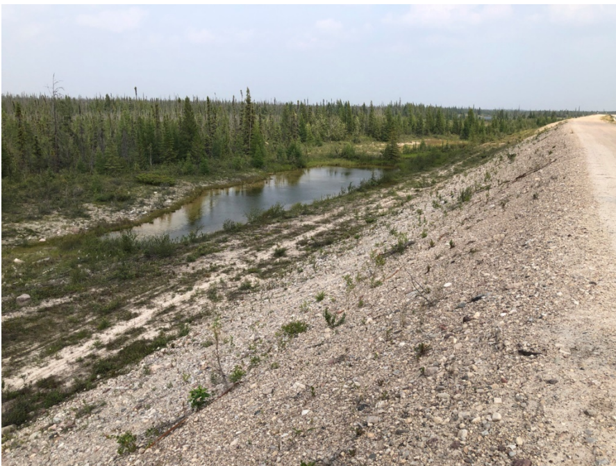
Photo II-24 North Dyke – looking northeast, pond near downstream toe
