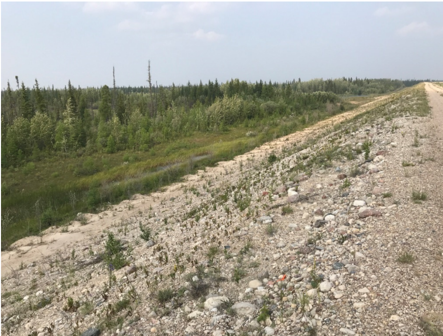
Photo II-16 West Dyke – looking west, seepage and pond downstream of dyke
