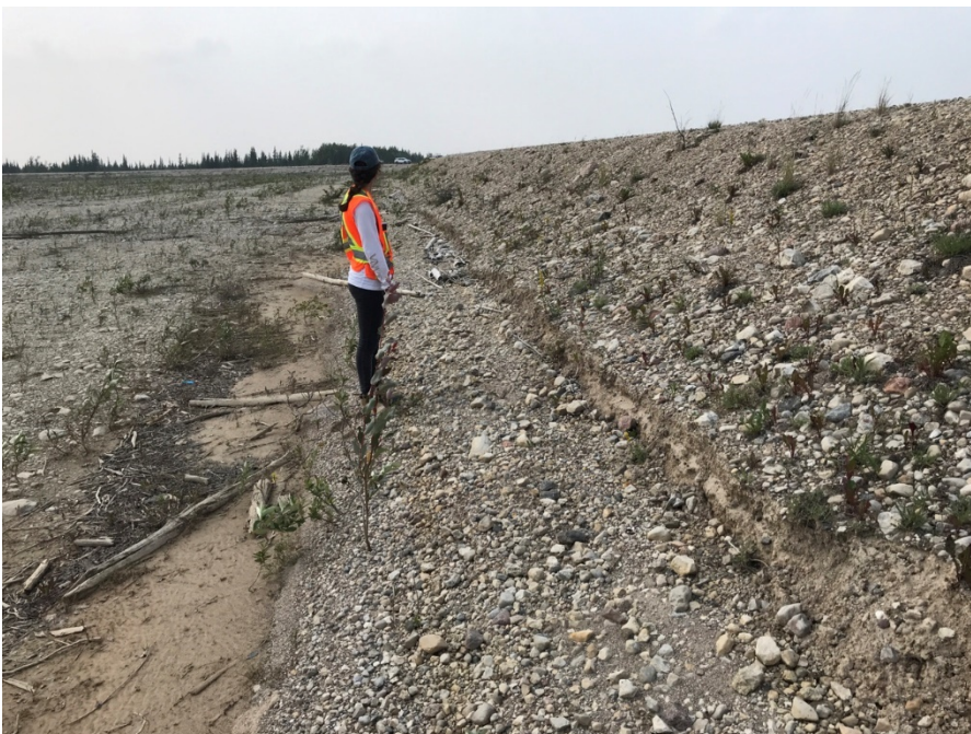
Photo II-20 North Dyke – looking west, slumping and erosion along toe of upstream slope
