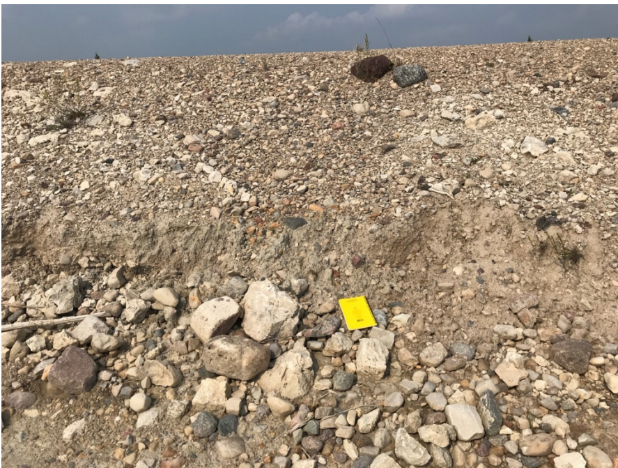
Photo II-26 North Dyke – looking north, slumping and erosion on upstream slope
