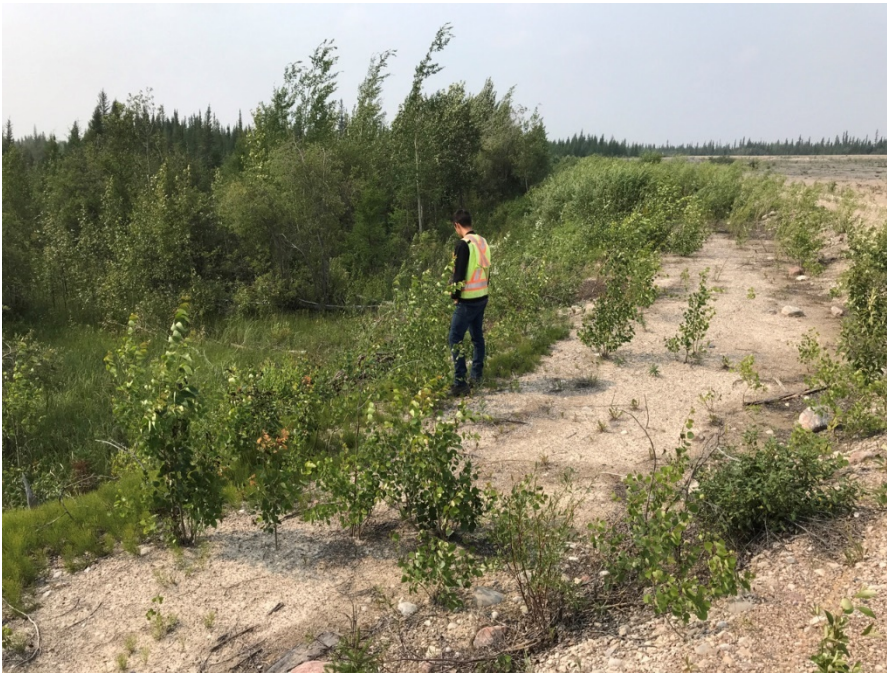
Photo II-12 West Dyke – looking north, minor vegetation on downstream slope
