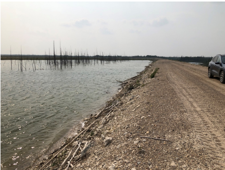
Photo II-22 North Dyke – looking east, minor erosion on upstream slope
