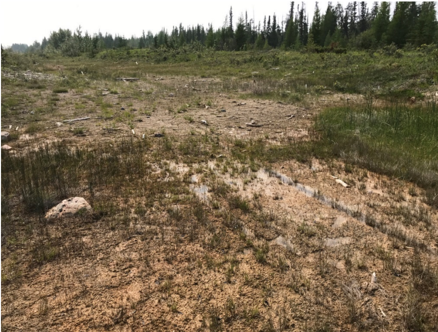
Photo II-14 West Dyke – looking east, erosion of tailings cover
