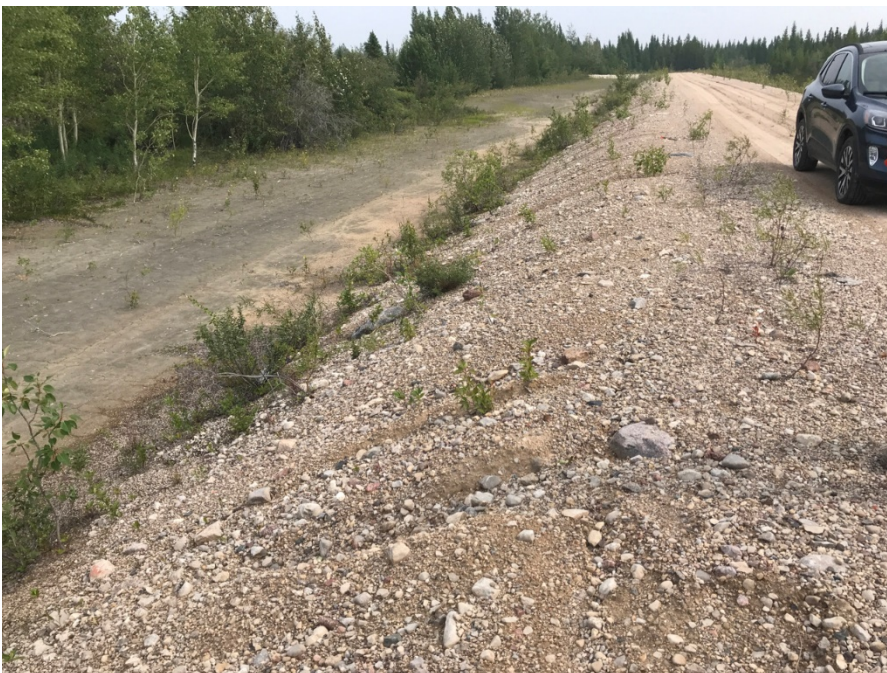
Photo II-2 South Dyke – looking northeast, minor rills on upstream slope, exposed tailings
