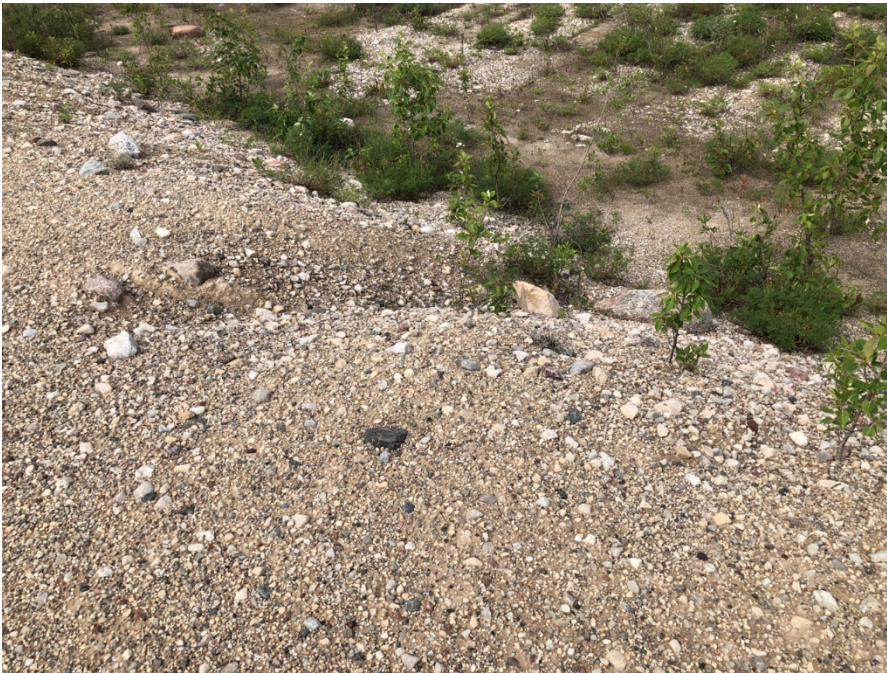
Photo II-4 South Dyke – looking southwest, minor rills on upstream slope
