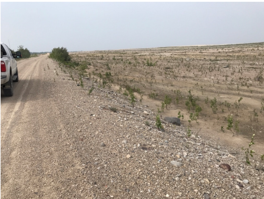
Photo II-4 South Dyke – looking southwest, minor rills on upstream slope
