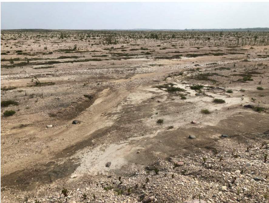
Photo II-14 West Dyke – looking east, erosion of tailings cover
