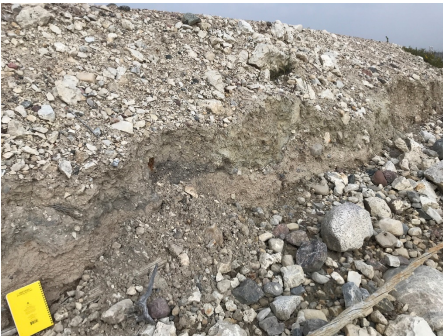
Photo II-28 North Dyke – looking north, slumping and erosion on upstream slope
