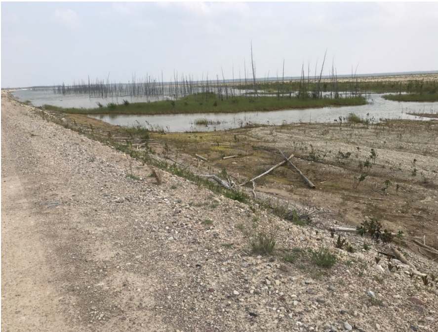
Photo II-20 North Dyke – looking west, slumping and erosion along toe of upstream slope
