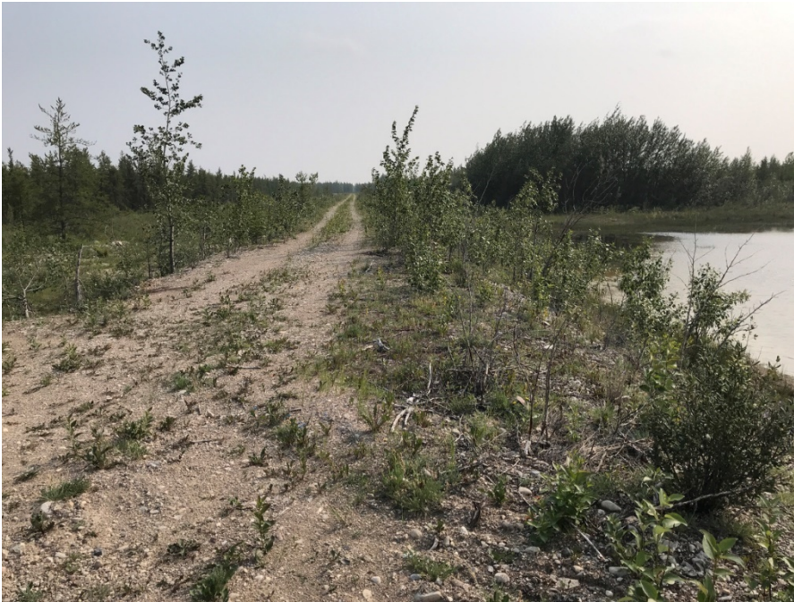
Photo II-30 East Dyke – looking southeast, rill observed on downstream slope
