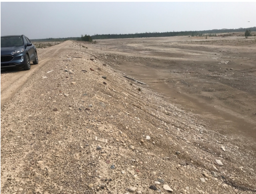
Photo II-6 South Dyke – looking northeast, minor rills on downstream slope
