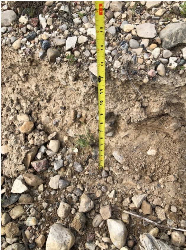
Photo II-22 North Dyke – looking east, minor erosion on upstream slope
