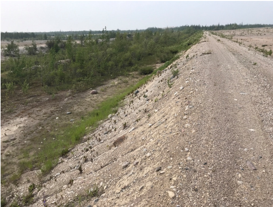
Photo II-8 South Dyke – looking northeast, standing water at downstream toe
