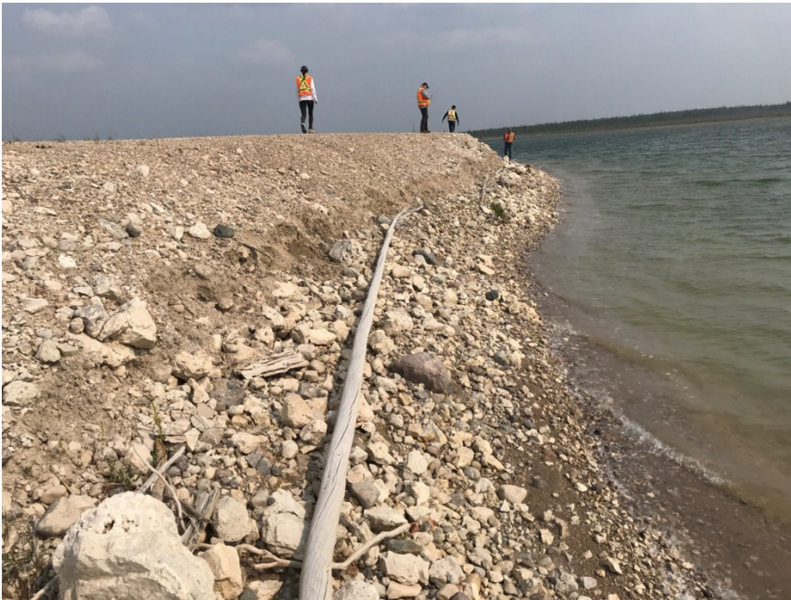
Photo II-26 North Dyke – looking north, slumping and erosion on upstream slope
