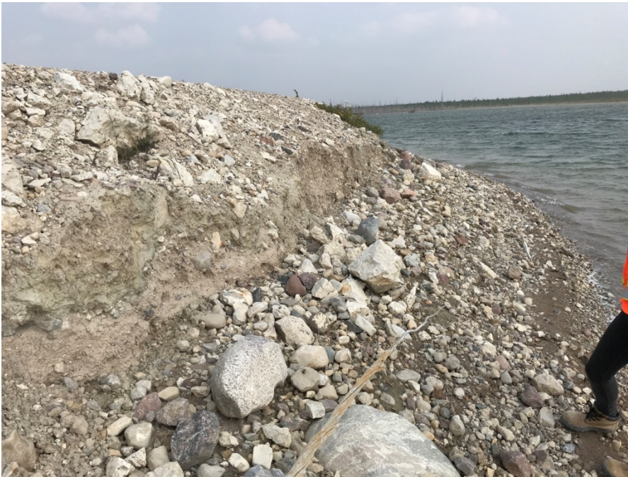
Photo II-28 North Dyke – looking north, slumping and erosion on upstream slope
