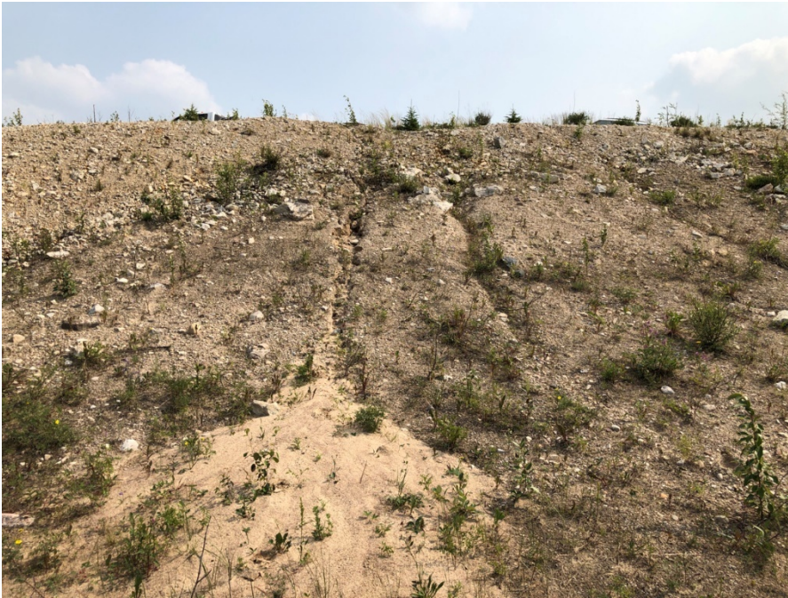
Photo II-18 North Dyke – looking south, minor slope repair on downstream slope
