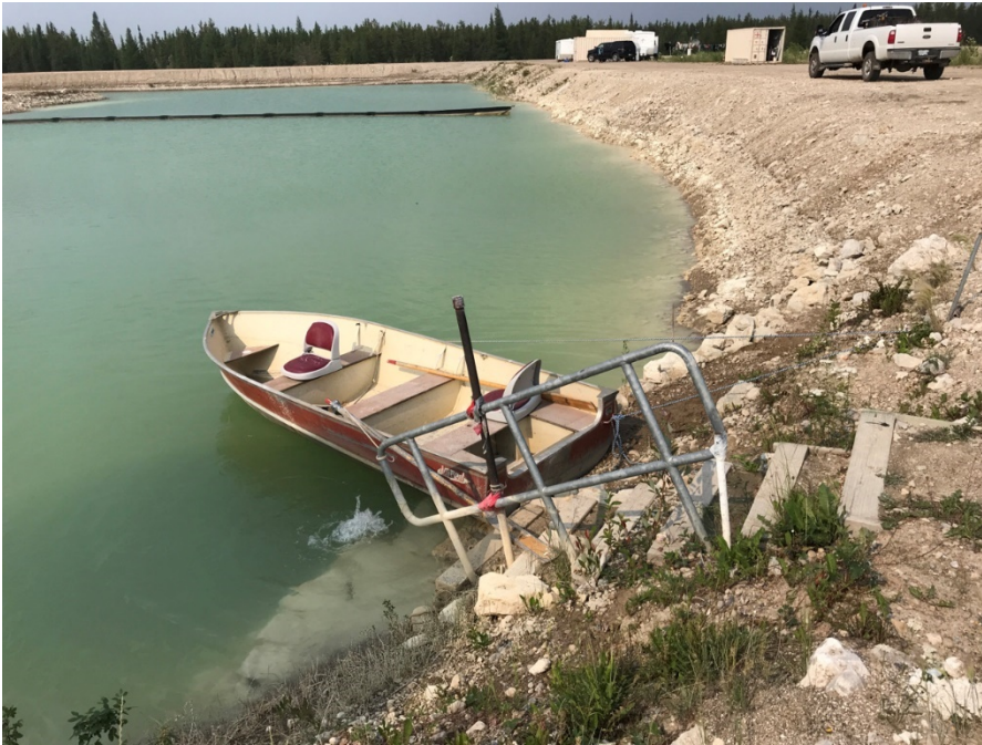
Photo II-34 Polishing Pond – looking southwest, staff gauge flagged for multiple levels
