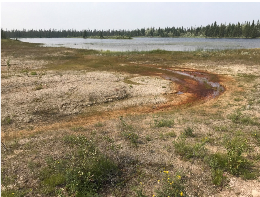
Photo II-16 West Dyke – looking west, seepage and pond downstream of dyke
