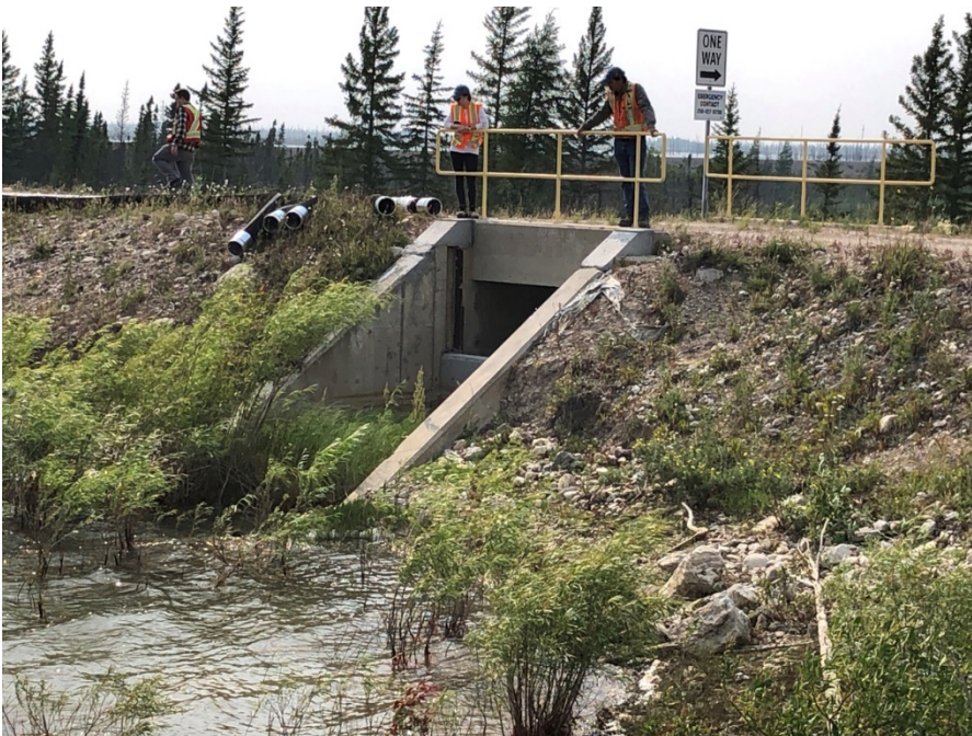
Photo II-32 Main Pond Spillway – looking southwest, erosion and slumping of upstream slope on either side of spillway wing walls
