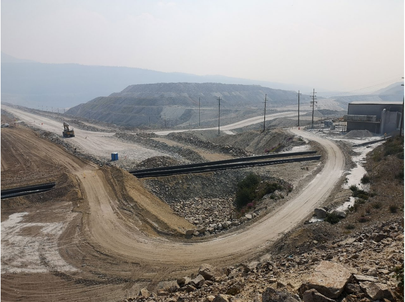
Photo I-B-2 Overview of West Abutment, SS1 pumphouse and where the drain pipelines cross the H-H Dam crest. The pipes have secondary containment berms where they cross the sand and gravel and core zones to prevent overflow onto the crest in the event of pipe breakage. (HH-2021-01)
