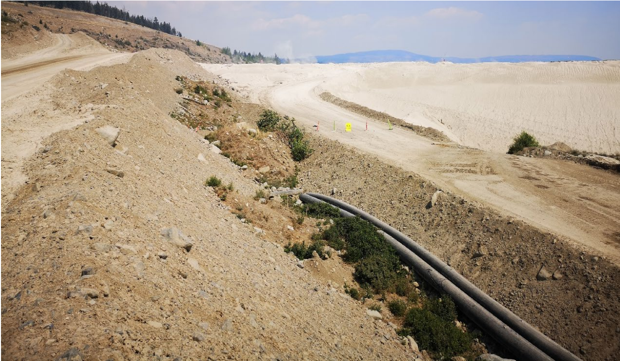
Photo I-A-5 Overview of downstream slope of North Dam U-GLU and Bedrock segments, looking south. North Dam buttress foundation preparation areas visible along toe (LL-2021-03)
