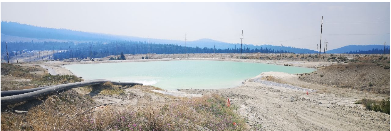
Photo I-A-16 Overview of Sediment Pond 2 which was at typical operating levels and receiving overflow from the VBBE temporary on-dam sediment cell. (LL-2021-06)
