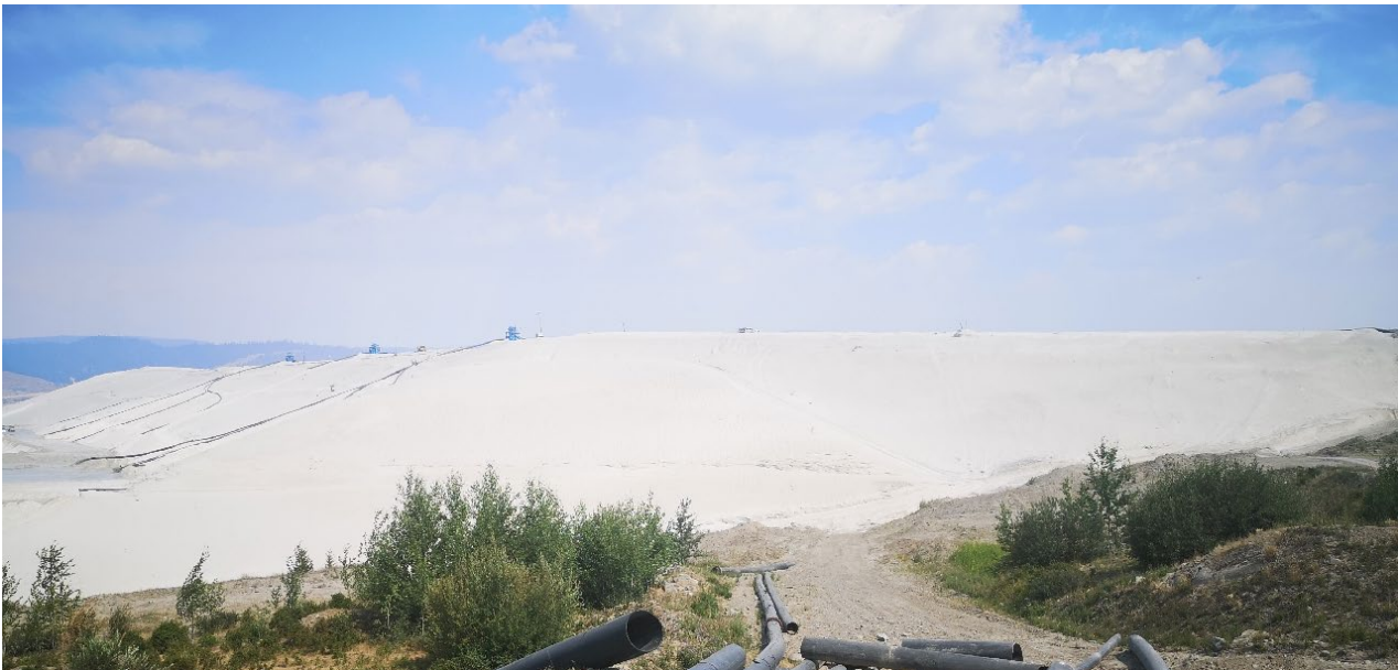
Photo I-A-14 Overview of downstream slope of South Dam and near South Abutment, looking North. No observations of seepage from cycloned sand slope or excessive erosion. (LL-2021-08)
