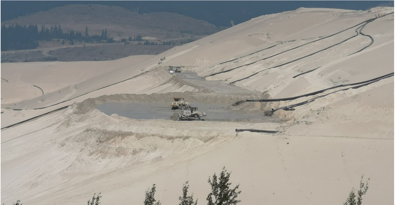
Photo I-A-13 Downstream hydraulic fill placement at the South Dam (LL-2021-08)
