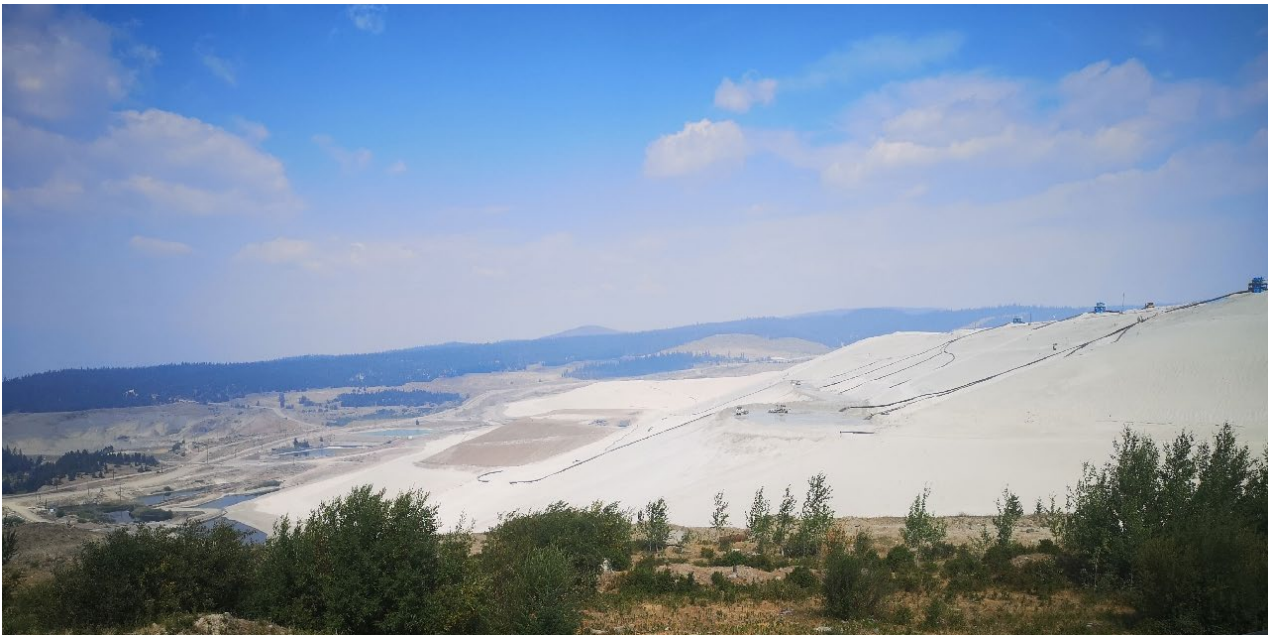
Photo I-A-12 Overview of VBB and South Dam downstream slope and toe area, looking North. Active hydraulic placement to raise South Dam to ultimate downstream slope was in progress during site visit (LL-2021-08)
