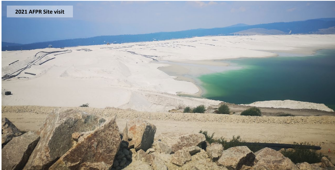
Photo I-A-3 Overview of Tailings Dam beach and crest at South Abutment and upstream of South Dam during 2021 AFPR site visit (top). Similar photo taken during 2020 AFPR site visit (bottom) included to show beach development over past year (LL-2021-02)
