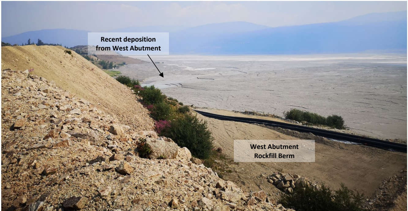
Photo I-B-4 Overview of H-H Dam eastern downstream slope. The light colour area of the slope is where Bethsaida sand was placed in the dam shell earlier in the mine life. Bethsaida sand does not meet the current fill placement specification for the downstream shell but this zone of material has been accounted for in the design. (HH-2021-03)
