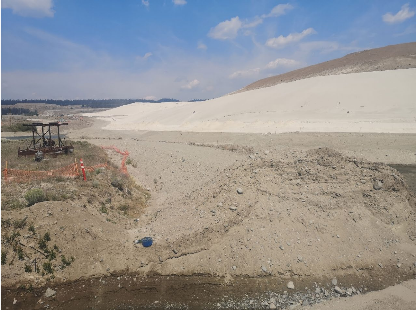
Photo I-A-9 Downstream toe of the VBB with no visible seepage from cycloned sand fill above underdrain, looking north. Sediment Pond 1 present along dam toe, as well as internal sand and gravel berms which prevent sediment from encroaching on archeologically sensitive native ground. (LL-2021-07)
