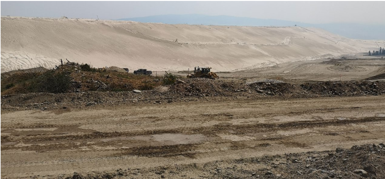
Photo I-A-5 Overview of downstream slope of North Dam U-GLU and Bedrock segments, looking south. North Dam buttress foundation preparation areas visible along toe (LL-2021-03)
