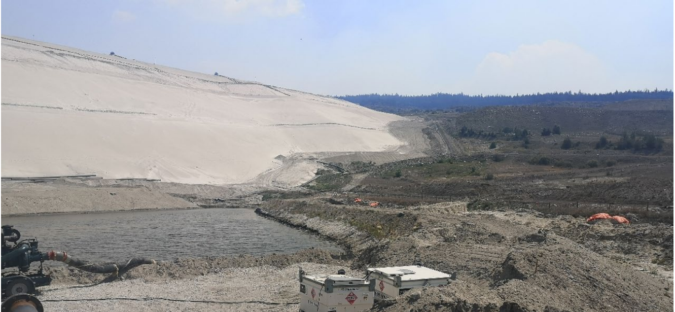
Photo I-A-12 Overview of VBB and South Dam downstream slope and toe area, looking North. Active hydraulic placement to raise South Dam to ultimate downstream slope was in progress during site visit (LL-2021-08)
