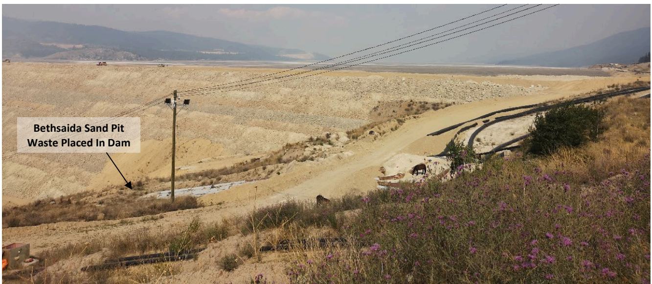
Photo I-B-4 Overview of H-H Dam eastern downstream slope. The light colour area of the slope is where Bethsaida sand was placed in the dam shell earlier in the mine life. Bethsaida sand does not meet the current fill placement specification for the downstream shell but this zone of material has been accounted for in the design. (HH-2021-03)
