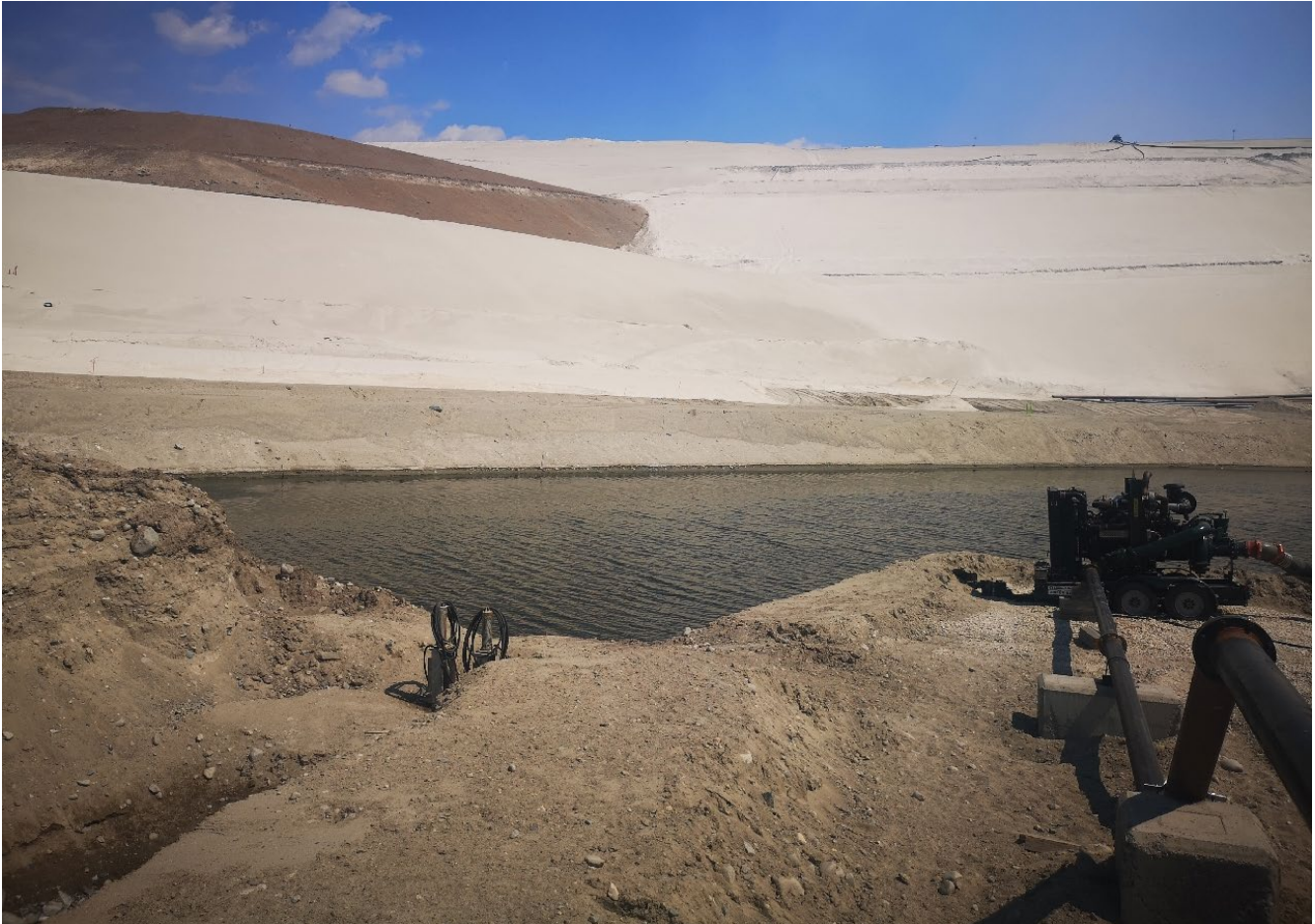
Photo I-A-10 Overview of VBB downstream slope with Sediment Pond 1 (south cell) at dam toe, looking east. Secondary pump added to increase reclaim capacity from SWRP visible in foreground. (LL-2021-07)
