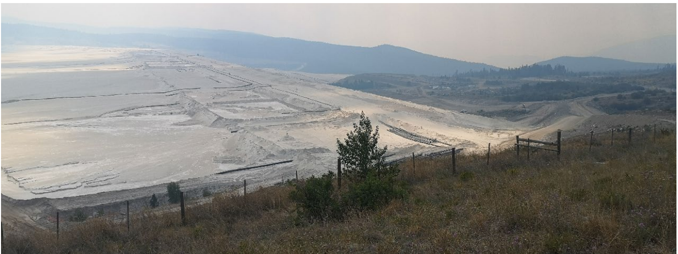
Photo I-A-2 Overview of Tailings Beach and upstream cycloned sand hydraulic placement cells at North Dam U-GLU (LL-2021-01)
