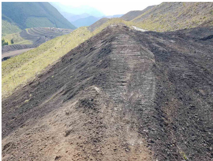
Photograph 19b: Site B CCR Facility – Repair of Erosion on Intermediate Bench at East Side of Facility; Looking South, 19 October 2021
