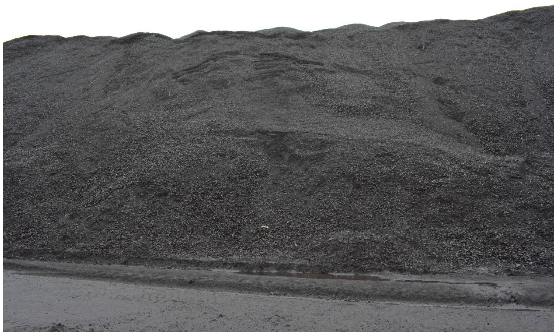
Photograph 21: Site B CCR Facility – Surficial Cracking at Overbuilt Portion of Slope at Northeast Side of Facility; Looking East, 17 August 2021
