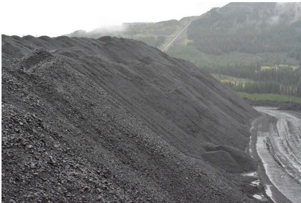
Photograph 20: Site B CCR Facility – Overbuilt Portion of Slope at Northeast Side of Facility; Looking East, 17 August 2021
