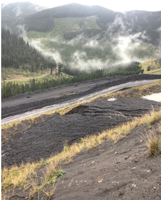
Photograph 19a: Site B CCR Facility – Erosion of Intermediate Bench at East Side of Facility; Looking Southeast, 17 August 2021
