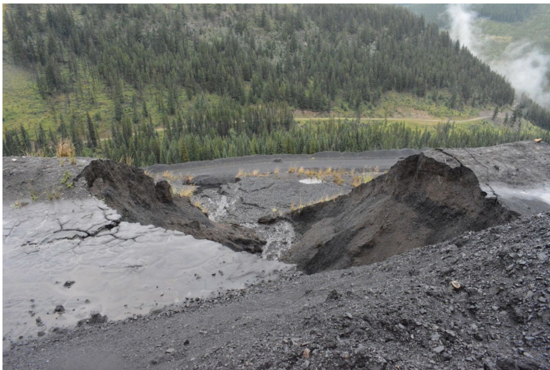
Photograph 18: Site B CCR Facility – Close-Up View of Erosion at East Slope; Looking East, 17 August 2021
