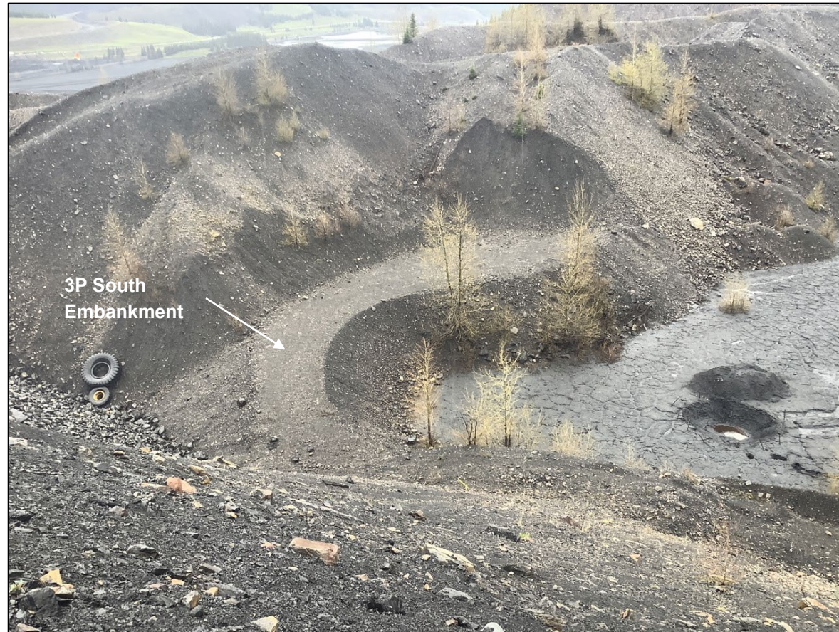
3 Pit South Desiccated Tailings Surface and Moist Conditions (from Rain) Observed in Test Pit Upstream of 3 Pit South Embankment, 3 Pit South Embankment Crest, Upstream, and Downstream Slope, Looking Southeast
