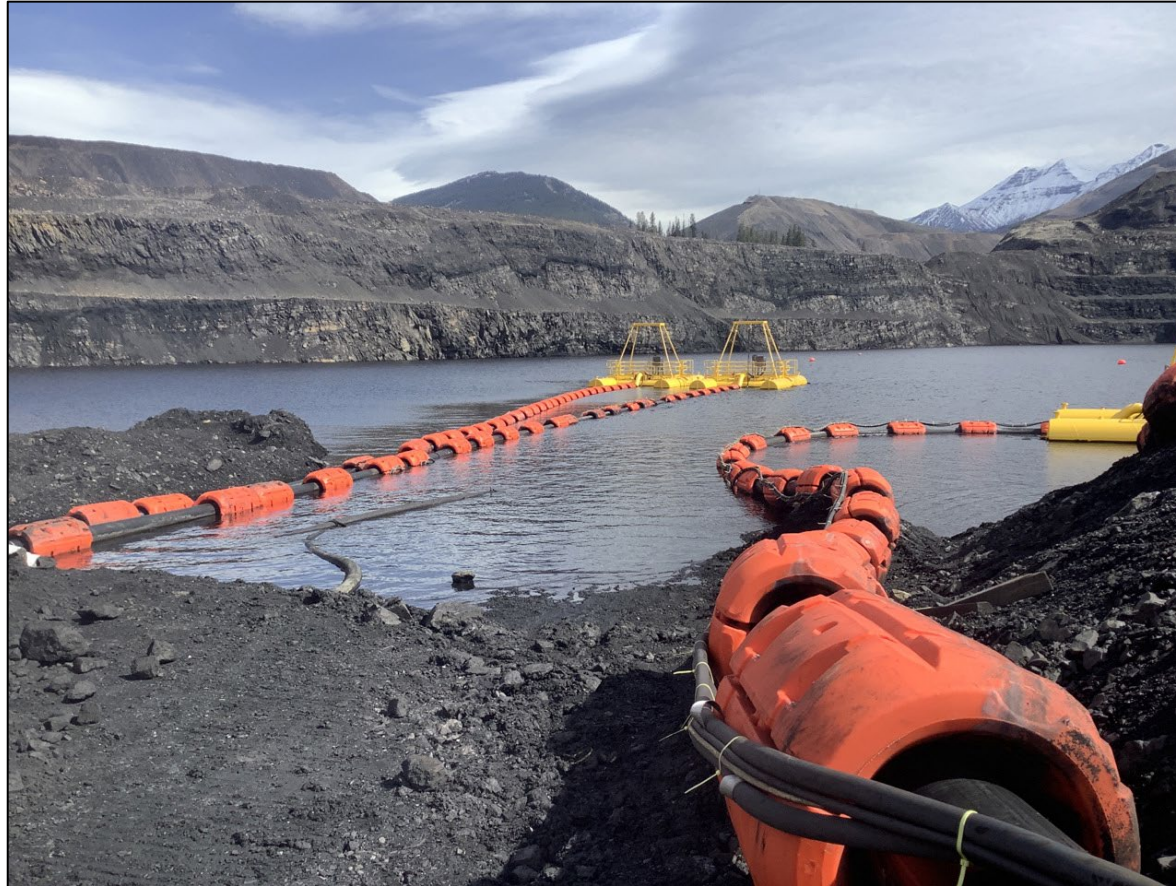
Turnbull TFS Pond, reclaim water intakes and pipelines, looking northeast.
