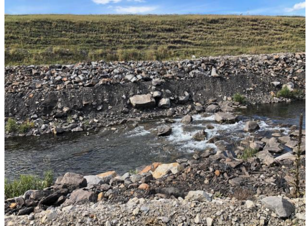
Photo 6: Looking at erosion of the gravel material placed on top of the riprap at one of the riffle crest bank tie-ins on the NTP (approx. Sta. 0+550)
