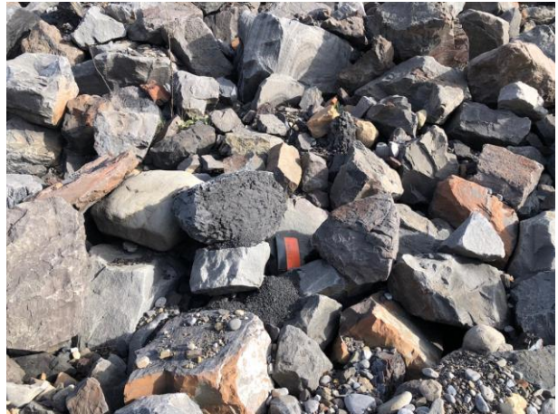
Photo 10: Riprap degradation due to weathering on several pieces of riprap
