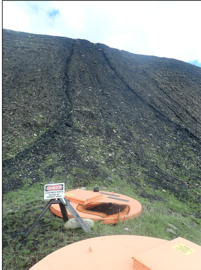
STP Main Dam downstream slope, erosion above well, looking northwest from approximately Sta. 1+400.
