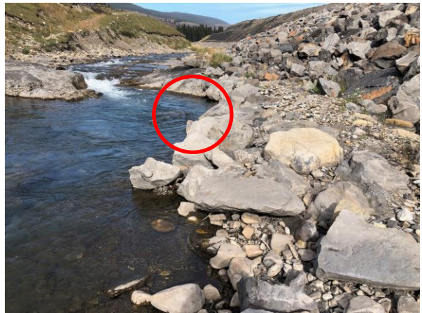
Photo 12: Erosion along the toe apron of the STP riprap at Sta. 0+670
