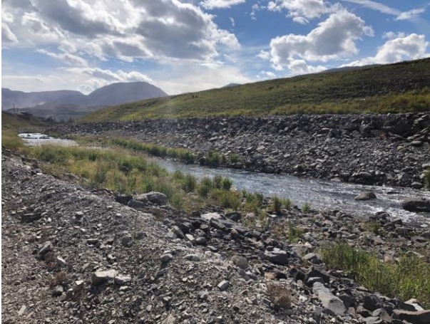
Photo 5: Looking downstream at NTP riprap (from approx. Sta. 0+350)
