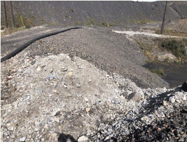
Photo 1: Looking upstream along alignment of NTP riprap that is buried (approx. Sta. 0+125)
