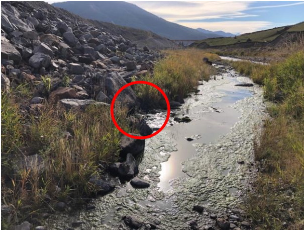
Photo 9: Looking downstream at STP riprap and where water is flowing out of riprap apron (approx. Sta. 0+365)
