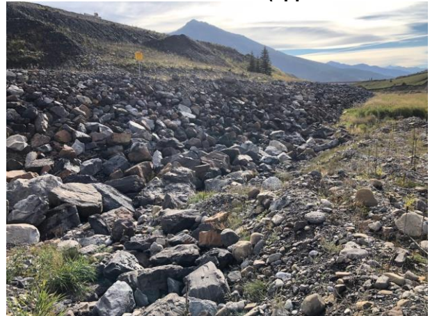
Photo 8: Looking downstream at STP riprap that is over-steepened (1.5H:1V) (from approx. Sta. 0+270)
