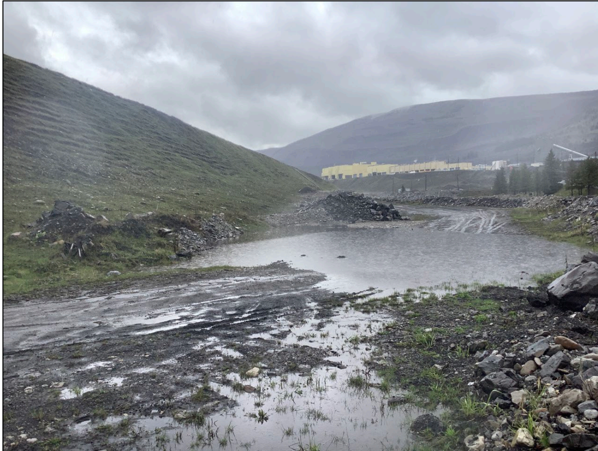
NTP Dam toe and area of ponding after rain events near at Sta. 1+250, looking northeast.
