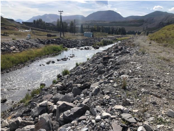
Photo 7: Looking downstream at NTP riprap (from approx. Sta. 0+705)
