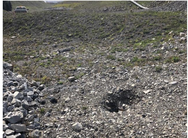
Photo 2: Small sinkhole about 0.9 by 0.6 m at approx. Sta. 0+140. This is along the alignment of the buried setback riprap
