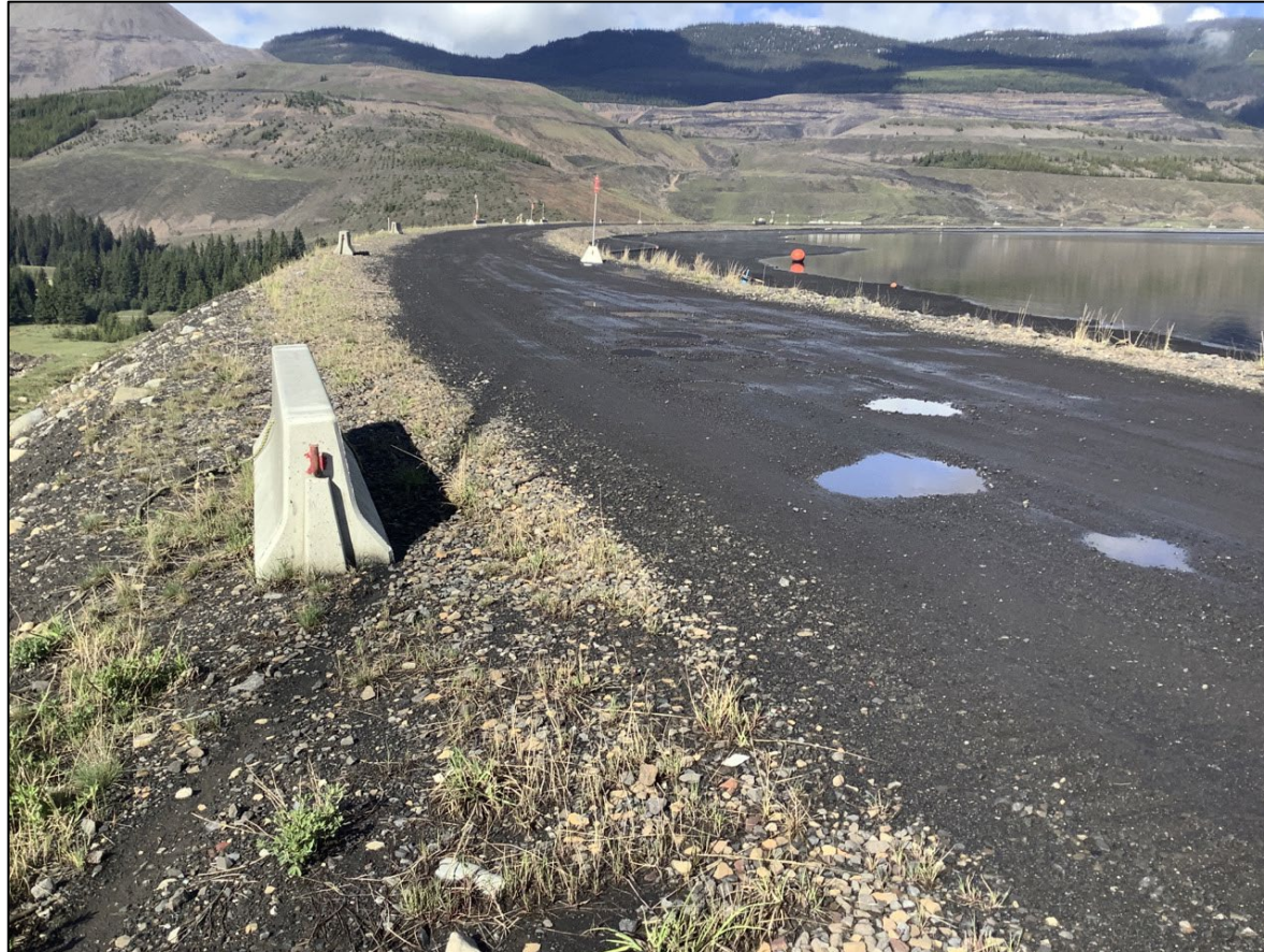
STP Main Dam crest, downstream slope, and tailings beach, looking southwest from approximately Sta. 1+650.
