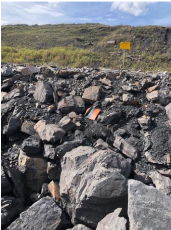
Photo 3: Riprap degradation due to weathering on several pieces of riprap along NTP (Sta. 0+225)
