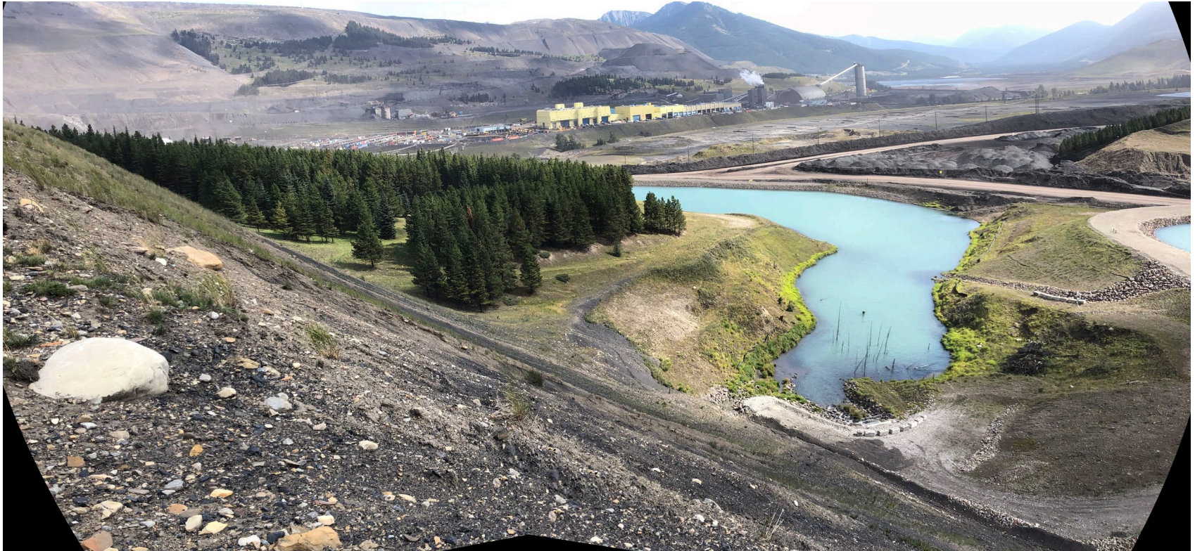
A-Spoil - South side on angle of repose slope above Liverpool Settling ponds, looking south
