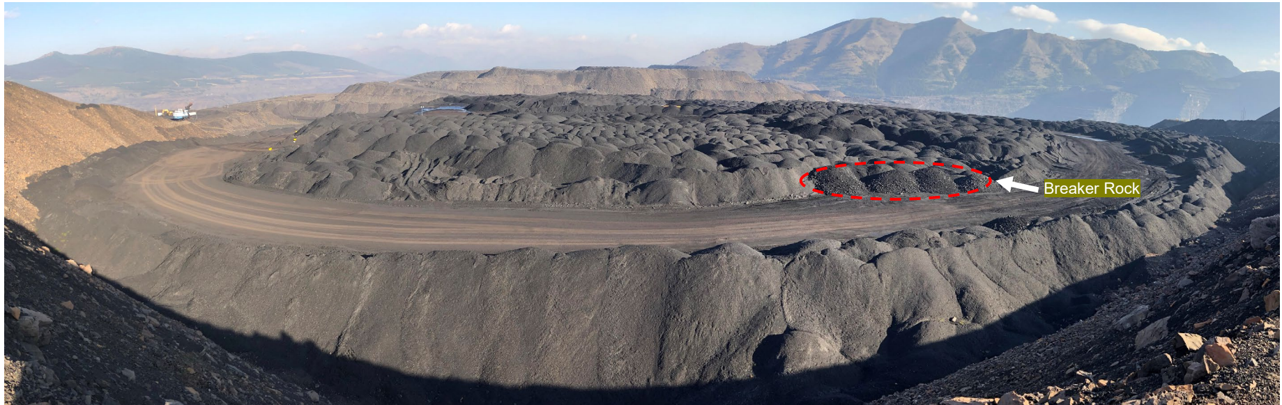
Eagle 4 South Backfill spoil - Overview, looking north
