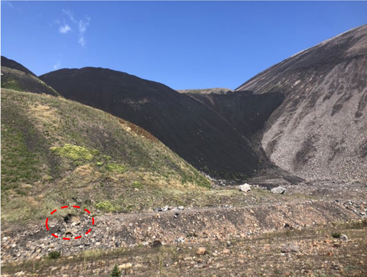
Kilmarnock / Toe Berm spoil - new erosion feature (shown in red) due to water seepage from Old South spoil, looking north
