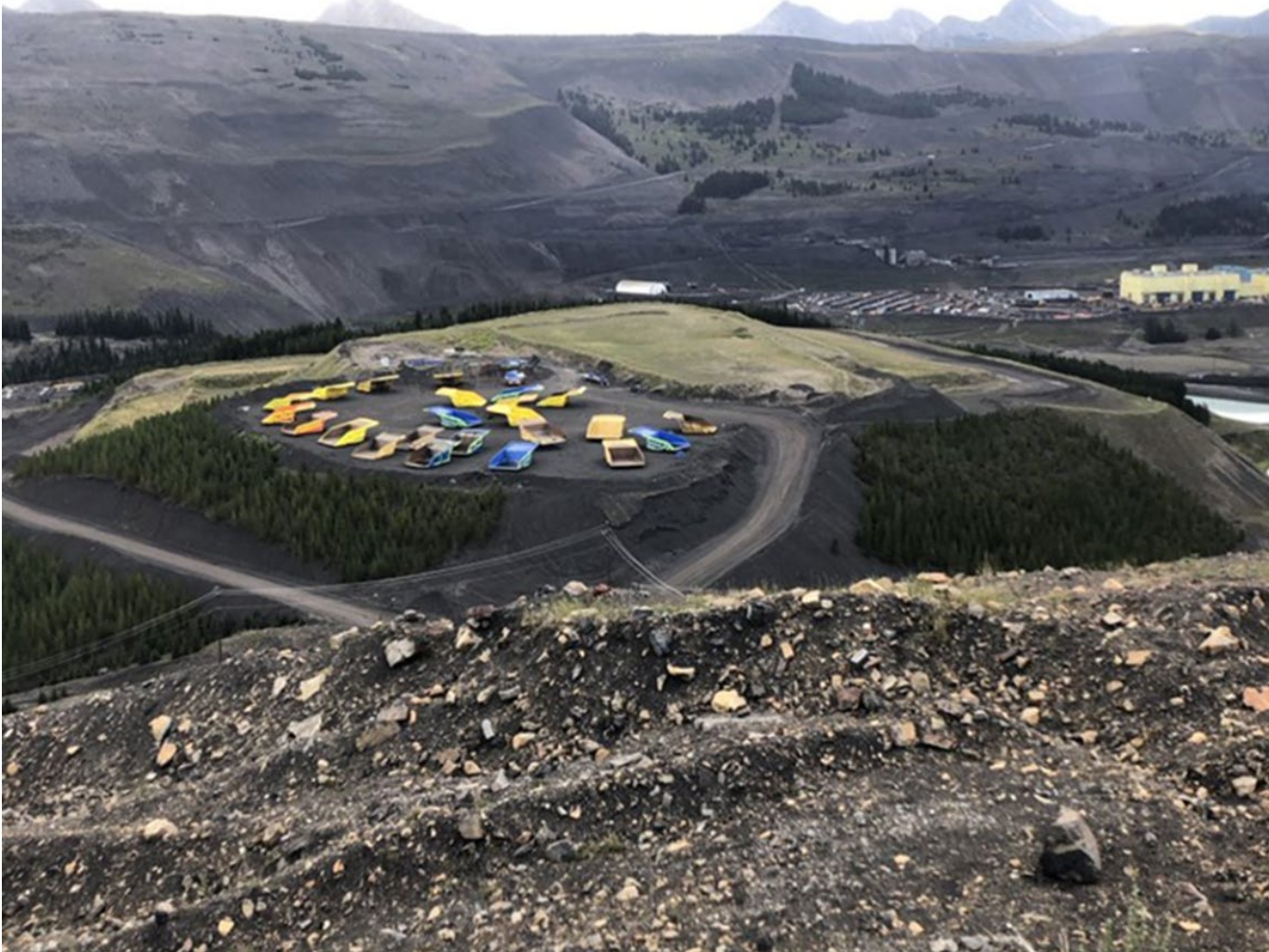
A-Spoil - Overview of crest including new shovel yard constructed in 2020/2021, looking east
