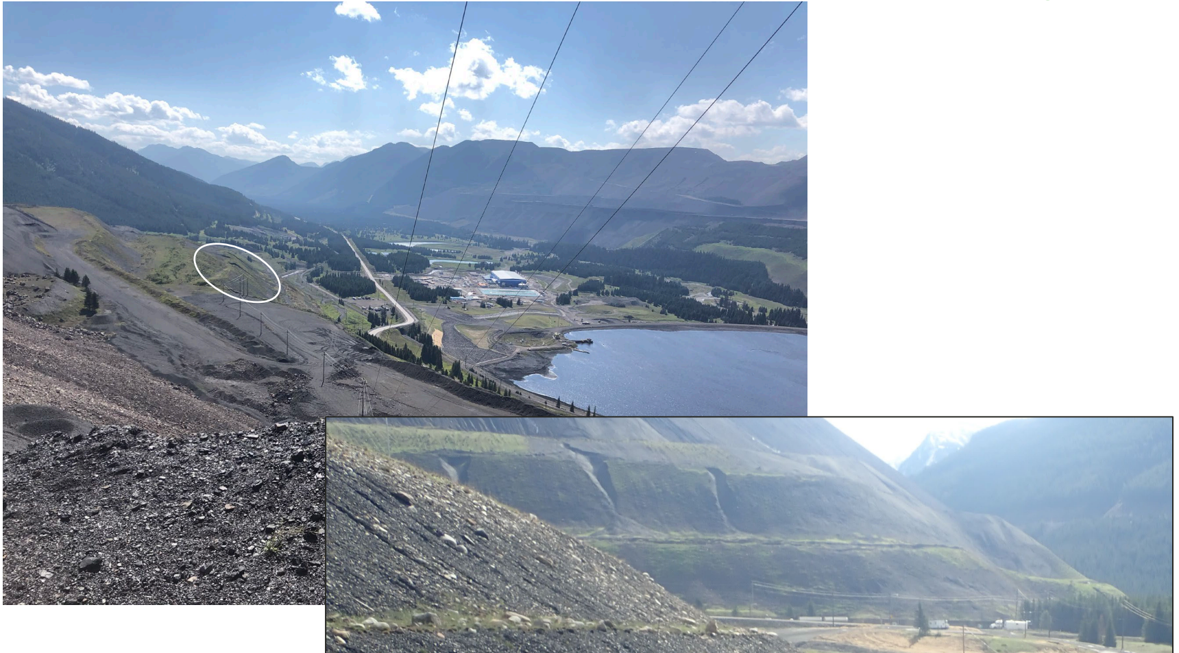
Kilmarnock /Toe Berm spoil - erosion gullies from the 2013 flood, looking south from Blake spoil (top left) and looking east from the South Tailings Pond (bottom right)
