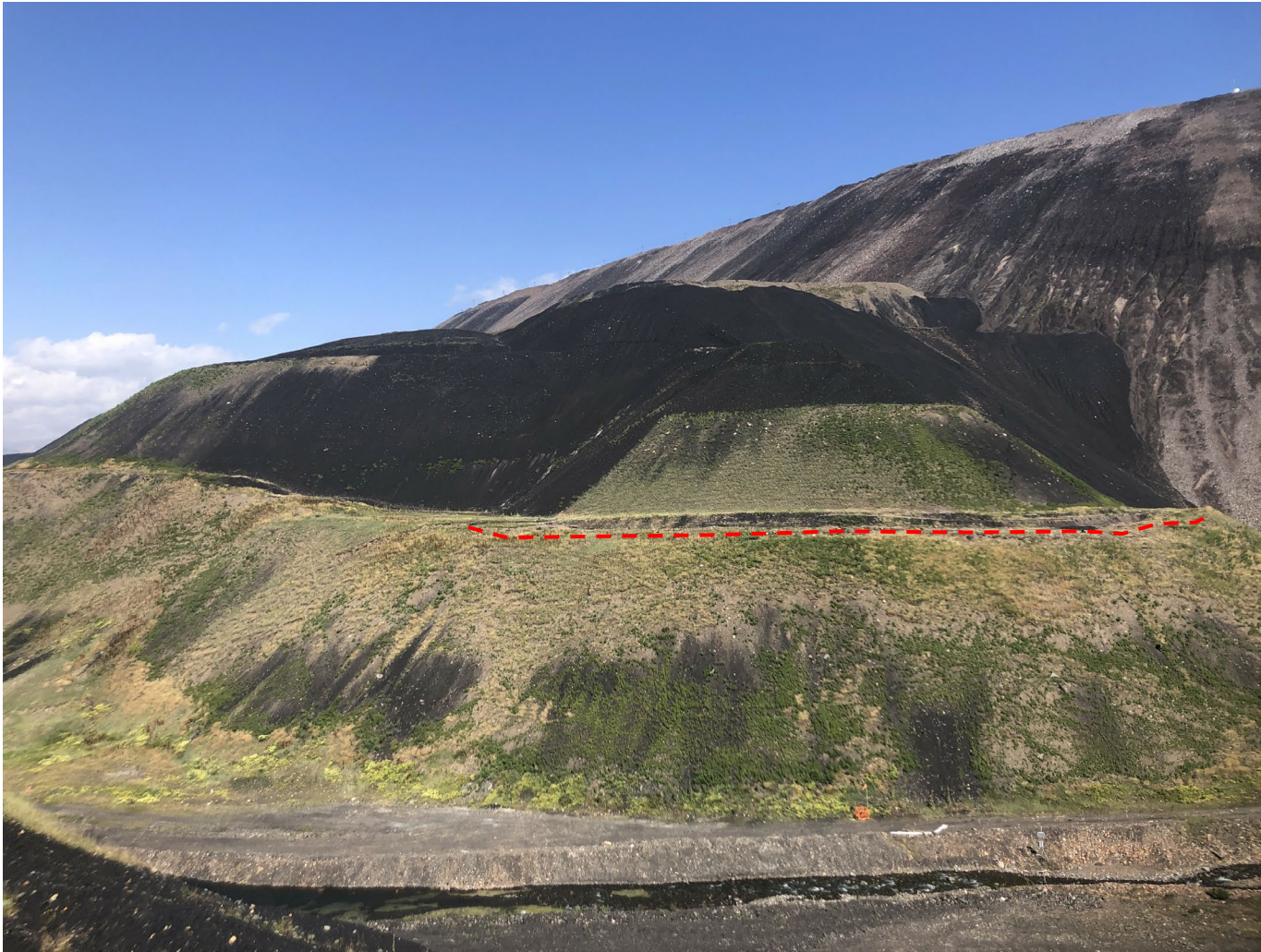
Kilmarnock /Toe Berm spoil - overview, crest settlement noted in red, looking north
