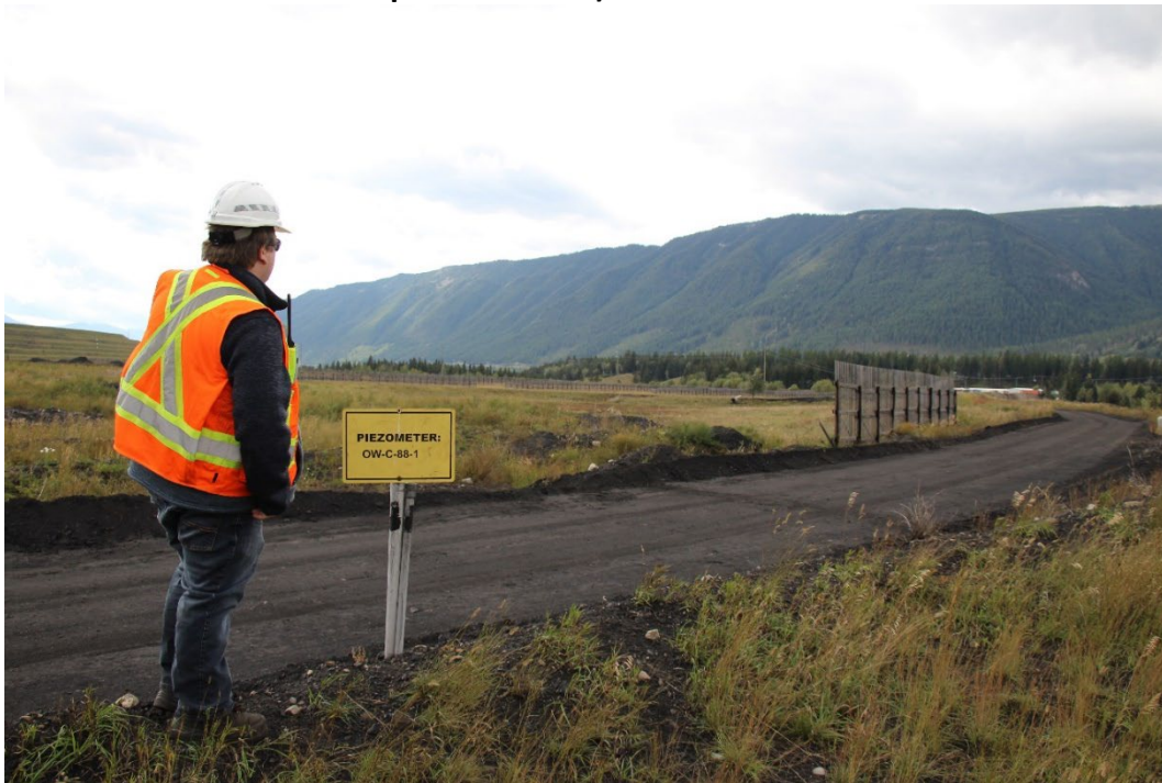
Photo IC-3 Lagoon C typical crest typical condition with piezometer OW-C-88-1. (Looking SW – Taken 15 September 2021)
