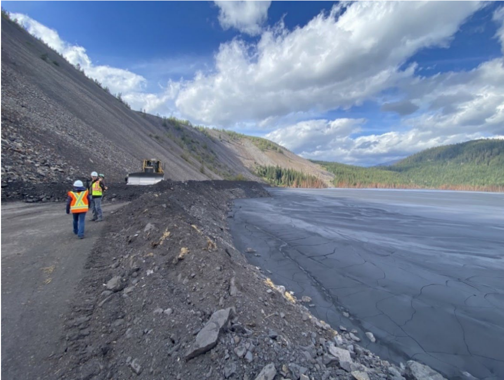
Photo IW-8 WFTF Adit Dump erosion above Adit Filter Berm. (looking west – Taken 15 September 2021)
