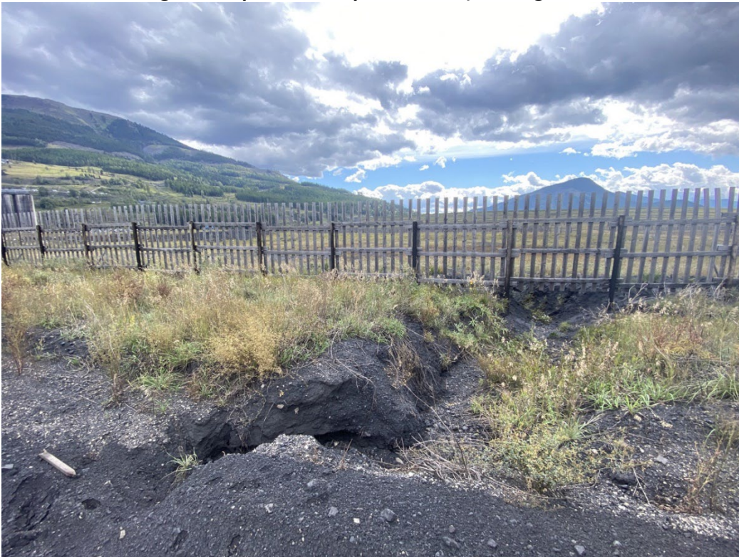
Photo IC-10 Lagoon C upstream slope erosion. (Looking South – Taken 15 September 2021)
