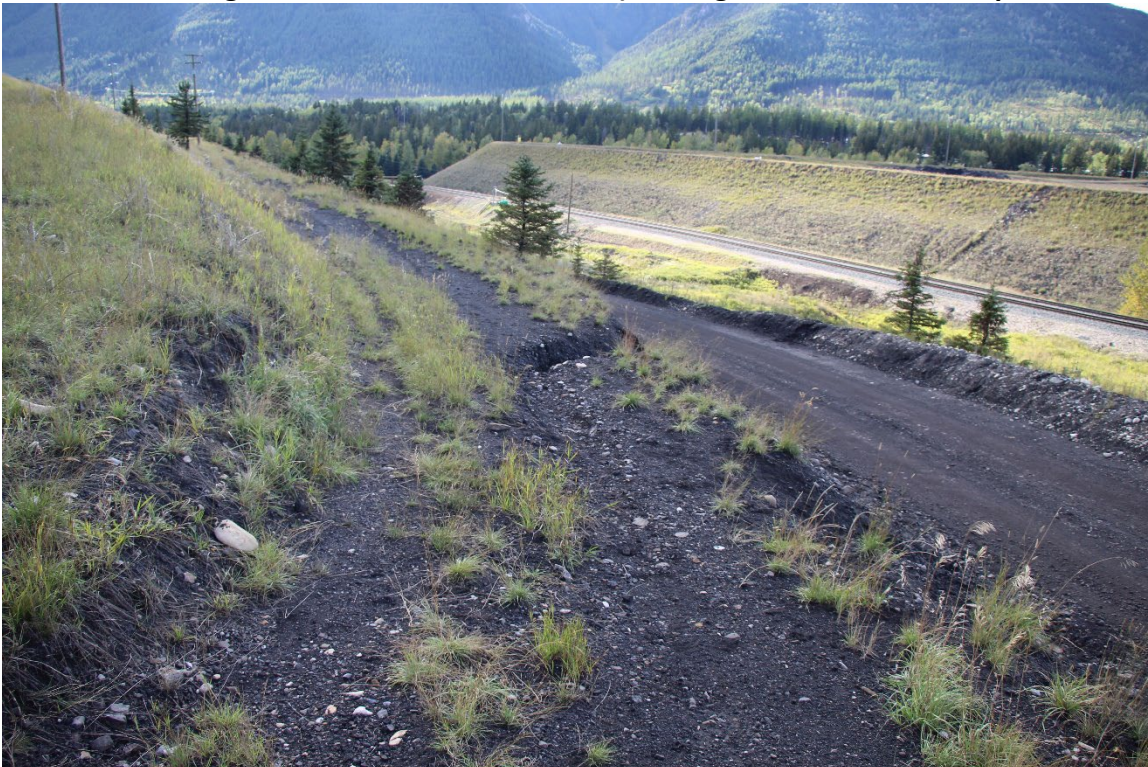
Photo ID-10 Lagoon D bench minor erosion. (Looking West – Taken 16 September 2021)
