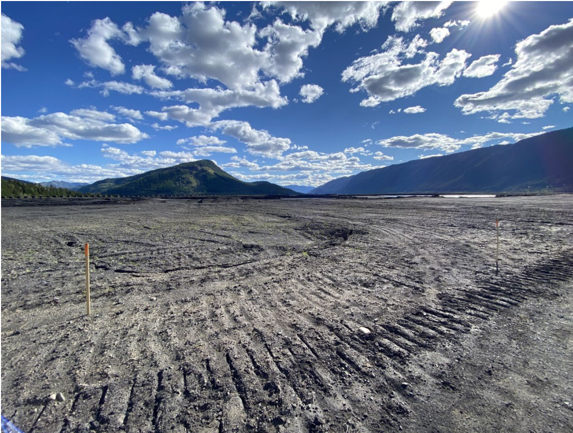
Photo ID-13 Lagoon D minor subsidence of backfilled north tailings cell. (Looking SW – Taken 16 September 2021)
