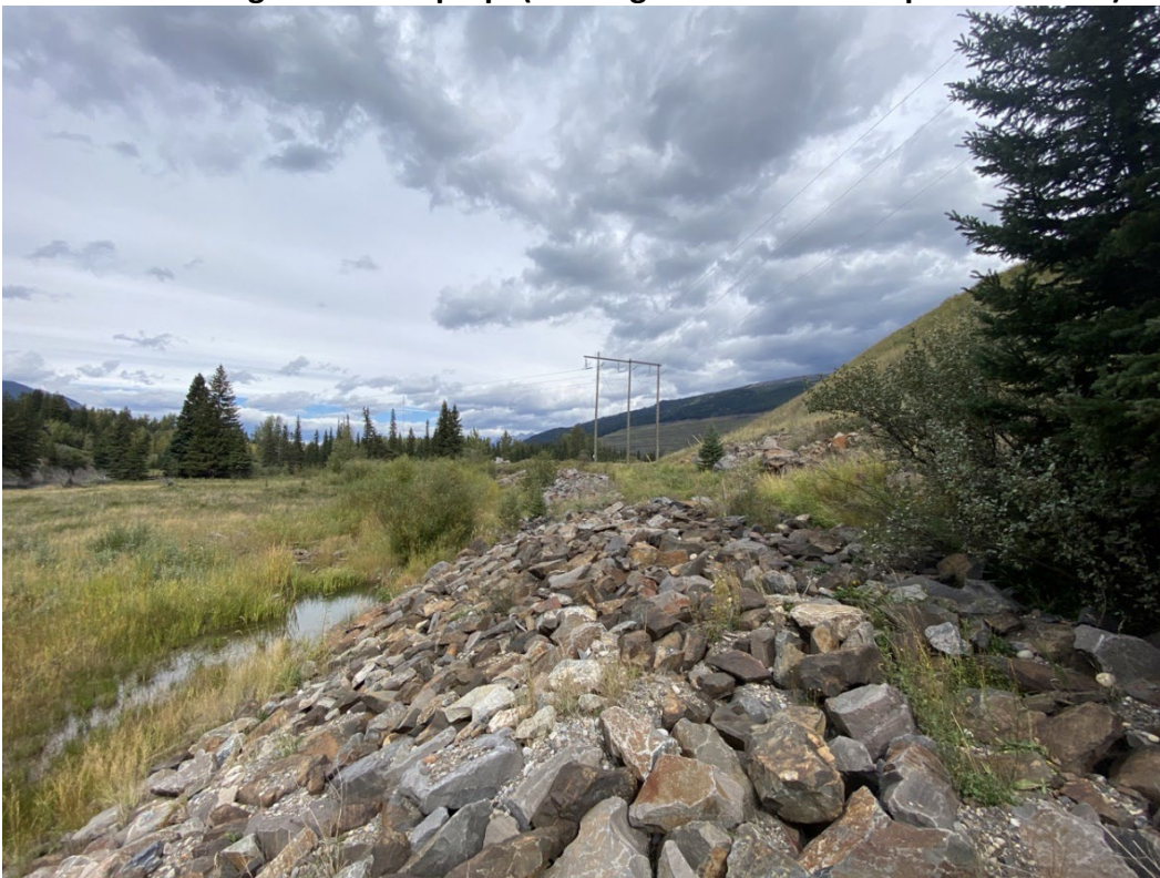
Photo IC-8 Lagoon C toe riprap. (Looking NE – Taken 15 September 2021)
