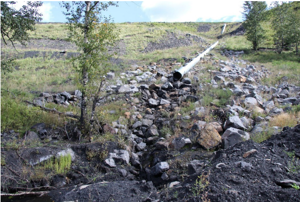
Photo I-12 CCR Dump Bench Erosion. (Looking SW – Taken 16 September 2021)
