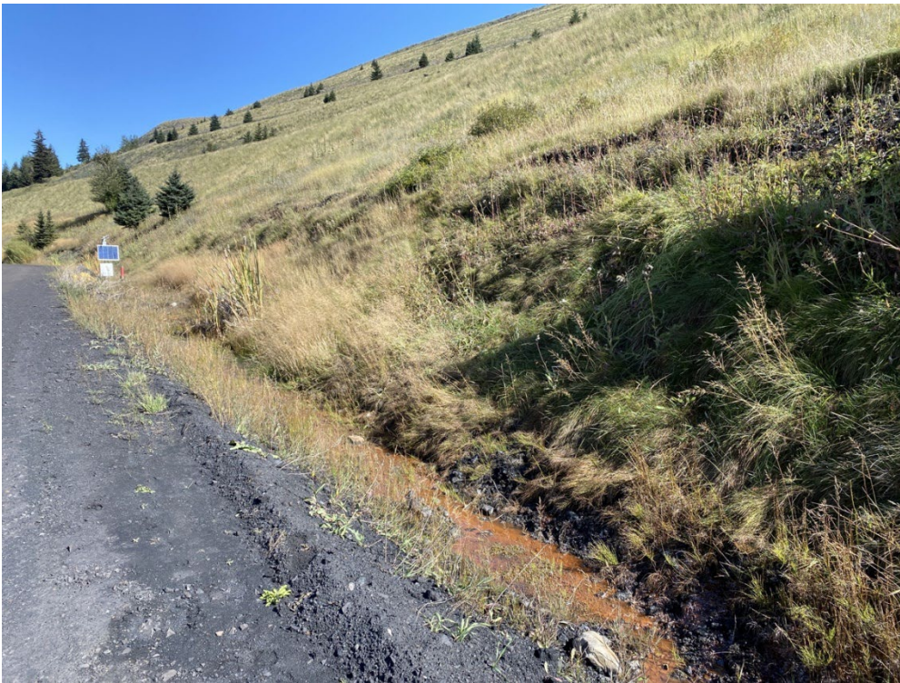
Photo I-8 CCR Dump natural hillside wet spot. (Looking South – Taken 16 September 2021)
