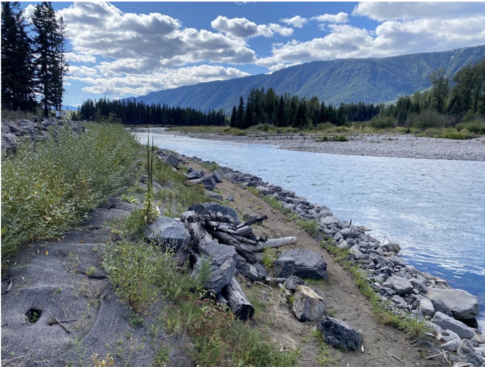
Photo I-16 CCR Dump toe riprap adjacent to the Elk River (Looking South – Taken 16 September 2021)
