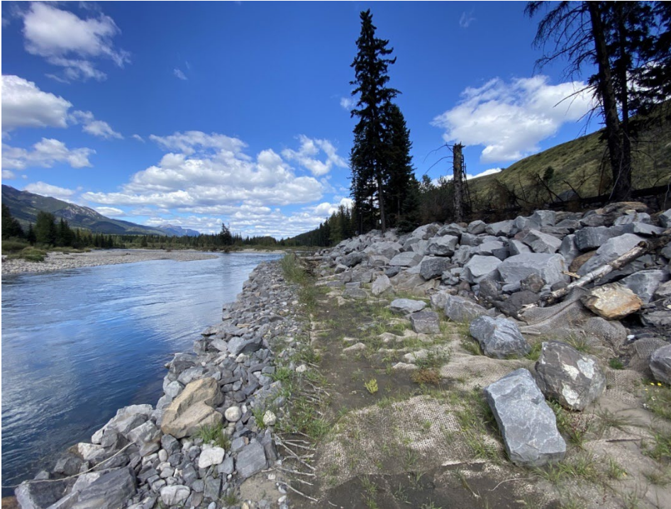
Photo I-16 CCR Dump toe riprap adjacent to the Elk River (Looking South – Taken 16 September 2021)
