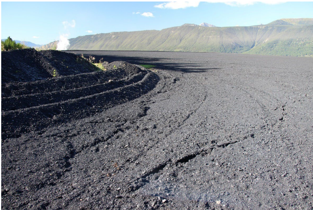
Photo I-14 Surficial cracks at the CCR dump. (Looking SW – Taken 16 September 2021)
