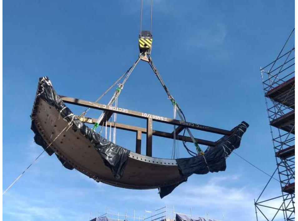
SAG Mill #1 Shell Lift, January 2020
