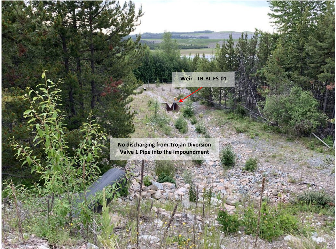
Photo I-A-23 No scour was observed at Trojan Diversion Valve 1 pipe discharge point (TRJ-2020-18)
