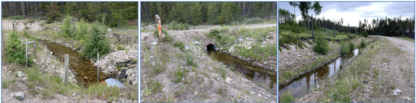
Photo I-A-22 Trojan Diversion (road junction). Culvert is clear. Low velocity flow of clear water into the unlined channel. (TRJ-2020-20)
