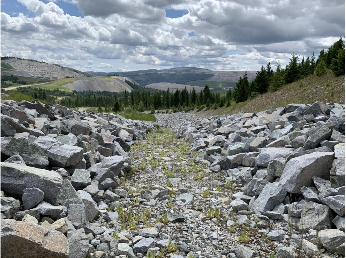
Photo I-A-13 Spillway channel downstream of the sand area observed in Photo I-A-12. No sand was observed downstream. No sign of recent flow or weathering/disruption of riprap was observed (TRJ-2020-12)
