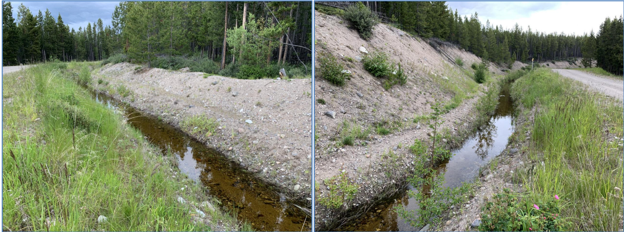
Photo I-A-22 Trojan Diversion (road junction). Culvert is clear. Low velocity flow of clear water into the unlined channel. (TRJ-2020-20)
