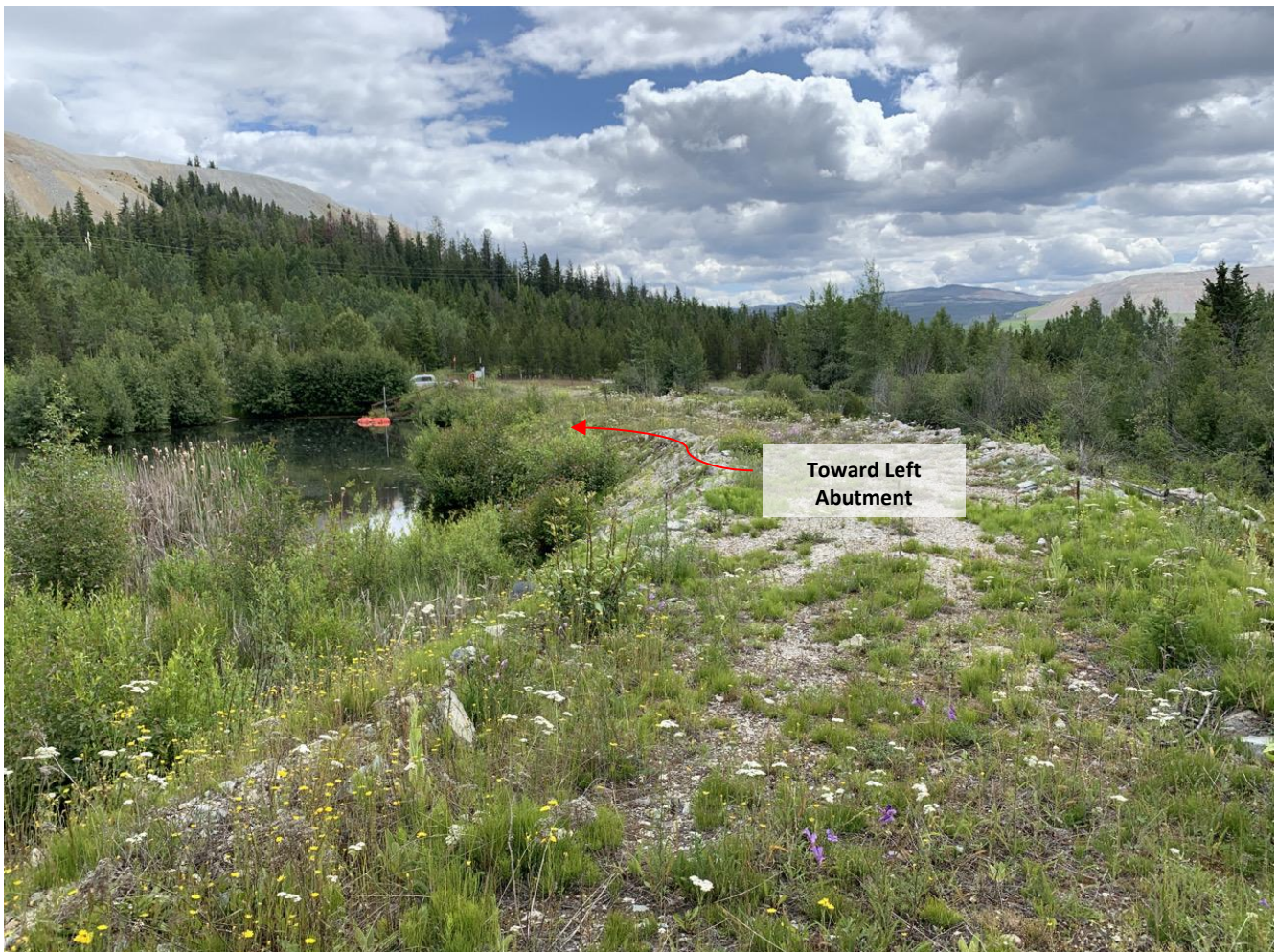
Photo I-C-1 Overview of crest from right abutment. Crest is uneven and appears to be sloped up to the west. THVCP should conduct a survey to confirm the low point (TRJ-2020-25)
