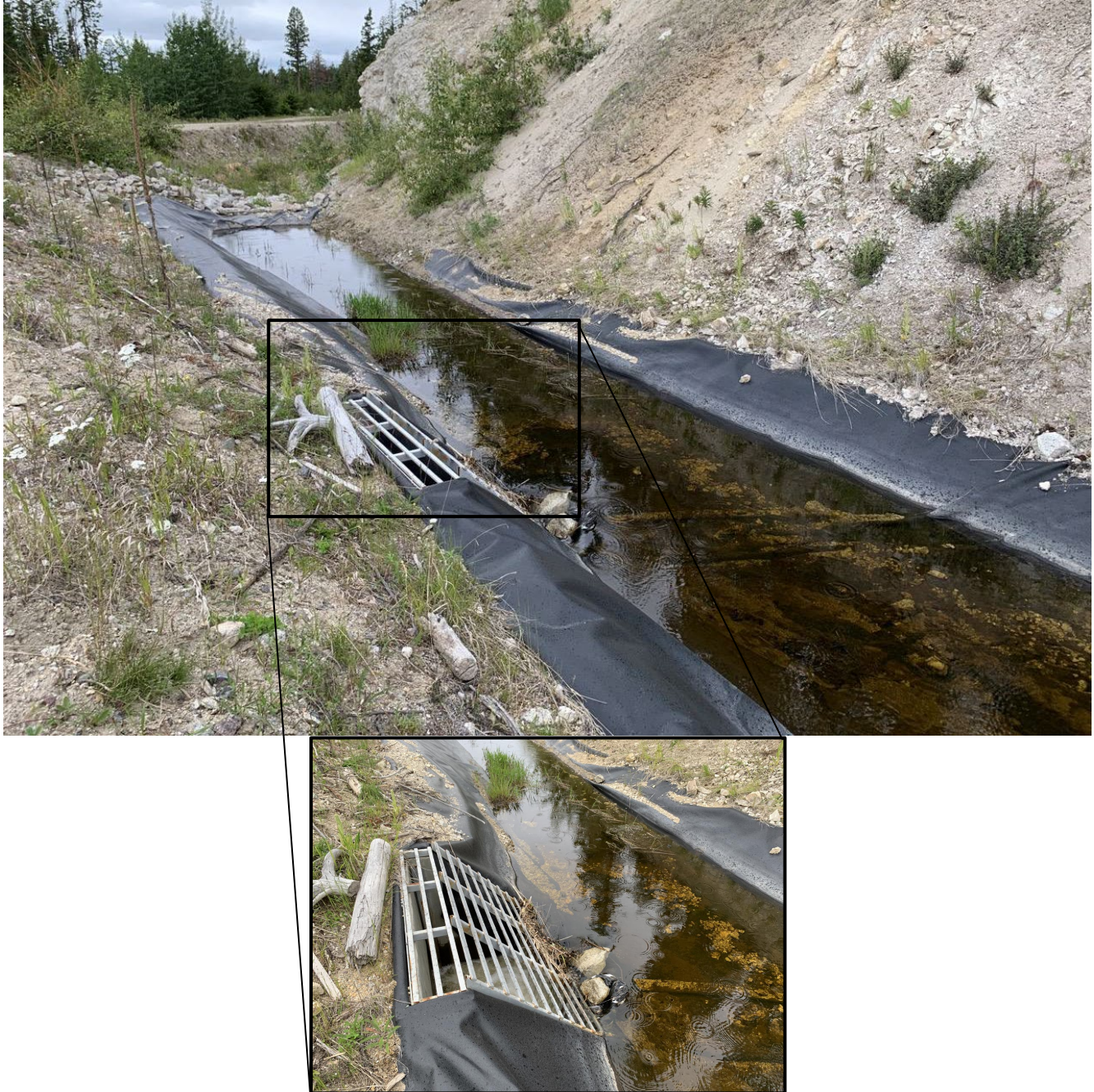
Photo I-A-18 Water flowing at the pipe intake southwest of Trojan TSF. Outlet valve here is open. Gate has minor debris accumulation. No flow bypassing diversion (i.e. flowing further downstream of channel. Trojan Diversion Valve 1 further upstream at Photo I-A-20 is closed (TRJ-2020-17)
