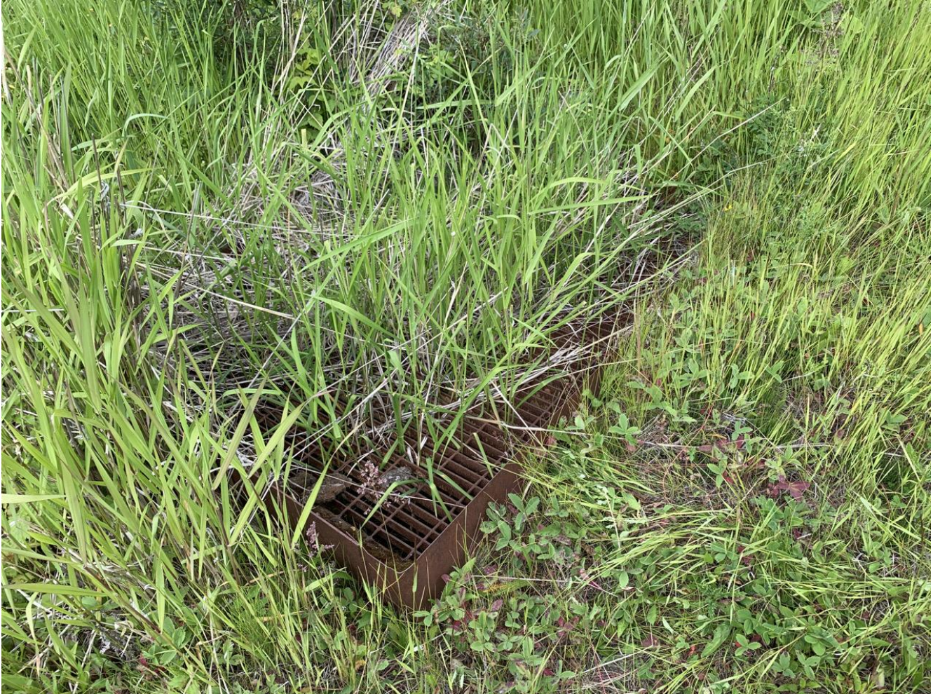
Photo I-C-6 Outlet which appeared to connect the upper basin to the lower basin at Lower Trojan Dam Pond. The inside was dry at the time of inspection and there were no sounds of flow. During inspection, flow from upper basin was reporting to lower basin via overland flow (TRJ-2020-28)
