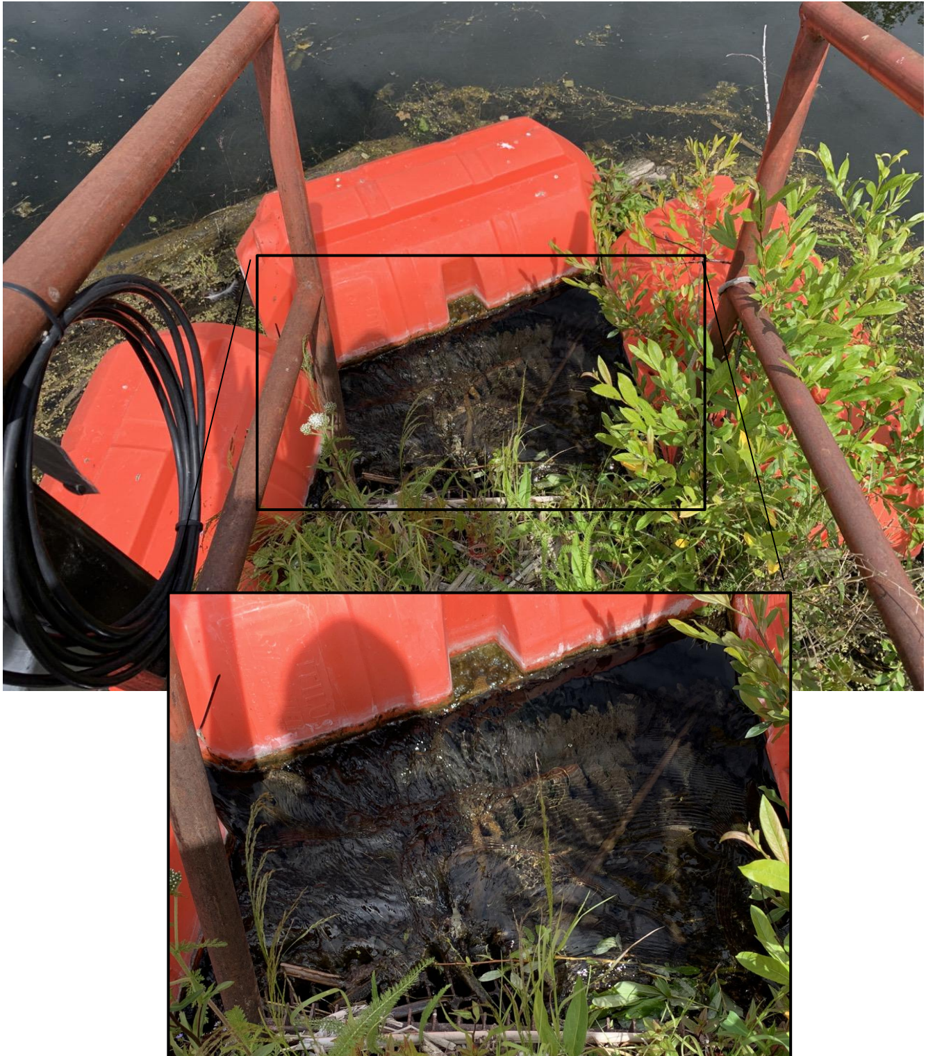
Photo I-C-10 Low-Level Outlet (LLO) inlet. Accumulated debris on trash rack was cleared by THVCP as part of routine maintenance after site visit (TRJ-2020-29)
