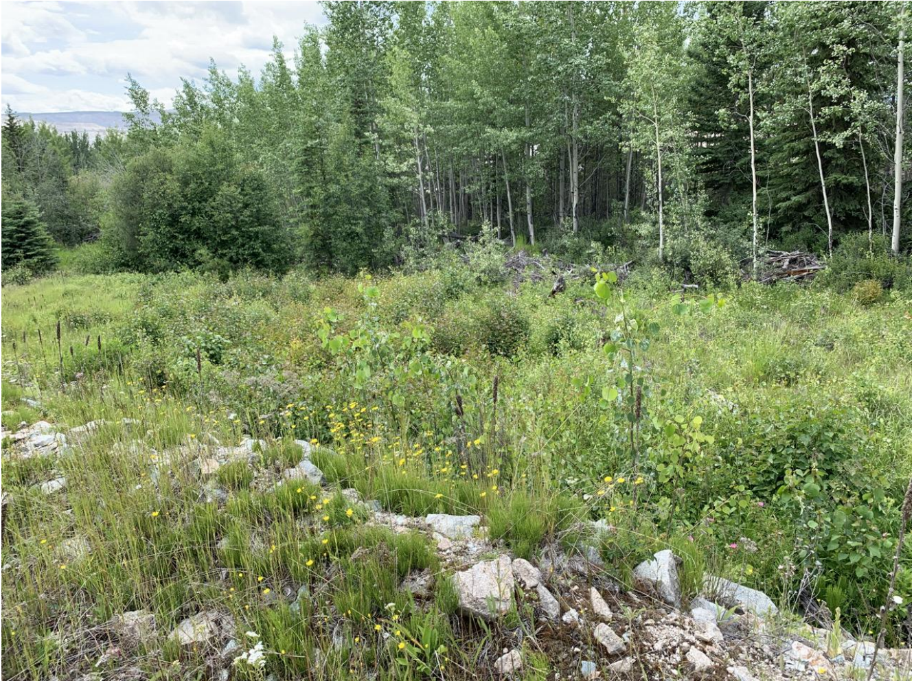
Photo I-C-8 Spillway channel looking toward south. Channel is heavily vegetated. THVCP received permit approval in December 2020 to complete clearing. Work is scheduled for spring 2021 (TRJ-2020-25)
