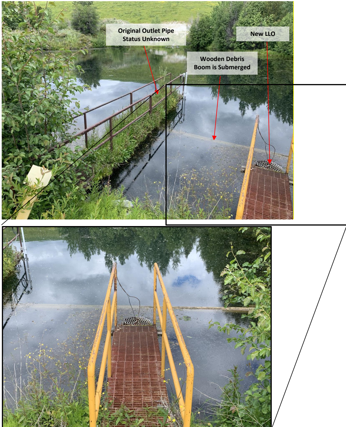
Photo I-B-3 Overview of the pond and low-level outlet to Witches Brook via Lower Trojan Dam with view of Trojan Dam downstream slope (TRJ-2020-22)
