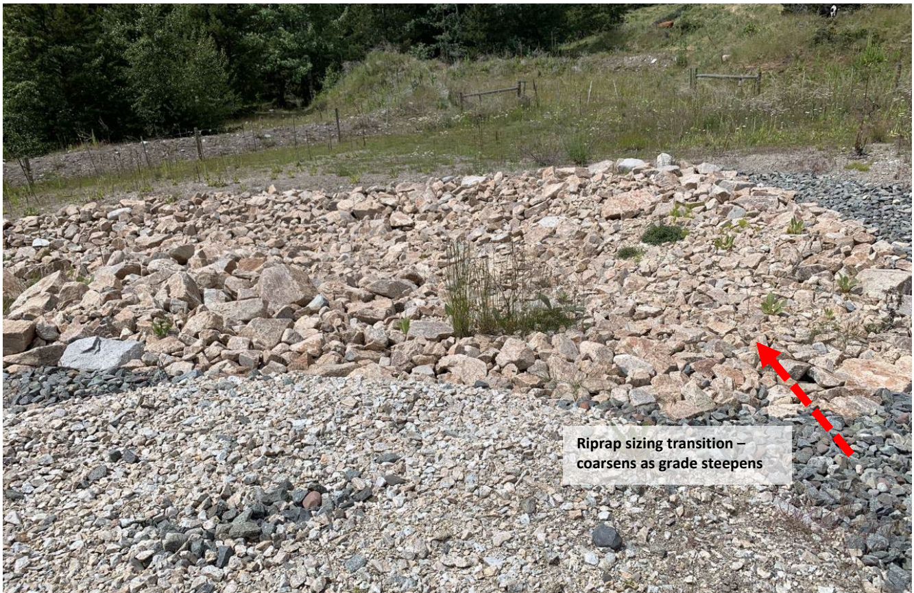
Photo I-B-6 Spillway Channel (TRJ-2020-24)
