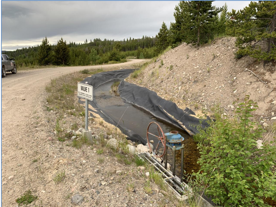
Photo I-A-20 Trojan Diversion Valve 1 is closed (no flow into impoundment) and locked. Valve is located at the transition of unlined to lined channel. Increased vegetation at the unlined channel (bottom photo), should be cleared for routine maintenance but is not a risk to Trojan flood routing) (TRJ-2020-18)
