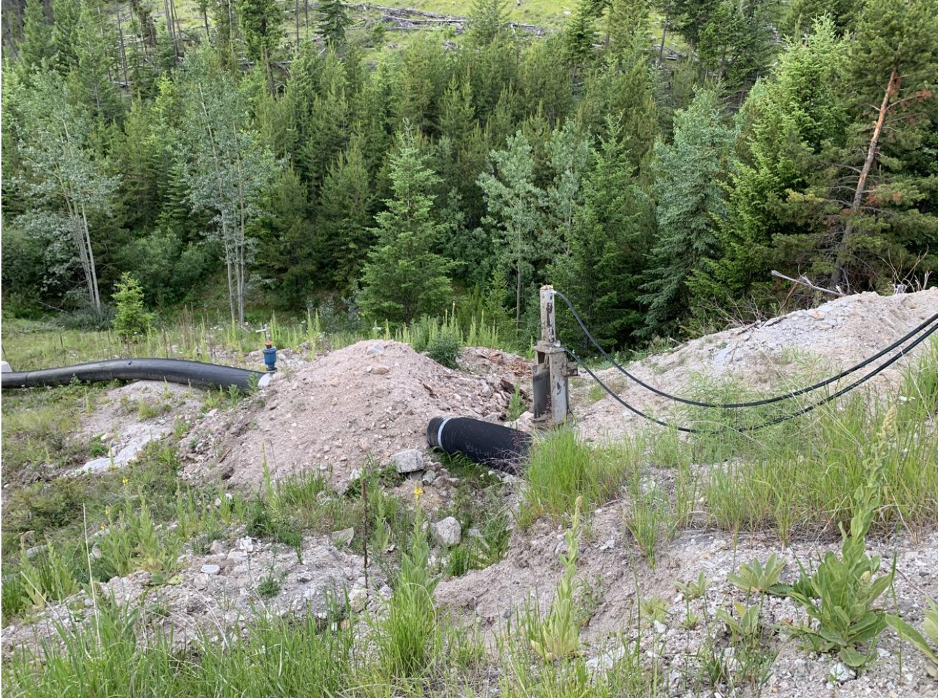
Photo I-A-19 Diversion pipe that was observed disconnected during 2019 AFPR site visit is repaired. Water discharging / valve open (TRJ-2020-17)
