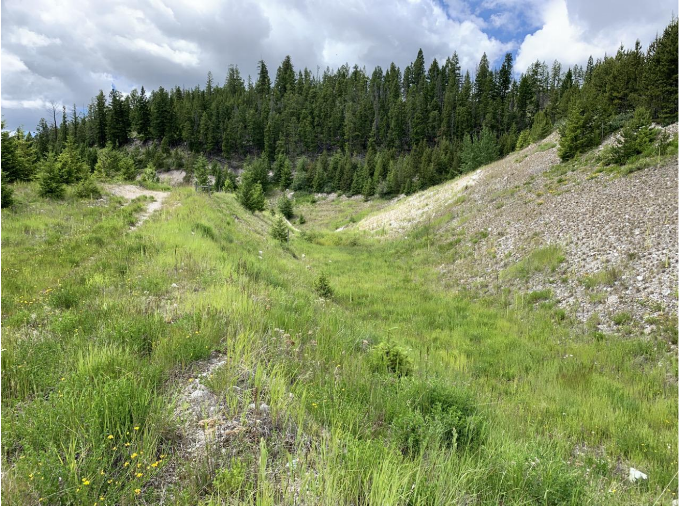
Photo I-A-10 Overview of spillway channel, downstream of chute. Slopes are in good condition. Channel is vegetated (TRJ-2020-09)
