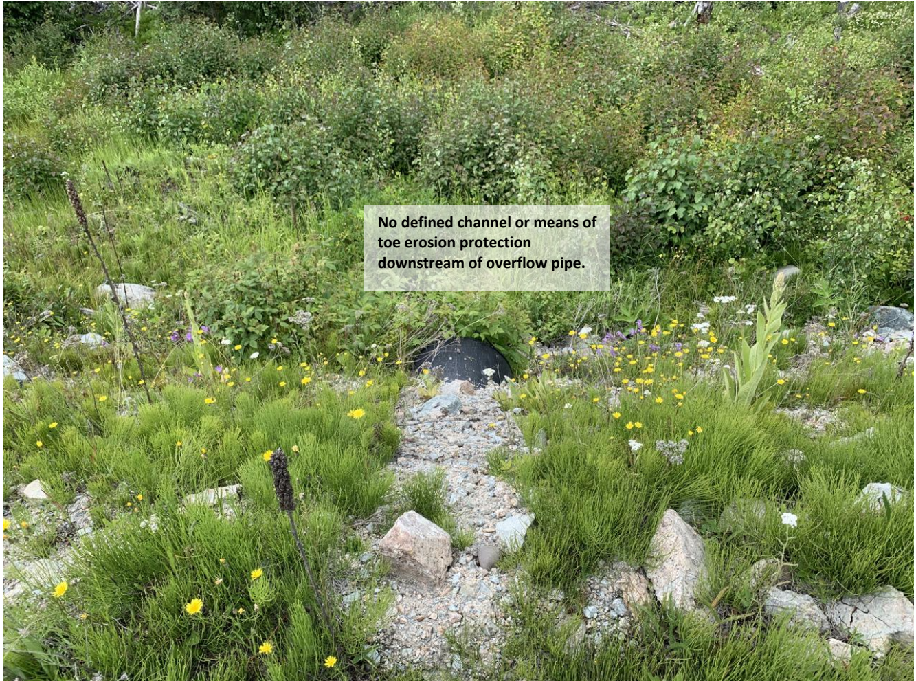
Photo I-C-3 Downstream slope near right abutment with overflow pipe through the dam. (TRJ-2020-26)
