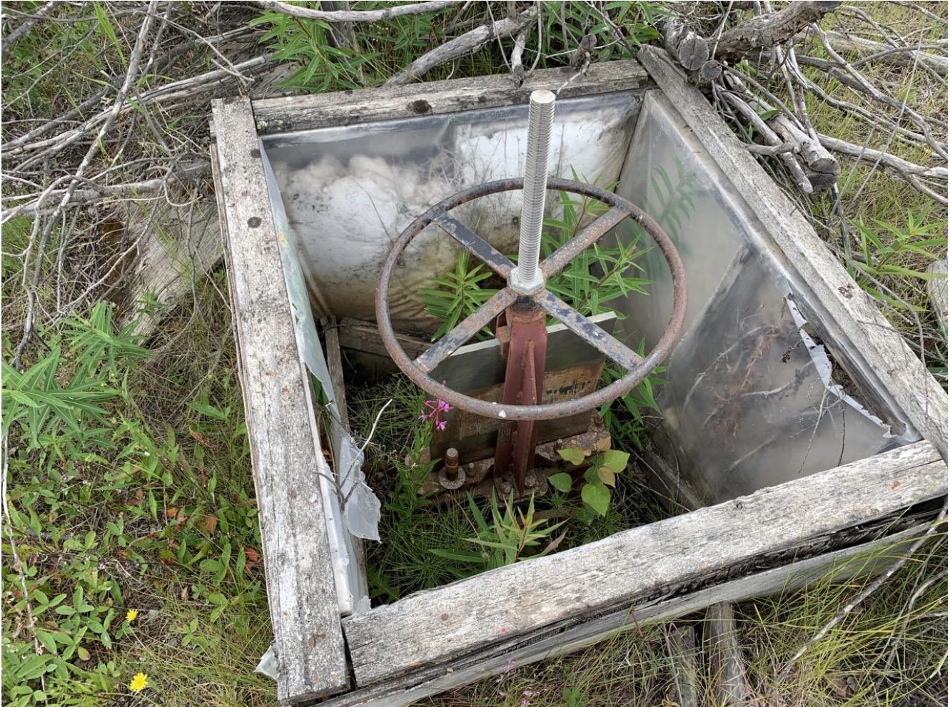
Photo I-C-11 Low-Level Outlet (LLO) valve can be hand operated to open and close (TRJ-2020-30)
