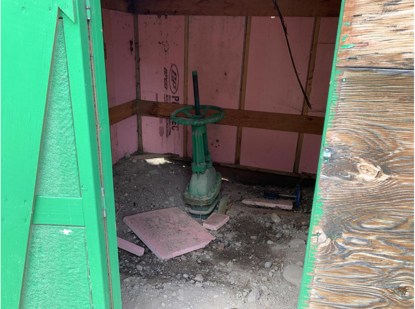
Photo I-B-4 Low Level Outlet valve in enclosure downstream of toe. The valve cannot be hand turned (TRJ-2020-23)
