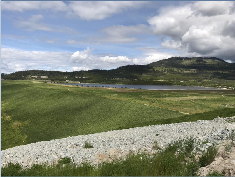
Photo I-A-3 Overview of Trojan Tailings Pond and Trojan Dam downstream slopes from left abutment. No visible erosion or scour (TRJ-2020-03)
