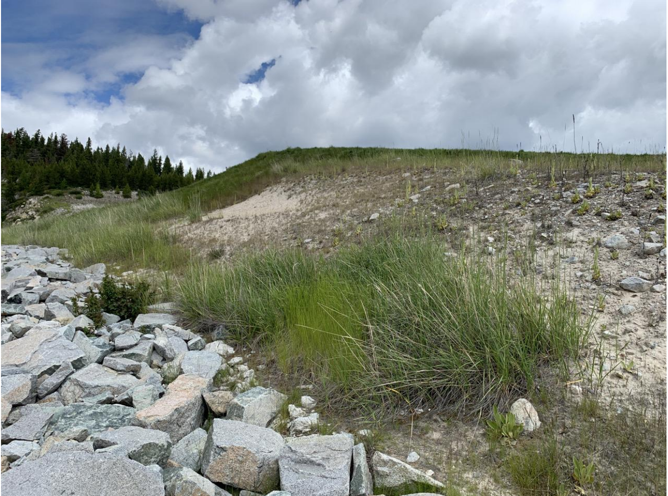
Photo I-A-15 Area of downstream slope without vegetation cover with sand exposed. Does not appear to be an active erosion area (TRJ-2020-14)
