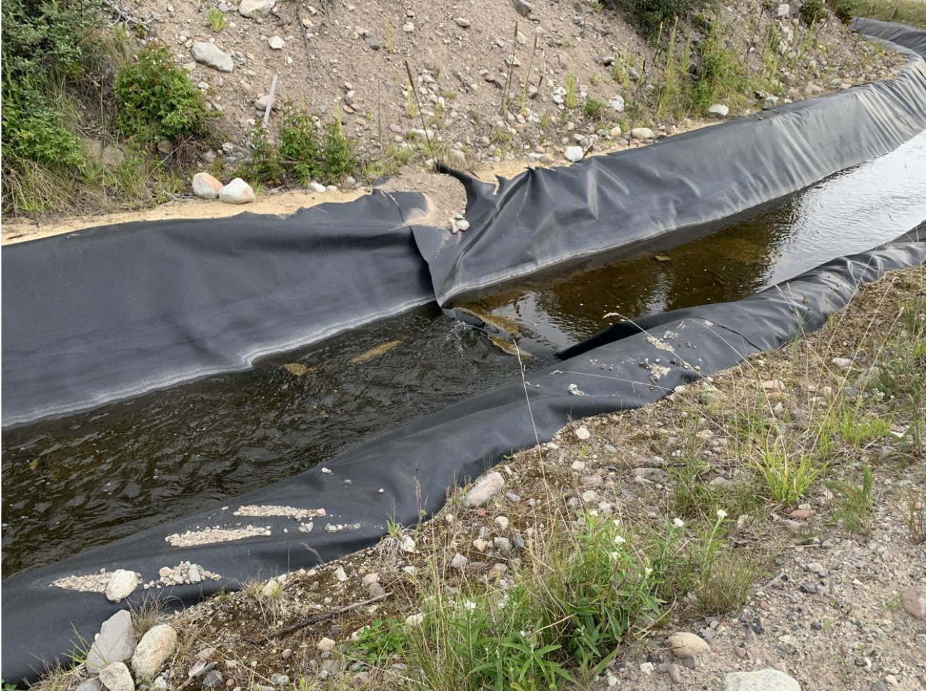
Photo I-A-17 Example of liner overlap point. No seepage faces observed on slope downstream of this area (TRJ-2020-16)
