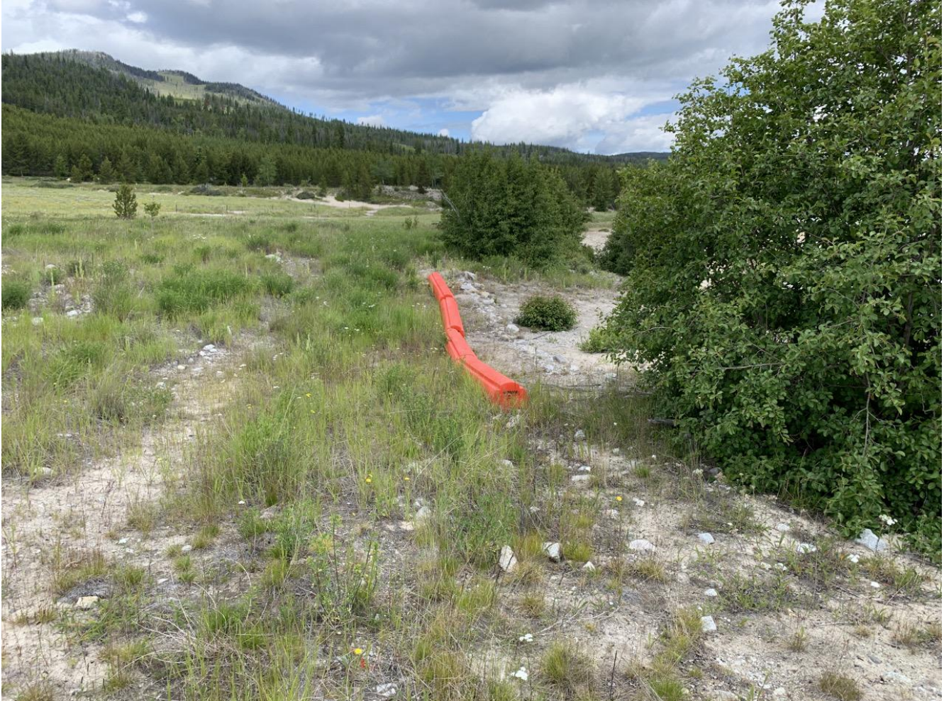
Photo I-A-7 Trojan spillway inlet. Approach channel is clear and debris boom is secured. (TRJ-2020-07)
