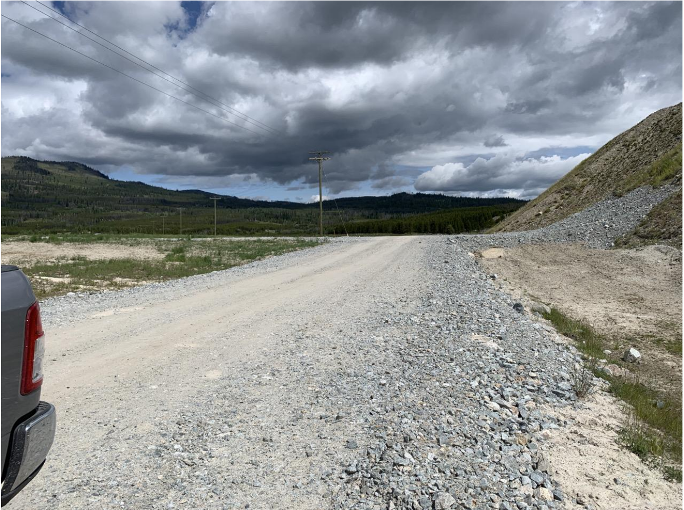
Photo I-A-2 Trojan Dam left abutment access road. Portion of road surface raised to provide minimum freeboard at design minimum flood beach width. Related recommendation was closed in 2019 AFPR (TRJ-2020-02)
