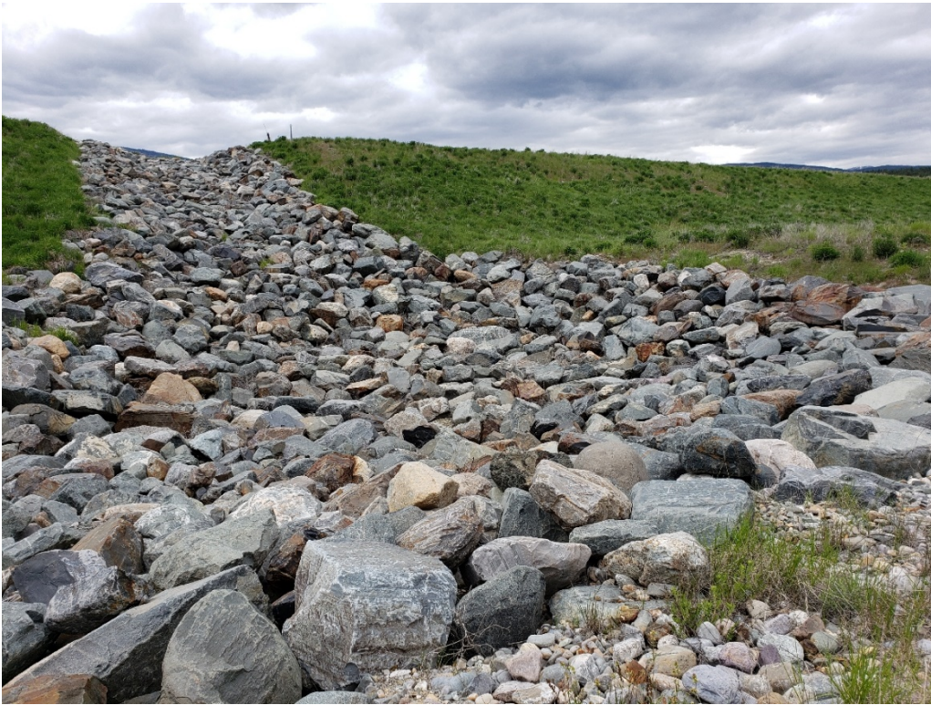
Photo II.18 Siliceous TSF Spillway on No. 3 Siliceous TSF
