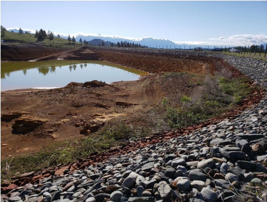
Photo II.2 North Dam Upstream Slope
