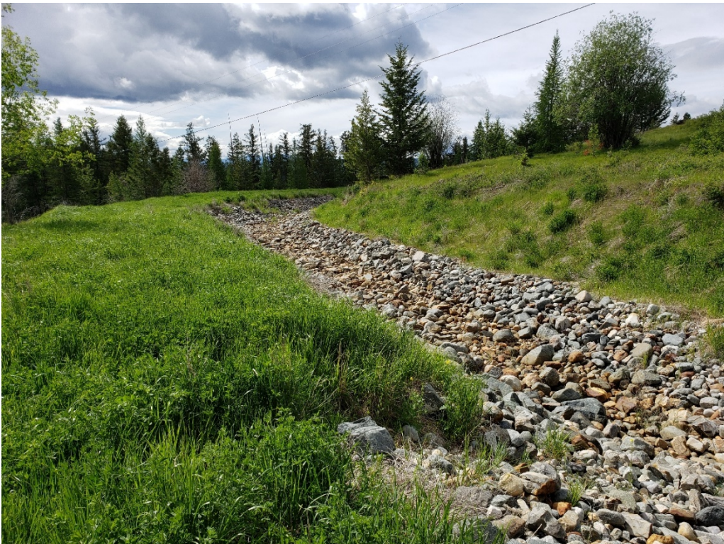
Photo II.12 Emergency Spillway Channel
