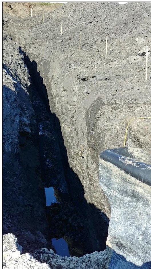
Photograph 18: West abutment cut-off wall extension under construction
