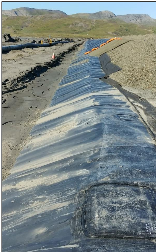
Photograph 11: Upstream slope of TMD under construction (looking toward west abutment)
