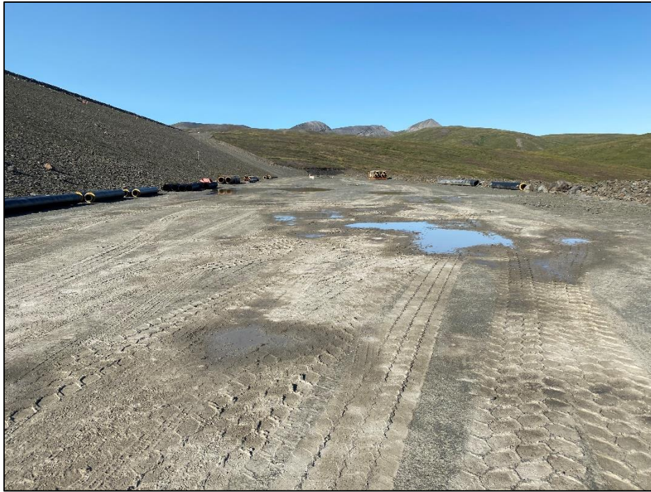
Photograph 01: Ponded water on Stage XI Buttress (looking southwest)
