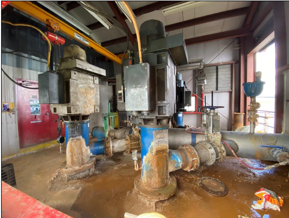
Photograph 09: Reclaim pumps inside reclaim barge
