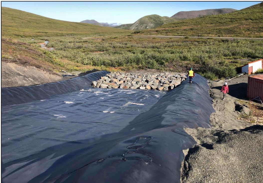
Photograph 10: Seepage collection pond spillway (looking northwest)
