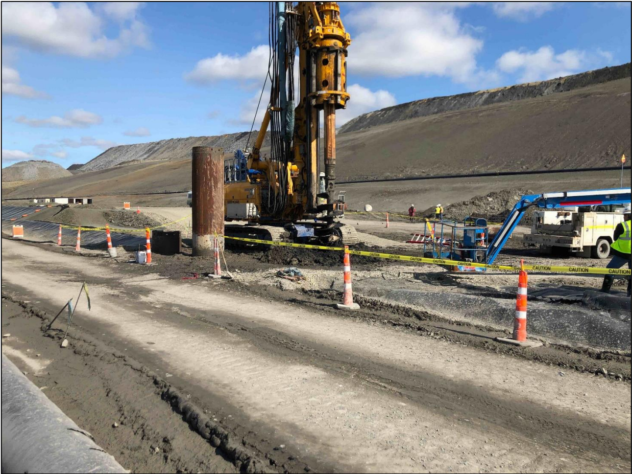
Photograph 21: Secant wall drilling
