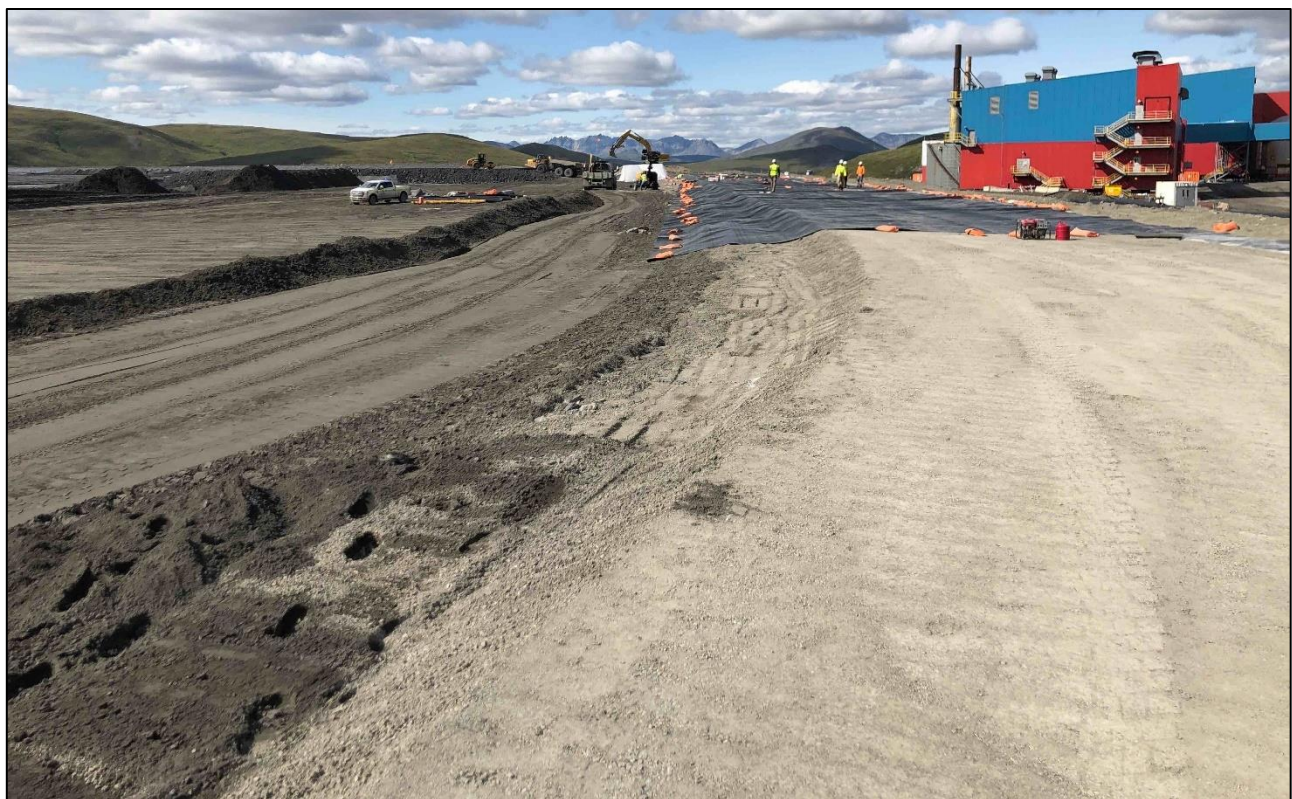
Photograph 20: Stage Xla wing wall under construction (near Sta. 40+00 looking northwest)
