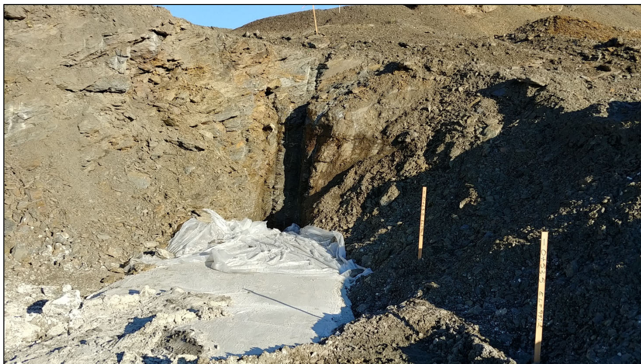
Photograph 12: West abutment excavation and cutoff wall excavation/construction
