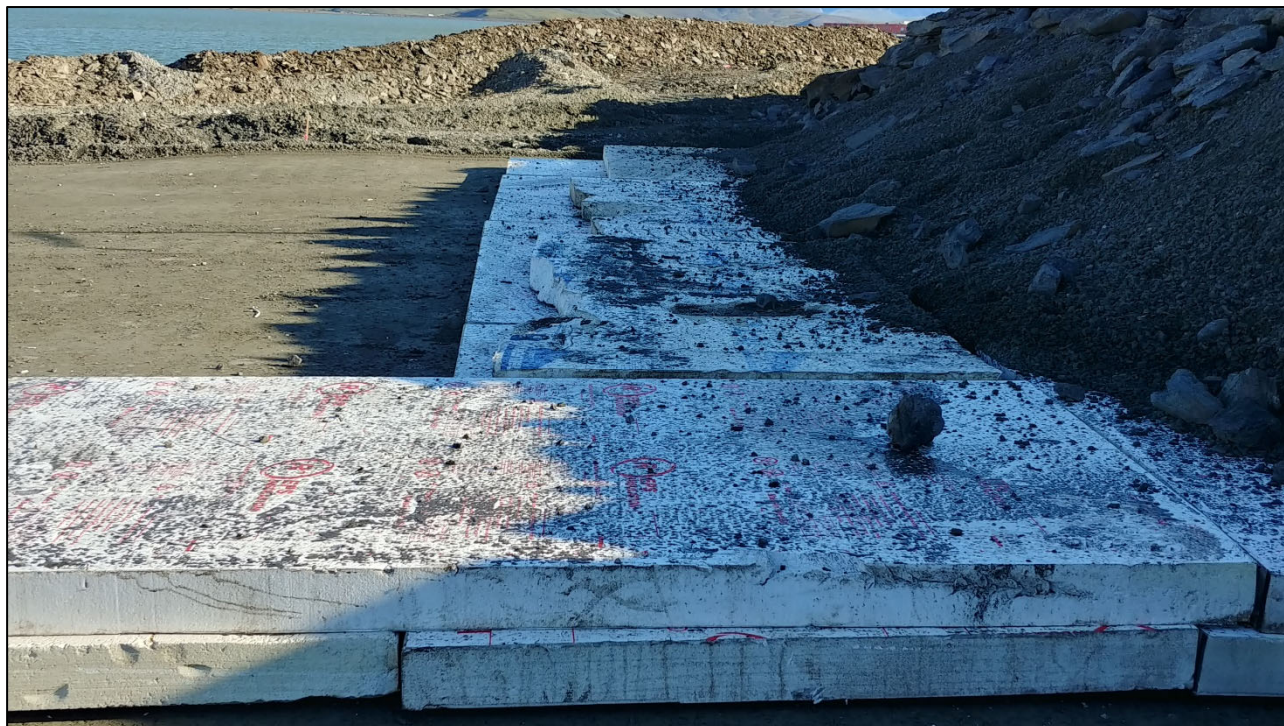
Photograph 19: Insulation installation at utility and road crossing near Sta. 42+50
