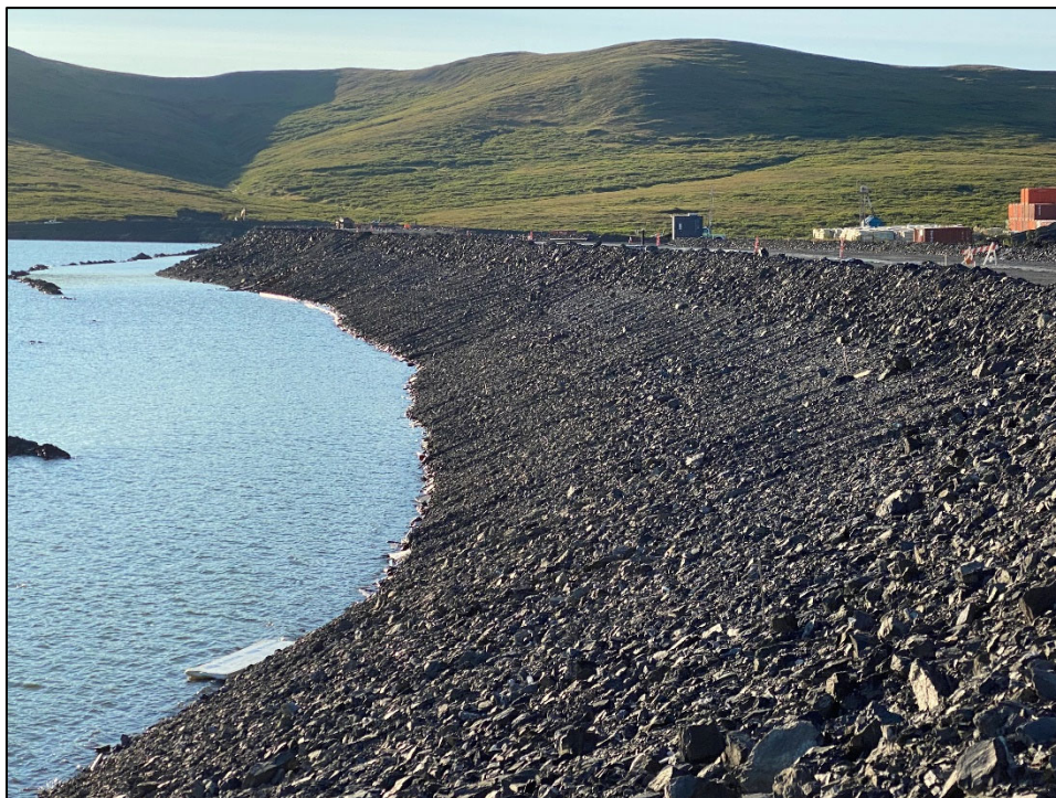
Photograph 05: Upstream slope (looking east)
