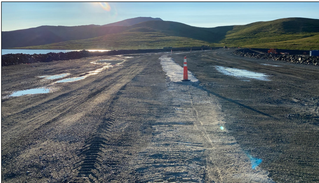
Photograph 01: TBD crest, near Sta. 25+00 (looking east)
