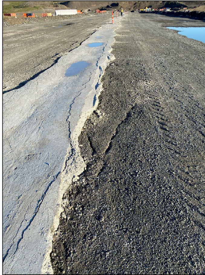
Photograph 17: Cut-off wall construction
