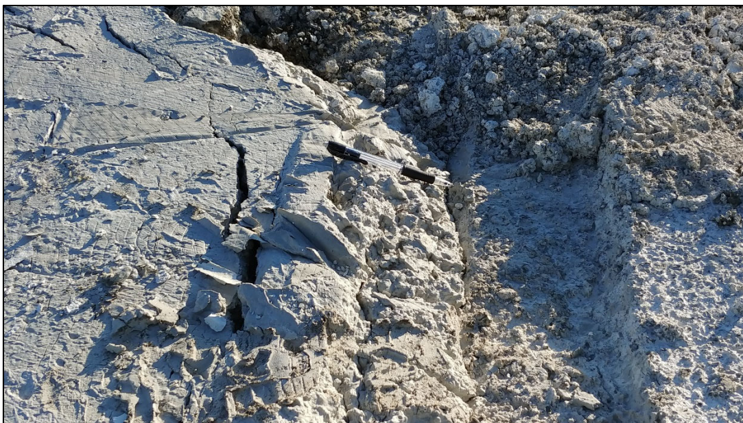
Photograph 18: Panel joint at cut-off wall (under construction)
