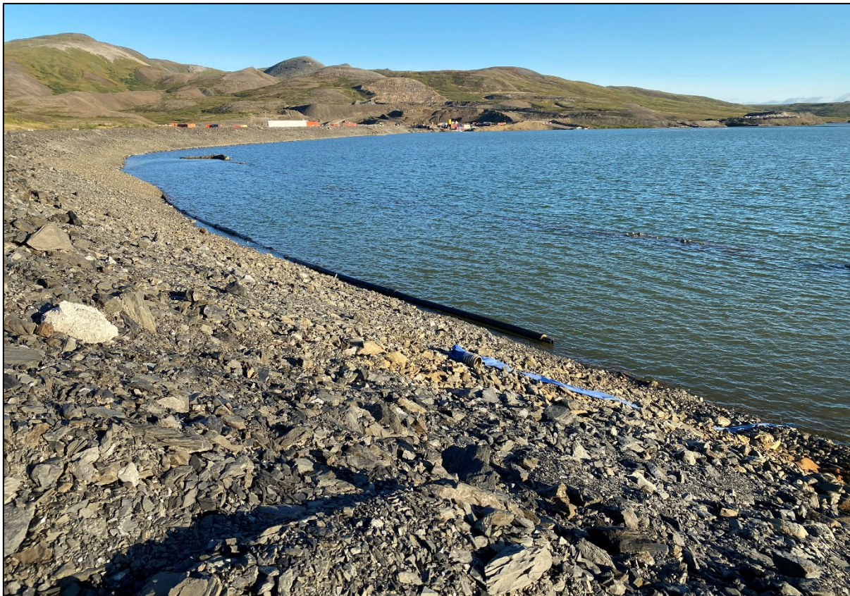
Photograph 04: Upstream slope (looking northwest)
