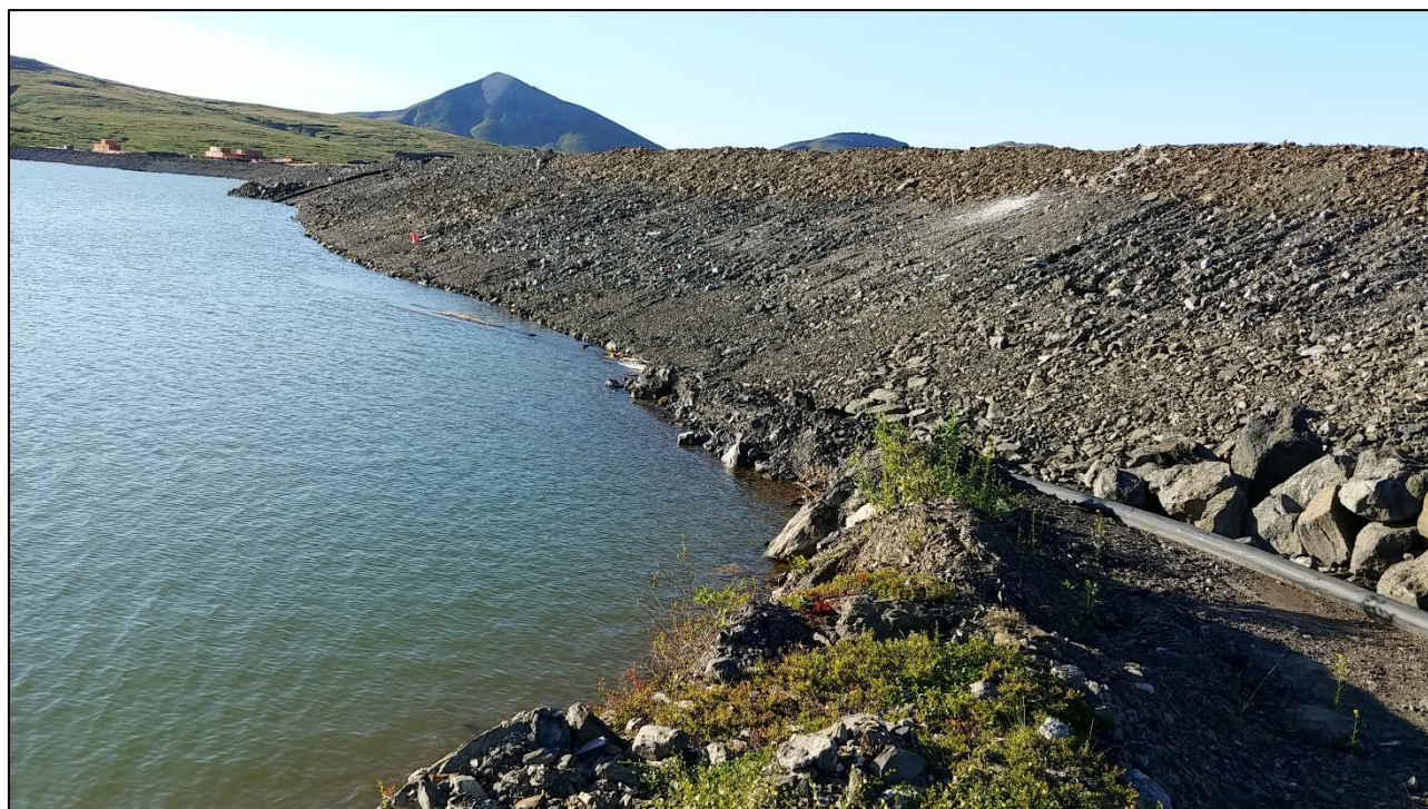
Photograph 06: Upstream slope near Sta. 6+00 (looking southeast)
