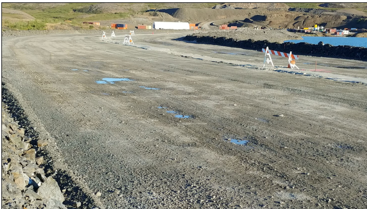
Photograph 02: TBD crest, near Sta. 22+50 (looking northwest)
