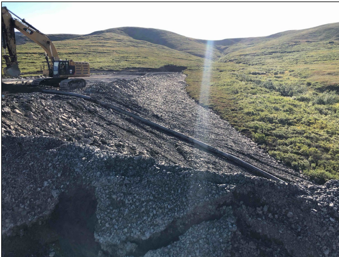
Photograph 10: Downstream slope near Sta. 42+50 (looking east)
