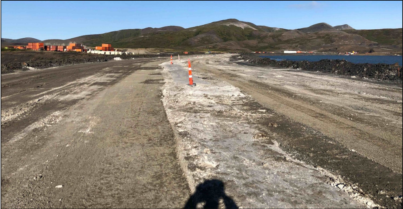
Photograph 03: TBD crest, near Sta. 26+00 (looking west)
