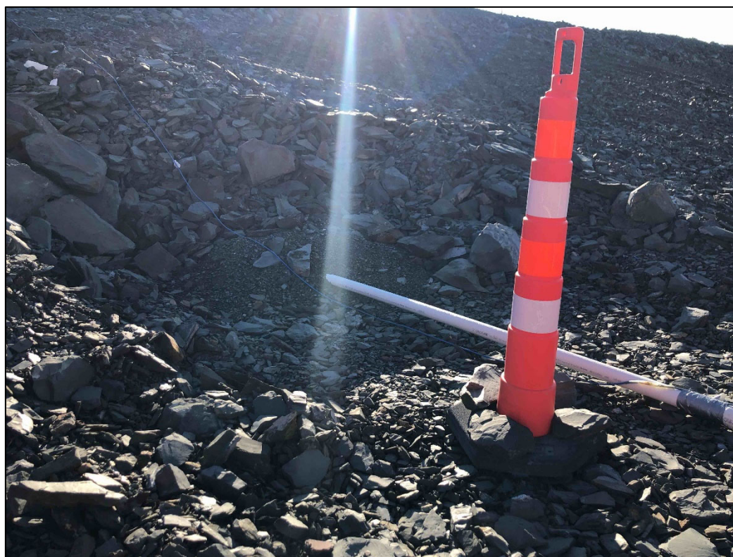
Photograph 16: Piezometer cable extension at downstream slope
