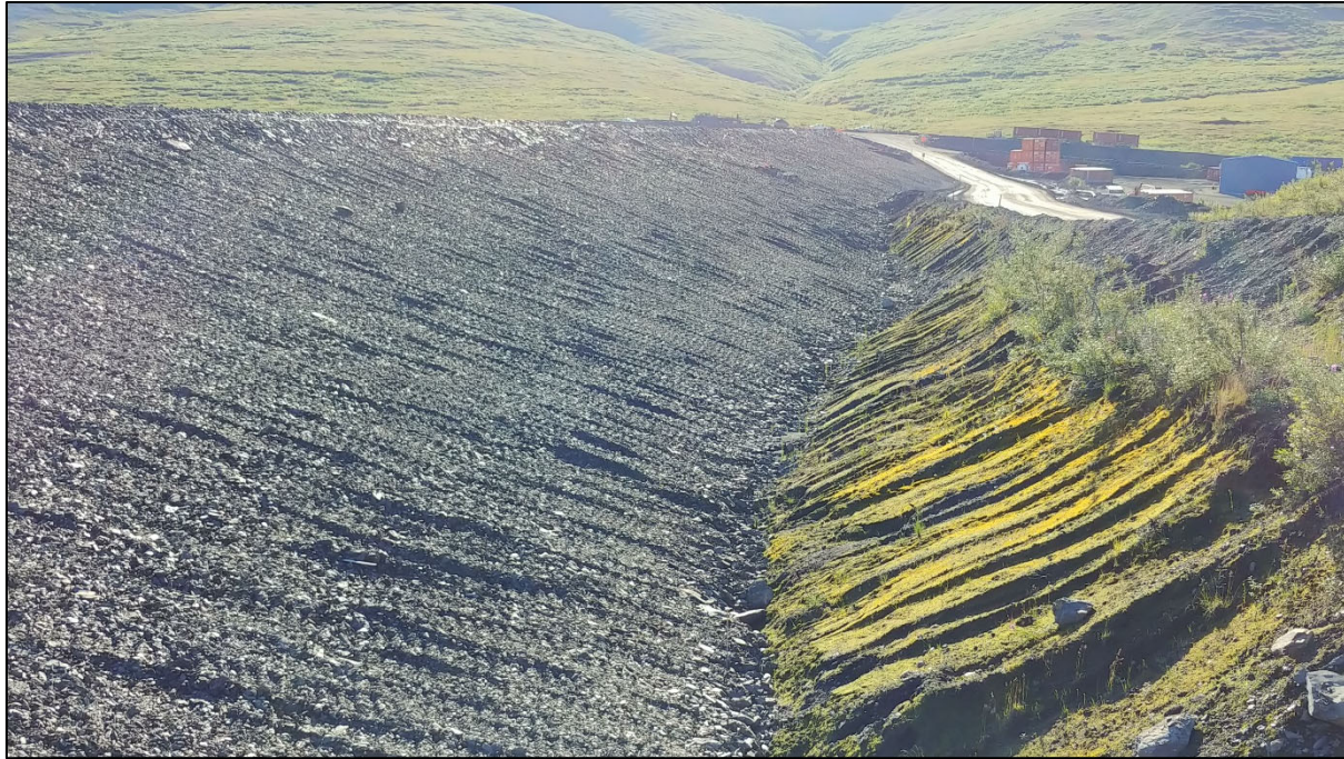
Photograph 09: Downstream slope near Sta. 27+00 (looking east)
