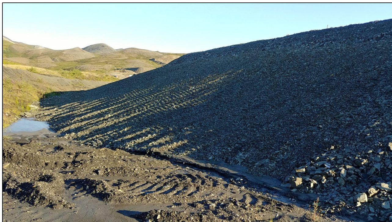
Photograph 08: Downstream slope near Sta. 22+50 (looking west)
