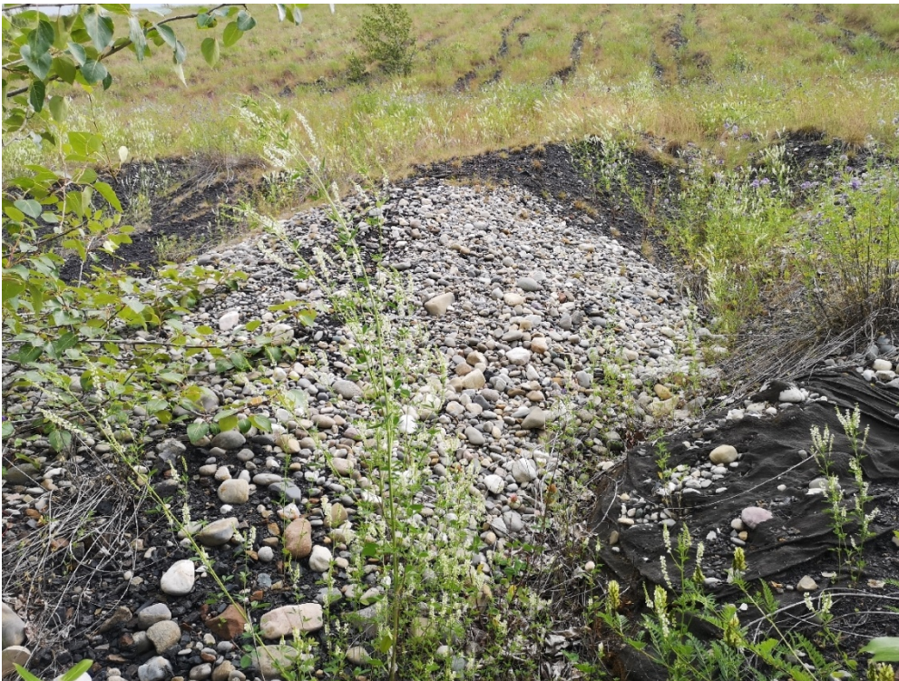
Photo I-43 Finger drain, no flow (PTD-DRAIN-10)
