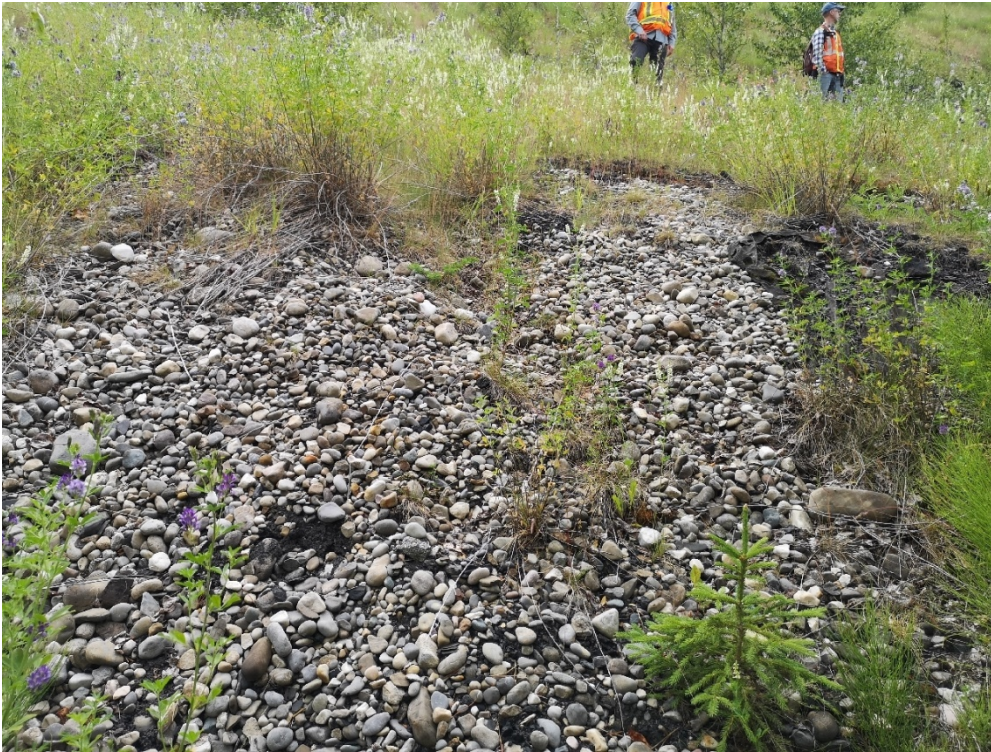
Photo I-64 Finger drain, downstream area is wet, no seepage visible (PTD-DRAIN-22)
