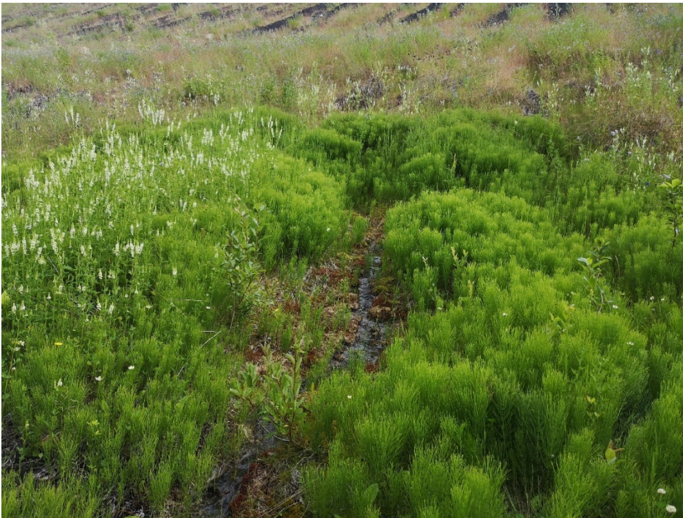
Photo I-55 Finger drain, flowing into two channels (PTD-DRAIN-19)
