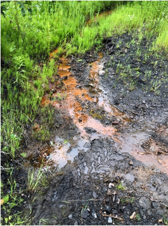
Photo I-39 Finger drain, no flow (PTD-DRAIN-02)
