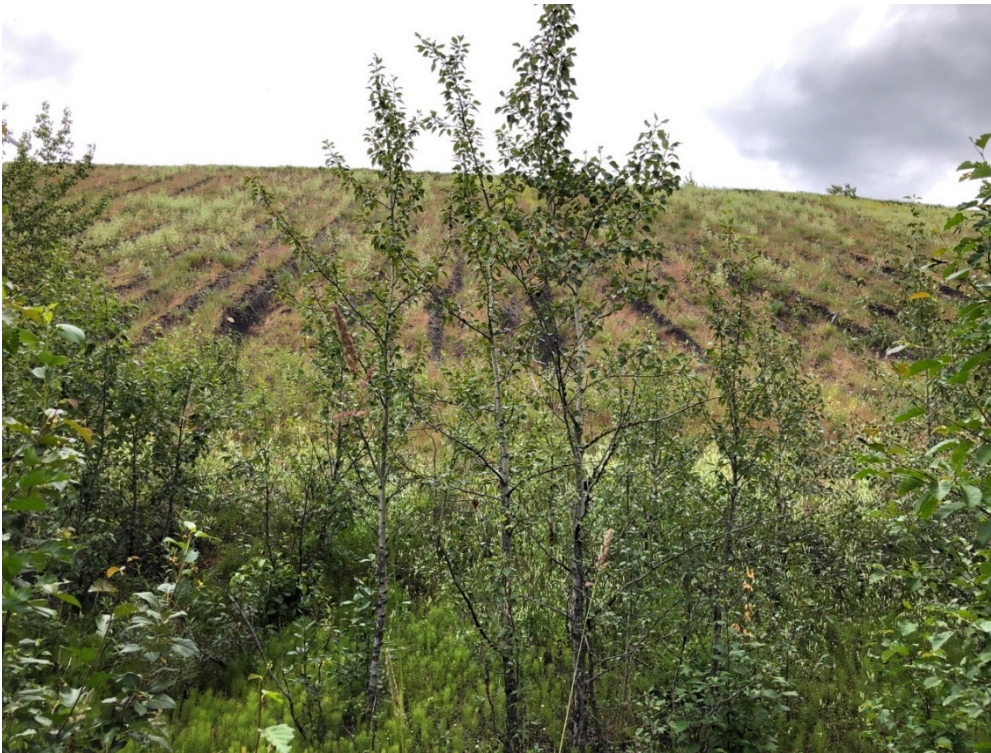
Photo I-37 Minor rilling along downstream slope. Refer to Appendix II for specific rill monitoring photos (PTD-2020-17)
