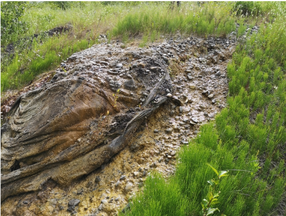
Photo I-65 Finger drain, some seepage (PTD-DRAIN-23)
