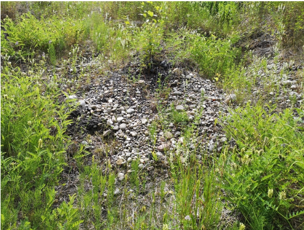
Photo I-67 Finger drain, dry (PTD-DRAIN-25)
