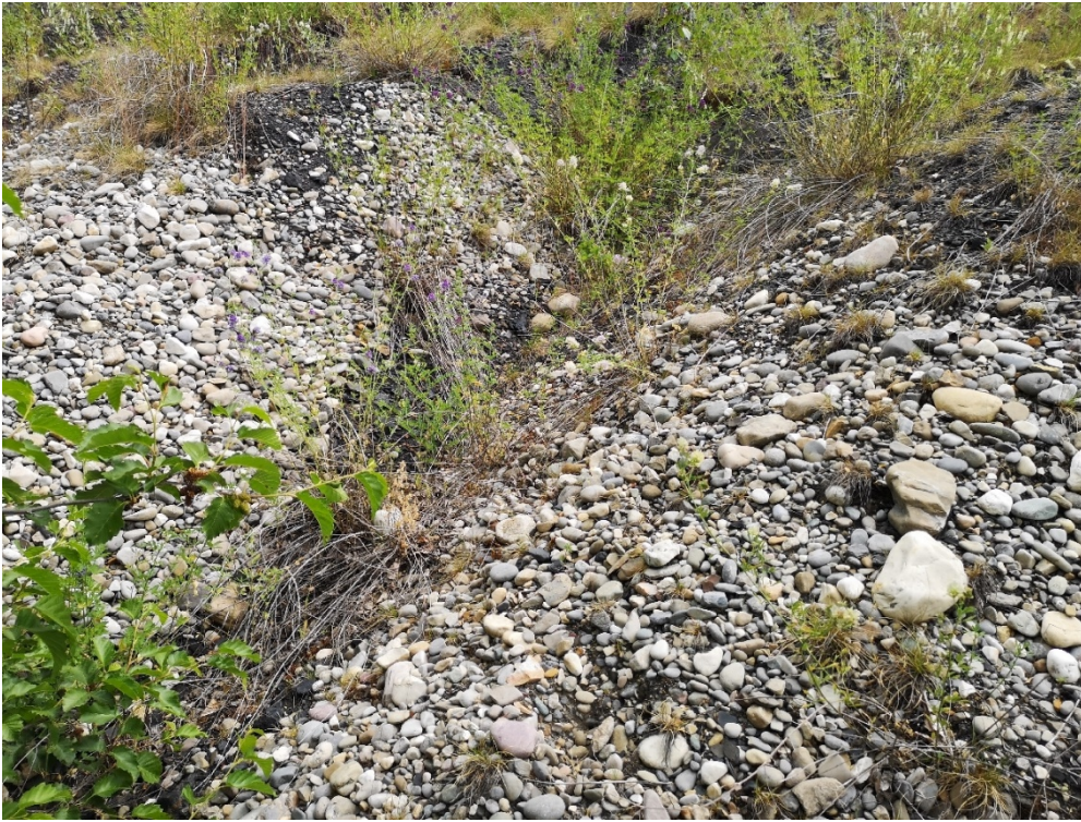
Photo I-51 Finger drain, dry (PTD-DRAIN-16)
