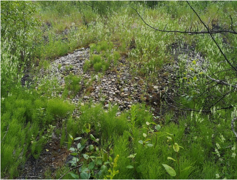
Photo I-53 Finger drain, dry (PTD-DRAIN-18)
