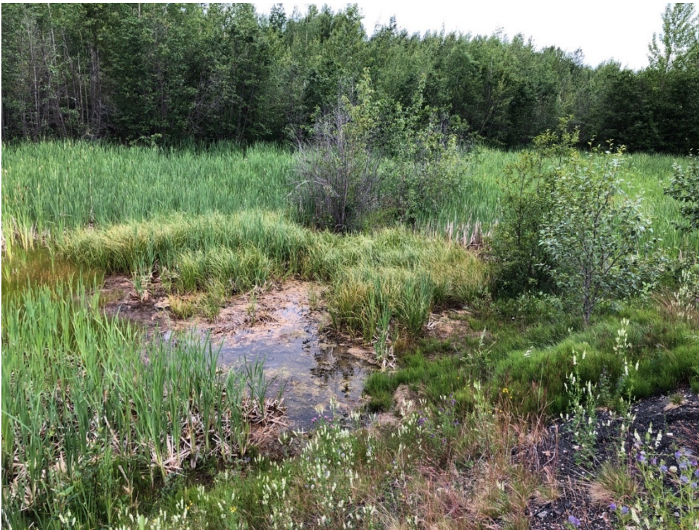
Photo I-33 Ponded water in low spot at toe of dam (PTD-2020-14)
