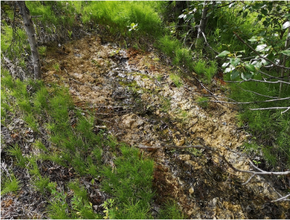
Photo I-47 Finger drain, no seepage (PTD-DRAIN-12)
