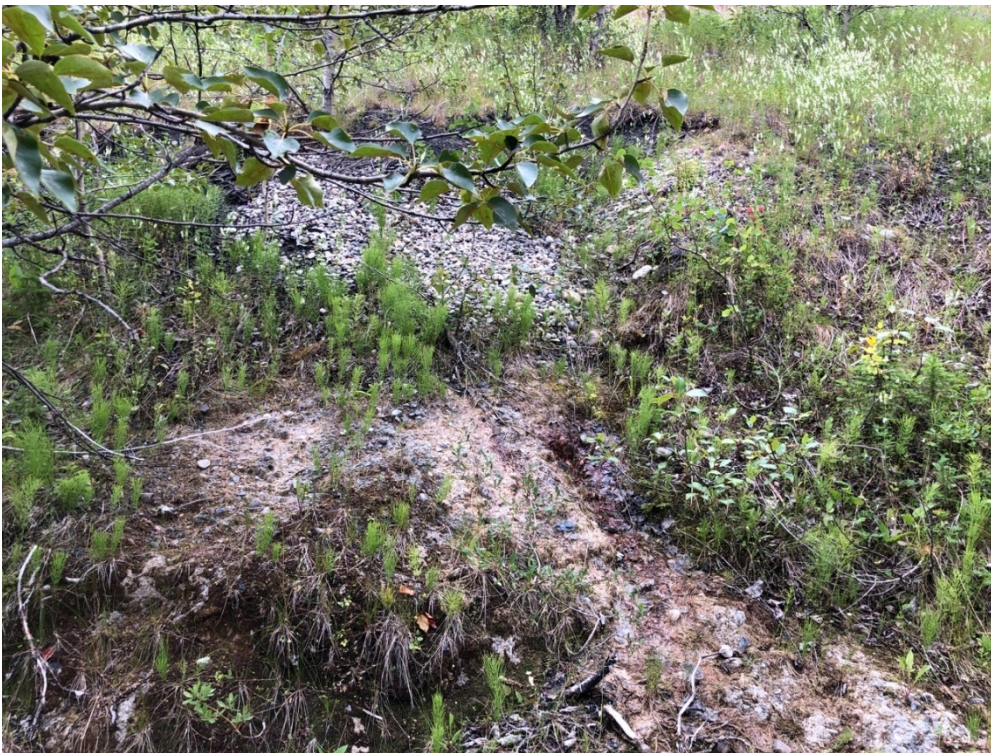
Photo I-39 Finger drain, no flow (PTD-DRAIN-02)
