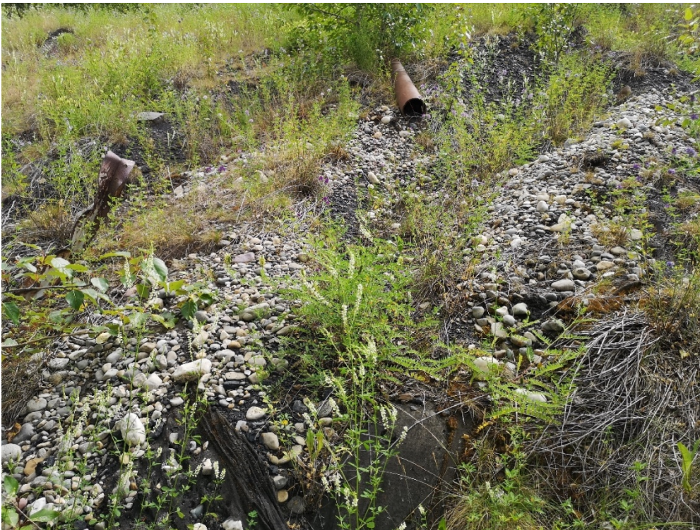
Photo I-47 Finger drain, no seepage (PTD-DRAIN-12)
