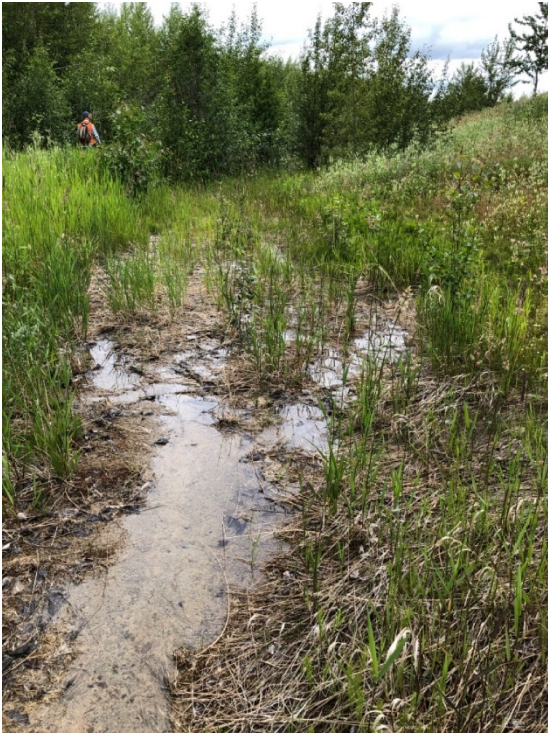
Photo I-37 Minor rilling along downstream slope. Refer to Appendix II for specific rill monitoring photos (PTD-2020-17)
