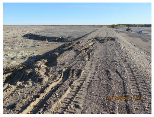
Photograph 4: South Dyke – Central Portion - Damage to Crest and Upstream Slope, Looking East, 22 September 2020 (Repaired same day)
