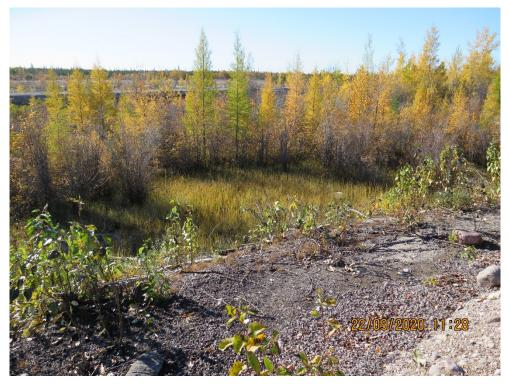
Photograph 6: South Dyke – West End - Downstream Slope Cleared of Vegetation and Toe Area with Wet Ground, Looking Southwest, 22 September 2020
