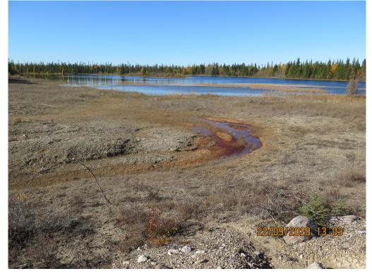
Photograph 10: West Dyke – North End - Downstream Toe Area with Staining Along Drainage, Looking West, 22 September 2020
