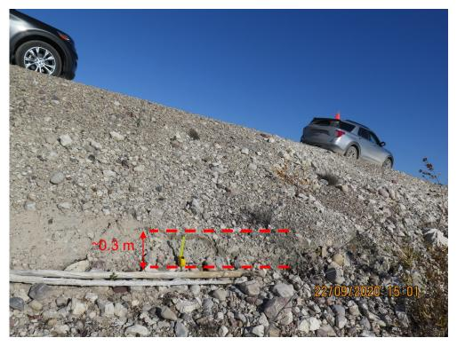
Photograph 19: North Dyke – Upstream Slope West of Dogleg, ~0.3 m Scarp with Exposed Core, Looking Northeast, 22 September 2020
