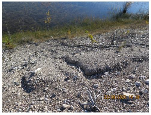
Photograph 27: North Dyke – East End - Upstream Slope with Erosion Rill, looking South, 22 September 2020
