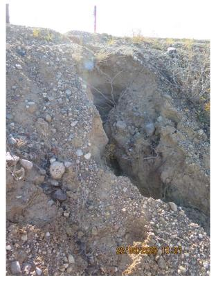
Photograph 14: North Dyke - West End - Erosion Rill on Downstream Slope, Detail, 22 September 2020
