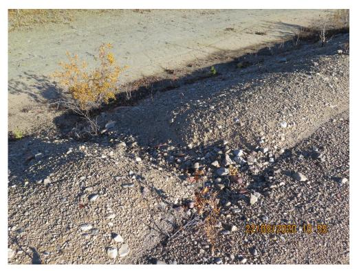
Photograph 2: South Dyke - East End – Erosion Rills on Upstream Slope, Looking Northeast, 22 September 2020
