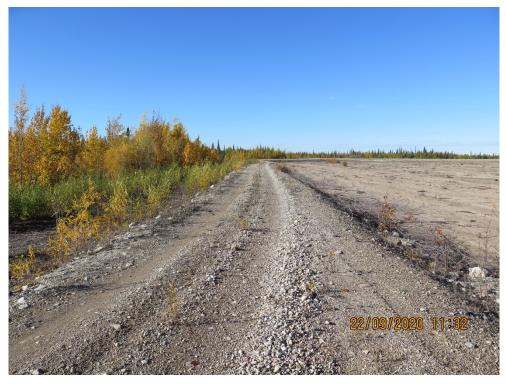
Photograph 5: South Dyke –West End - Crest with Vegetation on Downstream Slope, Looking West, 22 September 2020
