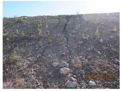
Photograph 13: North Dyke – West End - Erosion Rills on Downstream Slope, Looking South, 22 September 2020
