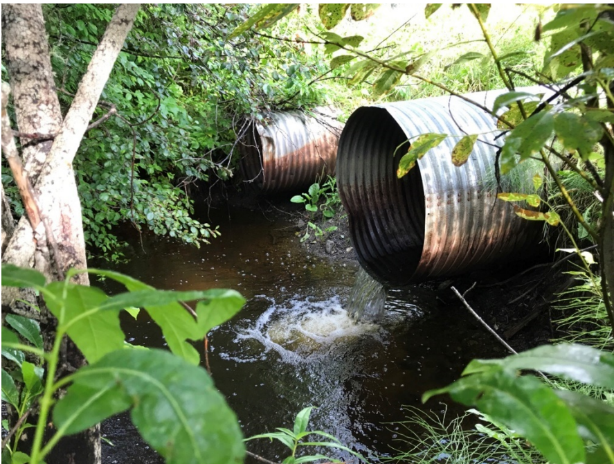
Photo II-50 Outlet of Ed Creek culverts under Pinchi Lake Road. Note only one culvert is flowing.
