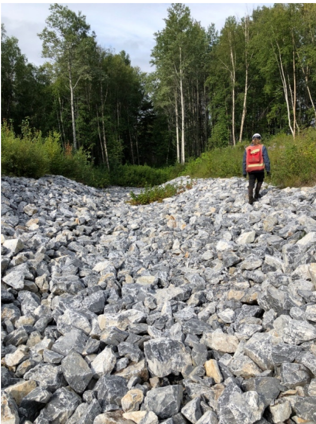
Photo II-22 Closure Spillway – looking downstream towards outlet. Note vegetation.
