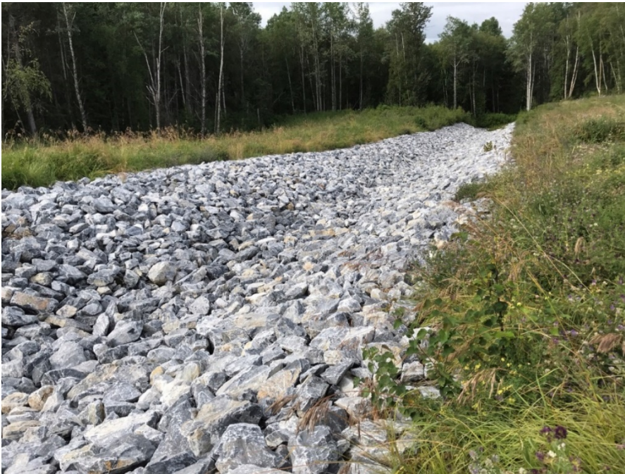
Photo II-22 Closure Spillway – looking downstream towards outlet. Note vegetation.
