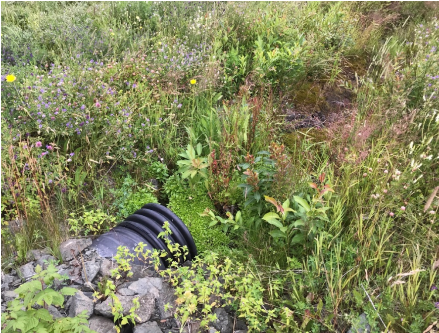
Photo II-45 Inlet of 460 mm culvert on north bank of Ed Creek Diversion Channel. There is minor vegetation upstream of the inlet.
