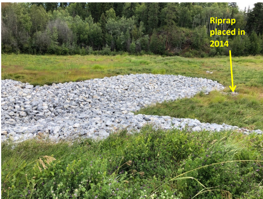
Photo II-16 Closure Spillway – Inlet apron.
