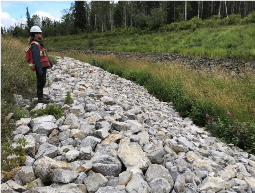
Photo II-39 Ed Creek Diversion Channel – looking upstream from near second bend. Light coloured area of riprap was replaced in 2014 and is in good condition.
