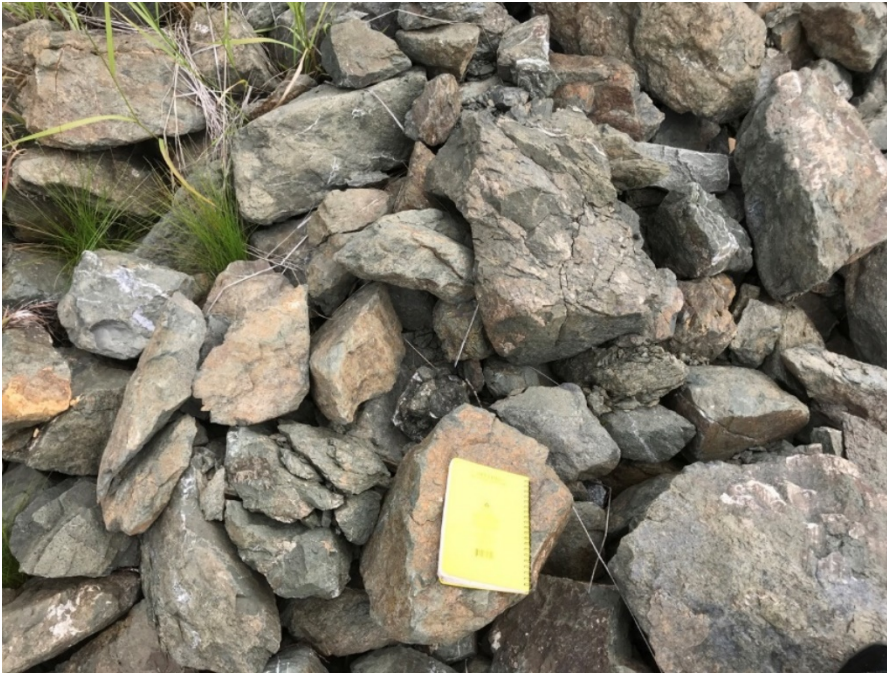
Photo II-35 Ed Creek Diversion Channel – Riprap on right bank, showing weathering and breakage.
