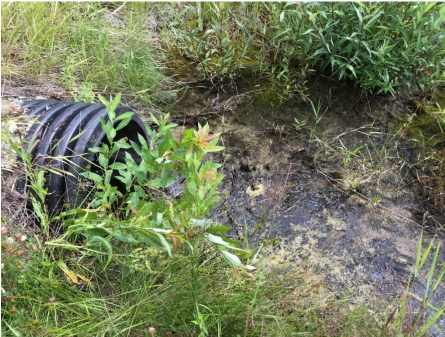
Photo II-26 Spillway Downstream Channel – Outlet of culvert beneath road to on-site residence.
