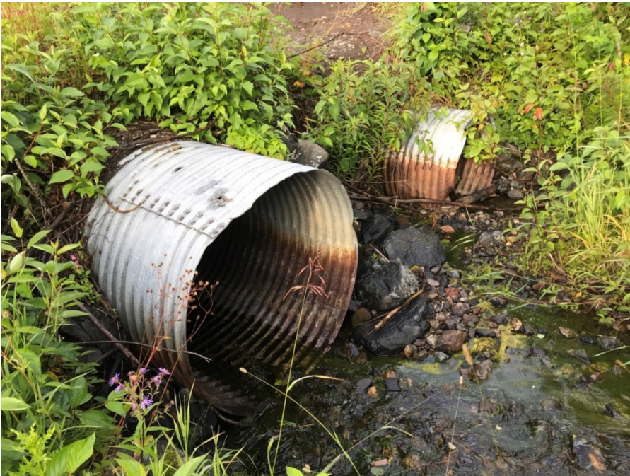
Photo II-47 Inlet of Ed Creek culverts under Pinchi Lake Road. Note only one culvert is flowing.
