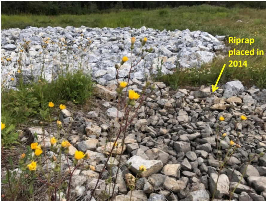
Photo II-17 Closure Spillway – Inlet apron.
