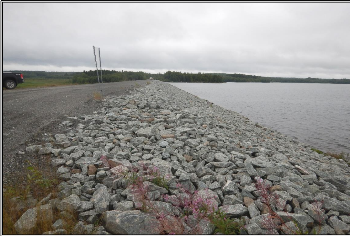
Photo 1 : Dam 1D - New rip rap placed in 2019 on upstream slope. View looking South-East.
