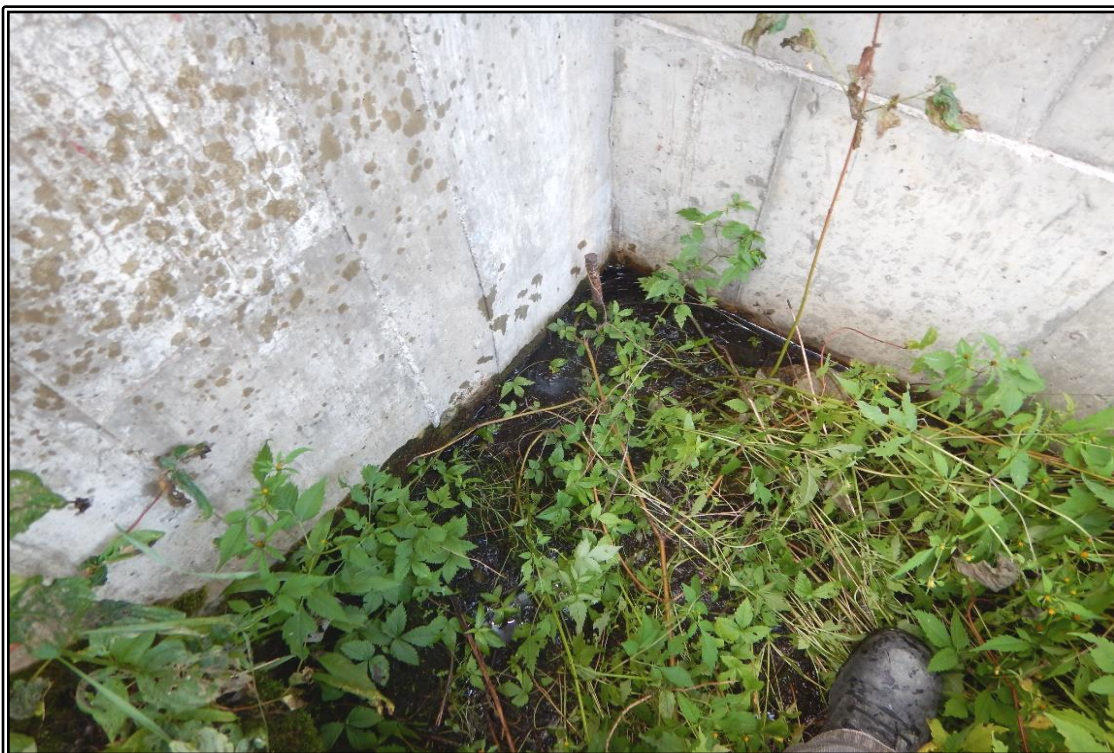
Photo 14 : Dam 4B – North shoulder of the service spillway. Minor seepage and ponding at the contact between the rock and the concrete structure.
