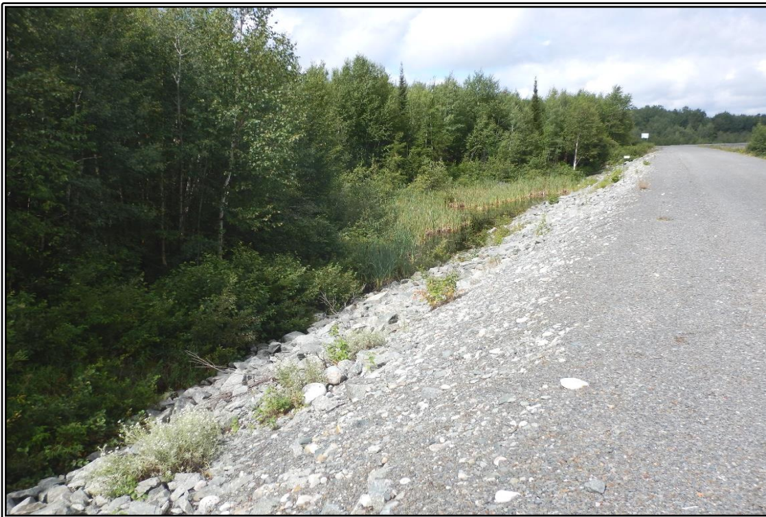
Photo 10 : Dam 2A - Stagnant water at the downstream toe of the dam. This area represents a zone where the natural topography drains towards the tailings pond; some accumulation at this location is expected.
