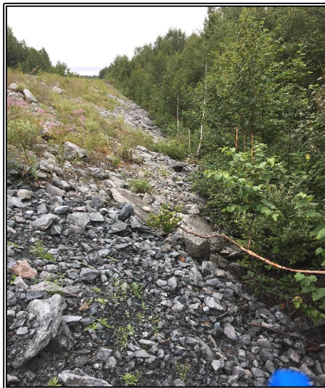
Photo 8 : Dam 1A – General view of vegetative growth at the toe of the embankment.
