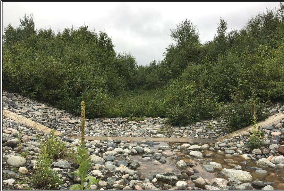
Photo 5 : Dam 1D – Concrete sill and upstream spillway channel at the TSF emergency spillway. Vegetation was cleared in 2020.
