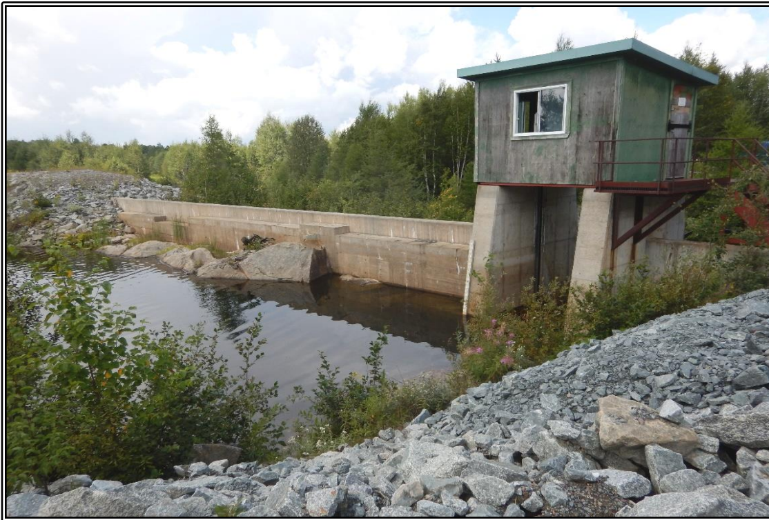
Photo 13 : Dam 4B – View of main spillway control structure and concrete outflow section adjacent to it. Good condition.
