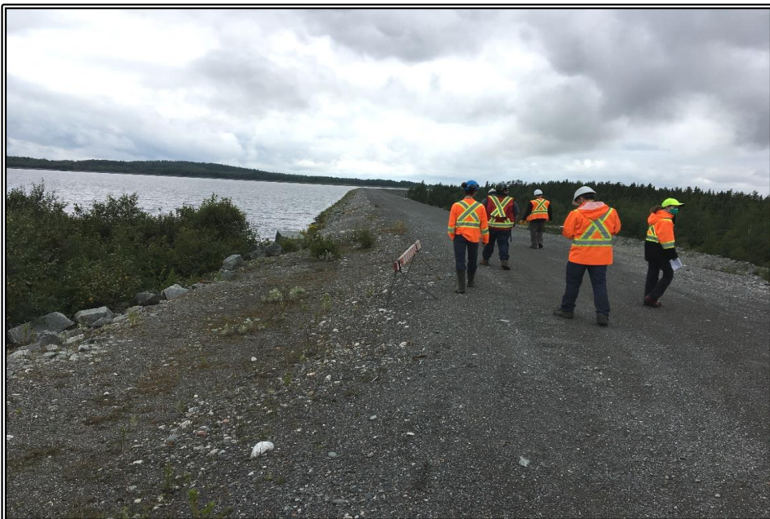
Photo 2 : Dam 1C – Degraded rip rap area on the upstream slope. View looking West.
