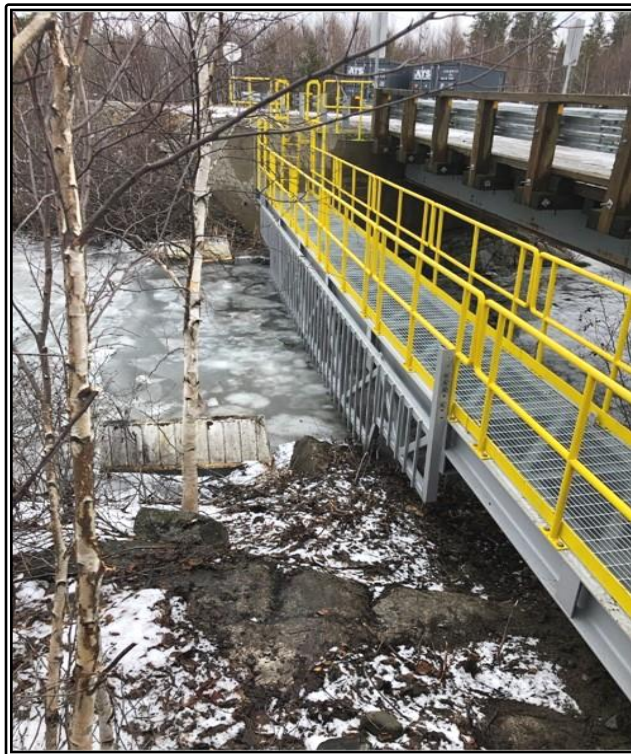
Photo 4 : Dam 1E – New trash rack structure upstream from the TSF operational spillway, installed in November 2020.
