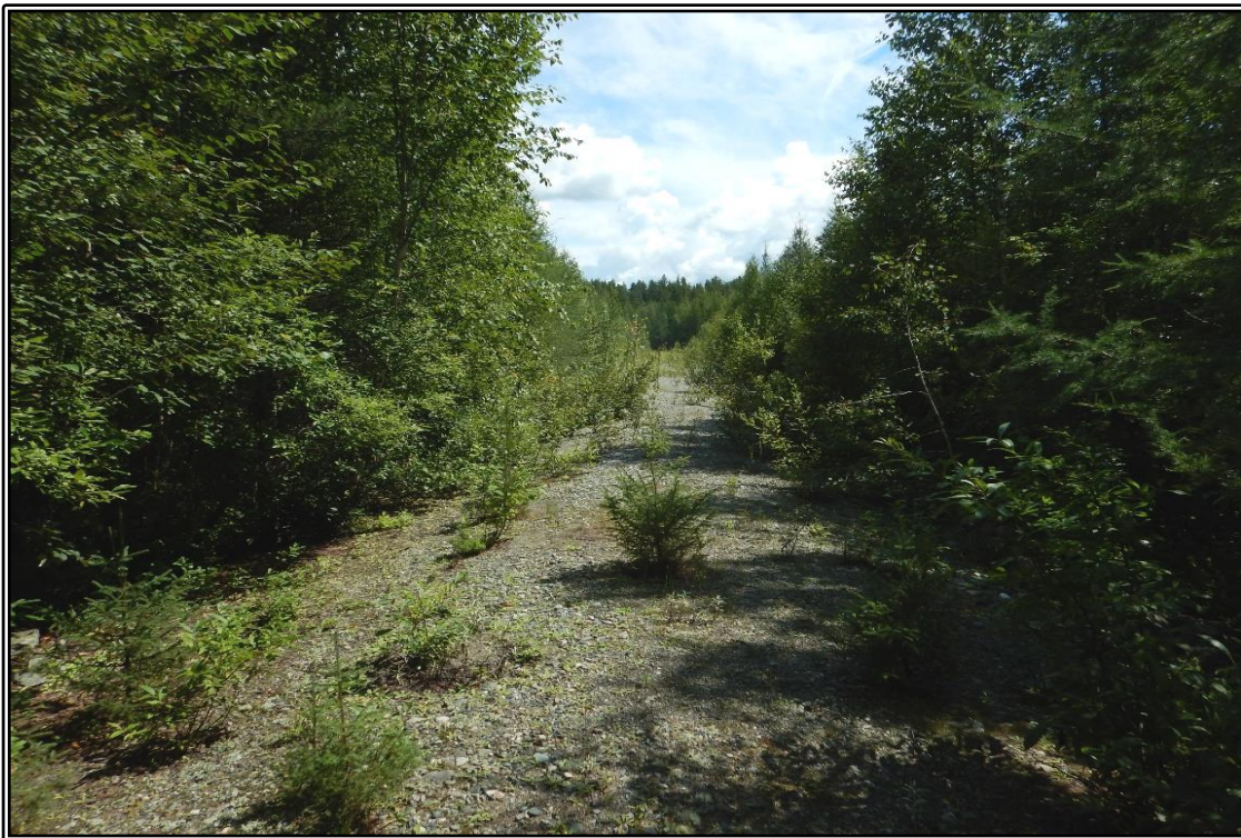
Photo 12 : Dam 4A – Vegetation on the side slopes and crest of the embankment.
