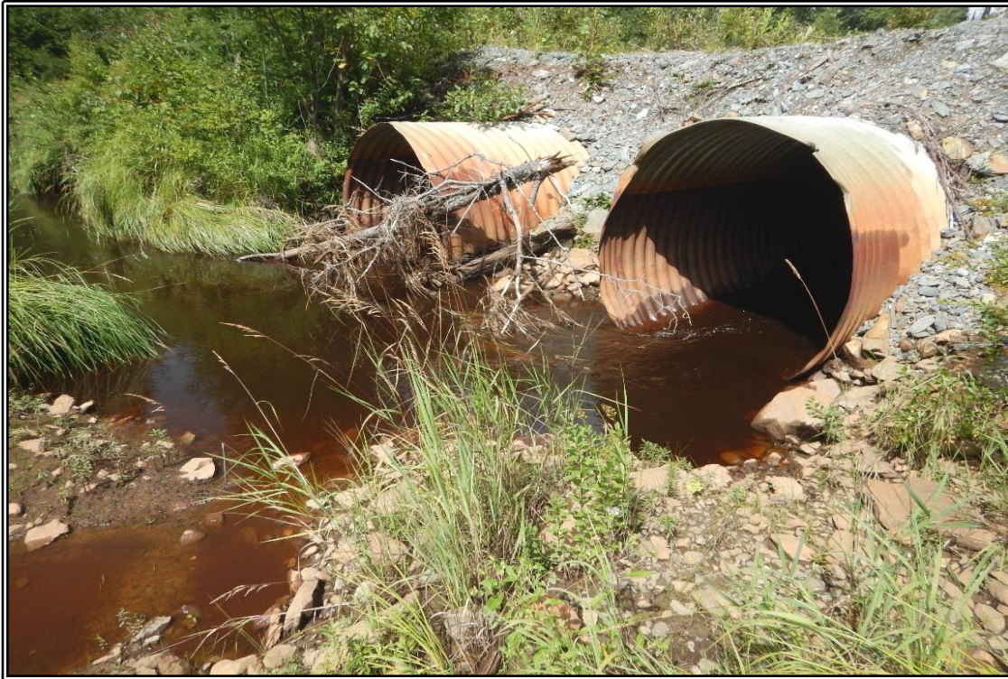
Photo 11 : Dam 2B - Culverts located northwest of the TSF - Drainage improved after clearing during last year.
