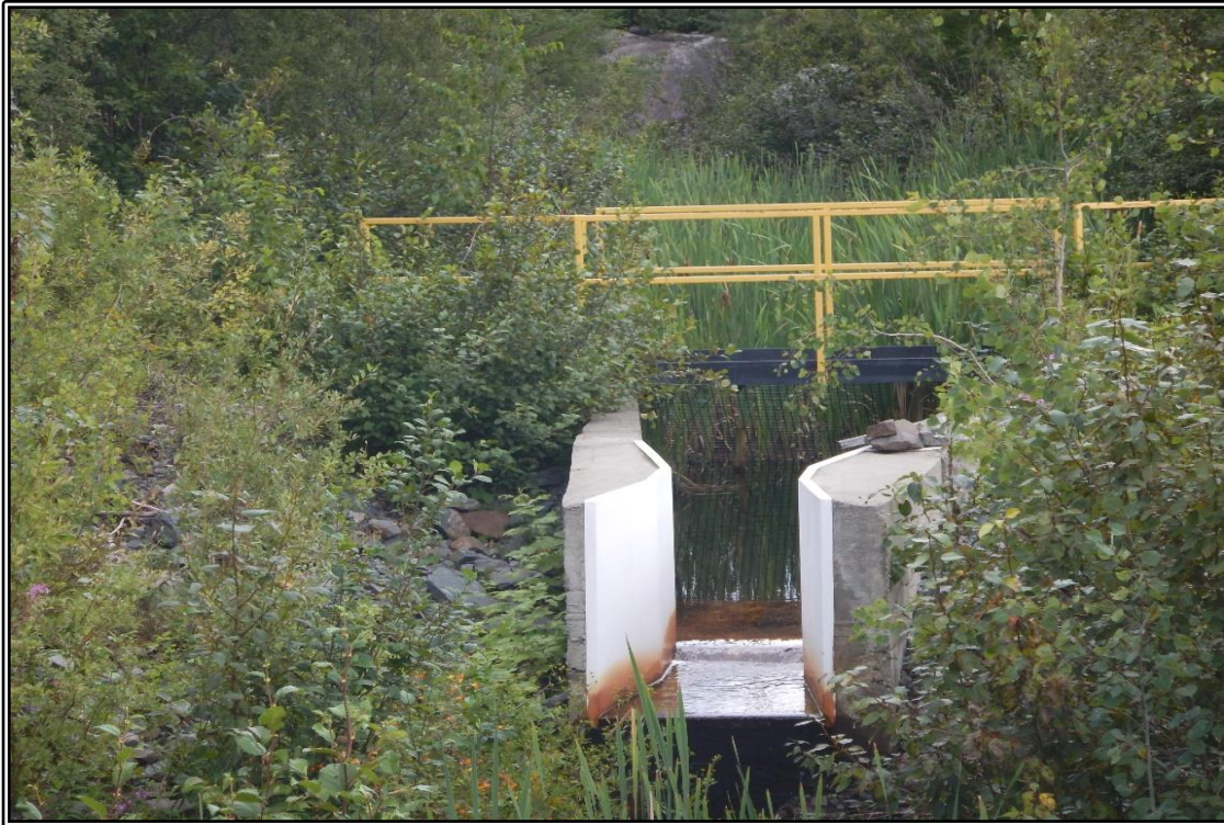
Photo 15 : Dam 4B – Vegetation at the outflow channel from the spillway to the Parshall flume.
