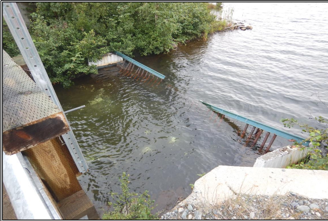
Photo 3 : Dam 1E – Damaged trash rack structure upstream from the TSF operational spillway, before a new installation in November 2020.
