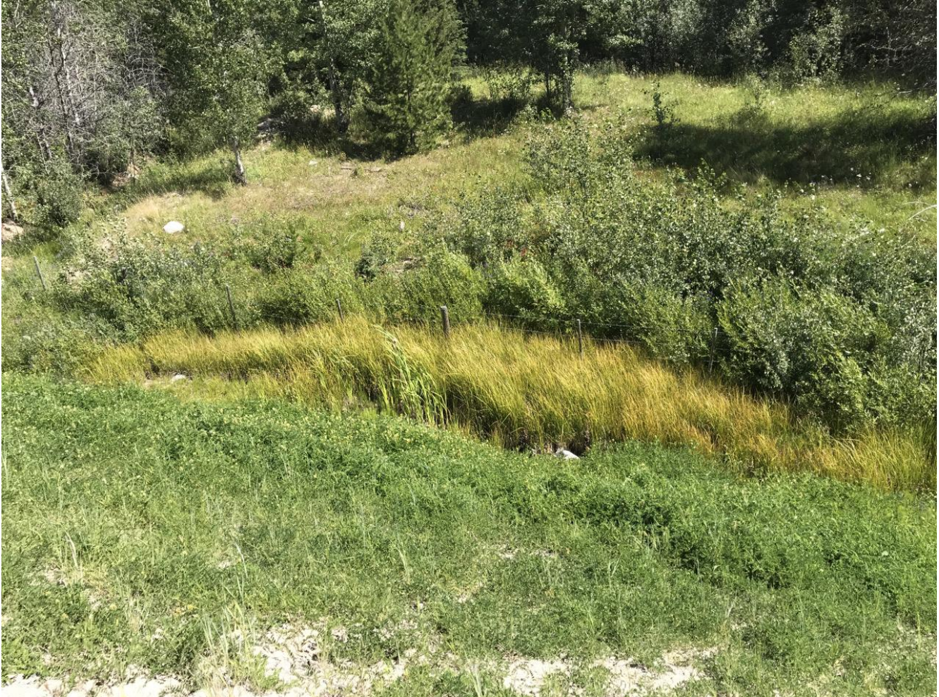
Photo I-B-42 S5 Pond: Downstream toe of perimeter crest. Change of vegetation suggests there has been temporary ponding at the toe likely due to the run-off (HGH-2020-48)
