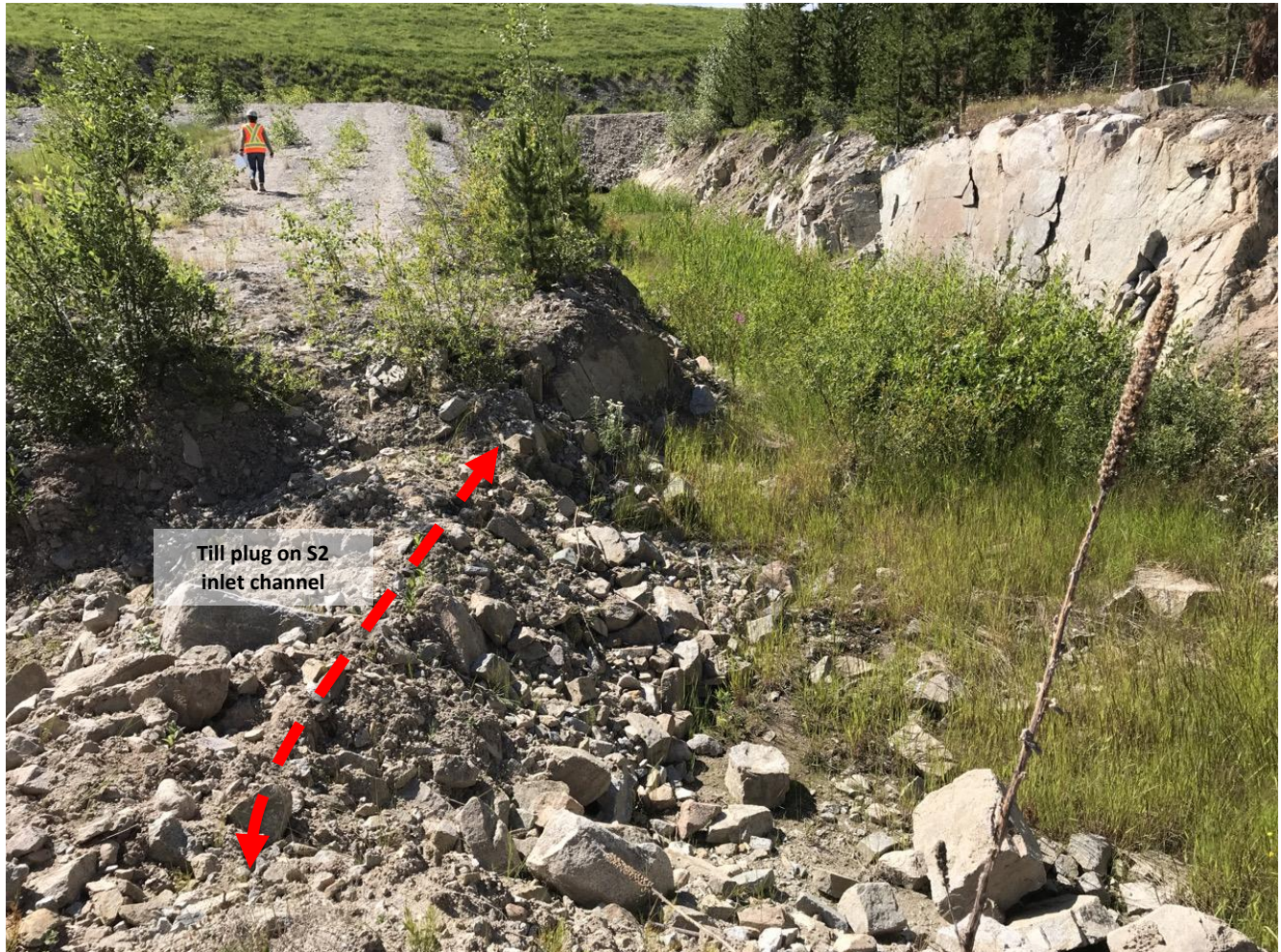
Photo I-B-14 S2 Pond: Till plug (~1.2 m high and ~ 1m wide) is placed in S2 inlet channel. Highmont TSF Spillway diversion channel is heavily vegetated. Vegetation was removed after the site visit as part of routine maintenance (HGH-2020-27)
