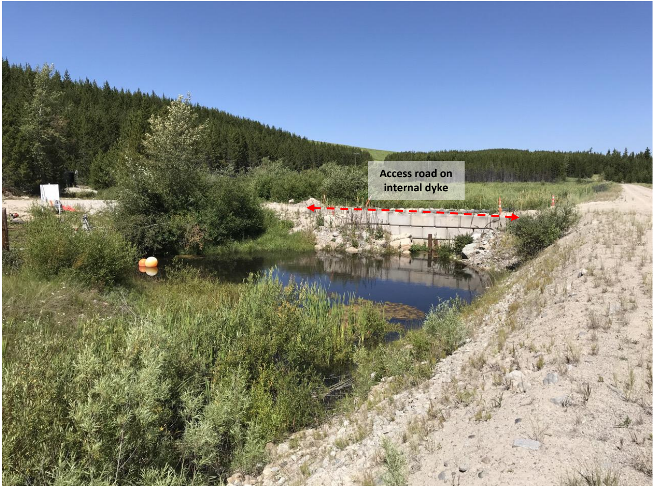
Photo I-B-35 S5 Pond: Overview of Pumping Sub-cell. Water was ponding in the spillway channel (HGH-2020-42)
