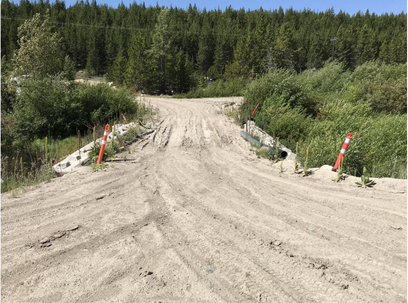
Photo I-B-32 S5 Pond: View of access road on the divider dyke. Minor rutting observed on crest of divider dyke is managed under routine maintenance (HGH-2020-39)
