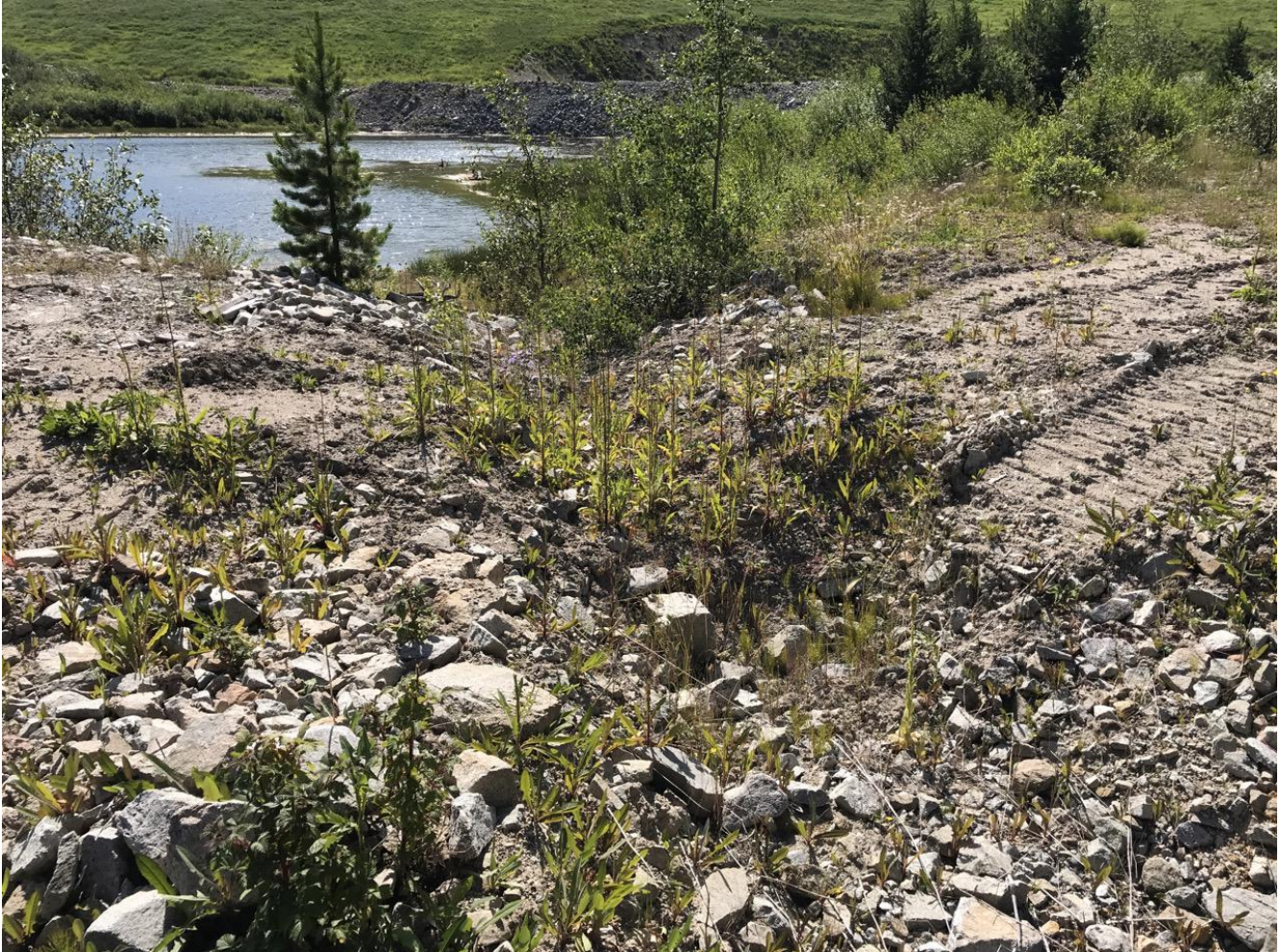
Photo I-B-16 S2 Pond: S2 Pond Spillway approach channel; remnant of a temporary access built over the channel remains in place which has reduced the spillway flow channel and should be removed as part of routine maintenance before freshet. Vegetation was removed after site visit as part of routine maintenance (HGH-2020-29)
