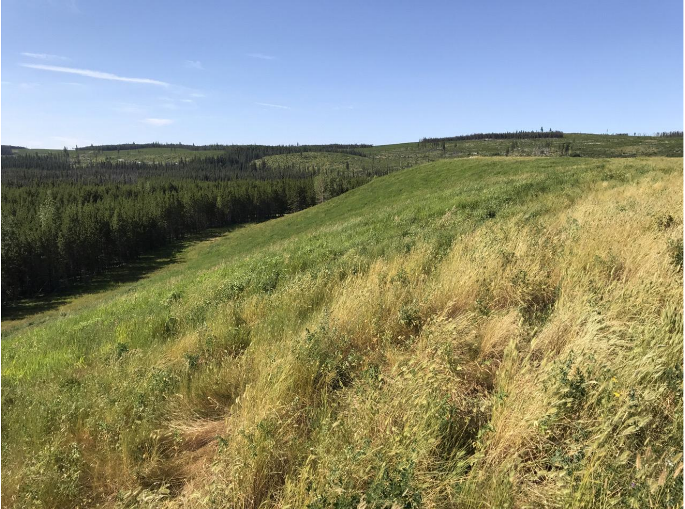
Photo I-A-15 View of South Dam downstream slope looking southwest. Slope is vegetated and in good condition (HGH-2020-09)
