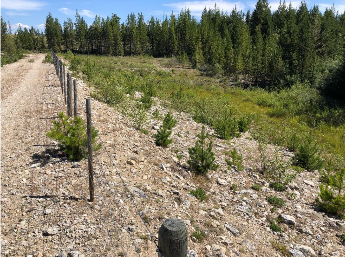
Photo I-B-24 S3 Pond: Overview of downstream slope with small trees from mid dam (HGH-2020-33)
