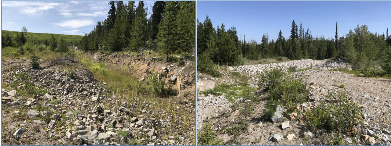
Photo I-B-17 S2 Pond: View of Highmont spillway channel. Channel is in good condition. Excess vegetation was removed after site visit as part of routine maintenance (HGH-2020-30)
