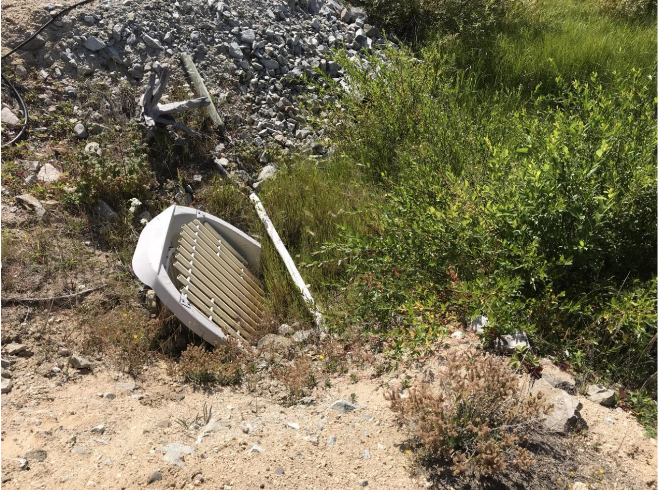
Photo I-B-49 S8 Pond: Overview of overflow pipe trash rack. Rack is clear of debris. Current water level is below the invert (HGH-2020-49)
