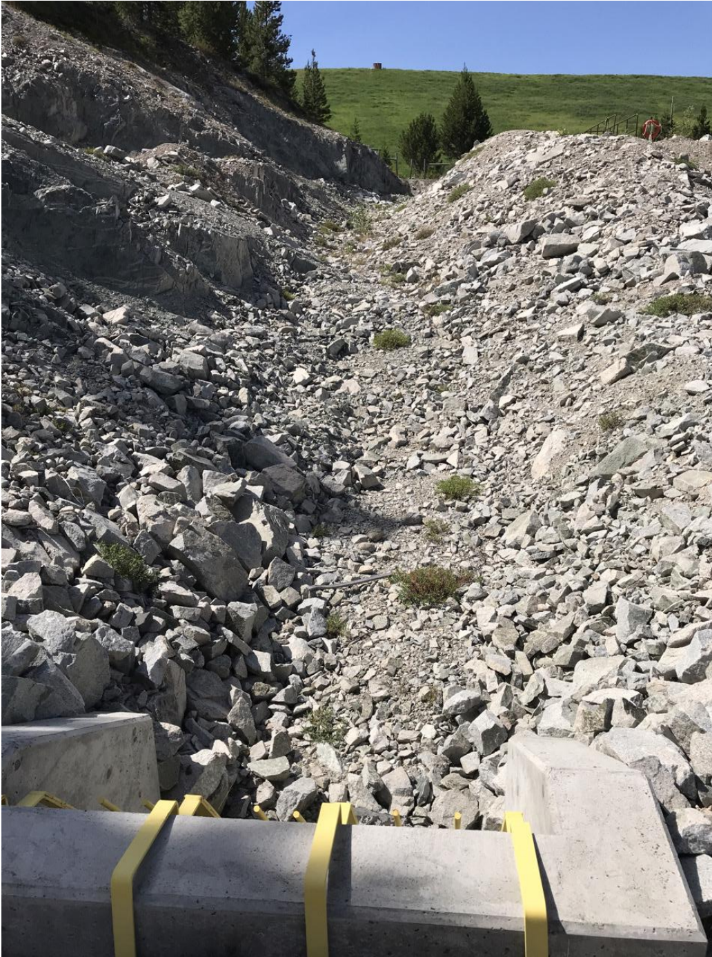
Photo I-B-6 S1 Pond: Spillway channel upstream of pipe intake, looking toward the pond (HGH-2020-22)
