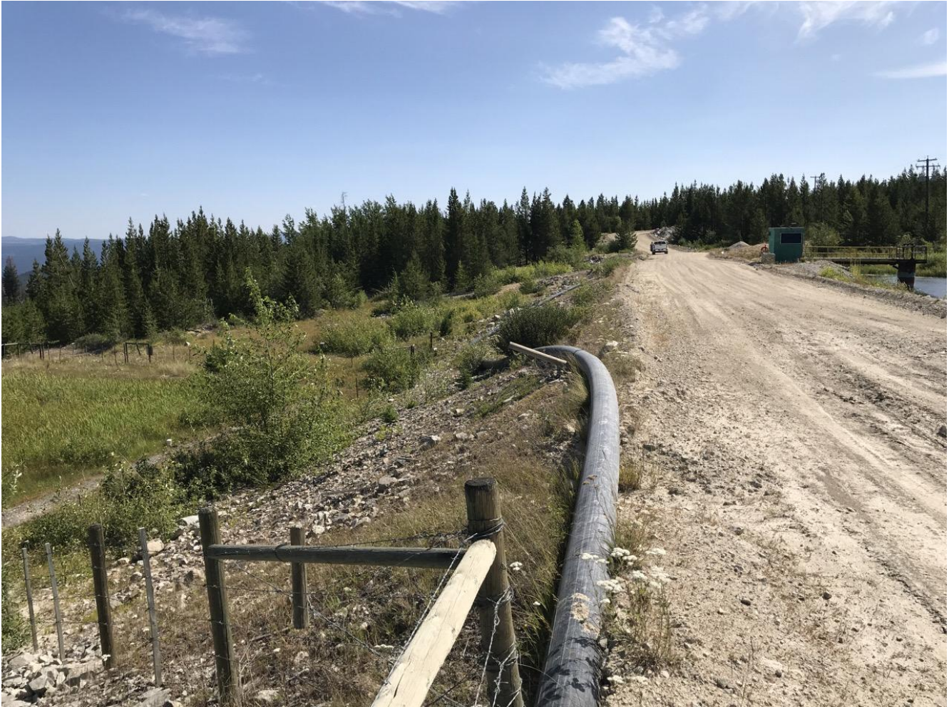
Photo I-B-45 S8 Pond: Downstream slope, looking east from left abutment. THVCP confirmed there are no potential hookups for the pipe in the current location. Therefore, the pipe presents no risk to the S8 Pond (HGH-2020-07)
