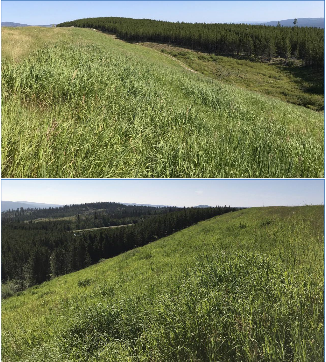
Photo I-A-12 East Dam downstream slope. Slope is vegetated and in good condition (HGH-2020-08)
