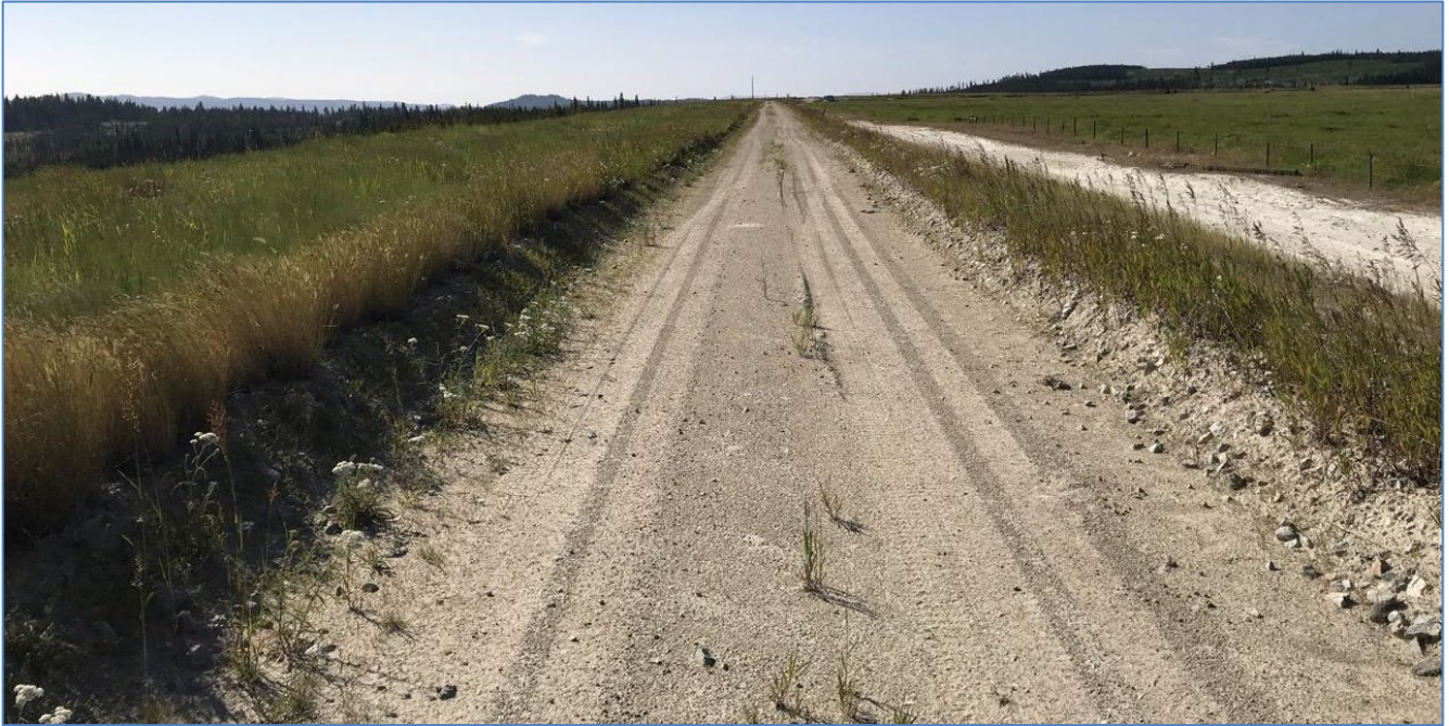
Photo I-A-7 East Dam crest. Crest is in good condition. No signs of deformation or distress were observed (HGH-2020-02)
