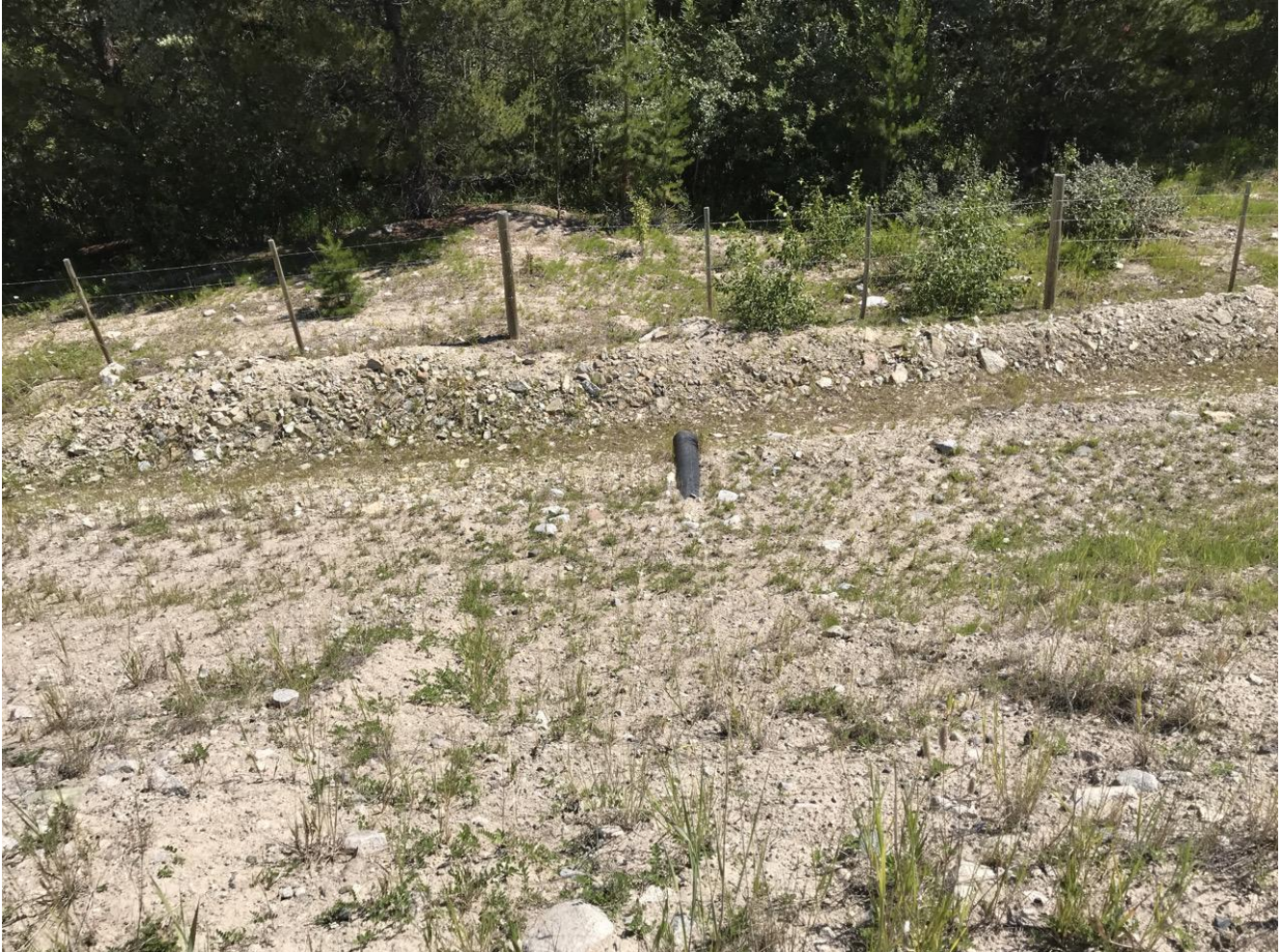
Photo I-B-39 S5 Pond: Overview of downstream slope and Outlet #2 pipe daylighting at toe, looking east (HGH-2020-45)
