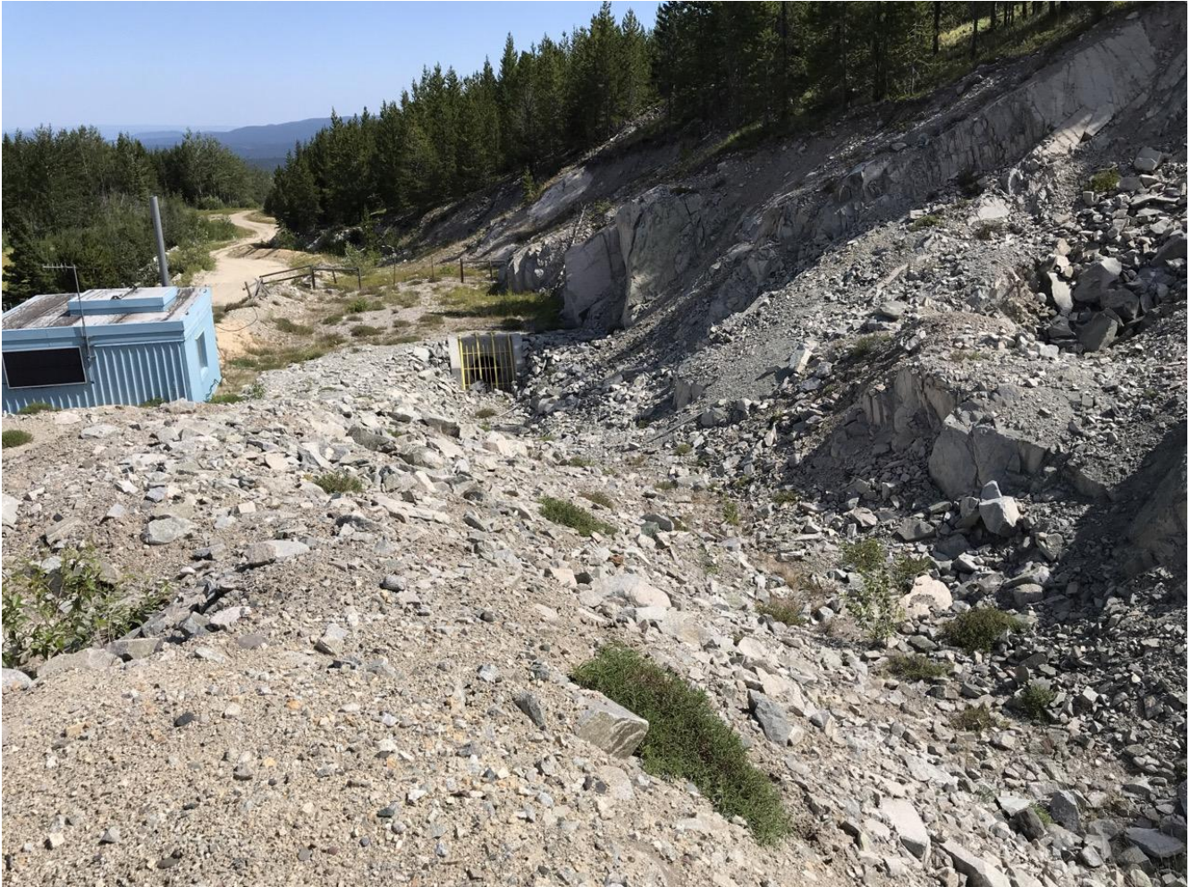
Photo I-B-5 S1 Pond: Spillway channel and pipe intake looking downstream. Channel is clear of vegetation and no sign of obstruction was observed at the pipe intake (HGH-2020-20)
