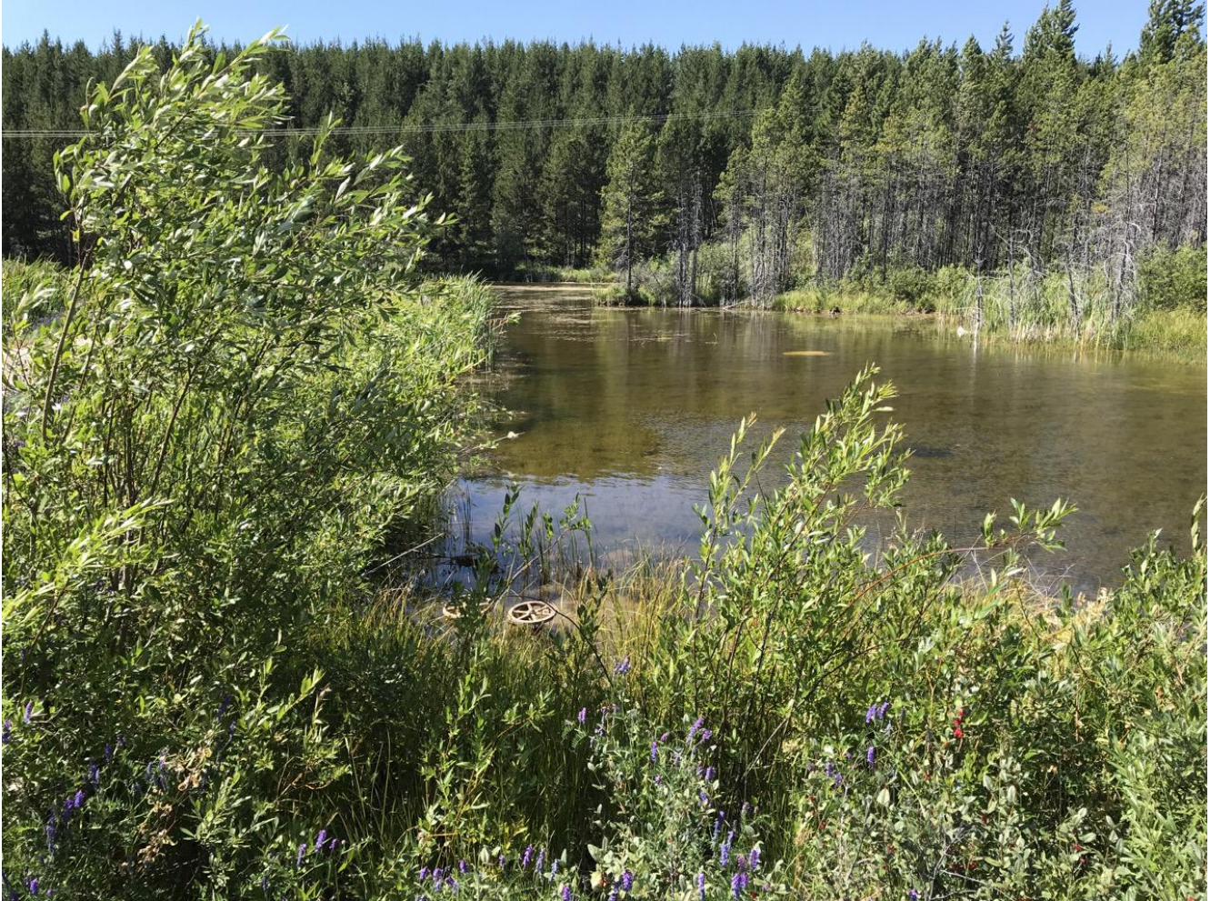
Photo I-B-34 S5 Pond: S5 Pond north outlet pipe, permanently sealed. Metal plates placed at intake and pipes filled with till in 2015 (HGH-2020-41)
