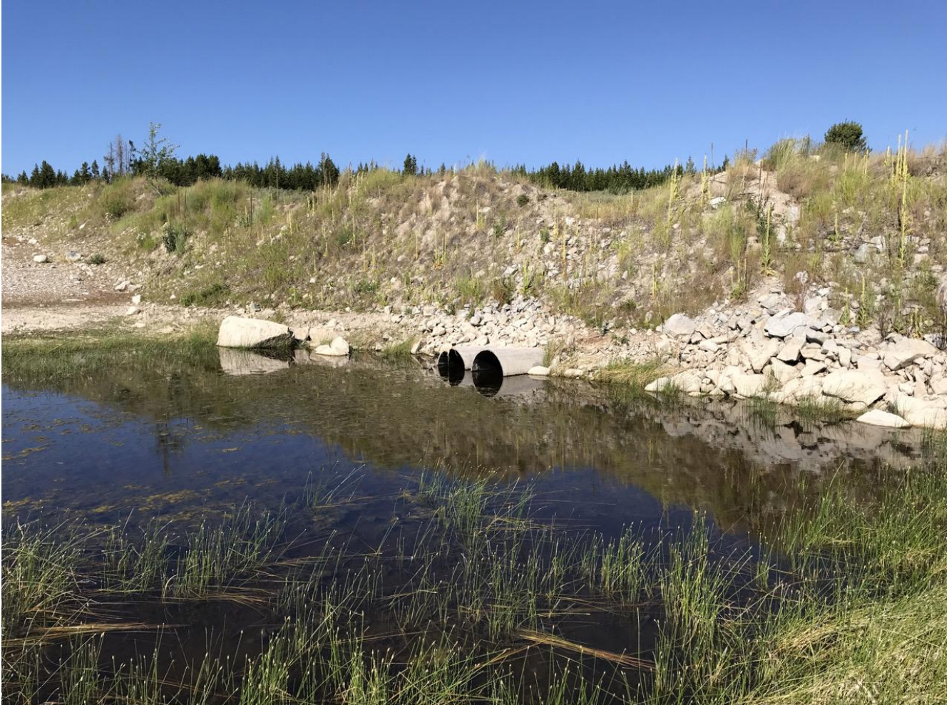
Photo I-A-20 Approach channel. Road culverts are partially submerged, section upstream of culverts is clear of debris and vegetation (HGH-2020-11)
