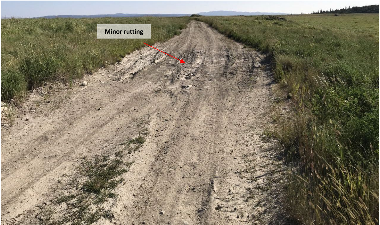
Photo I-A-4 North Dam crest is in good condition. No signs of distress, settlement or depression; minor rutting observed is managed under routine maintenance (HGH-2020-01)
