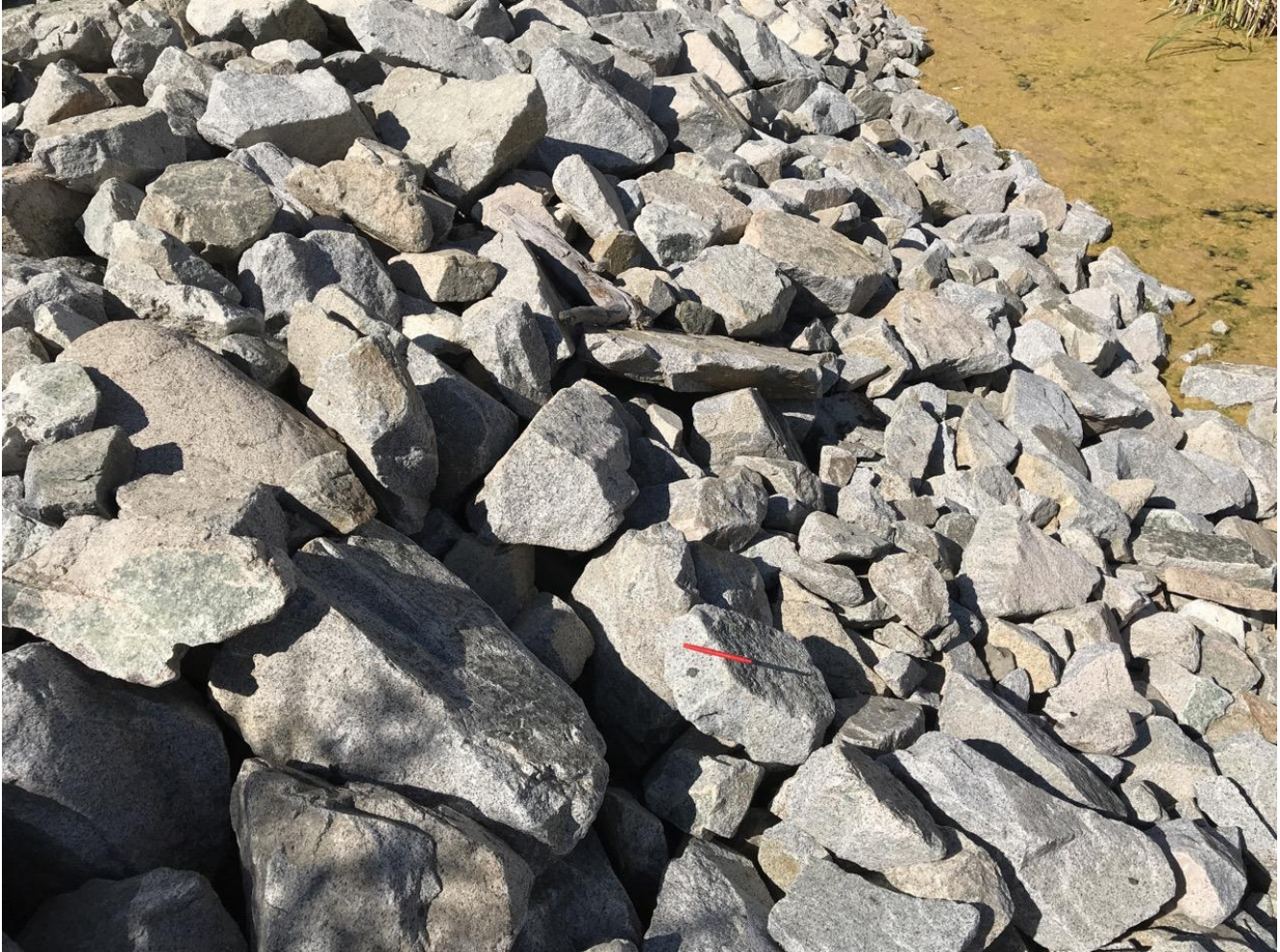
Photo I-A-32 Riprap at spillway stilling pond and channel with maximum size of approximately 1 m (HGH-2020-18)
