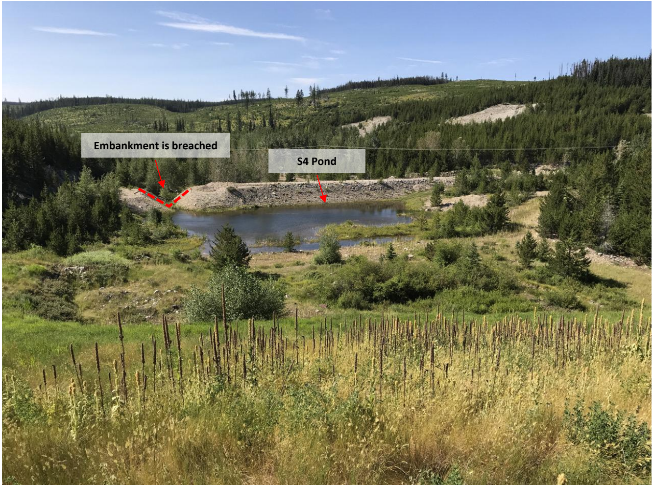
Photo I-A-17 South Dam downstream slope and view of S4 Pond from South Dam. S4 embankment is breached (HGH-2020-03)
