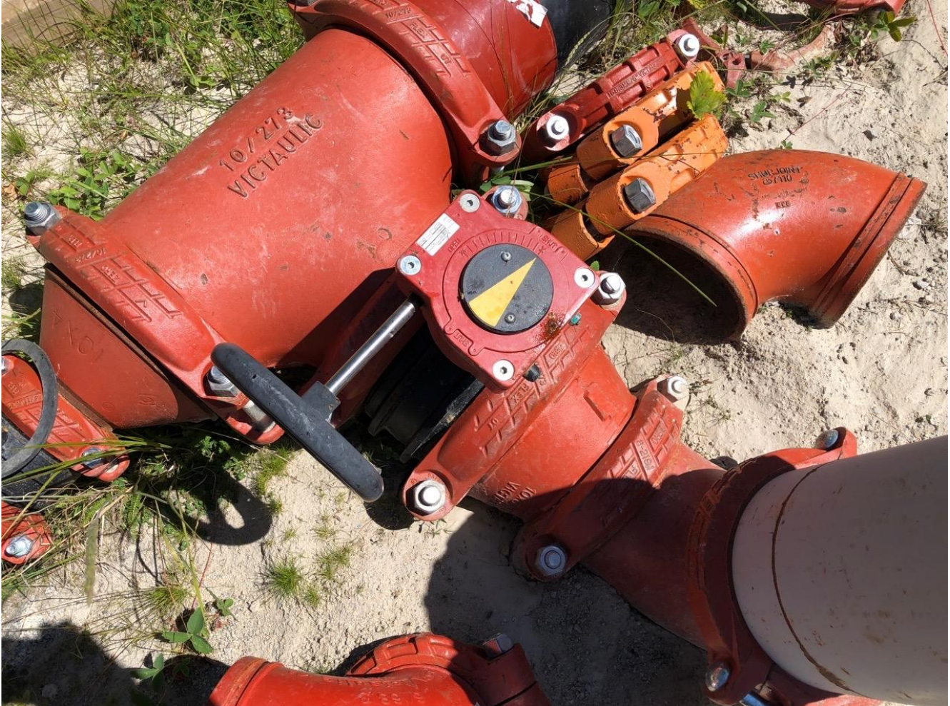
Photo I-B-30 S3 Pond: S3 inlet pipe valve works. System is clear and easily understandable (HGH-2020-38)
