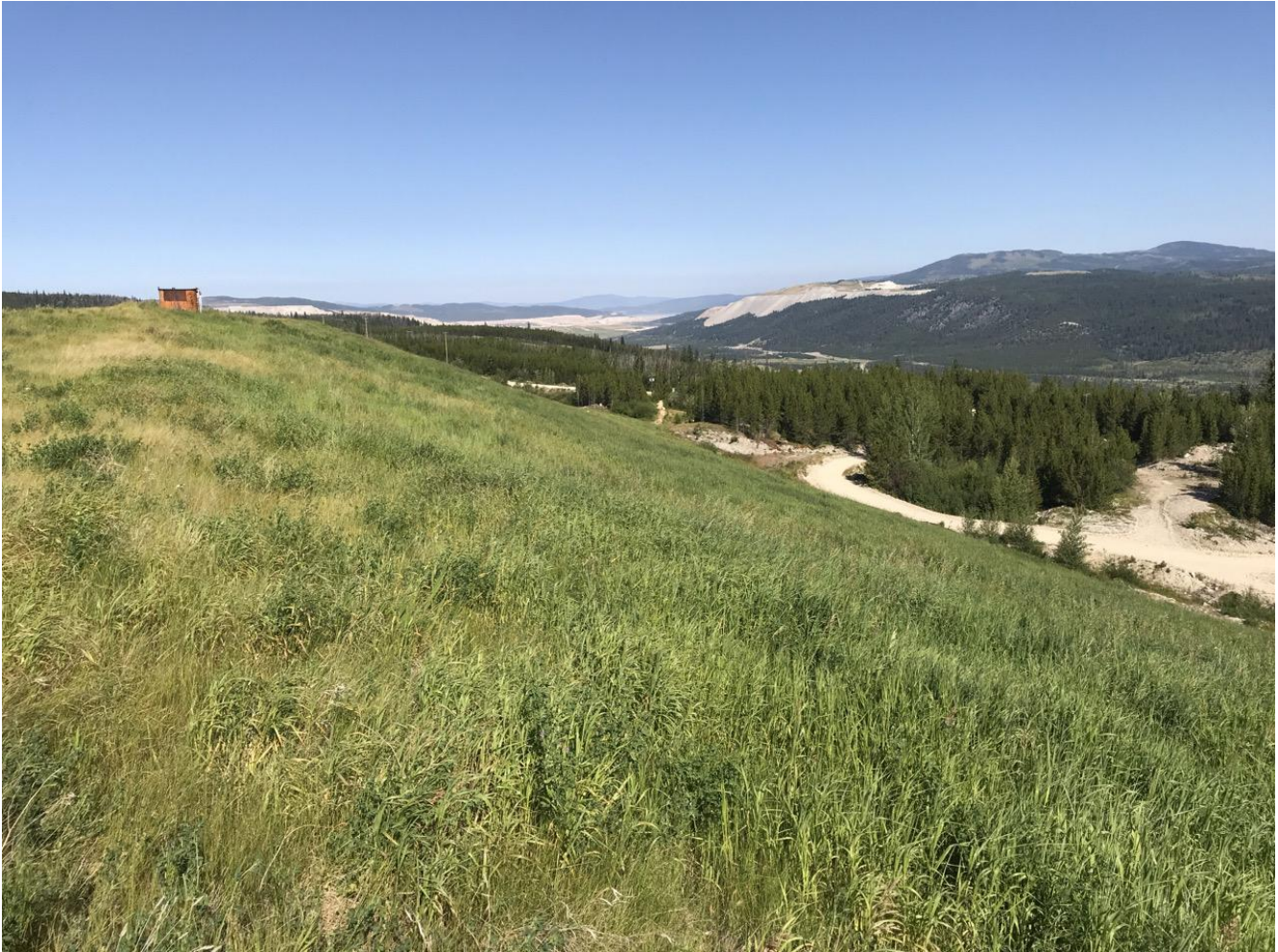
Photo I-A-8 View of North Dam downstream slope looking northwest. Vegetation was about 0.5 m tall which made inspection difficult, but no signs of distress or deformation were observed (HGH-2020-06)
