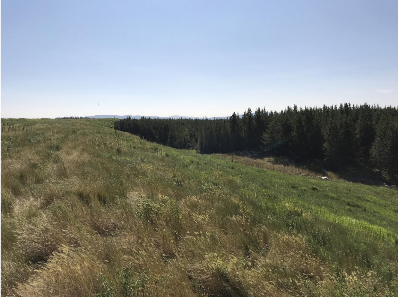
Photo I-A-16 View of South Dam downstream slope at right abutment looking east. Slope is vegetated and in good condition (HGH-2020-03)
