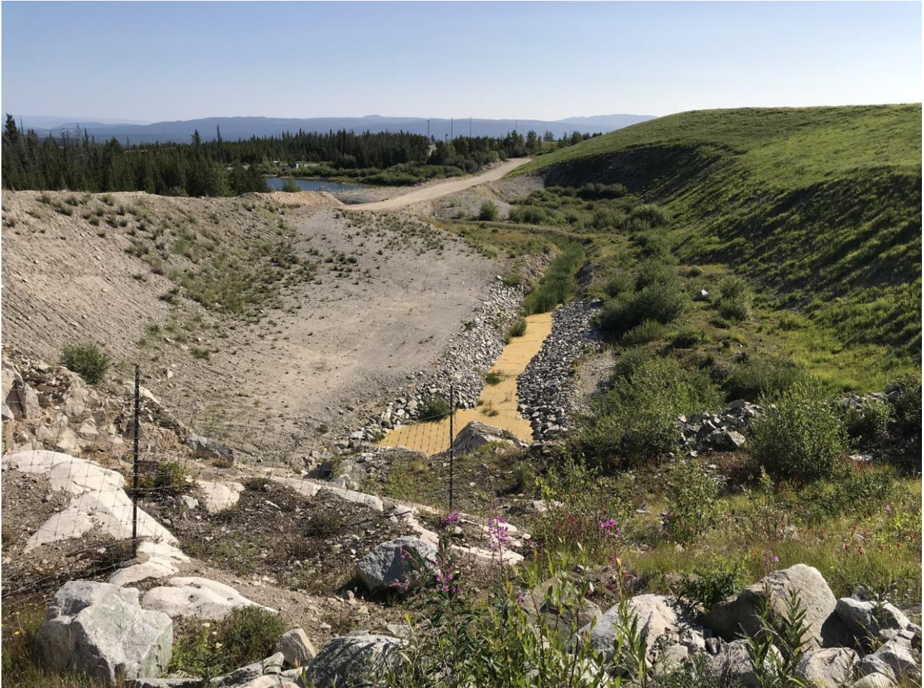
Photo I-A-28 Highmont Spillway channel downstream of spillway drop. Channel is in good condition. North Dam downstream toe is visible. No signs of distress or deformations (HGH-2020-16)
