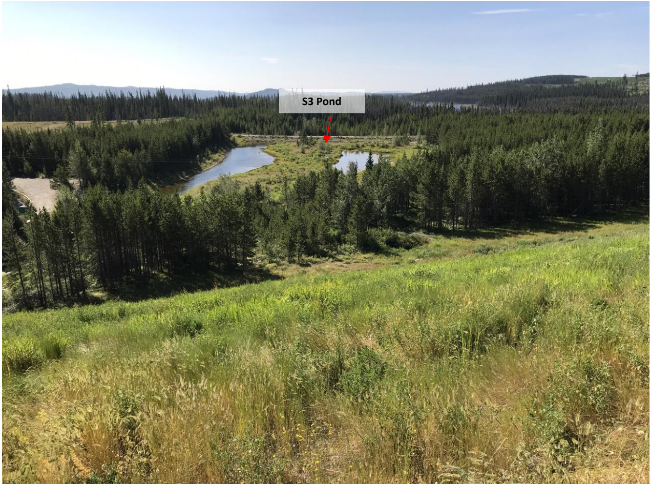
Photo I-A-14 South Dam downstream slope and view of S3 Pond downstream of the dam with two pools of water. South Dam slope is vegetated and in good condition (HGH-2020-09)
