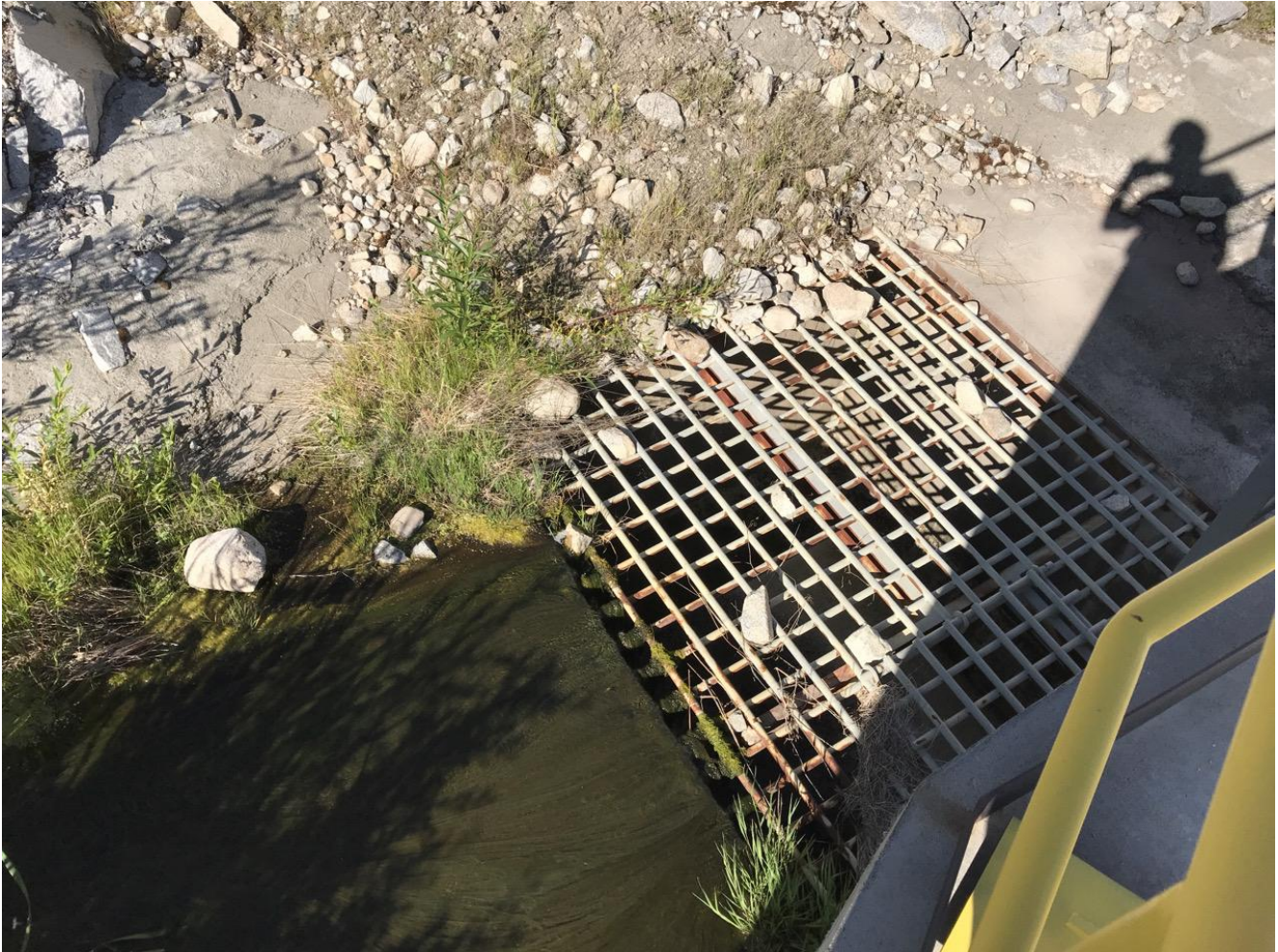
Photo I-A-24 Highmont Spillway channel, S1 Pond diversion trash rack. Minor flow into the diversion. Trash rack is clear of debris. No flow downstream of diversion (HGH-2020-15)
