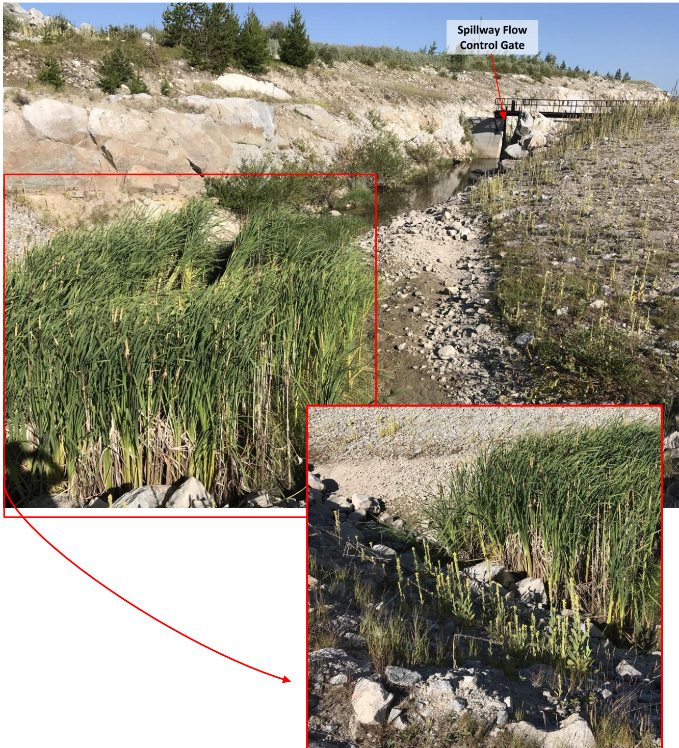
Photo I-A-21 Area downstream of approach channel culverts and upstream of flow control gate – Culverts and channel are partially obstructed by vegetation which should be removed as part of routine maintenance (HGH-2020-12)
