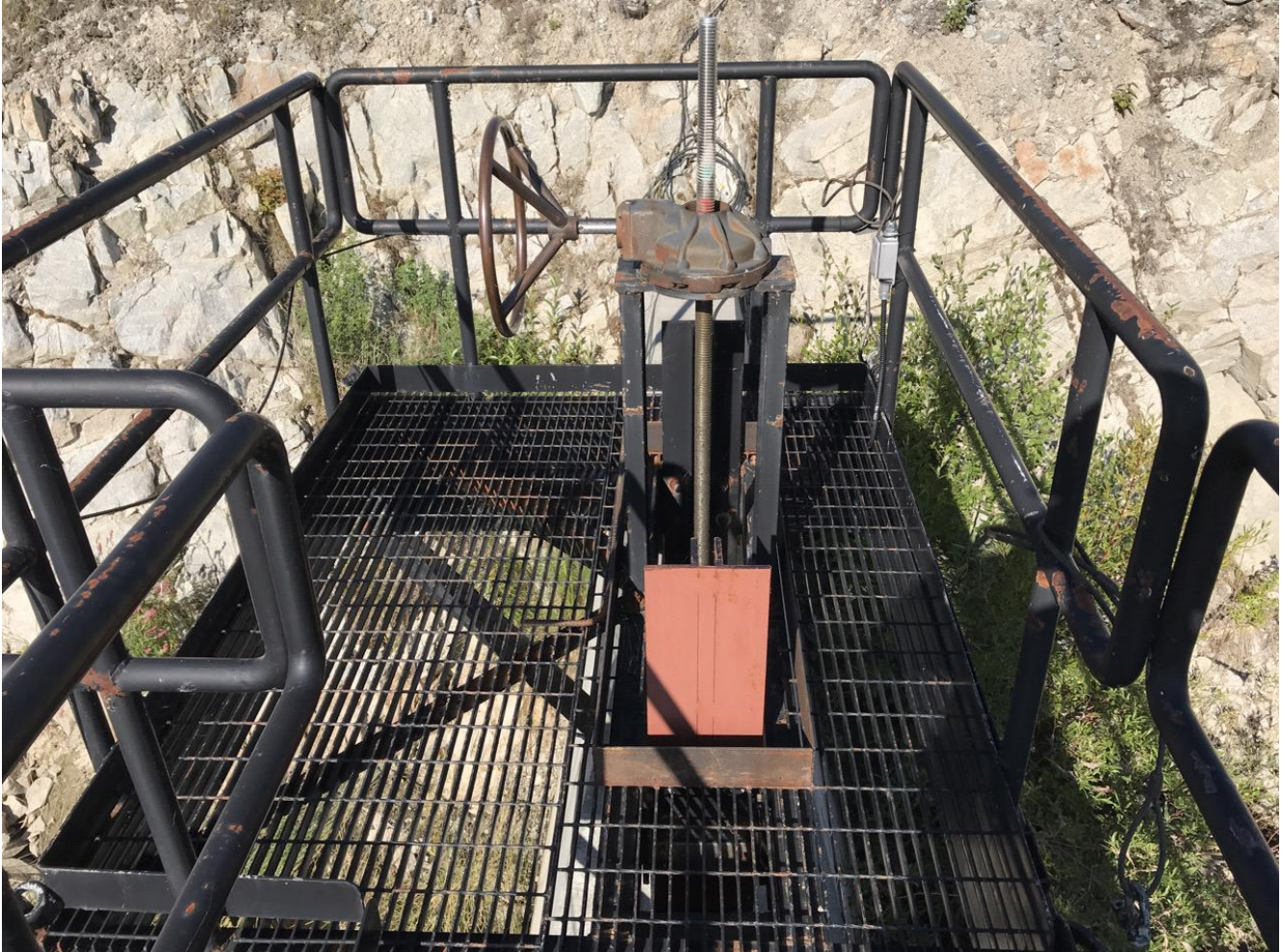
Photo I-A-22 Spillway flow control gate. Valve is operational and could move up and down (tested for slight movement). Sliding gate is slightly open (HGH-2020-13)
