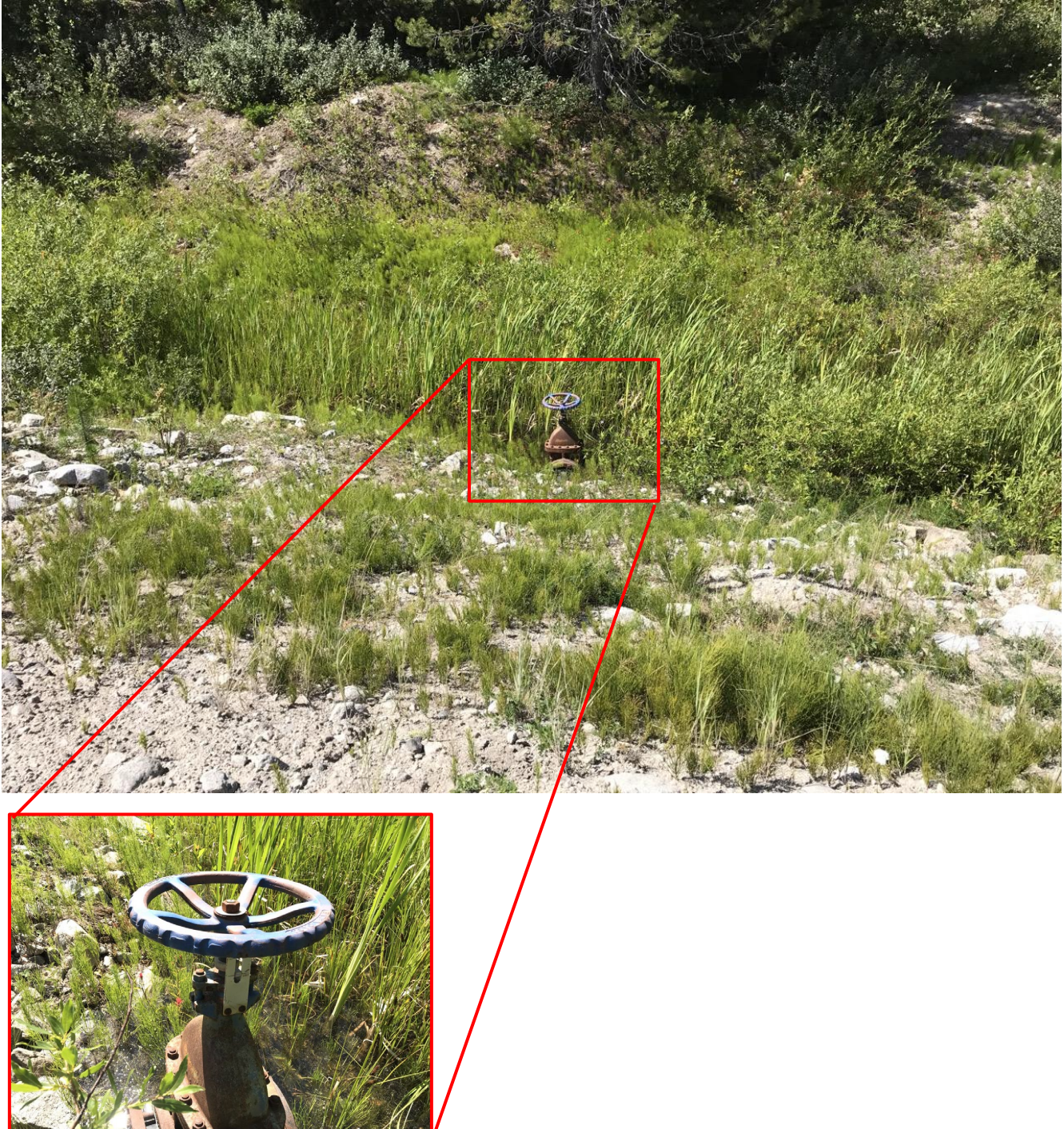
Photo I-B-38 S5 Pond: Pumping Sub-cell Outlet #2 (South). Metal plates placed at intake and pipes filled with till in 2015 (HGH-2020-45 and HGH-2020-46)
