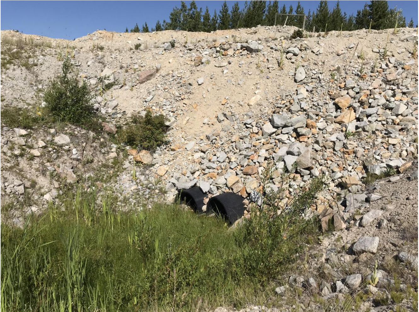
Photo I-A-33 North Dam toe access road crossing culverts. Culverts are misshapen (HGH-2020-17)
