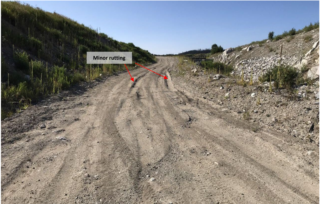
Photo I-A-5 North Dam crest access road to S1 Diversion. Minor rutting observed is managed under routine maintenance (HGH-2020-04)
