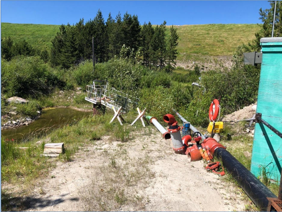
Photo I-B-29 S3 Pond: Catwalk and outlet pump to Highmont Distribution Box, personal flotation device is in place (HGH-2020-36 and HGH-2020-37)
