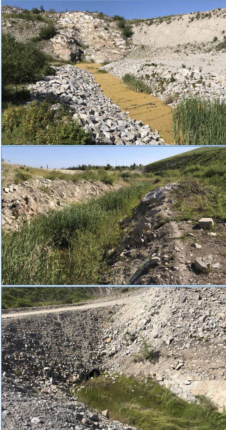
Photo I-A-31 Water is ponded downstream of spillway drop. Vegetation obstructing spillway channel (HGH-2020-18 and HGH-2020-19)
