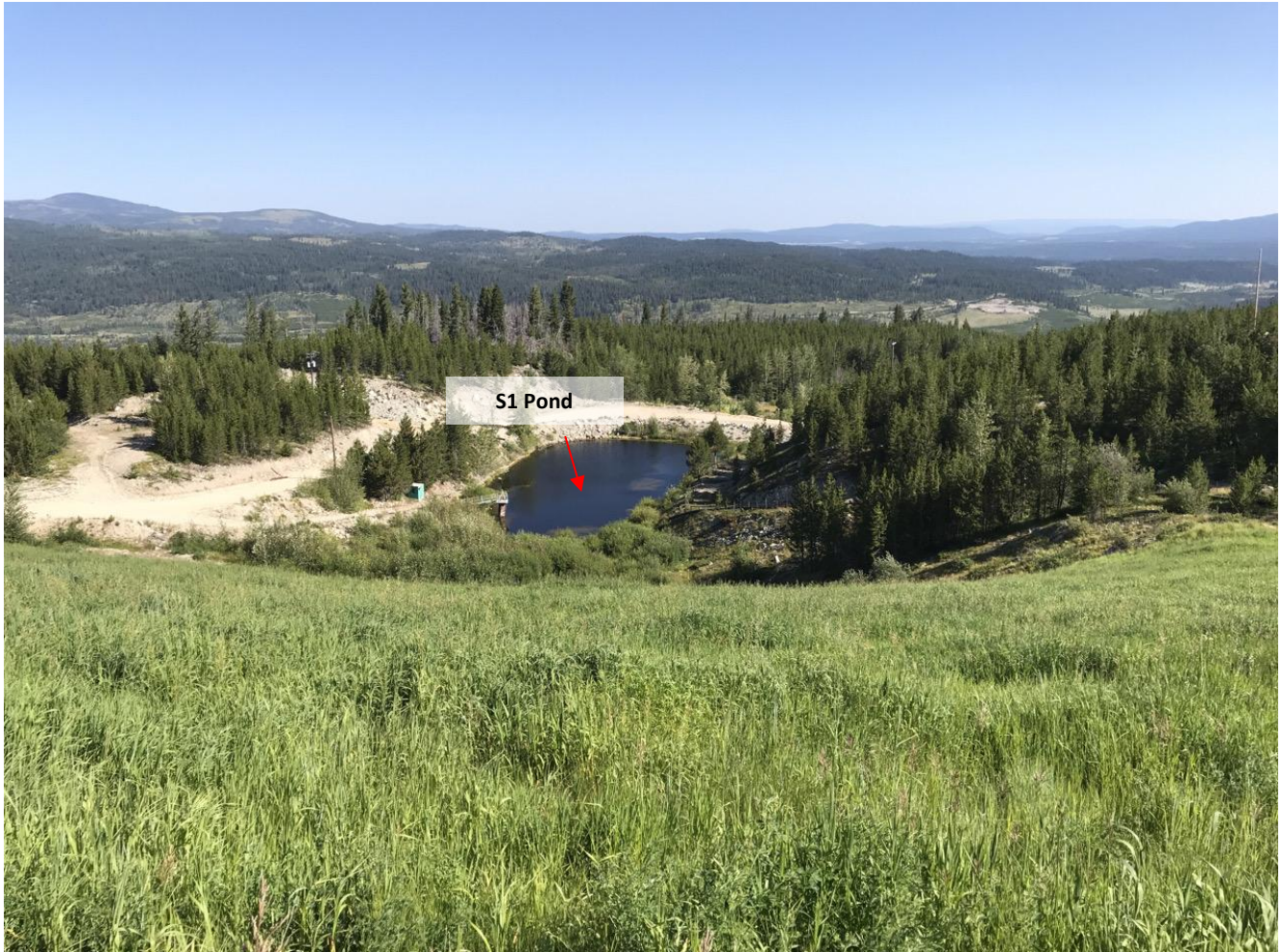
Photo I-A-9 View of North Dam downstream toe and S1 Pond. No signs of distress or deformation were observed (HGH-2020-06)
