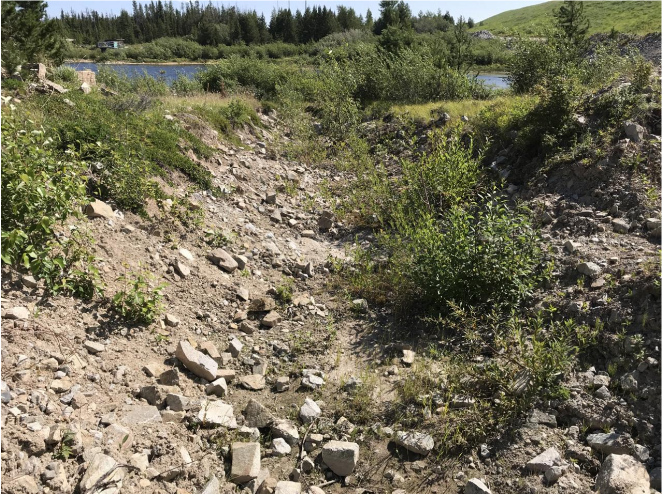
Photo I-B-15 S2 Pond: S2 Pond inlet and channel from Highmont Spillway Diversion. Channel and the inlet are heavily vegetated. Vegetation was removed after the site visit as part of routine maintenance (HGH-2020-28)
