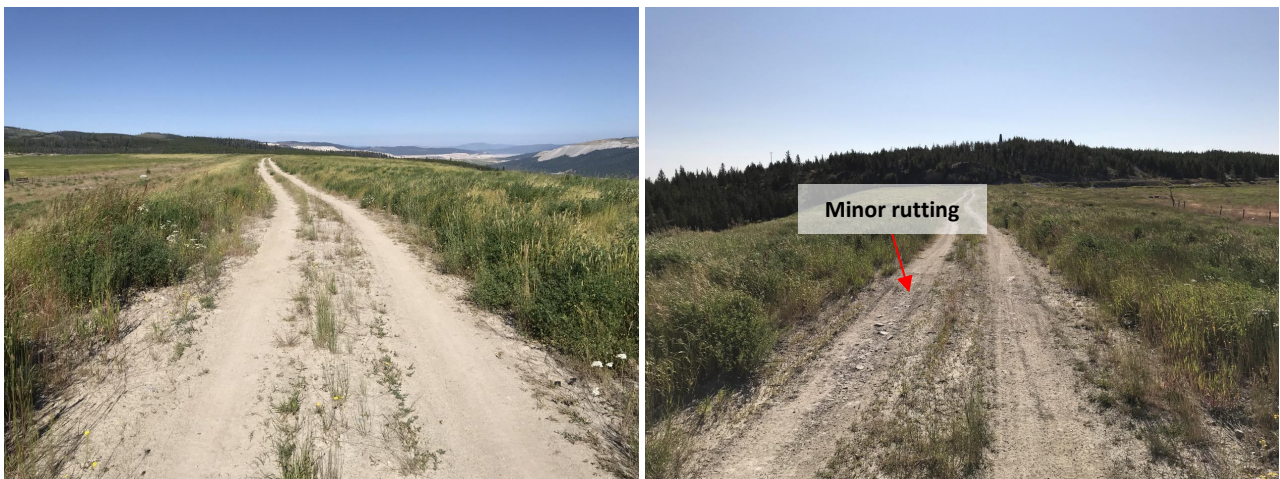
Photo I-A-6 North Dam crest near right abutment. Crest is in good condition. Minor rutting observed in access road is managed under routine maintenance (HGH-2020-05)
