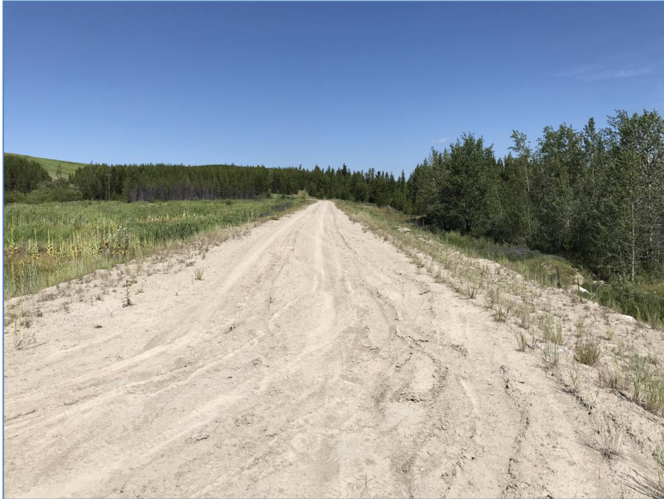
Photo I-B-31 S5 Pond: Overview of crest. Minor rutting observed on crest and access road is managed under routine maintenance (HGH-2020-39)
