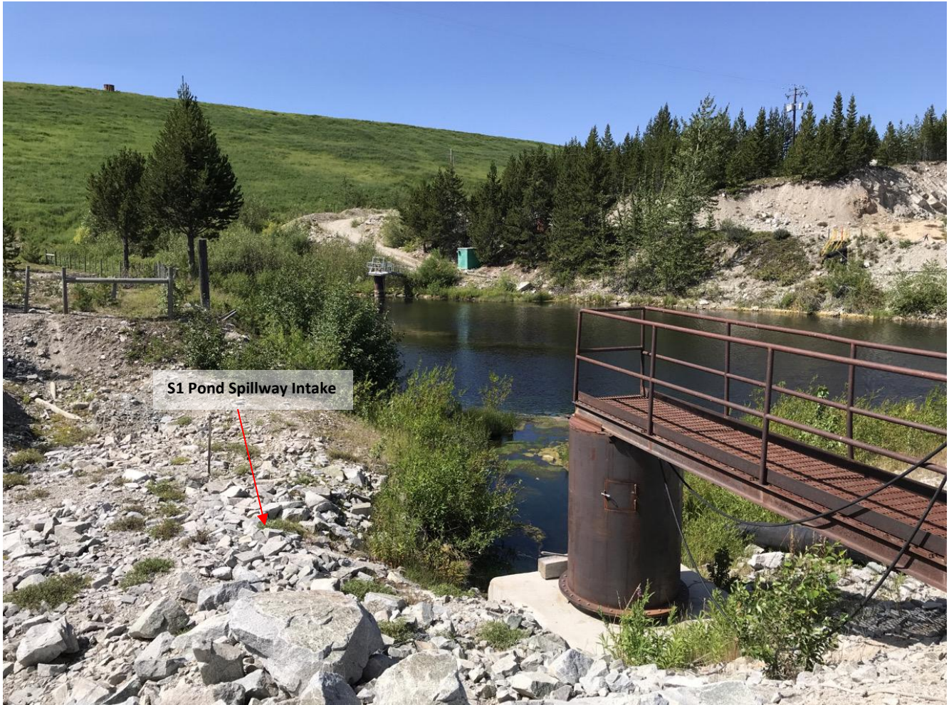
Photo I-B-3 S1 Pond: View of S1 Pond, Spillway intake, and Low-Level Outlet (LLO) (HGH-2020-20)
