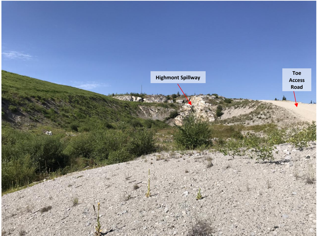
Photo I-A-29 North Dam downstream slope and toe, downstream of Highmont Spillway. North dam toe is in good condition. Spillway stilling basin is heavily vegetated (HGH-2020-17)
