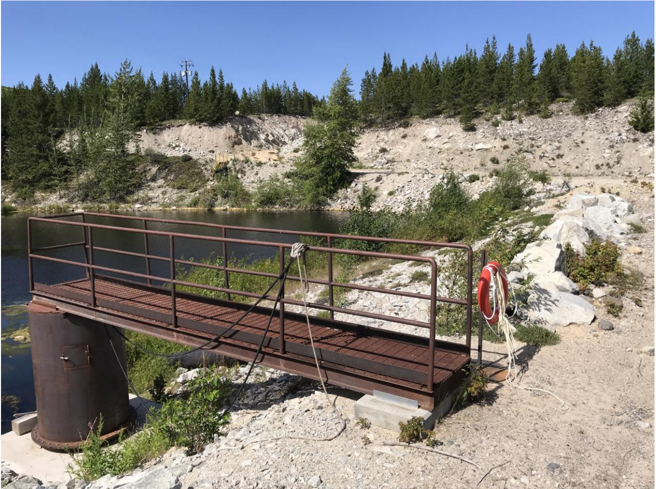
Photo I-B-4 S1 Pond: Low-Level Outlet (LLO) to the left of spillway intake. Pond level was about 1 m below inlet. Vegetation partially obstructing intake; will be cleared during routine maintenance (HGH-2020-20)
