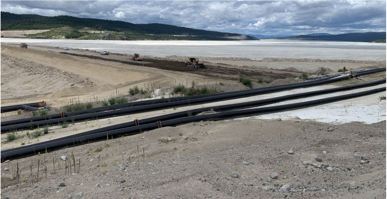
Photo I-B-5 Active spigot point (>500 m) upstream of H-H Dam. No flow towards HH Dam. Wetted beach near the dam is from local runoff (HH-2020-03)
