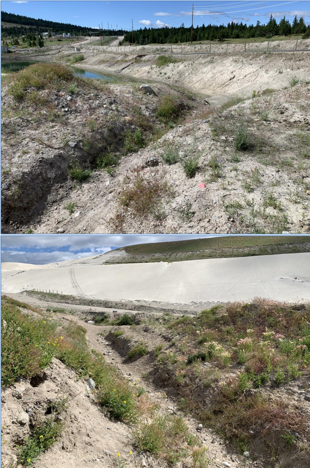
Photo I-A-28 View of channel into Sediment Pond 4 (LL-2020-16)
