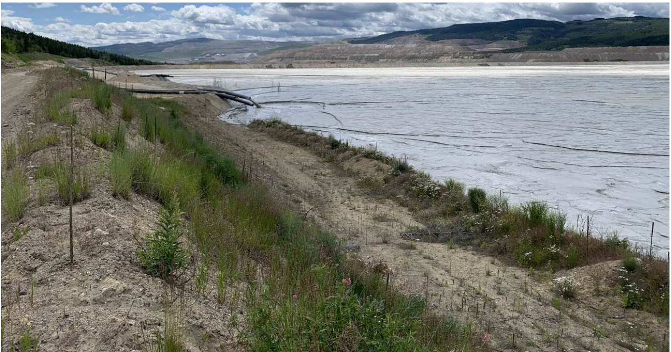
Photo I-B-5 Active spigot point (>500 m) upstream of H-H Dam. No flow towards HH Dam. Wetted beach near the dam is from local runoff (HH-2020-03)
