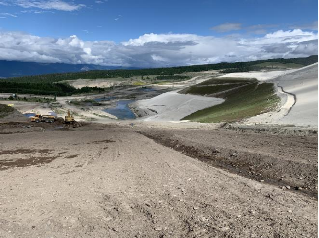
Photo I-A-15 Overview of South Dam downstream foundation area for 2020 fill placement (LL-2020-09)
