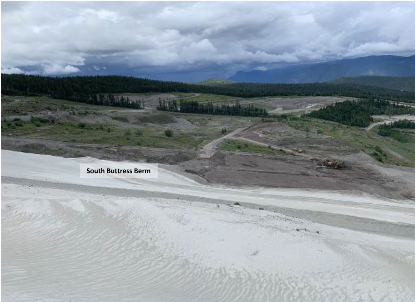
Photo I-A-18 Overview of South Dam foundation area prepared for fill placement, looking south (LL-2020-04)
