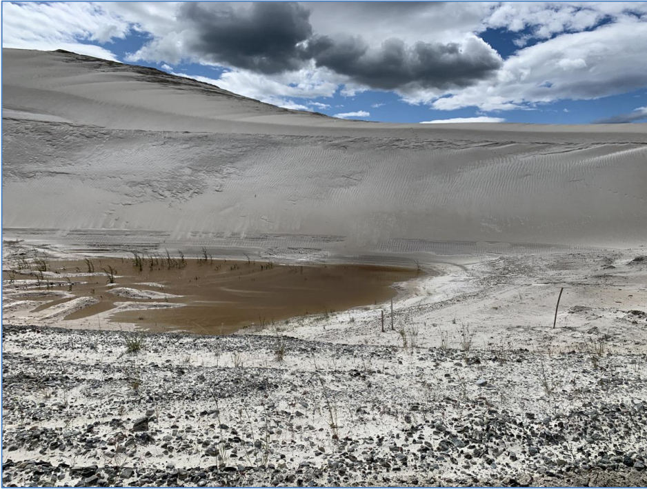
Photo I-A-29 North Buttress Berm low point on north side. Some ponded water was observed which is typical at this location and reoccurs after freshet due to runoff. The ponded water drains draining through the major drain which daylight on north side of NBB. Area is planned to be raised with mechanical placement in 2020 (LL-2020-17)
