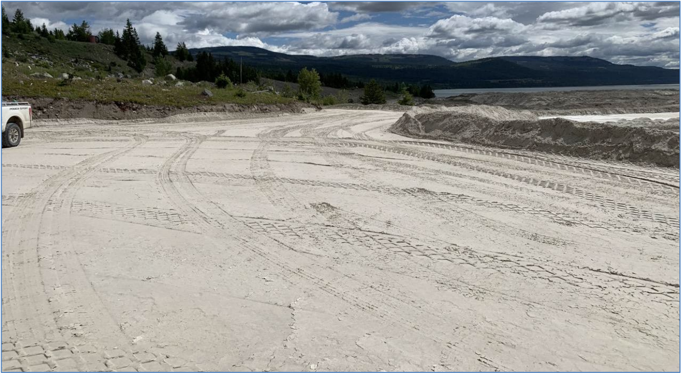
Photo I-A-7 View of key-in of Core Zone at North Abutment (LL-2020-05)
