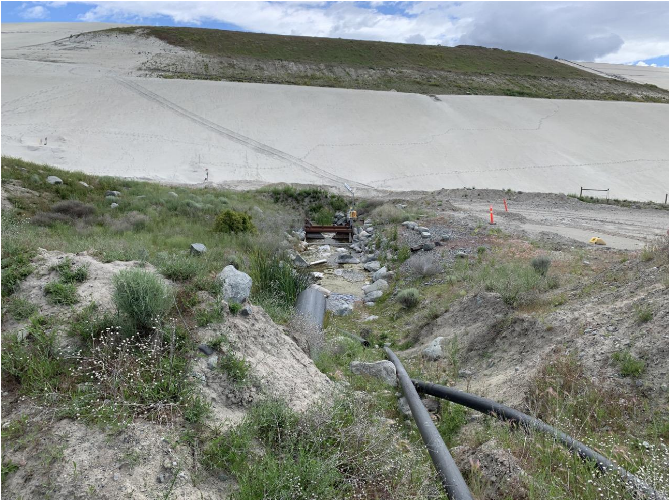
Photo I-A-25 View of Seepage Pond 2 outflow and weir (LL-2020-08)
