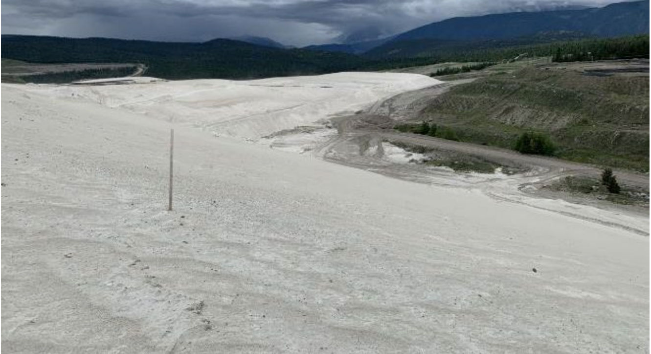
Photo I-A-10 View of Valley Buttress Berm downstream slope and south of Sediment Pond 1. Prepping for downstream sand placement (LL-2020-07)
