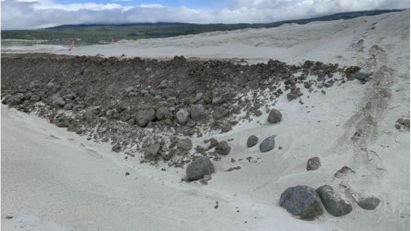
Photo I-A-5 View of raised Till Core Zone at South Dam. Oversized were pushed to edge of lift (LL-2020-04)
