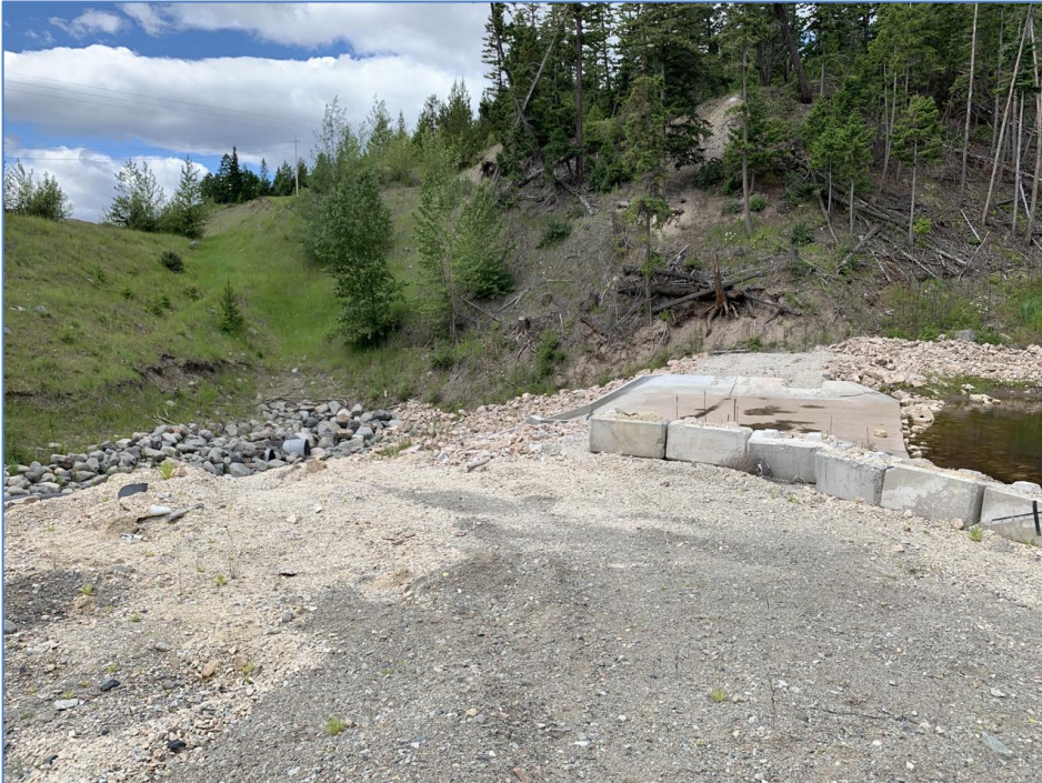
Photo I-A-30 View of Woods Creek Diversion. Pumps were working and there was no overflow into impoundment (LL-2020-18)
