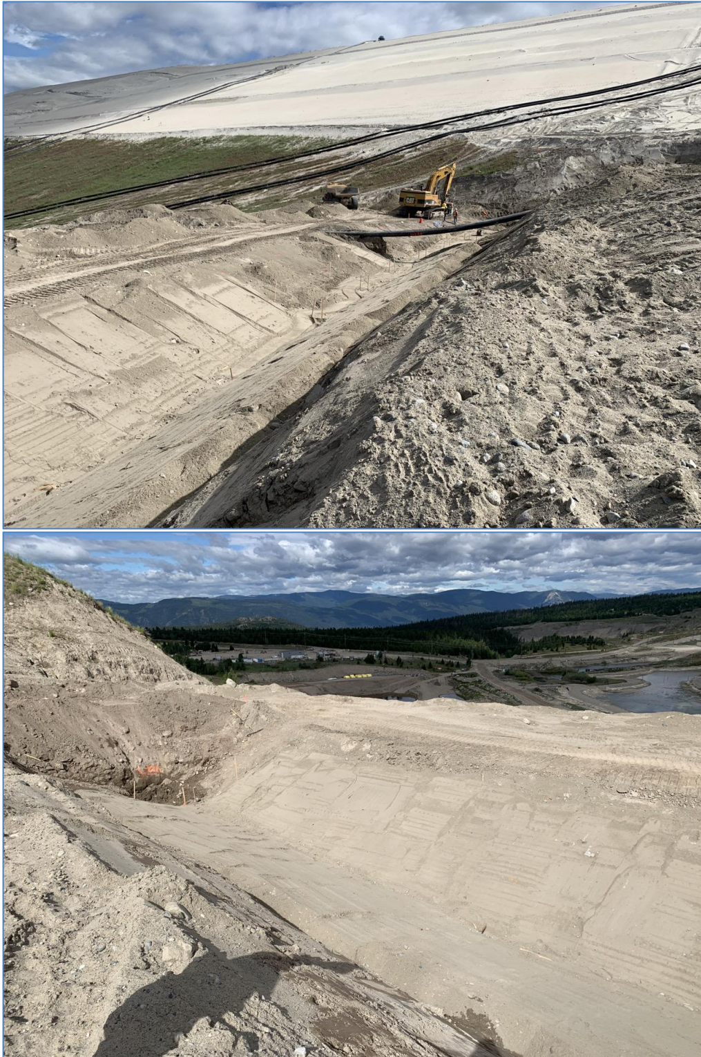
Photo I-A-16 View of Minor Drain being constructed at South Dam (LL-2020-10)
