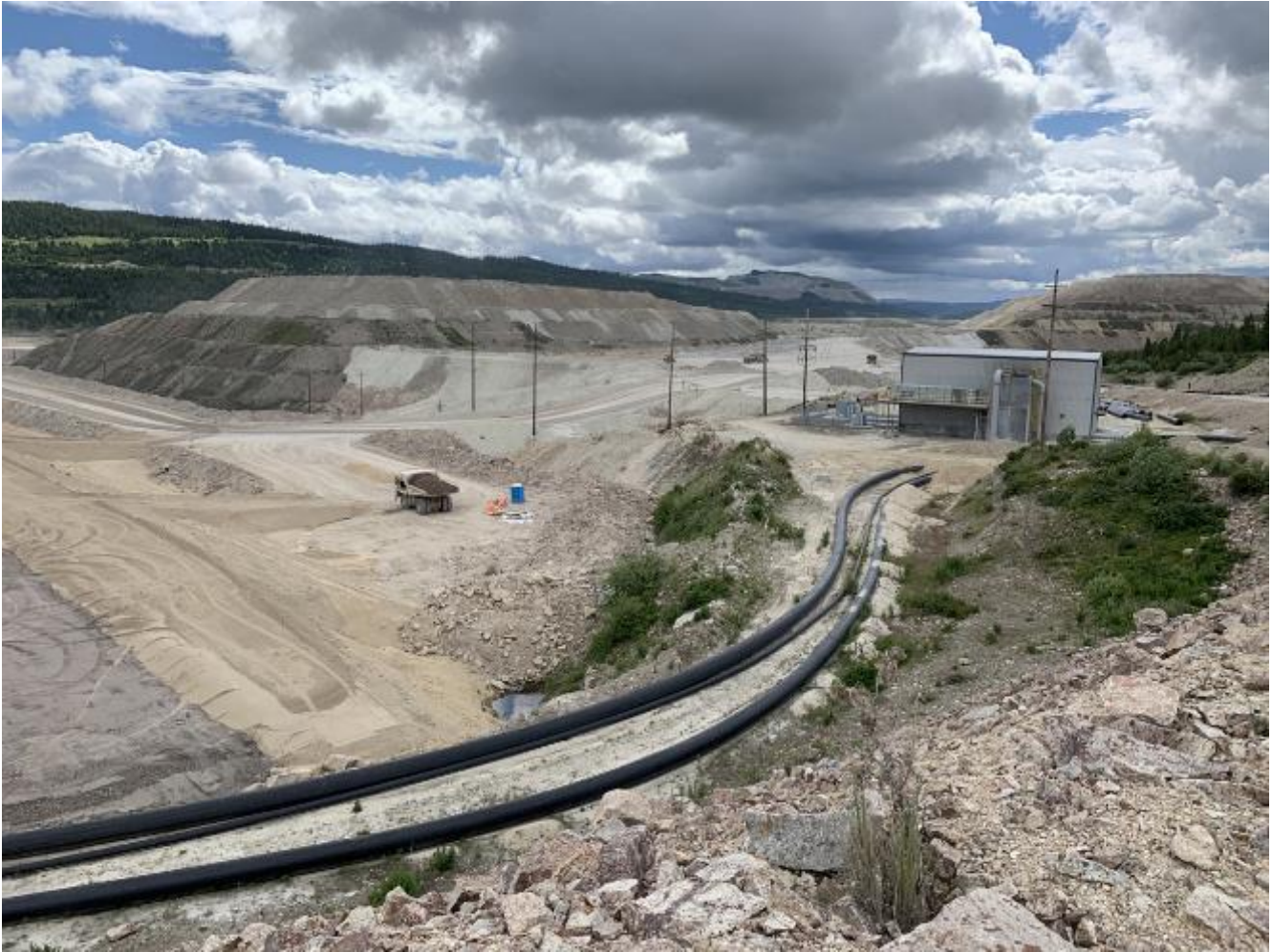
Photo I-B-2 Overview of West Abutment and H-H Dam Pumphouse No.1. SS1 pipes to be relocated over till core (temporarily) to allow West abutment construction to be completed, looking southeast (HH-2020-01)
