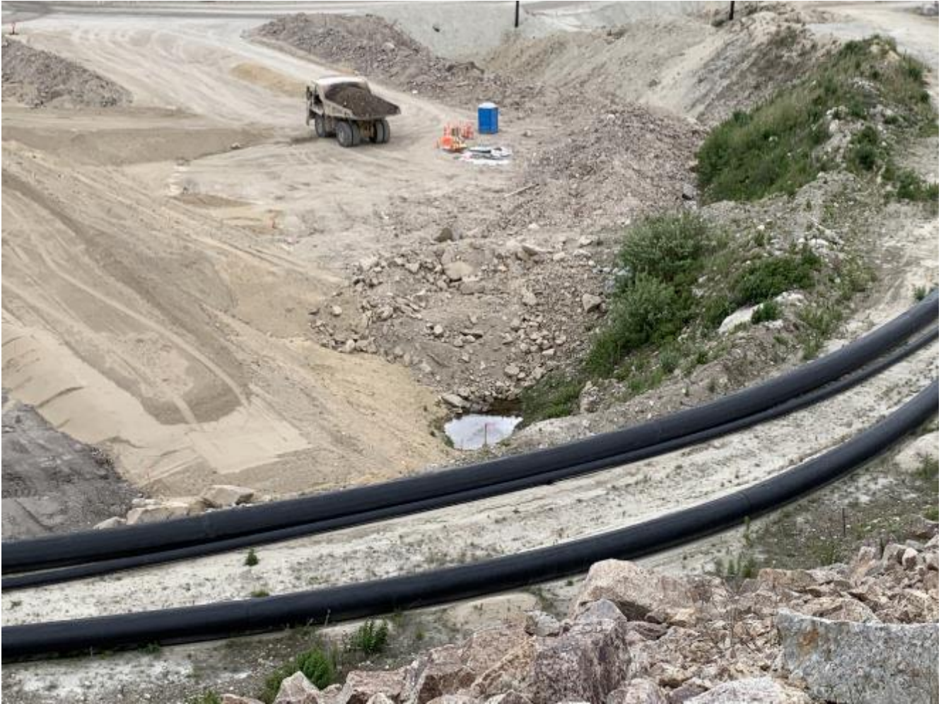
Photo I-B-3 Overview of West Abutment dam raise. SG2 fill was pulled back near abutment to avoid culvert (ponded area). This area will be prepared for 2021 raise, looking southeast (HH-2020-01)
