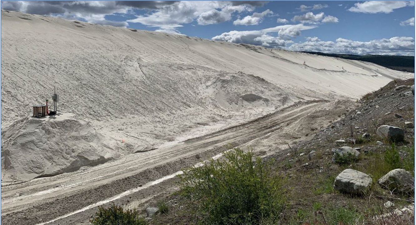
Photo I-A-8 Overview of the downstream slope of North Dam near I19-04. Wet area in low point of toe road but no seepage faces or wet areas on dam slope (LL-2020-06)
