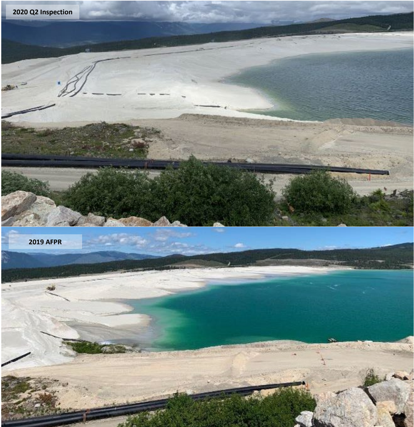
Photo I-A-19 Overview of L-L Dam beach and pond from South Abutment (top). Comparison with photo from 2019 AFPR site visit (bottom) shows beach width increase. (LL-2020-11)
