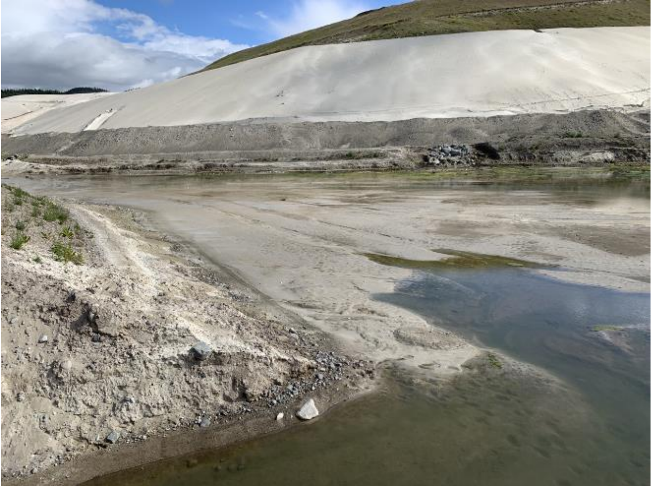
Photo I-A-20 View of Sediment Pond 1 and downstream toe of the Valley Buttress Berm (VBB) (LL-2020-12)
