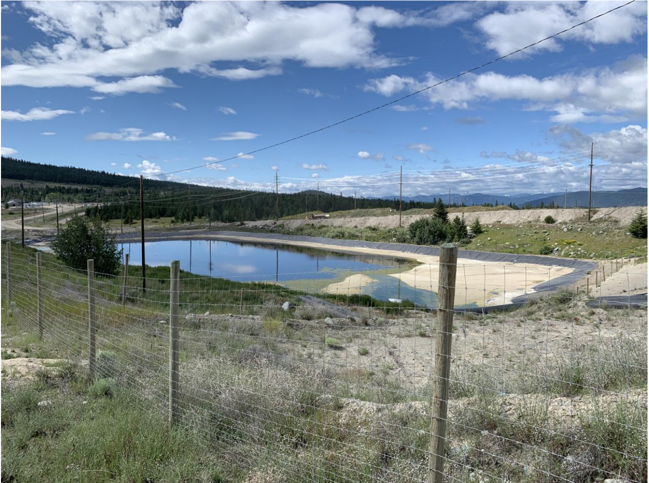
Photo I-A-24 Overview of Seepage Pond 2 (LL-2020-13)
