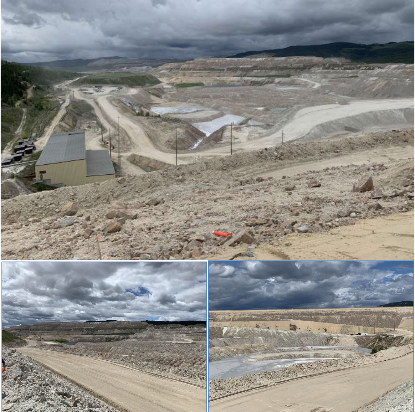
Photo I-B-7 Overview of 24 Mile Waste Dump, 24 Mile Spill Pond and HH Pumphouse. Tailings deposition area of flow from HH Pumphouse to 24 Mile Spill Pond, visually appeared greater than expected (HH-2020-04 and HH-2020-05)
