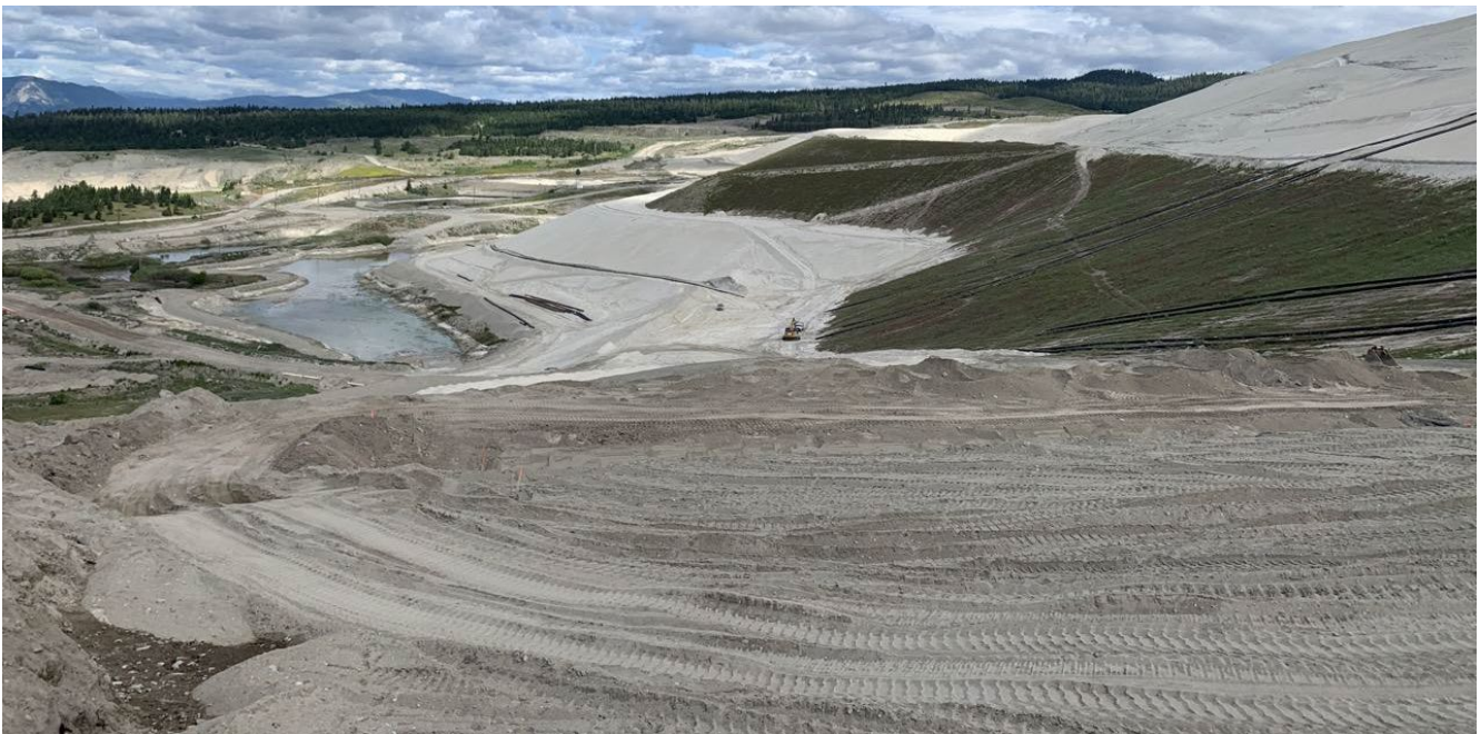
Photo I-A-10 View of Valley Buttress Berm downstream slope and south of Sediment Pond 1. Prepping for downstream sand placement (LL-2020-07)
