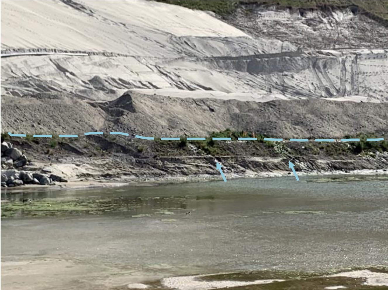
Photo I-A-23 Overview of Sediment Pond 1. Seepage visible on exposed divider dyke slope at the expected location. No seepage or wetted face was observed within the dam fill or drainage blanket (LL-2020-12)
