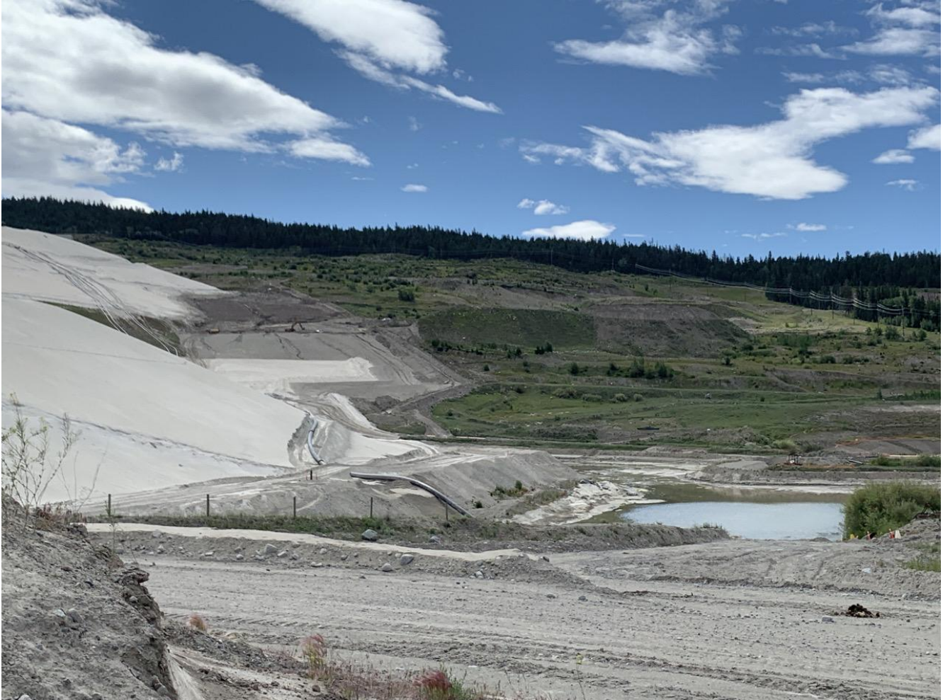
Photo I-A-11 View of Valley Buttress Berm and South Dam downstream slope and toe area. Ponded water is in Sediment Pond 1 (LL-2020-08)
