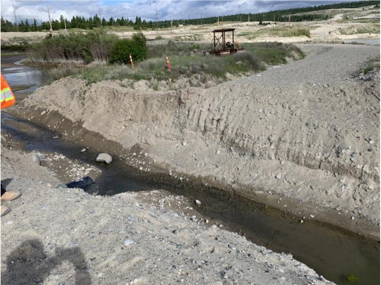
Photo I-A-21 View of Sediment Pond 1 draining to Seepage Water Reclaim Pond (SWRP) via a channel which will be backfilled and replaced with a pipe as part of prep activities to get Sediment Pond 1 to receive hydraulic placement overflow (LL-2020-12)
