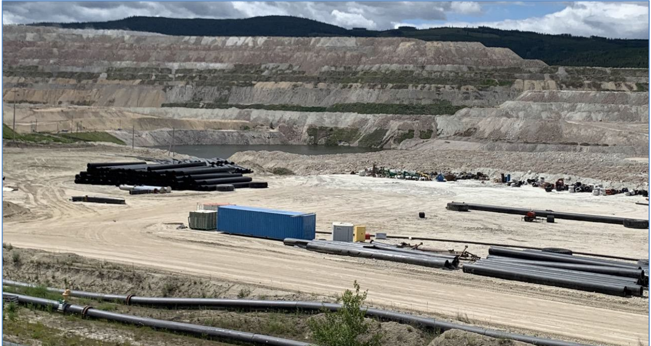
Photo I-B-9 View of 24 Mile Spill Pond and 24 Mile Waste Dump with relocated pipe laydown in foreground (HH-2020-07)
