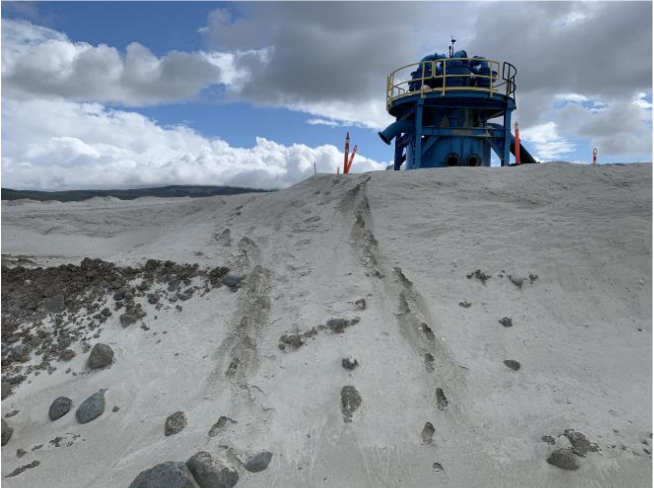
Photo I-A-17 View of Secondary Cyclones at South Dam crest – looking upstream (LL-2020-04)
