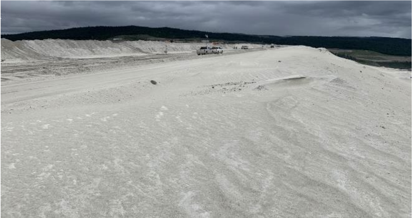
Photo I-A-4 View of L-L Dam crest – looking south (LL-2020-03)
