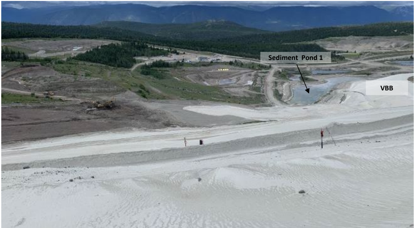
Photo I-A-13 Overview of South Dam downstream slope from crest – looking west (LL-2020-04)
