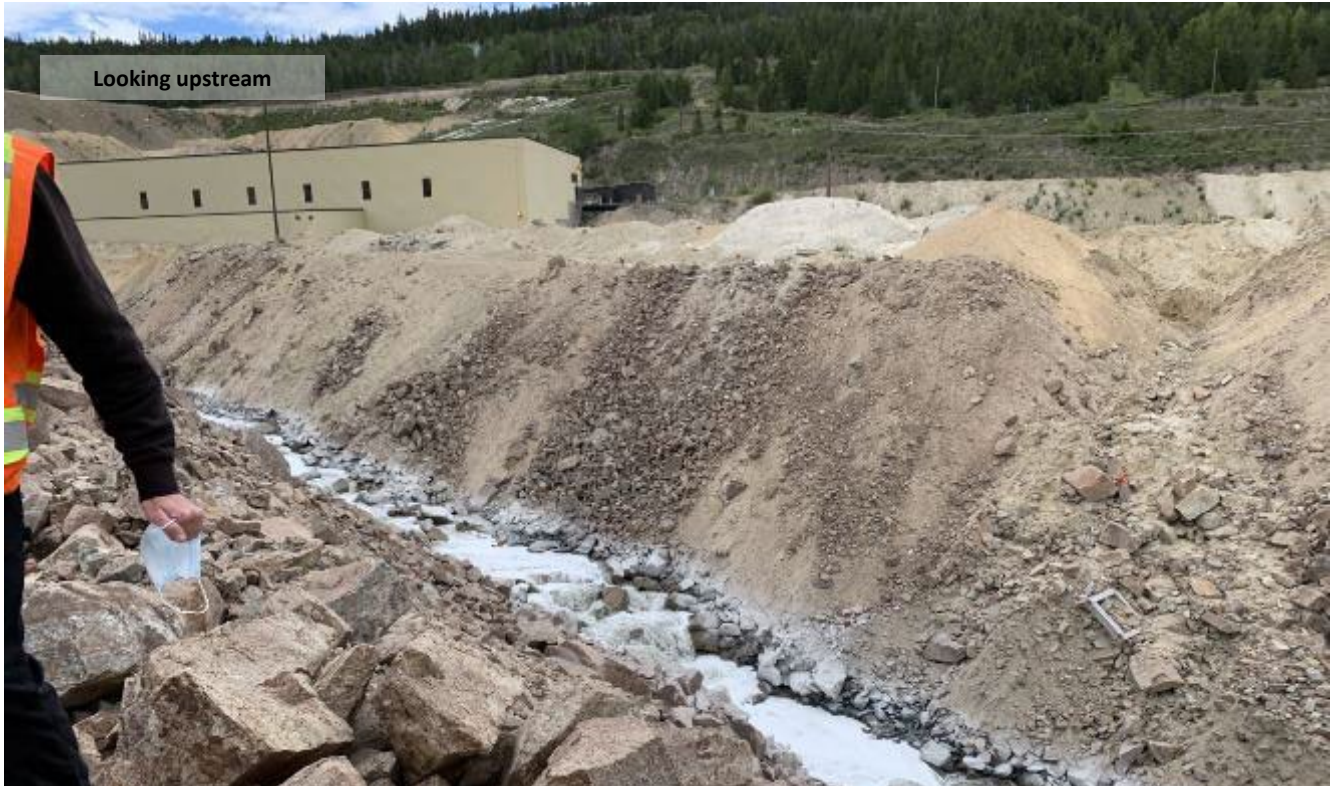
Photo I-B-8 View of tailings overflow, discharging from HH Pumphouse, flowing along new tailings channel, over pipe laydown area, to 24 Mile Spill Pond (HH-2020-06)
