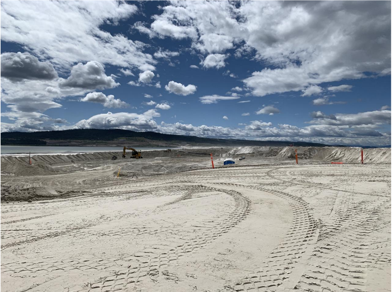
Photo I-A-6 View of an upstream hydraulic placement cell (LL-2020-05)
