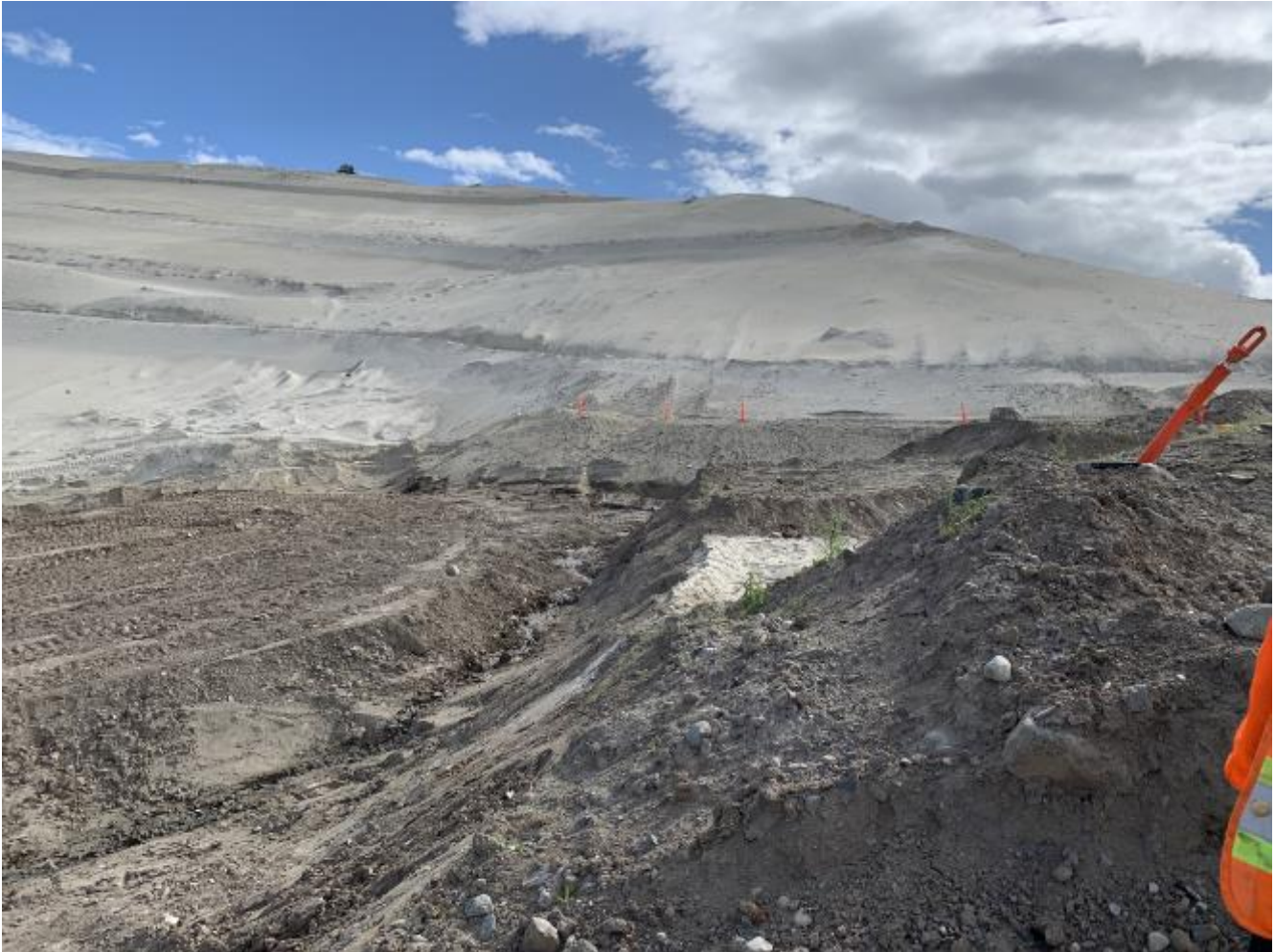
Photo I-A-14 View of South Buttress Berm downstream toe, slope, and foundation area. Seepage was observed at the toe, from area of underdrain, no seepage face observed within cycloned sand. All seepage flows are collected (LL-2020-09)
