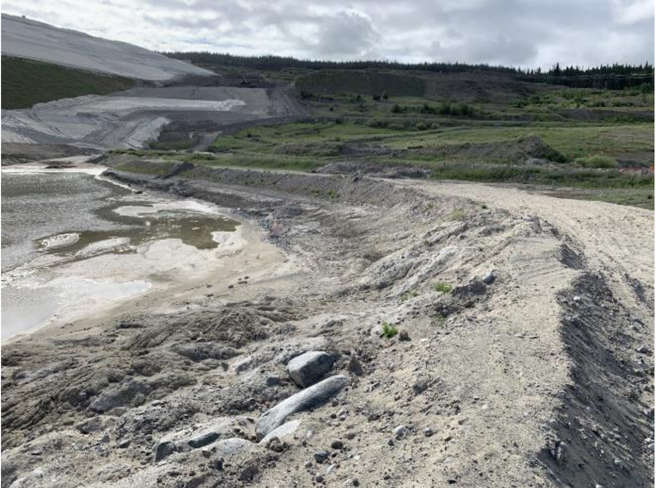
Photo I-A-22 Sediment Pond 1 downstream berm. No ponding water was observed downstream side of berm – looking toward South Abutment (LL-2020-12)
