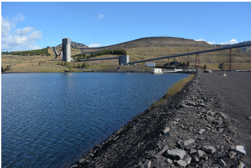
Photograph 7: Main Tailings Dam – Upstream Crest and Reclaim Barge; Looking Northeast, 1 September 2020
