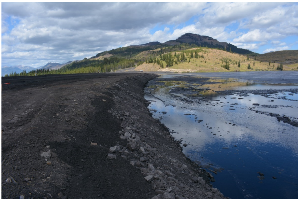
Photograph 33: West Tailings Dam – Till Blanket and Upstream Slope; Preparation in Progress for 2020 Dam Raise; Looking North, 1 September 2020
