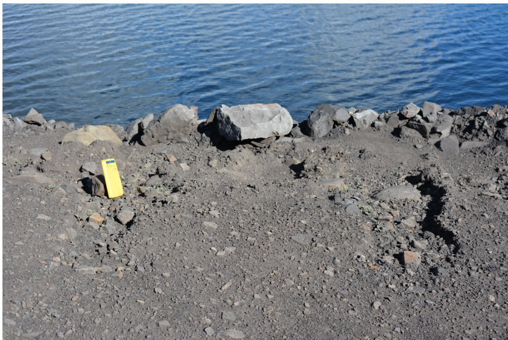
Photograph 15: Main Tailings Dam – Minor Erosion Rills on Upstream Crest; Looking North, 1 September 2020
