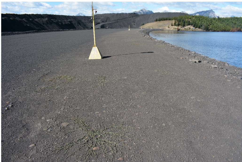
Photograph 13: Main Tailings Dam – Prism and Vegetation on Dam Crest; Looking West, 1 September 2020
