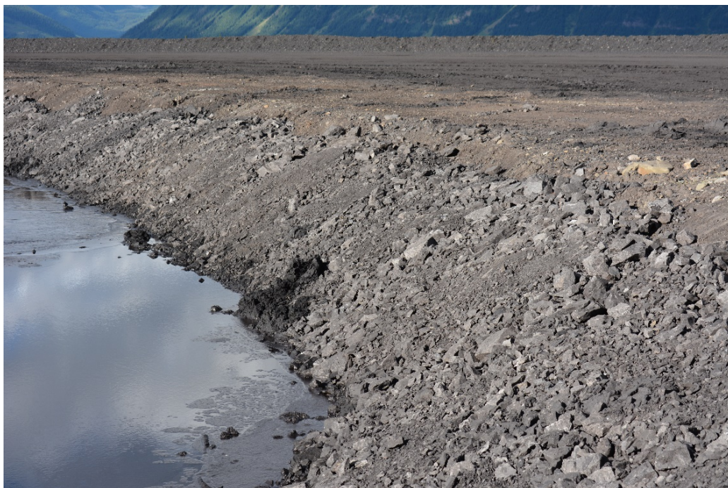
Photograph 38: West Tailings Dam – Upstream Slope; Preparation in Progress for 2020 Dam Raise; Looking West, 1 September 2020
