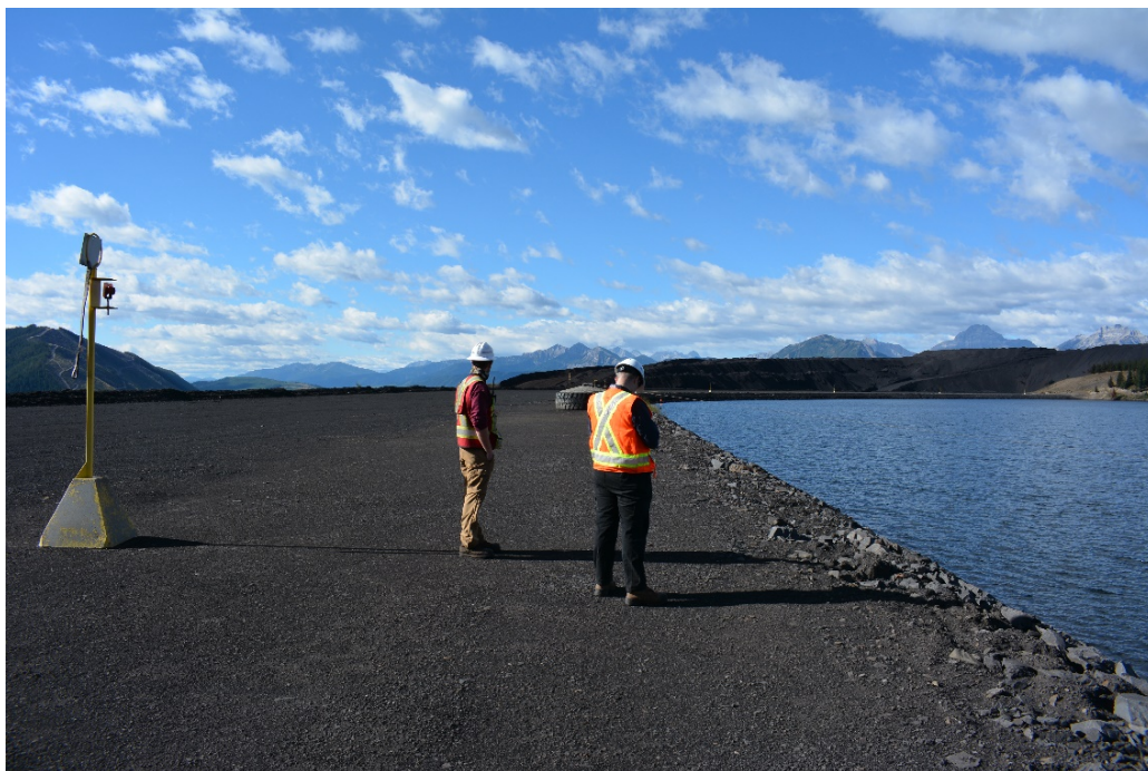
Photograph 5: Main Tailings Dam – Till Blanket and Dam Crest; Looking Southwest, 1 September 2020
