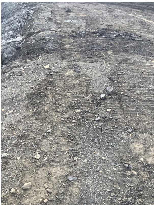
Photograph 37: West Tailings Dam - Superficial Cracking on Till Blanket; Looking South, 1 September 2020
