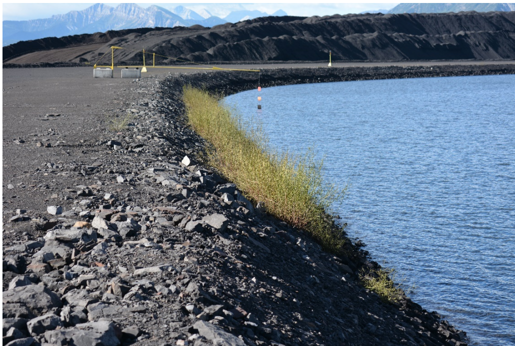
Photograph 6: Main Tailings Dam – Vegetation on Upstream Crest; Looking Southwest, 1 September 2020
