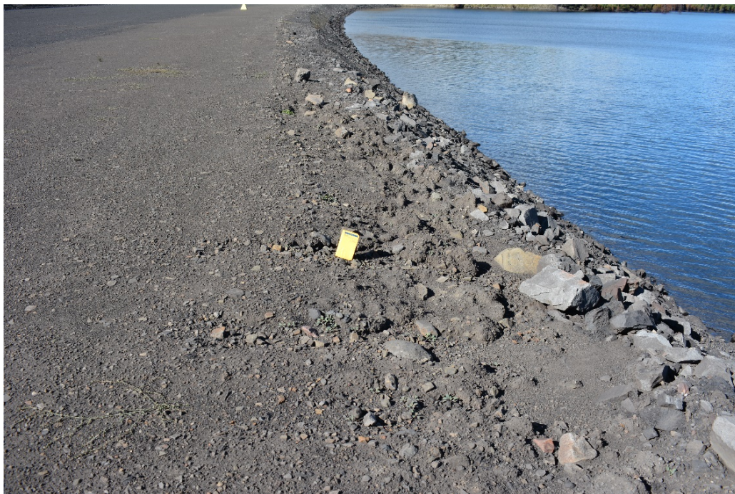
Photograph 14: Main Tailings Dam – Minor Erosion Rills on Upstream Crest; Looking West, 1 September 2020
