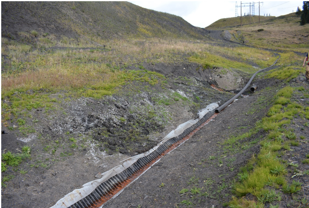
Photograph 26: Site C Coarse Refuse Facility – Smart Ditch at Toe; Looking Northeast, 1 September 2020
