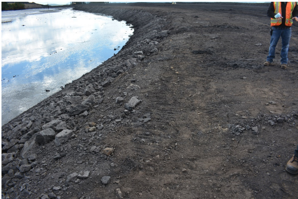
Photograph 36: West Tailings Dam – Till Blanket; Preparation in Progress for 2020 Dam Raise; Looking South, 1 September 2020
