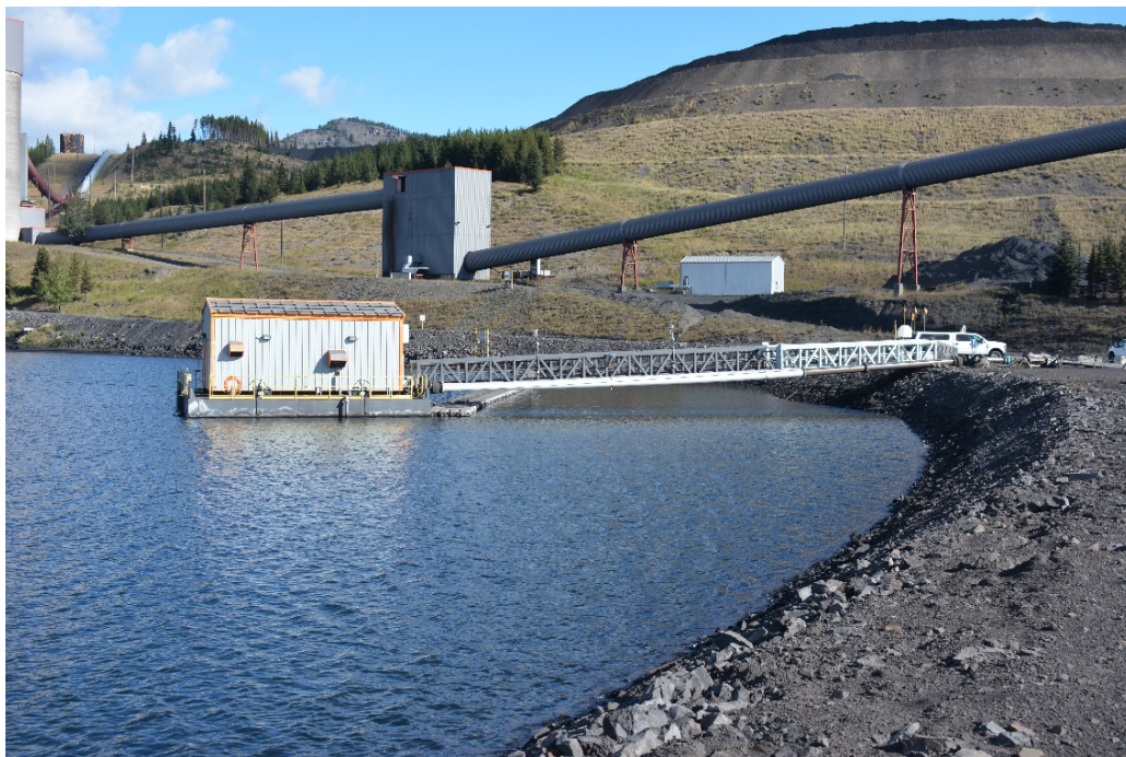
Photograph 4: Main Tailings Dam – Reclaim Barge and Upstream Crest; Looking North, 1 September 2020
