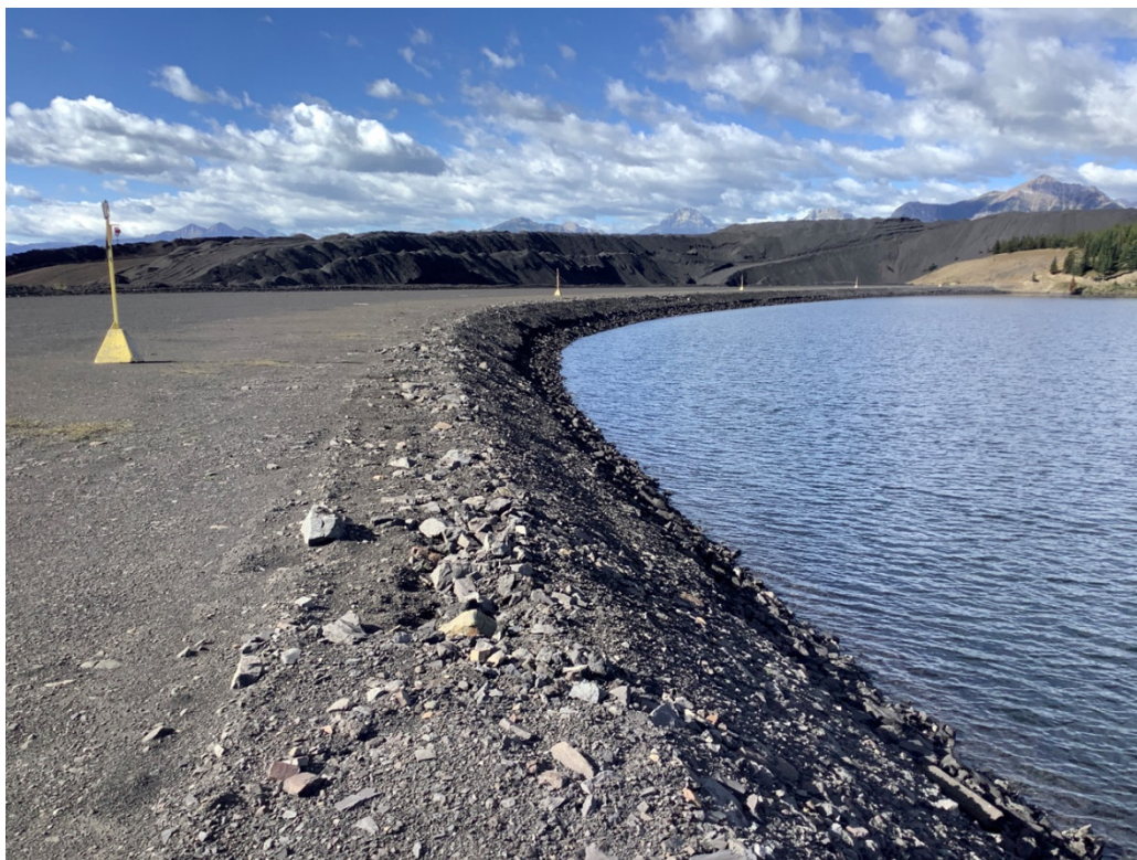
Figure 11: Main Tailings Dam - Upstream Crest Riprap Erosion; Looking West, 1 September 2020
