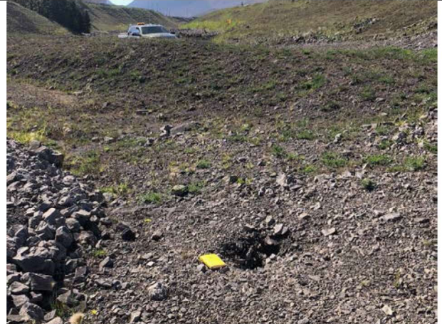
Photo 2: Small sinkhole about 0.5 by 0.5 m at approx. Sta. 0+140. This is along the alignment of the buried setback riprap.
