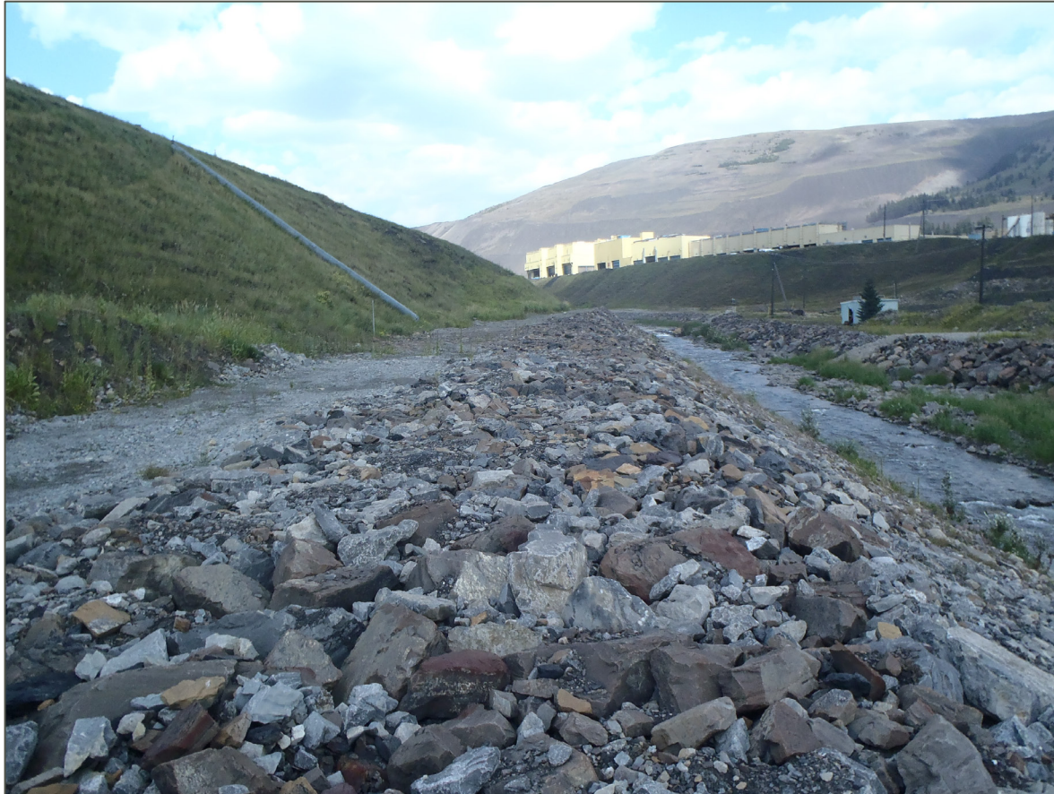
NTP Dam downstream slope and riprap along Fording River; looking northeast from approximately Sta. 0+950
