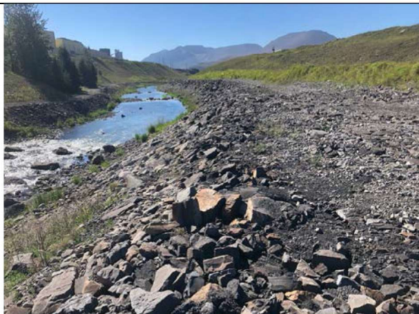
Photo 3: Looking downstream at NTP riprap (from approx. Sta. 0+225).
