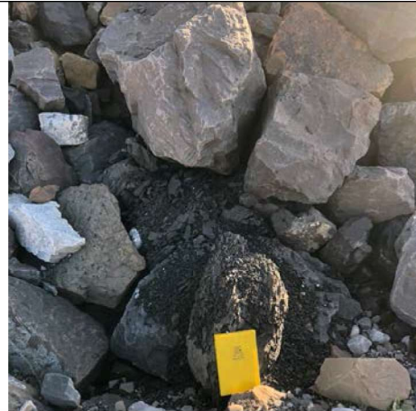
Photo 10: Riprap degradation due to weathering on several pieces of riprap.
