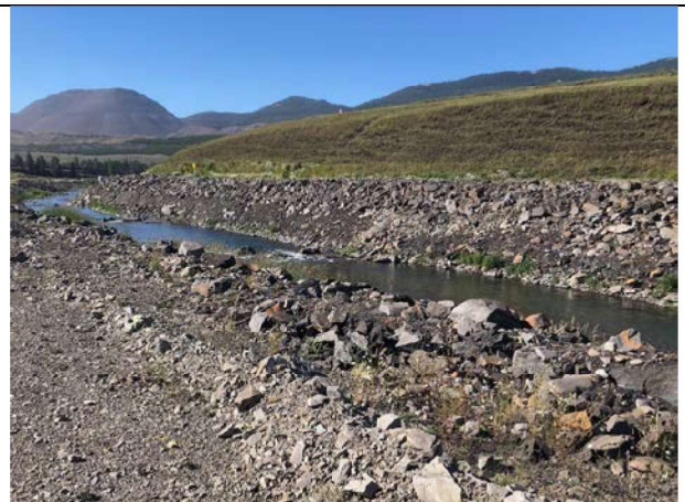
Photo 4: Looking downstream at NTP riprap (from approx. Sta. 0+475).
