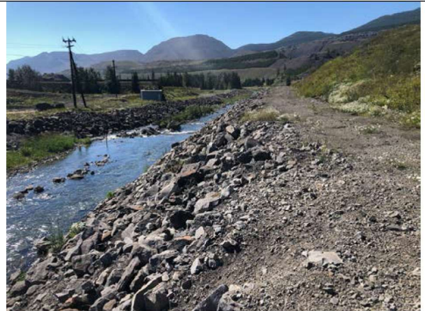
Photo 6: Looking downstream at NTP riprap (from approx. Sta. 0+725).
