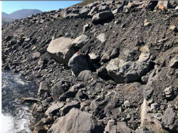
Photo 5: Looking at erosion of the gravel material placed on top of the riprap at one of the riffle crest bank tie-ins on the NTP (approx. Sta. 0+550).
