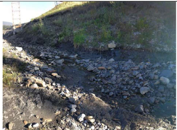
Photo 12: Erosion along the toe of the STP downstream of the pipe bridge. The erosion has exposed bedrock in some areas.
