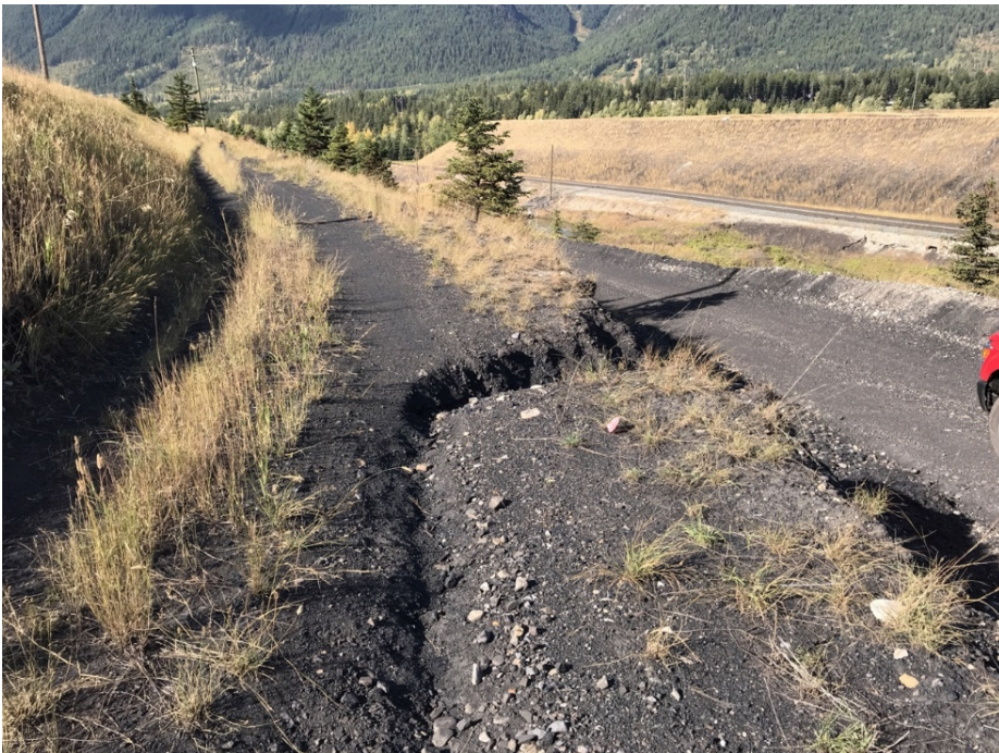
Photo ID-14 Lagoon D bench minor erosion. (looking west)
