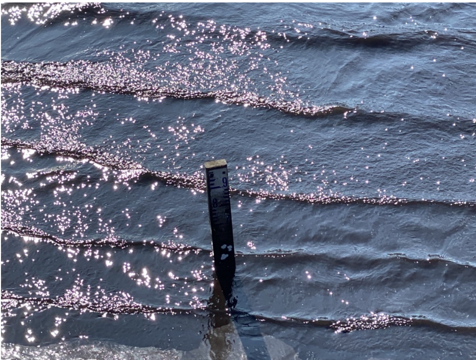
Photo ID-10 Lagoon D decant pond staff gauge unreadable (looking south).
