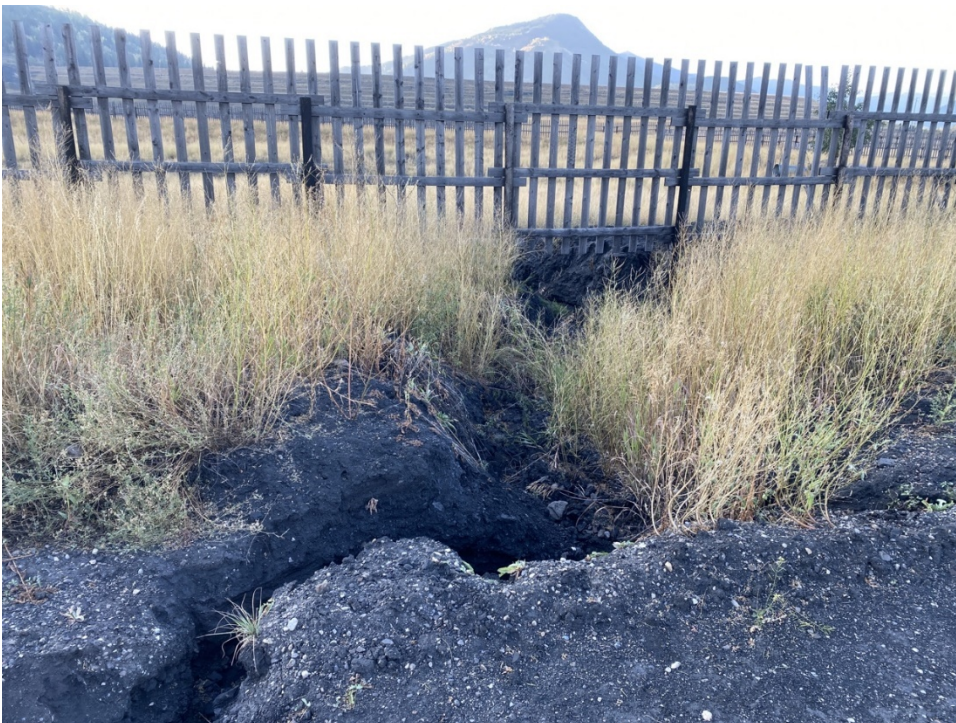
Photo IC-4 Lagoon C minor erosion upstream of crest near pumphouse. (looking southeast)
