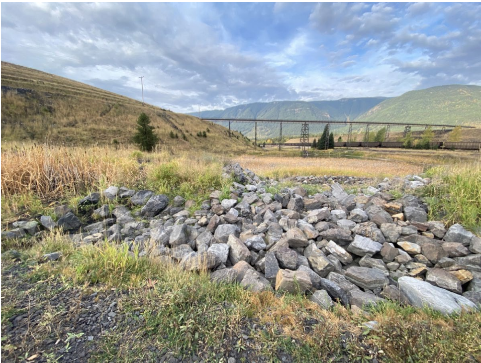
Photo IA-4 Lagoon A Spillway riprap. (looking west)
