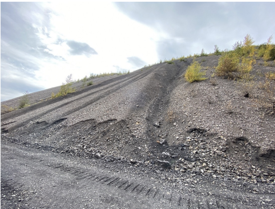
Photo IW-8 WFTF Adit Dump erosion above Adit Toe Berm. (looking west)
