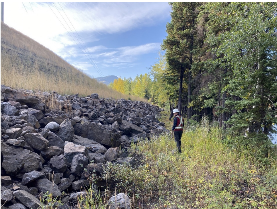
Photo IC-12 Lagoon C toe riprap, adjacent to the Elk River. (looking south)
