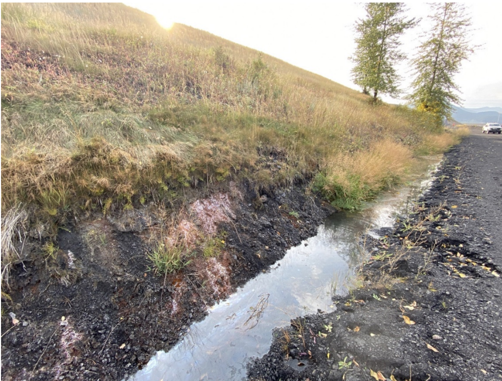
Photo I-6 CCR Dump seepage at bench ditches. (looking south)
