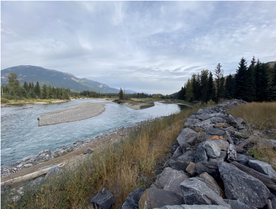
Photo I-15 CCR Dump toe riprap adjacent to the Elk River (looking north).
