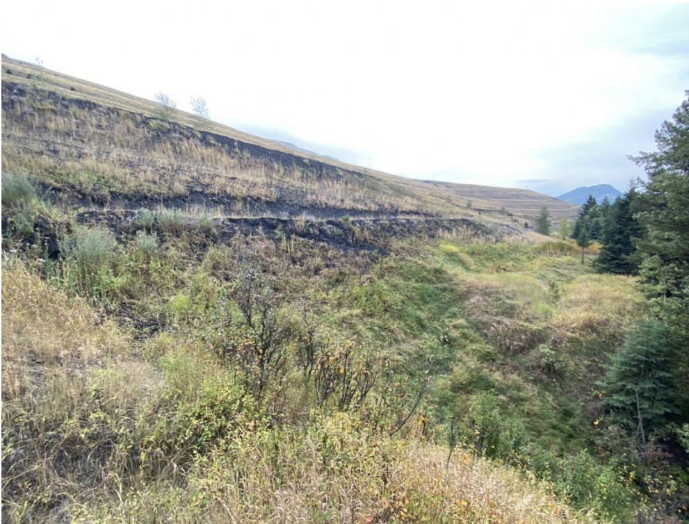
Photo I-5 CCR Dump sparse vegetation at toe benches. (looking southeast)
