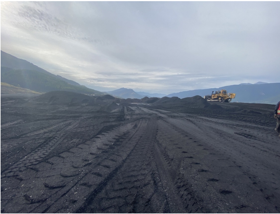
Photo I-3 CCR Dump crest construction in progress. (looking south)
