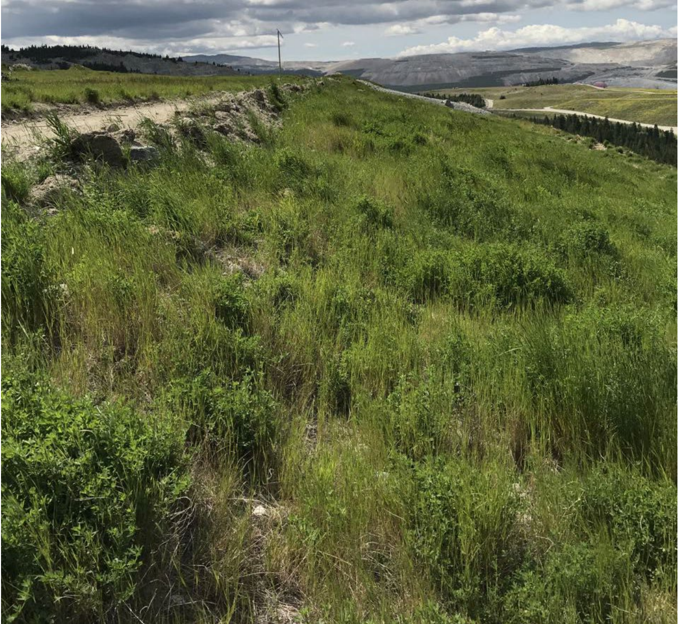
Photo I-A-7 Overview of downstream slope and toe from crest road, looking south. No major erosion areas were observed. (BTH-2020-01)
