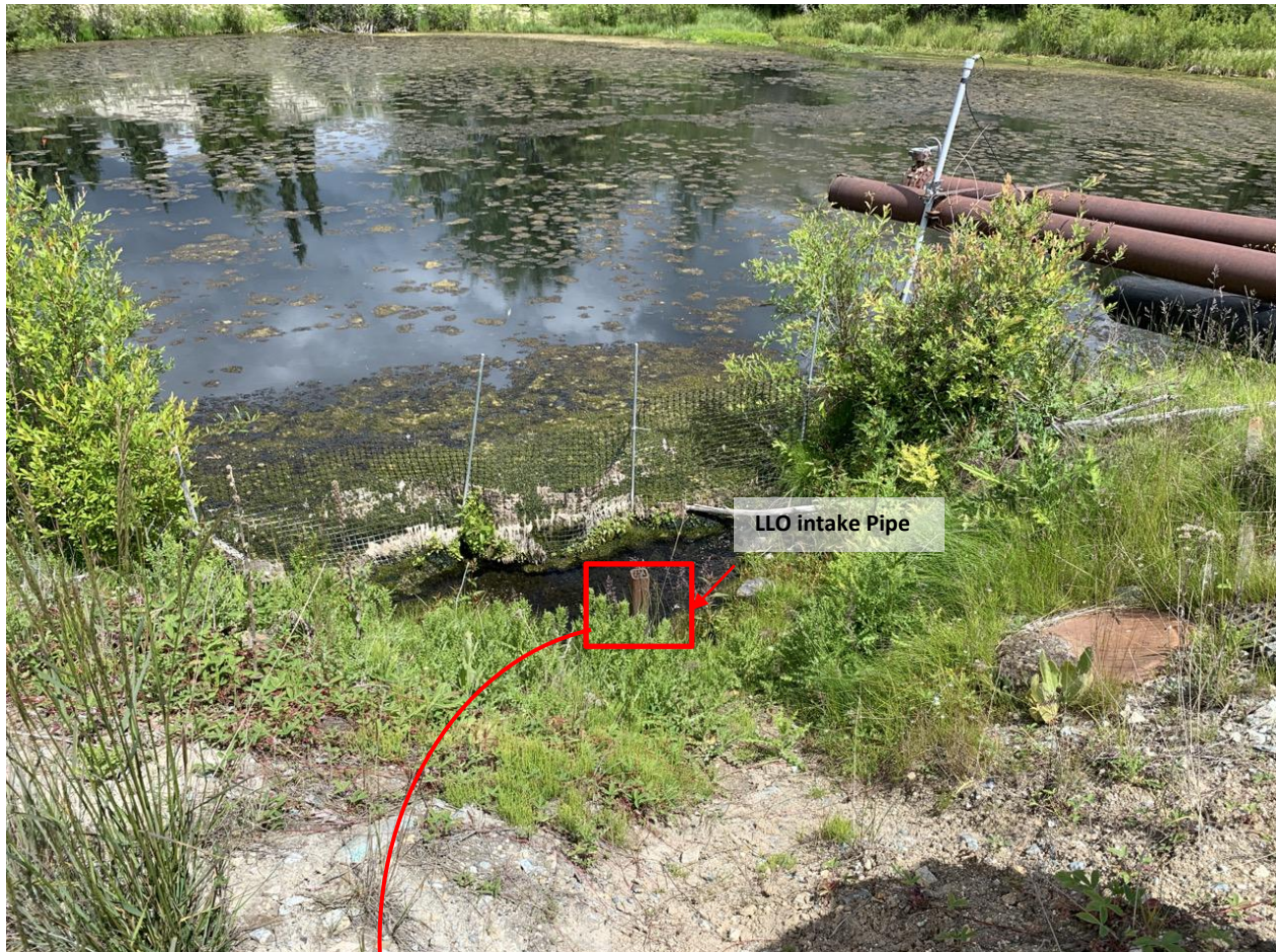
Photo I-C-4 View of R3 Seepage Pond and debris mesh for Low-Level Outlet (LLO). Clear water was flowing at the time of inspection. The debris mesh is clogged below and above water. This does not impact flood routing but could be part of routine maintenance. (BTH-2020-30)
