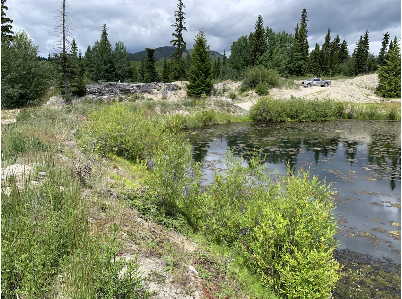
Photo I-C-3 R3 Seepage Pond upstream slope heavily vegetated. Vegetation should be removed as part of routine maintenance (BTH-2020-30)
