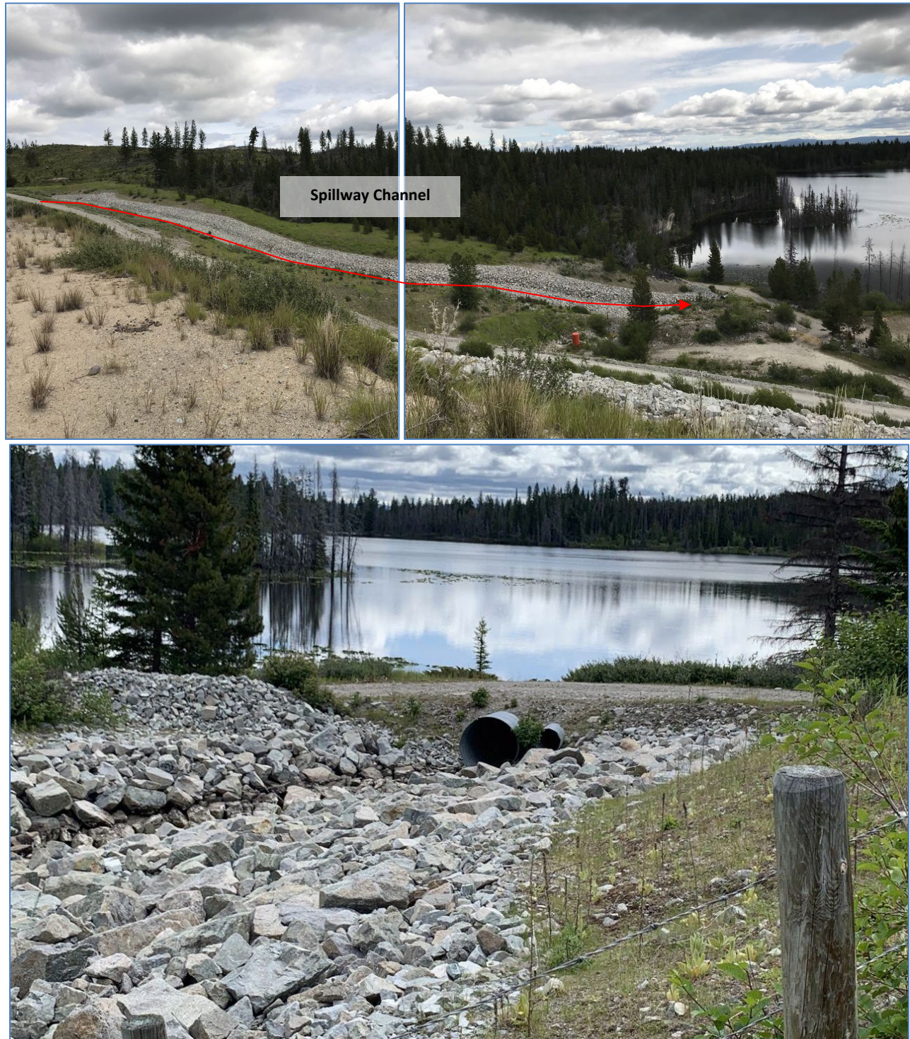
Photo I-B-20 Spillway channel and outlet to Bose Lake. Downstream spillway culverts are unobstructed. Sign of water pooling upstream of culverts in channel but no sign of flow through spillway. Likely pooled runoff (BTH-2020-09 and BTH-2020-27)
