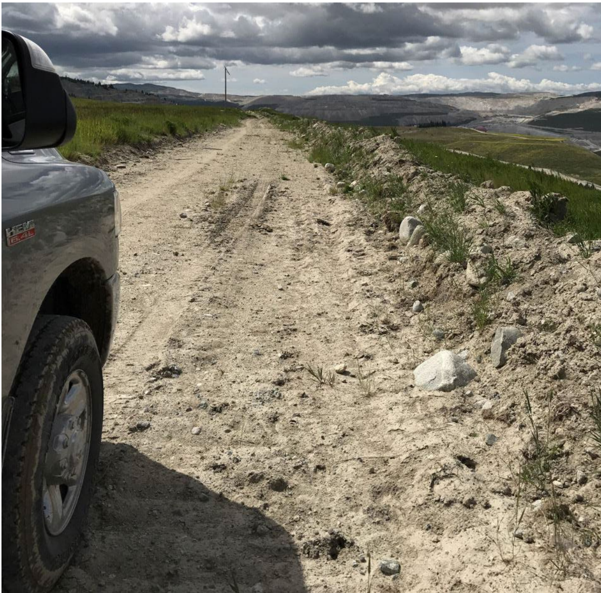
Photo I-A-1 Dam No. 1 crest road. No evidence of erosion or depression was observed (BTH-2020-01)
