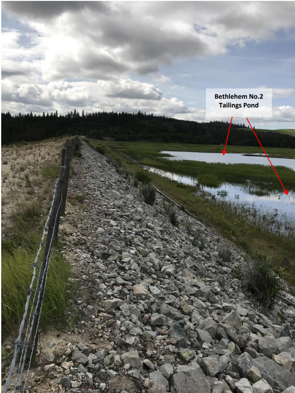
Photo I-B-15 Overview of upstream riprap and tailings beach from left abutment (BTH-2020-13)
