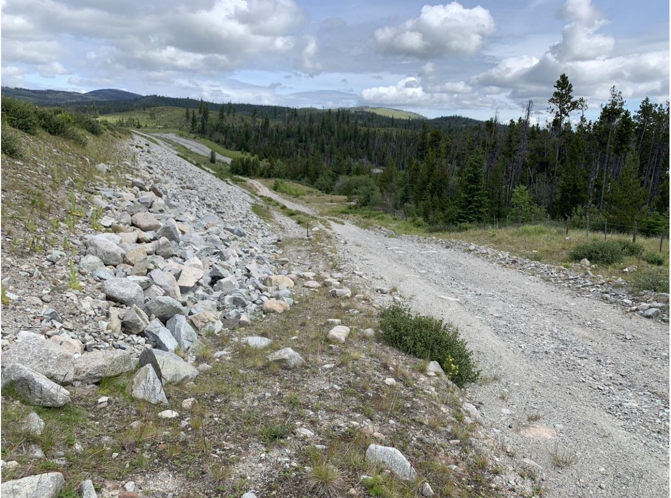
Photo I-B-8 Overview of downstream slope from right abutment. No ongoing erosion, road in good condition, and no seepage or wet sections observed in area (BTH-2020-16)
