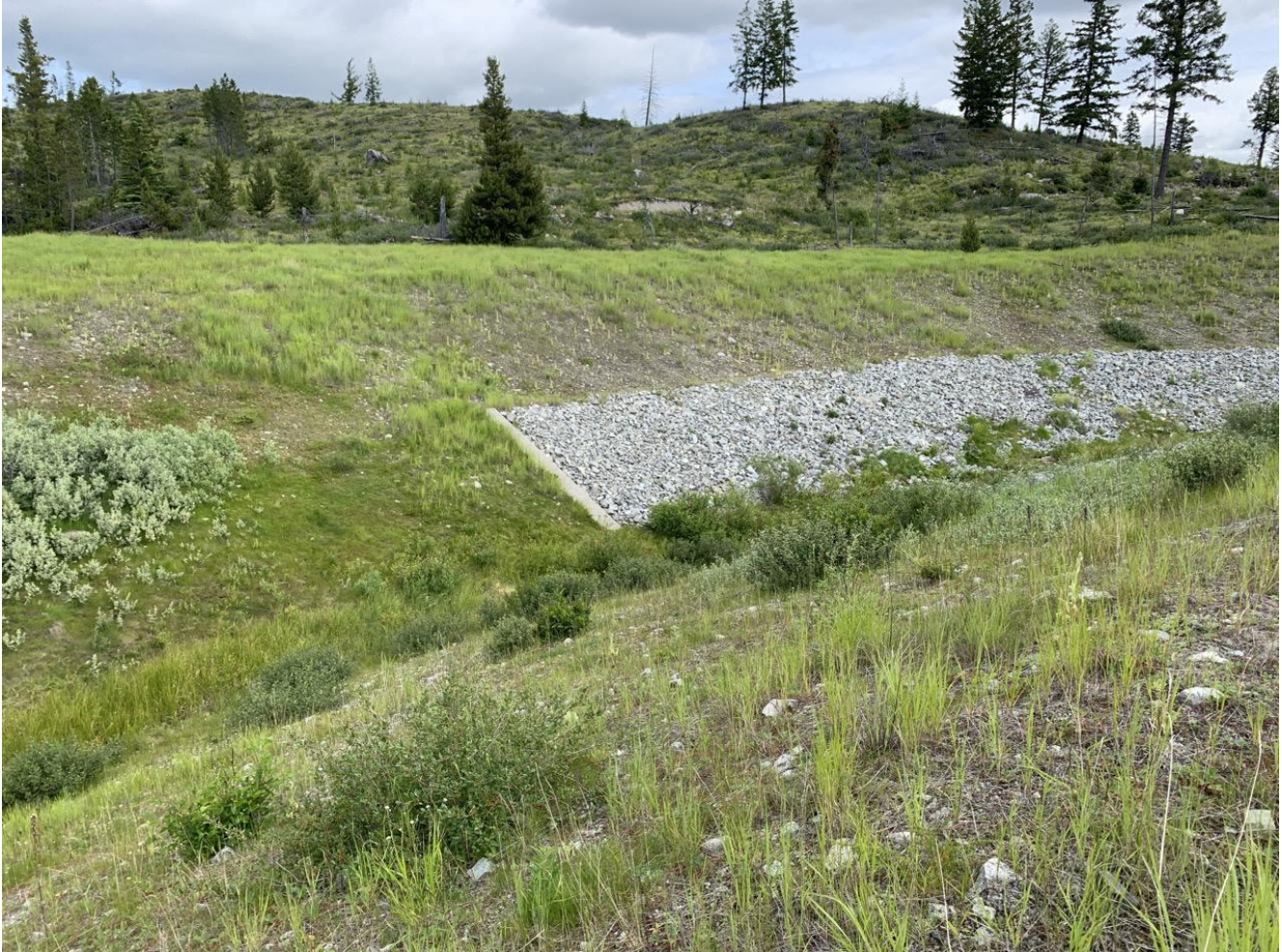
Photo I-B-18 Spillway channel at transition point between inlet and riprap-lined segment, looking towards north (BTH-2020-25)
