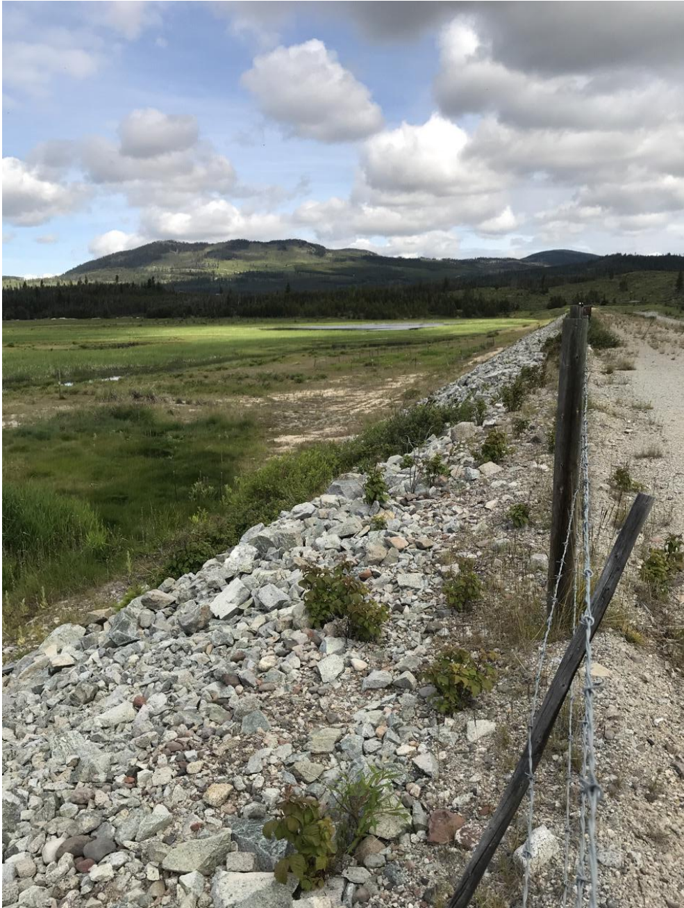
Photo I-B-14 Overview of upstream riprap and tailings beach from right abutment (BTH-2020-23)
