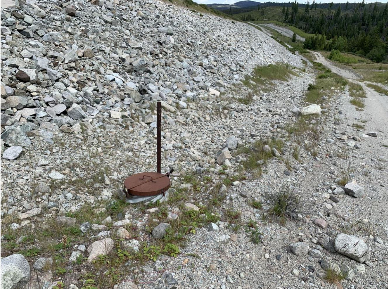
Photo I-B-9 Upslope extent of toe drain along abutment. Toe drain access point is visible. Cap is sealed (BTH-2020-17)
