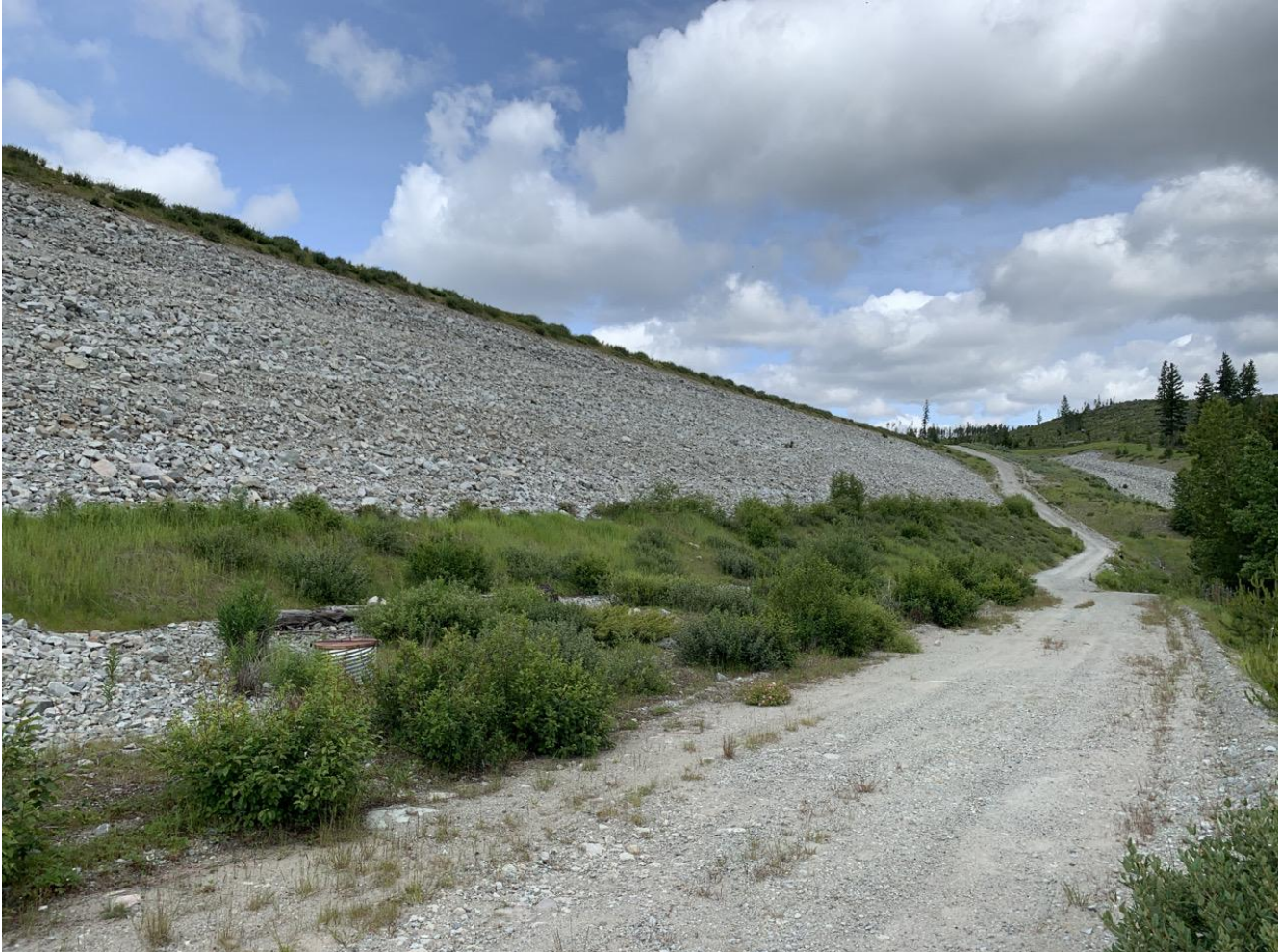
Photo I-B-10 View of downstream slope. Vegetation cover over lower portion of slope, comprised of till fill. No erosion of slope (rock of till) was observed (BTH-2020-18)
