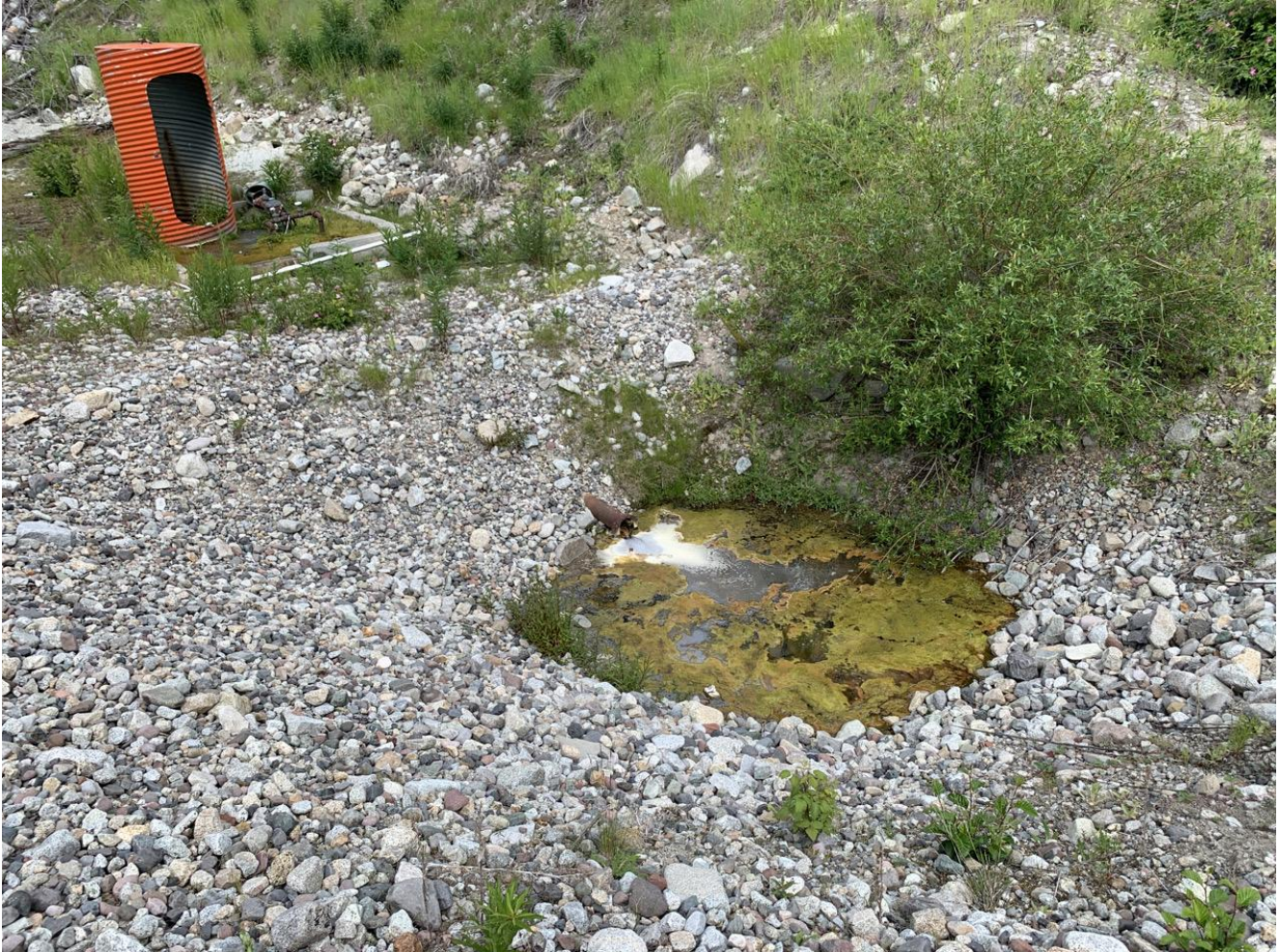
Photo I-B-21 Seepage flow from toe drain is clear. Pond drainage conditions unchanged from 2019 observations (BTH-2020-27)
