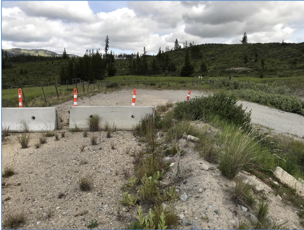
Photo I-B-5 View of left abutment. No sign of erosion or unusual condition (BTH-2020-13 and BTH-2020-14)
