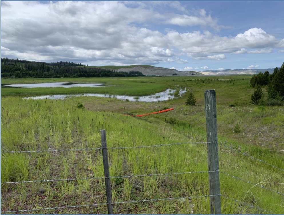
Photo I-B-17 Spillway inlet and approach channel. Vegetation to be cleared from flow channel as part of routine maintenance (BTH-2020-25)
