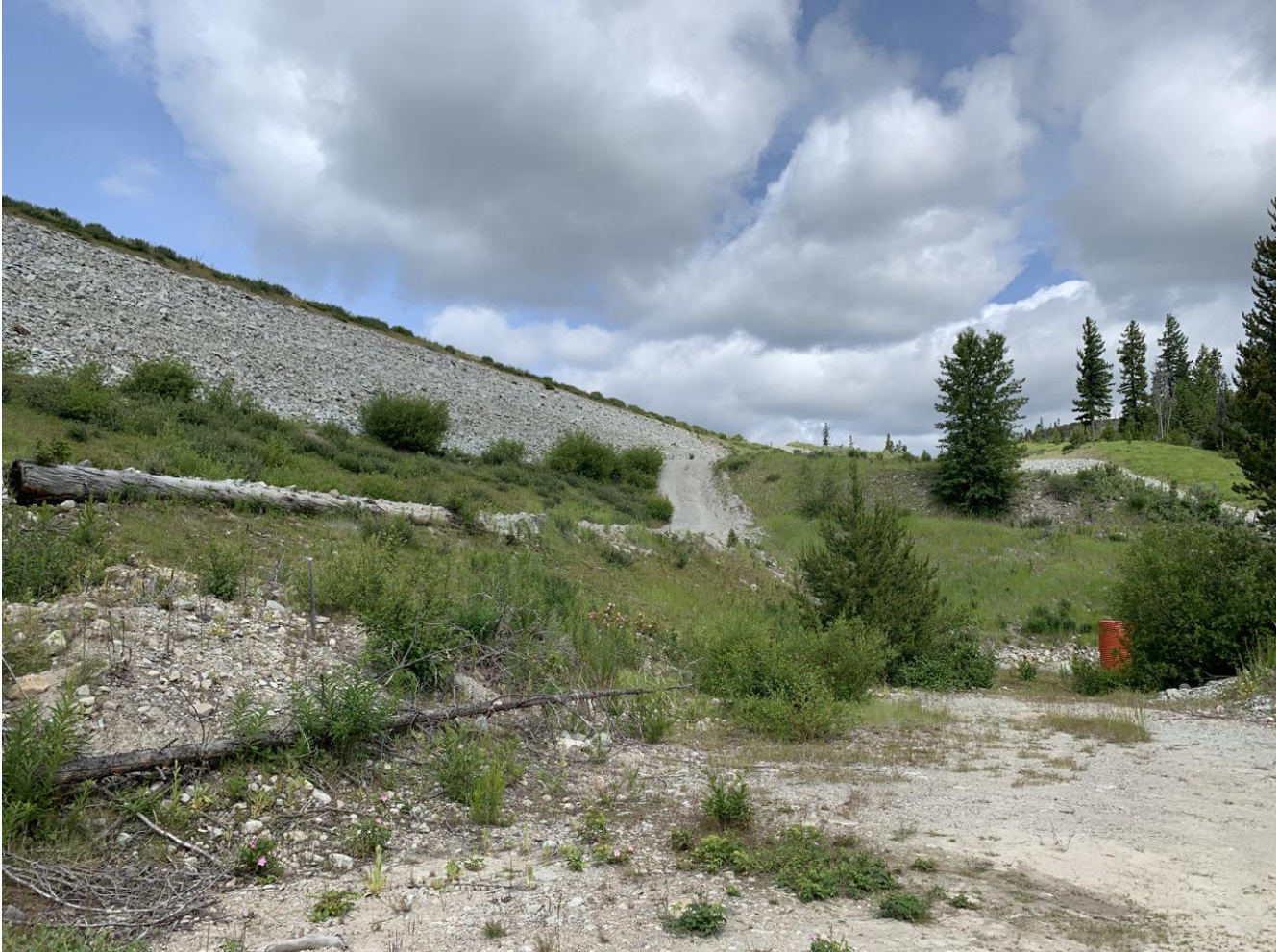
Photo I-B-11 Downstream slope and lower part of left abutment. No sign of unusual condition or erosion (BTH-2020-19)
