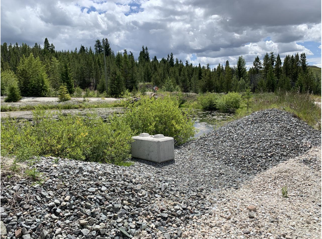
Photo I-C-5 View of spillway inlet. Lock-block and vegetation to be cleared from inlet (BTH-2020-31)
