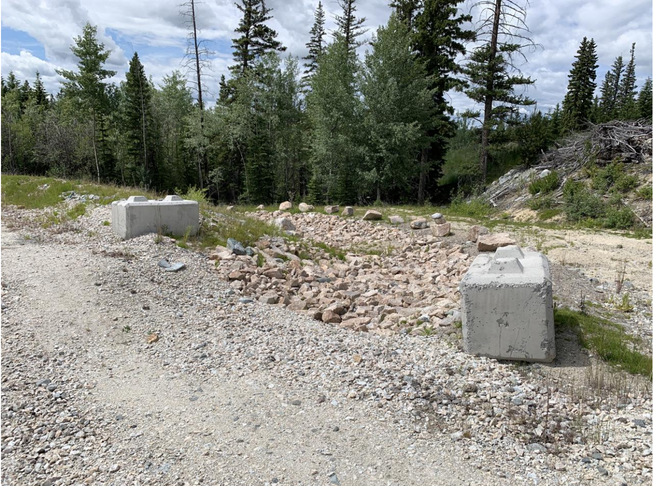
Photo I-C-6 Spillway channel and road crossing at right abutment, looking downstream (BTH-2020-31)
