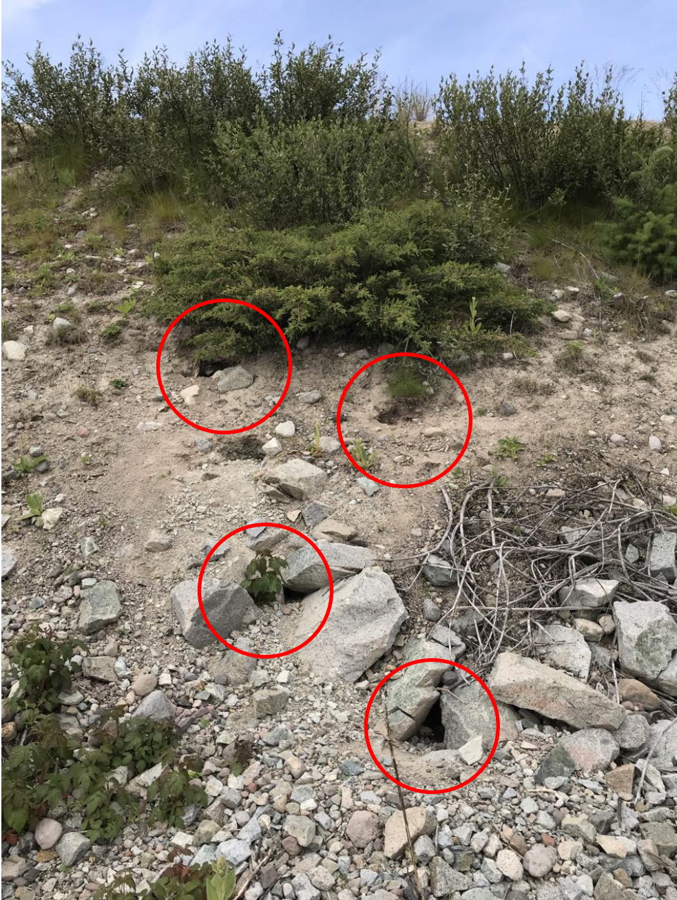
Photo I-B-6 Multiple animal burrows observed at downstream slope near left abutment. Before 2021 freshet, THVCP should conduct an inspection of the upper downstream slope of till, where horizontal width between tailings and downstream slope is narrowest, and fill animal burrows (BTH-2020-15)
