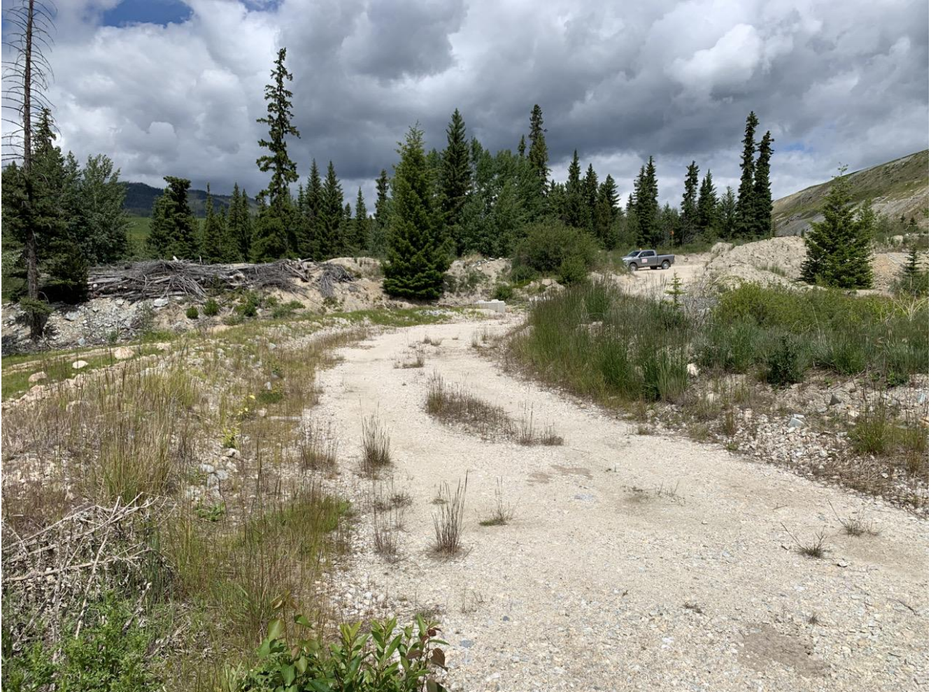
Photo I-C-2 R3 Seepage Pond dam crest. No cracking or no sign of distress was observed (BTH-2020-29)
