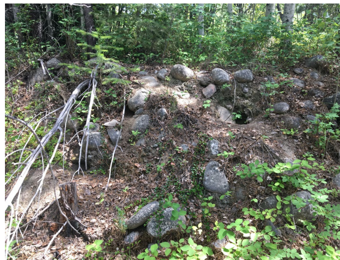
Photograph 2: South TSF, Cell 1, west side downstream toe area with animal burrows, looking east. 21 July 2019.
