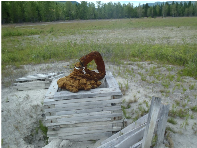
Photograph 27: North TSF, Cell 6, tailings surface and plugged decant tower looking northwest. 21 July 2020.
