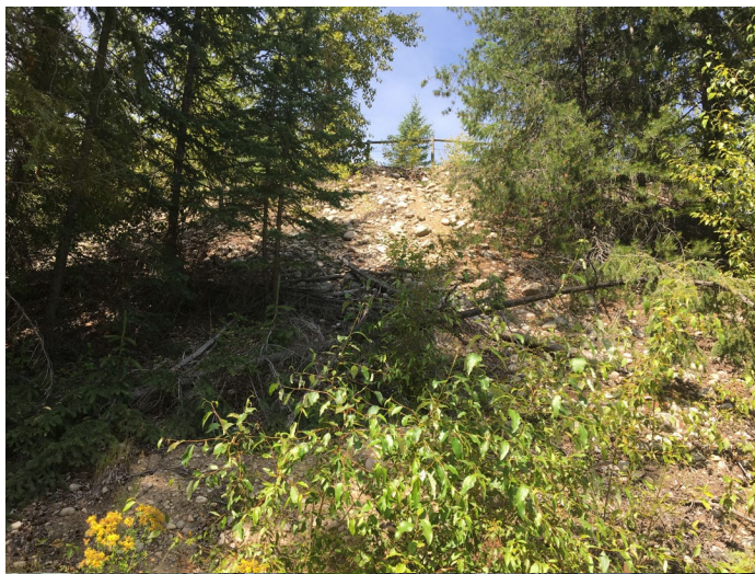
Photograph 7: South TSF, Cell 5, downstream slope, minor erosion, looking northwest. 21 July 2020.
