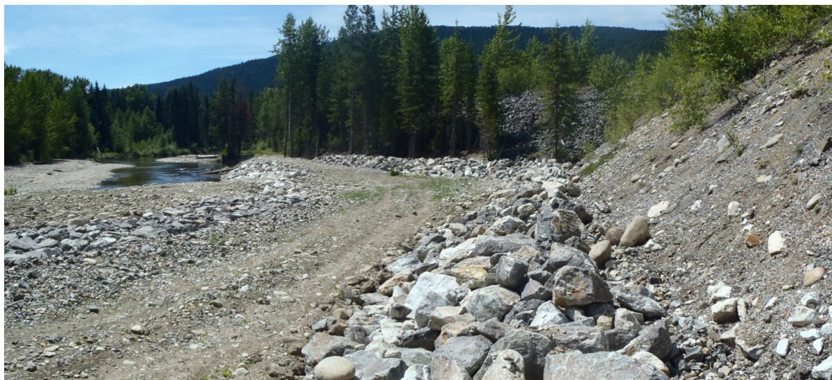
Photograph 9: South TSF, Cell 4/5 downstream toe with recently installed riprap along West Kettle River, looking south. 21 July 2020.
