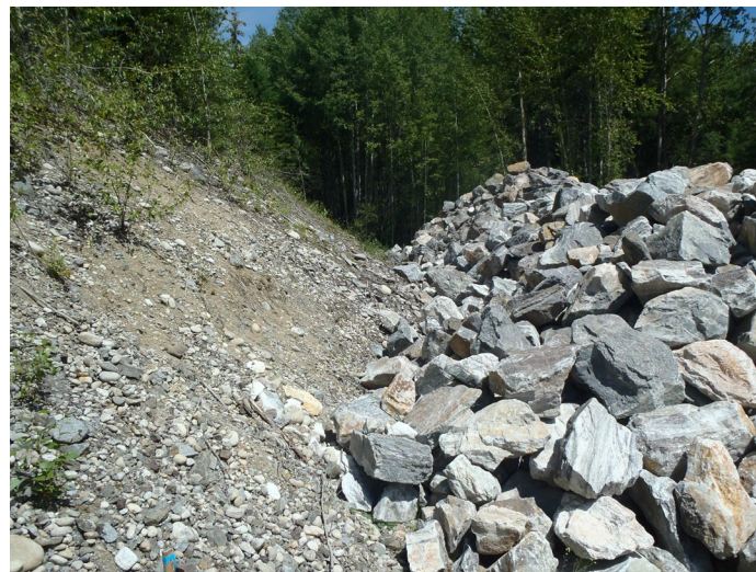
Photograph 13: South TSF, Cell 4, downstream slope and emergency riprap stockpile, looking northeast. 21 July 2020.
