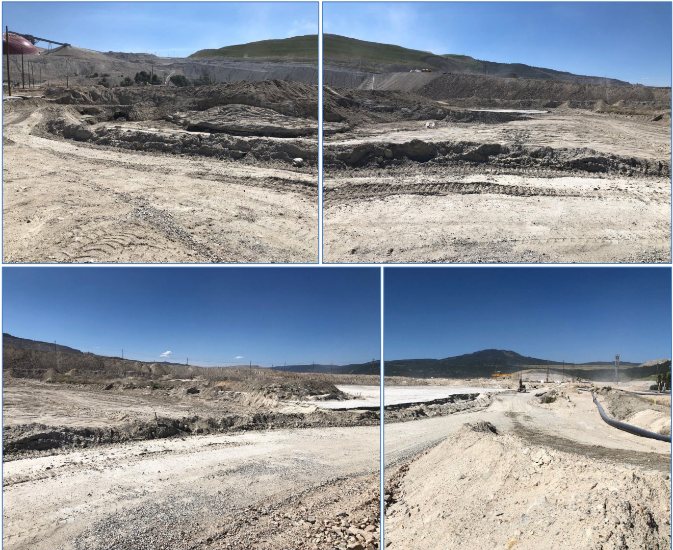
Photo I-1 7-Day Pond. No discharge to the pond. Tailings were being excavated at the time of inspection (SDP-2020-01)
