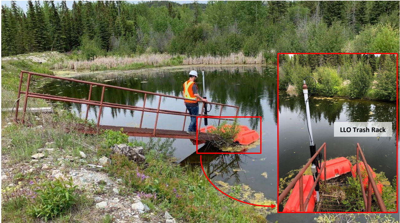
Photo II-C-10 Overview of the pond, catwalk and Low-Level Outlet (LLO) inlet (TRJ-2019-20 and TRJ-2019-26)
