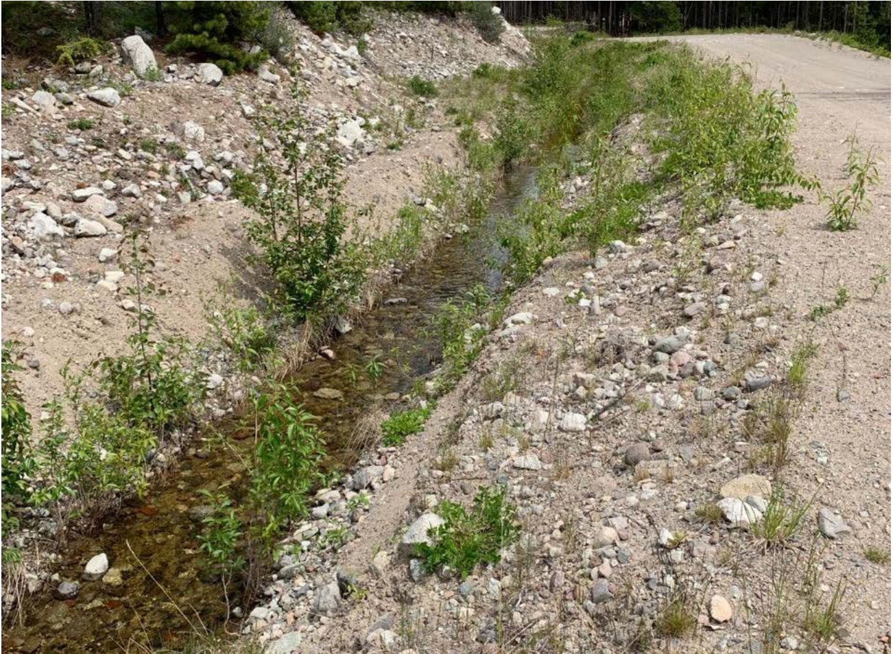
Photo II-A-26 Water flowing in the unlined section of channel upstream of Valve 1 (TRJ-2019-16)
