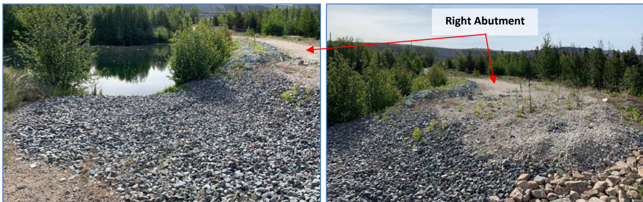
Photo II-B-5 Overview of pond and spillway inlet – Spillway inlet is clear of debris. Vegetation build up near inlet to be cleared as part of routine maintenance prior to 2020 freshet. (TRJ-2019-21)
