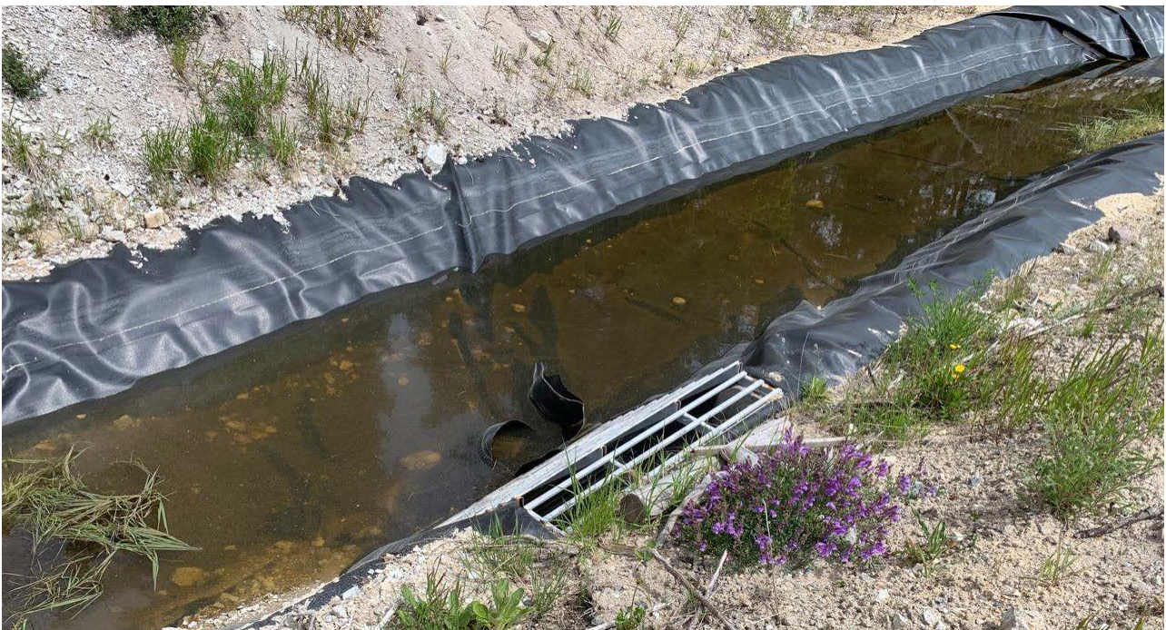
Photo II-A-23 Water standing at the pipe intake. No outflow was observed, outlet valve is closed. Diversion channel flow being discharges from outlet further upstream at Photo II-A-26. (TRJ-2019-14)
