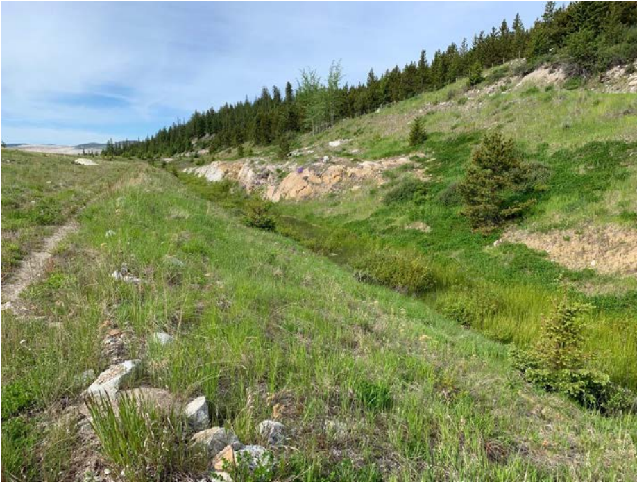
Photo II-A-11 Overview of first length of spillway channel, looking toward southwest (top photo) and looking toward northeast (bottom photo). No sign of recent flow or weathering / disruption of riprap was observed. No evidence of sloughing of cut slopes was observed. Channel is heavily vegetated and should be cleared as part of routine maintenance (TRJ-2019-07)
