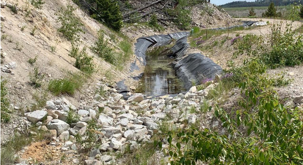
Photo II-A-23 Water standing at the pipe intake. No outflow was observed, outlet valve is closed. Diversion channel flow being discharges from outlet further upstream at Photo II-A-26. (TRJ-2019-14)
