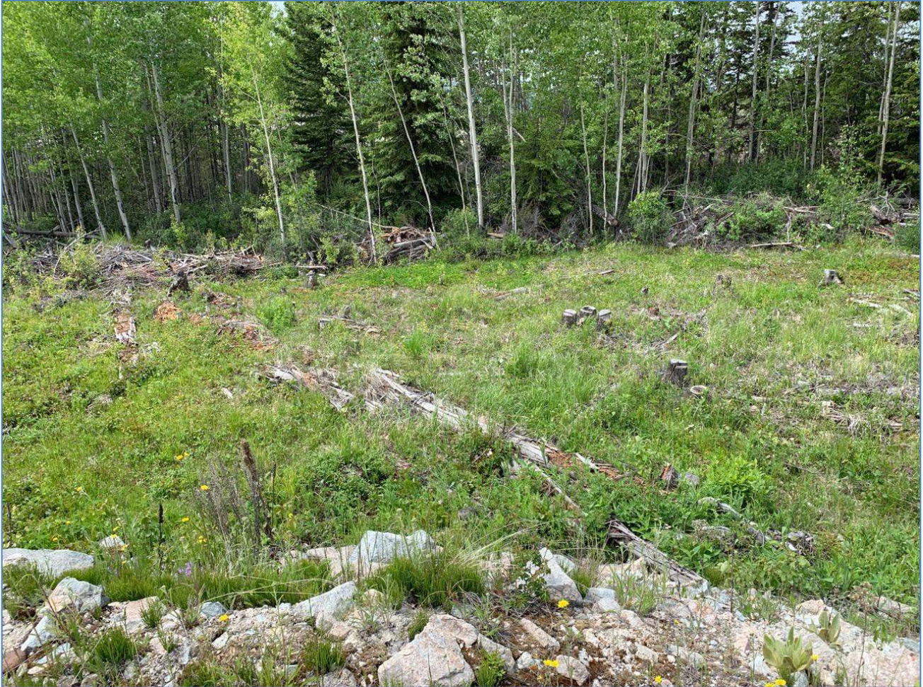
Photo II-C-8 Spillway channel looking toward west (TRJ-2019-25)
