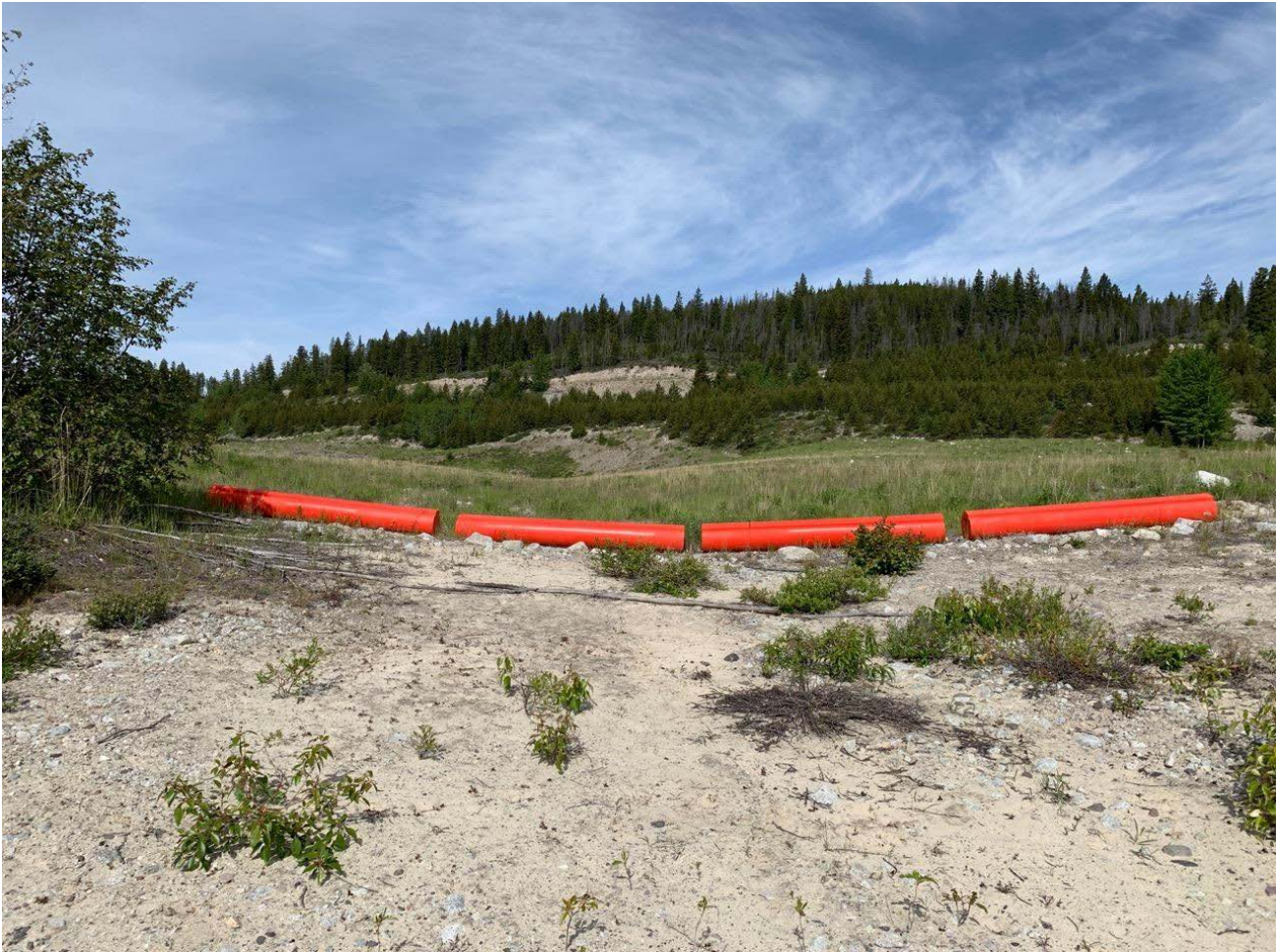
Photo II-A-10 Trojan spillway inlet. Approach channel is clear and debris boom is secured. (TRJ-2019-06)
