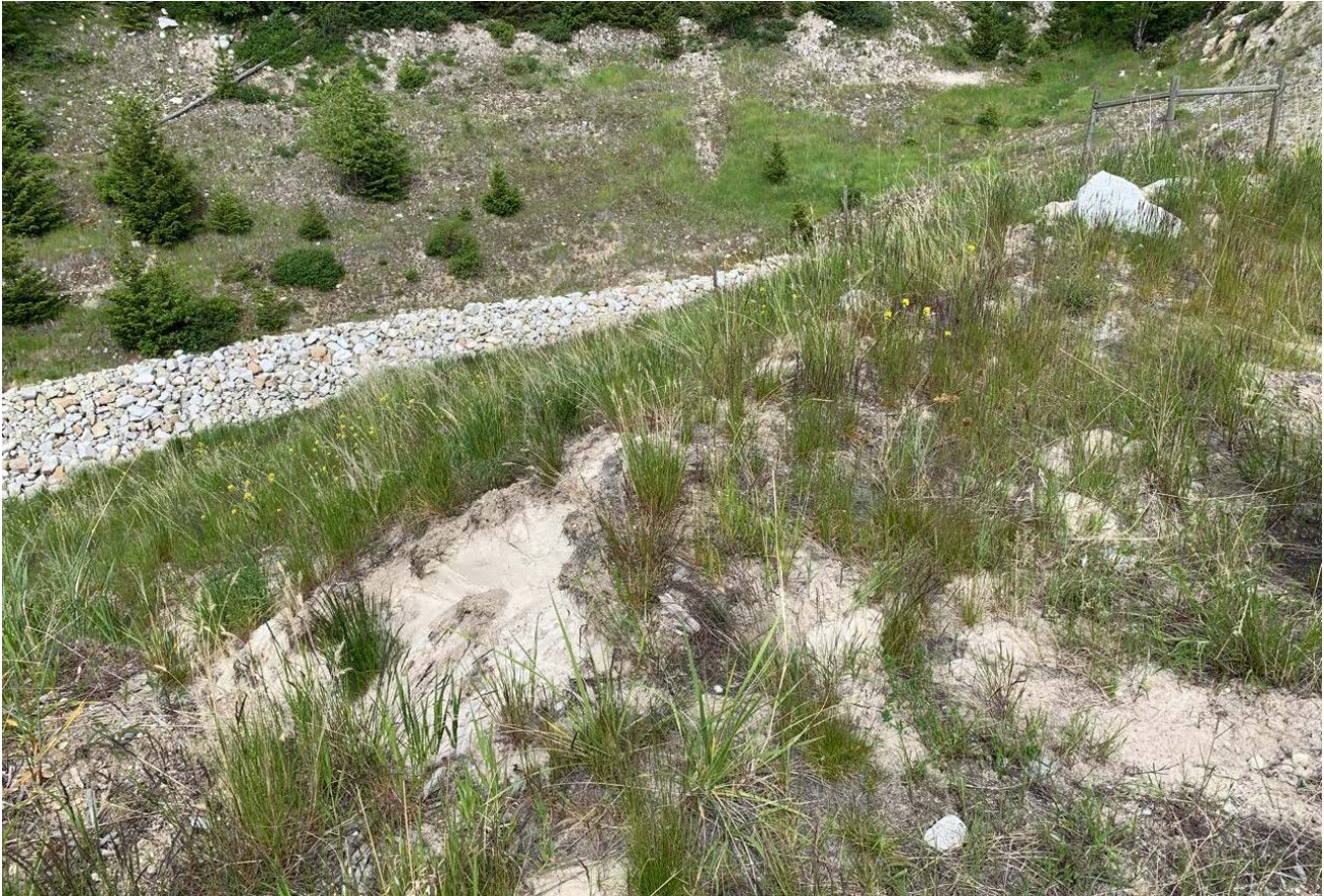
Photo II-A-20 Surface erosion scour upslope of the u/s sand observed in spillway channel (refer to Photo II-A-14). Not seepage flow related. KCB recommends repairing the area. (TRJ-2019-11)
