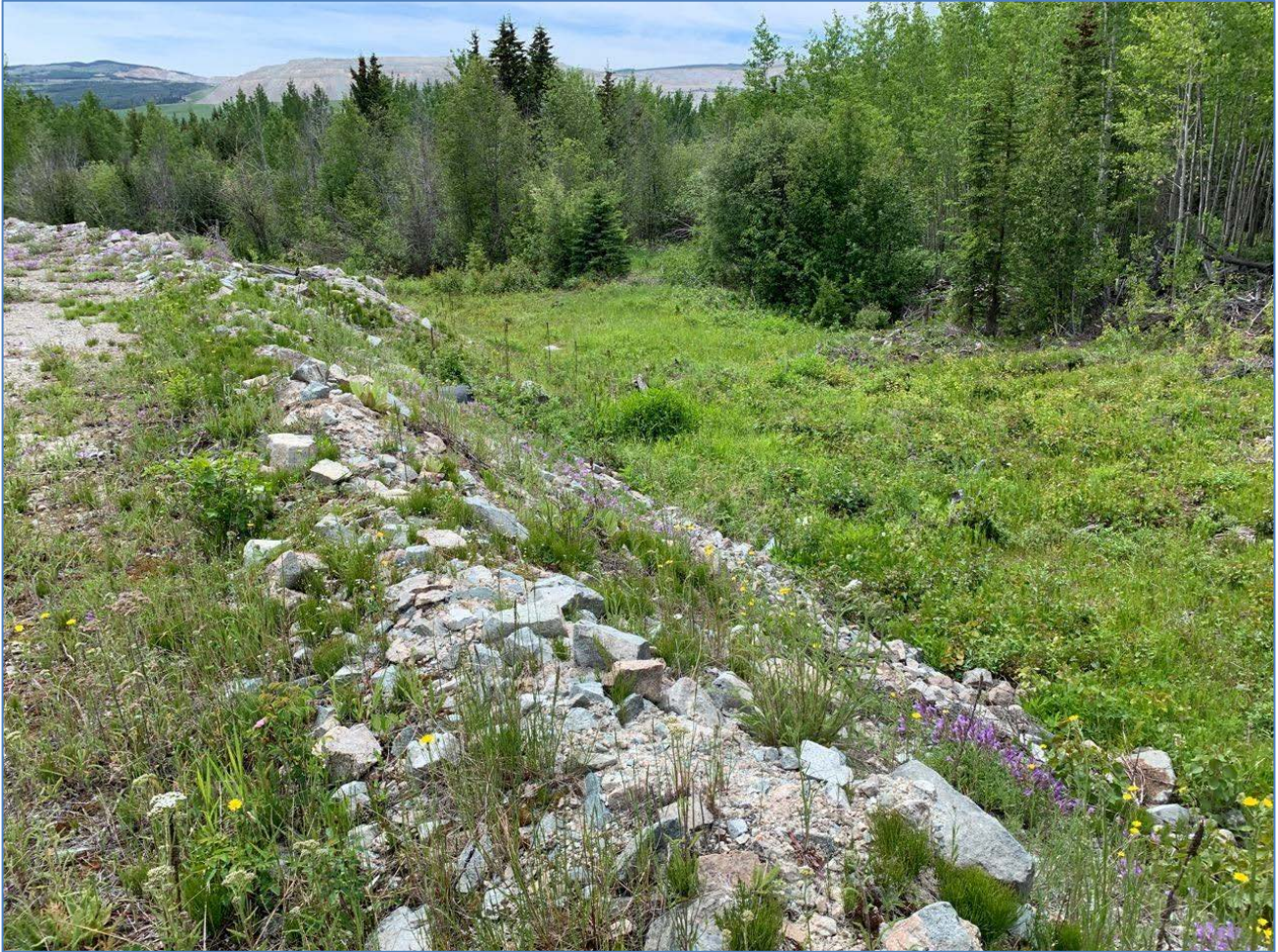
Photo II-C-7 Spillway channel looking toward southwest. Channel is cleared from trees or major debris (TRJ-2019-25)
