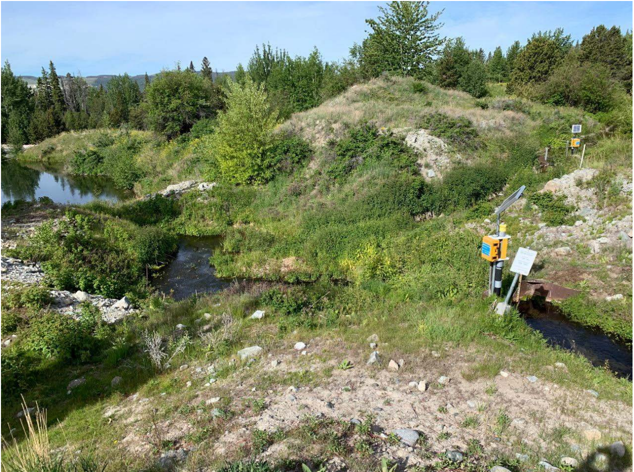
Photo II-A-7 Overview of weir TD-R4-SF01 and weir TD-R4-SF02 downstream of East and West Seepage Collection Ditches (TRJ-2019-04)
