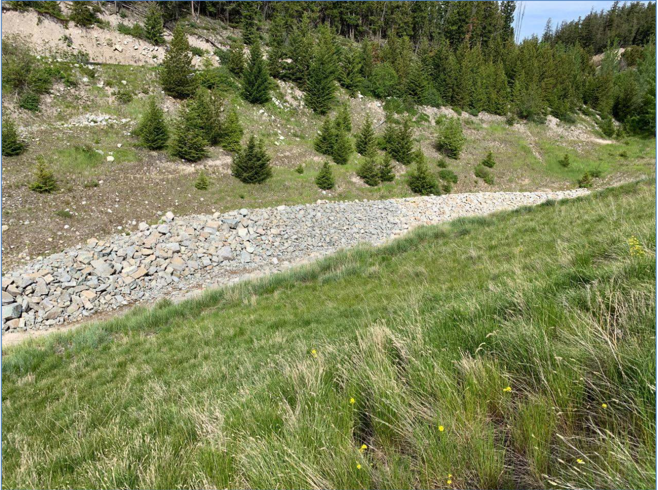
Photo II-A-13 Overview of spillway channel, looking toward north. (TRJ-2019-09)
