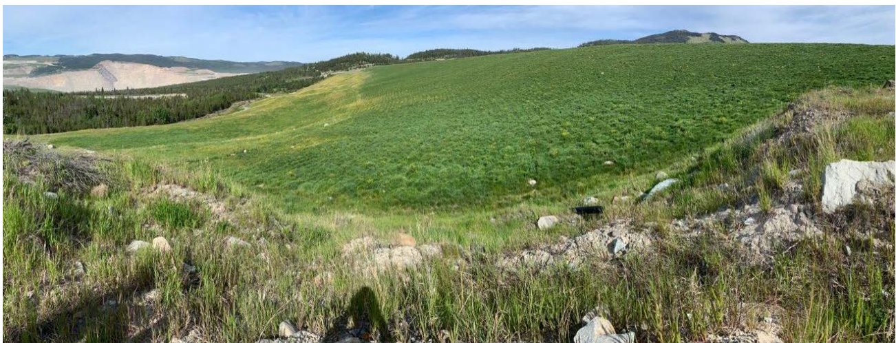
Photo II-A-2 Panoramic overview of Trojan Dam downstream slopes from left abutment. No visible erosion or scour. (TRJ-2019-02)
