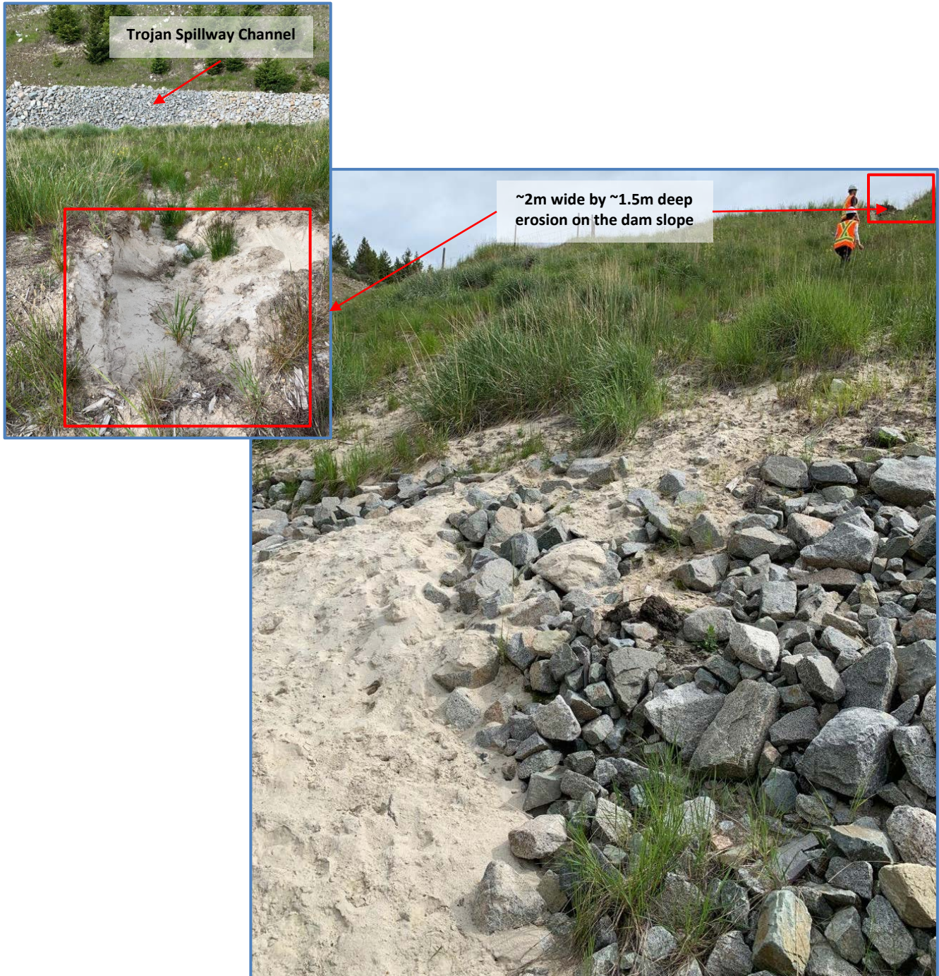
Photo II-A-18 Fan shape sand area observed in spillway channel. Surface erosion / scour evidence was observed upslope on dam slope. Visually looks more fluviially deposited and is not seepage-related. KCB recommends THVCP repair the scour and re-establish the cover. (TRJ-2019-11 and TRJ-2019-12)
