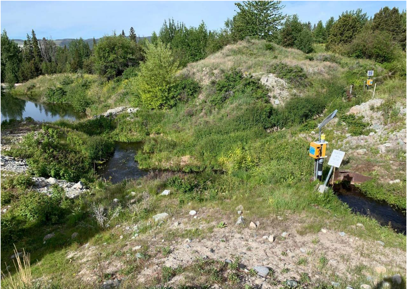
Photo II-B-8 Overview of weir TD-R4-SF01 and weir TD-R4-SF02, downstream of East and west Seepage Collection Ditches (TRJ-2019-04)
