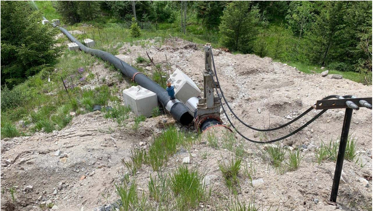
Photo II-A-25 Valve 1 is open and no flowing water bypassing this point was observed. Valve is located at the transition of unlined to lined channel. (TRJ-2019-16)
