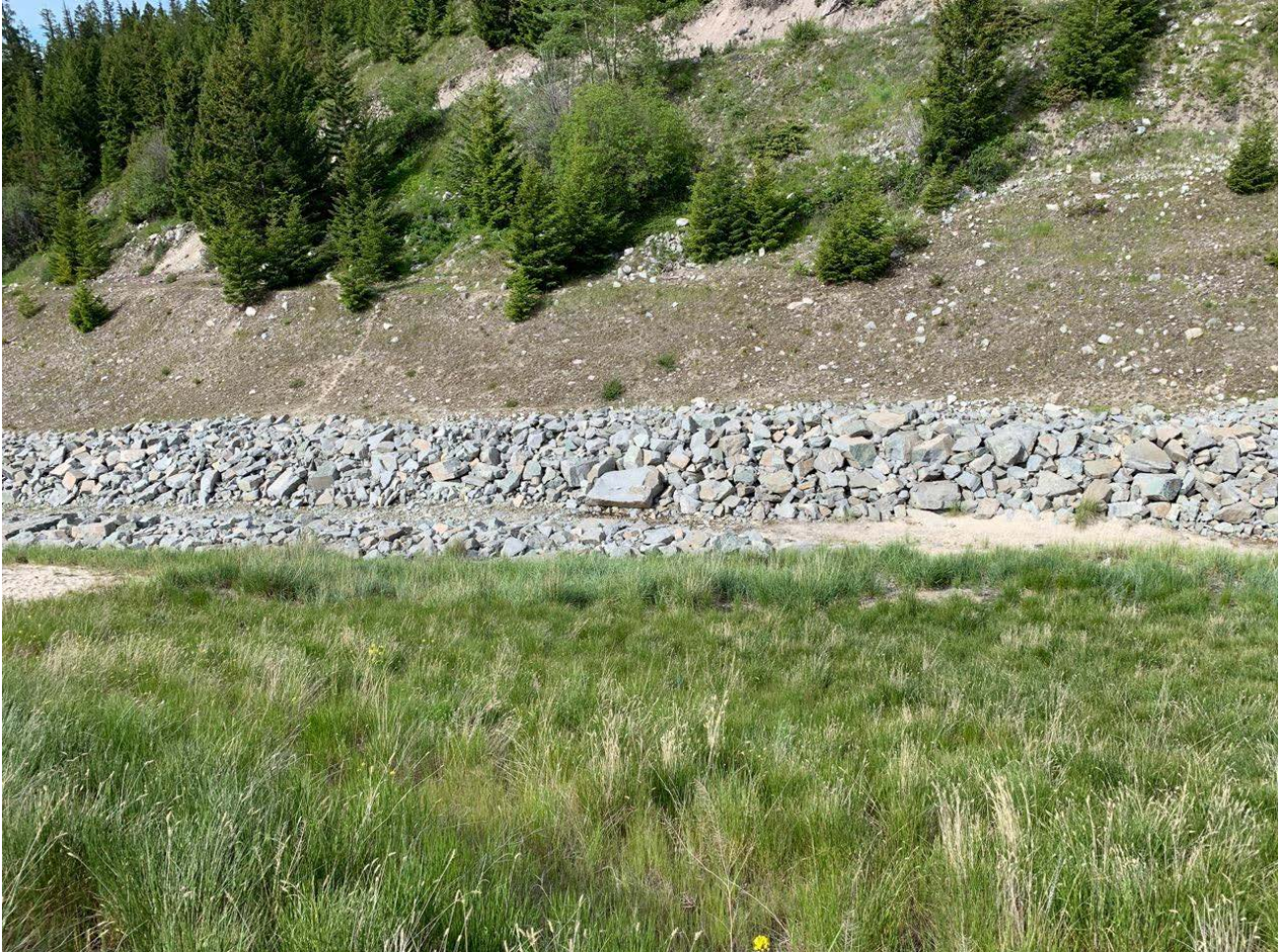
Photo II-A-15 Overview of spillway channel, looking toward west. Some eroded sand from area has accumulated in channel. Not a concern as it would be washed away by flow. (TRJ-2019-09)
