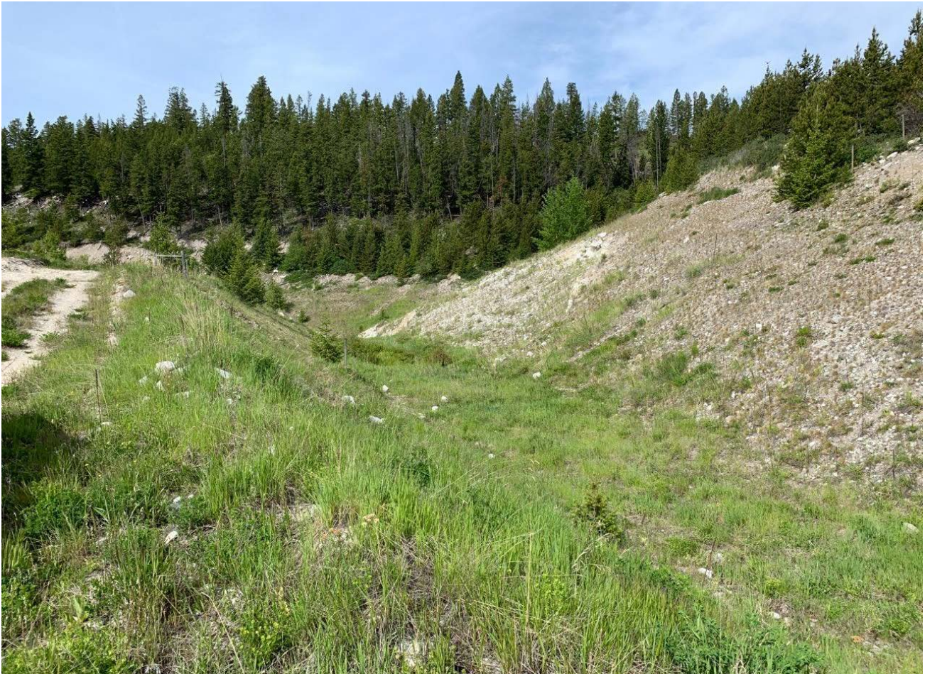
Photo II-A-12 Overview of spillway channel, downstream of chute. Slopes are in good condition. (TRJ-2019-08)
