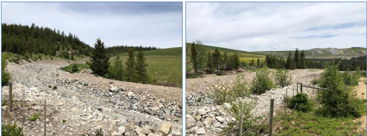
Photo II-A-21 Overview of 2018 Extension Trojan Dam spillway and the toe of right abutment (TRJ-2019-13)
