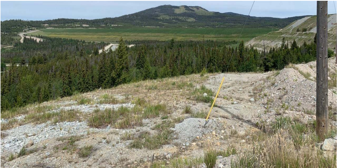
Photo II-A-9 Overview of Trojan Tailings Pond. Pond level appears similar to previous years. Sand beach is exposed. (TRJ-2019-06)
