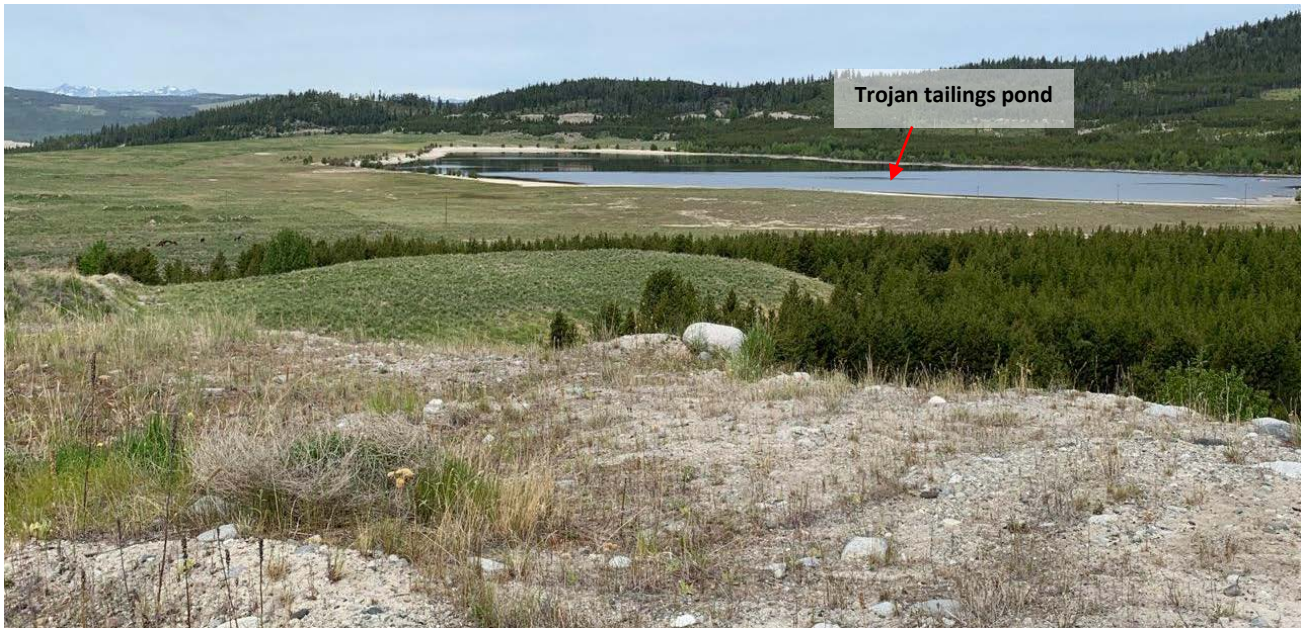
Photo II-A-2 Panoramic overview of Trojan Dam downstream slopes from left abutment. No visible erosion or scour. (TRJ-2019-02)
