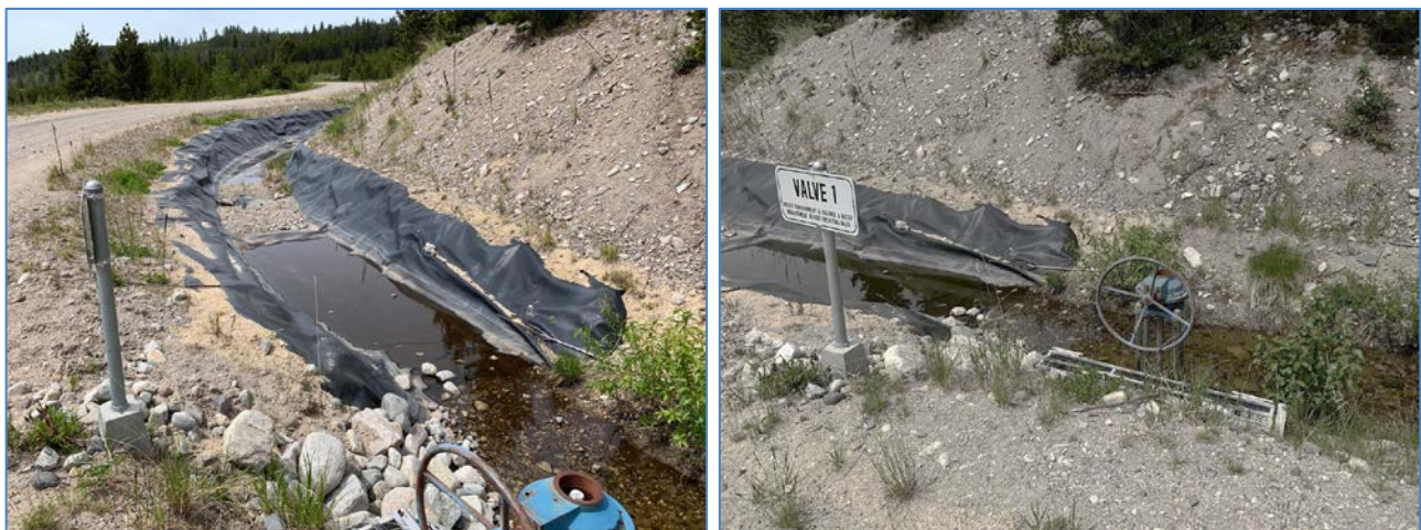
Photo II-A-25 Valve 1 is open and no flowing water bypassing this point was observed. Valve is located at the transition of unlined to lined channel. (TRJ-2019-16)
