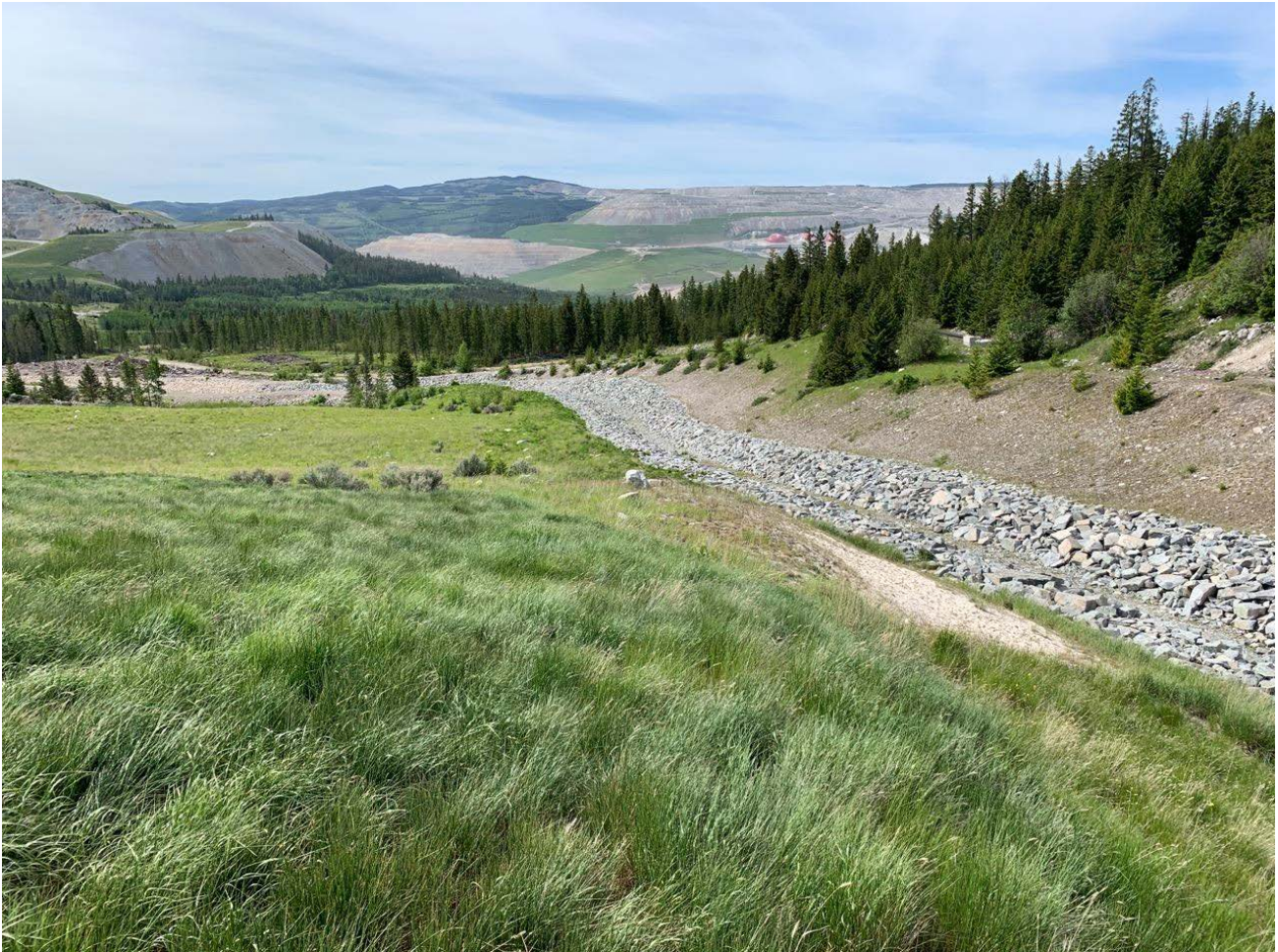
Photo II-A-14 Overview of spillway channel, looking toward south. No sign of recent flow or weathering / disruption of riprap was observed. Exposed sand in slope (as per 2018 DSI) was not covered. Not a dam safety concern as there is no active seepage faces or erosion were observed. (TRJ-2019-09)
