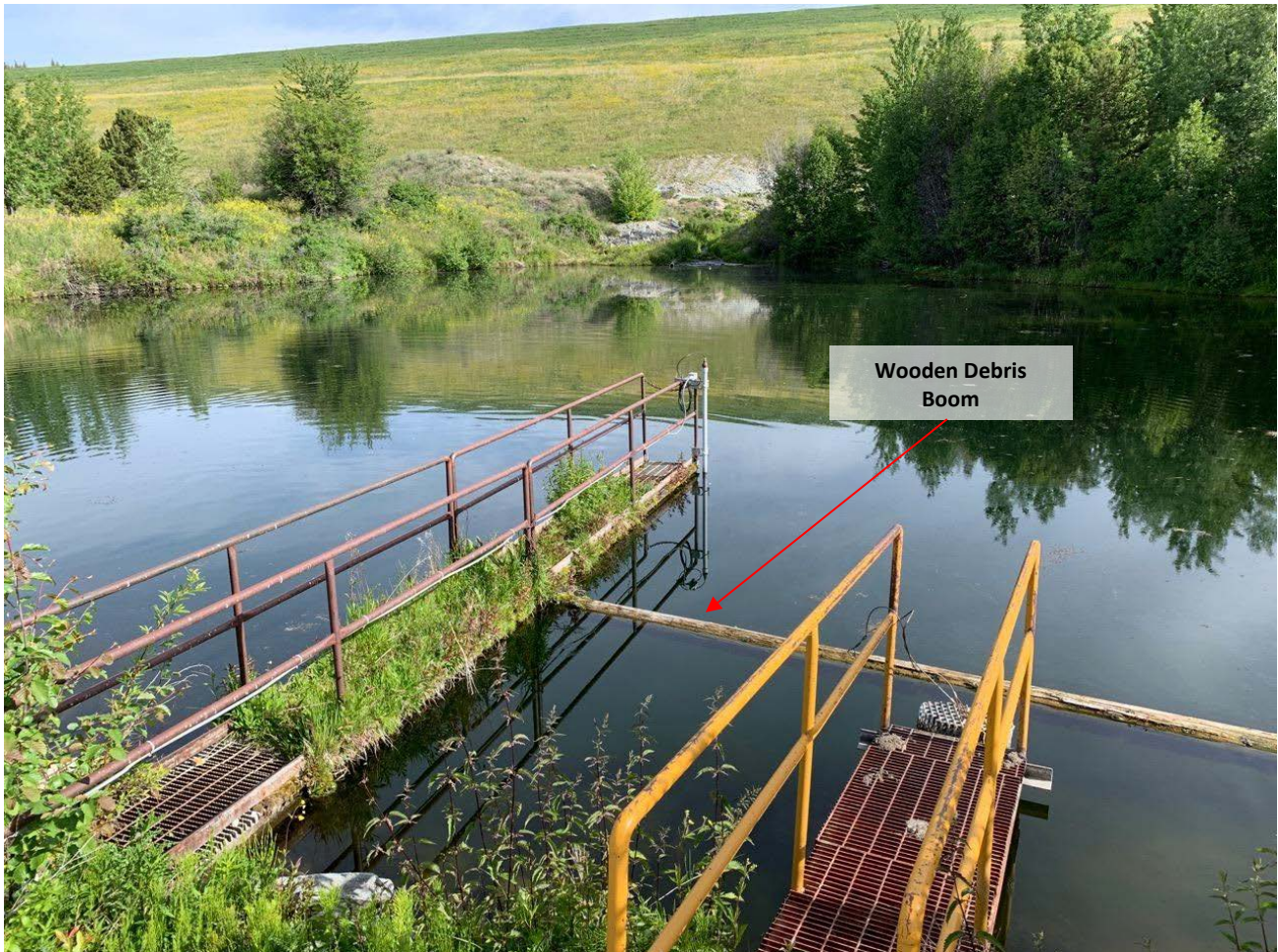
Photo II-B-5 Overview of pond and spillway inlet – Spillway inlet is clear of debris. Vegetation build up near inlet to be cleared as part of routine maintenance prior to 2020 freshet. (TRJ-2019-21)
