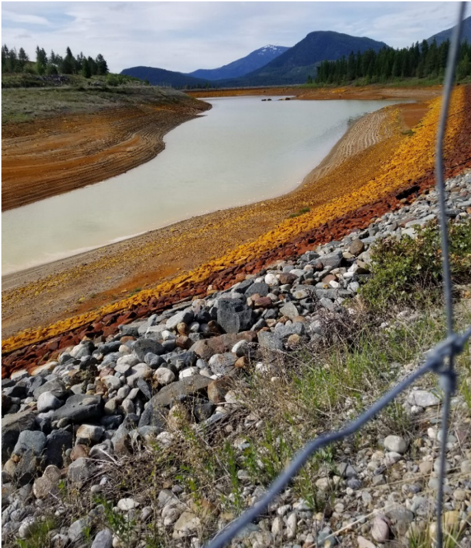
Photo 1.8 ARD North Dam Downstream Slope (251)
