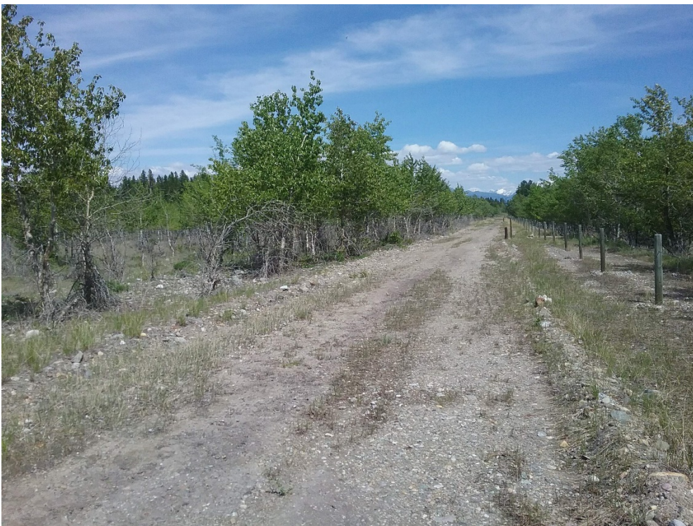
Photo 6.1 Crest of Calcine Dike (358)
