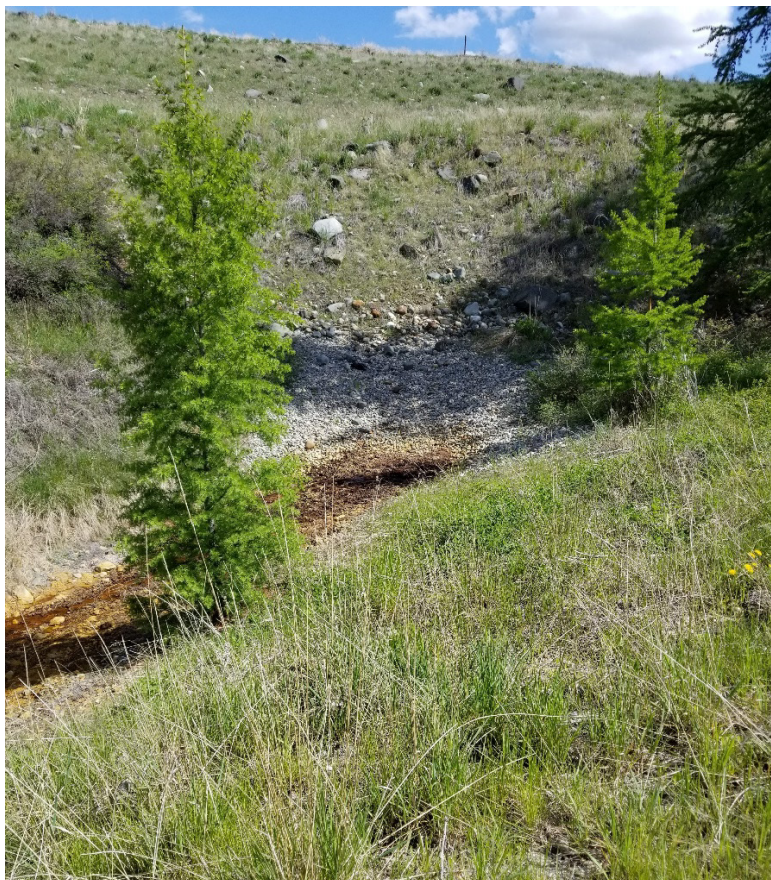
Photo 2.6 Seepage at Toe of Iron Dike (139)
