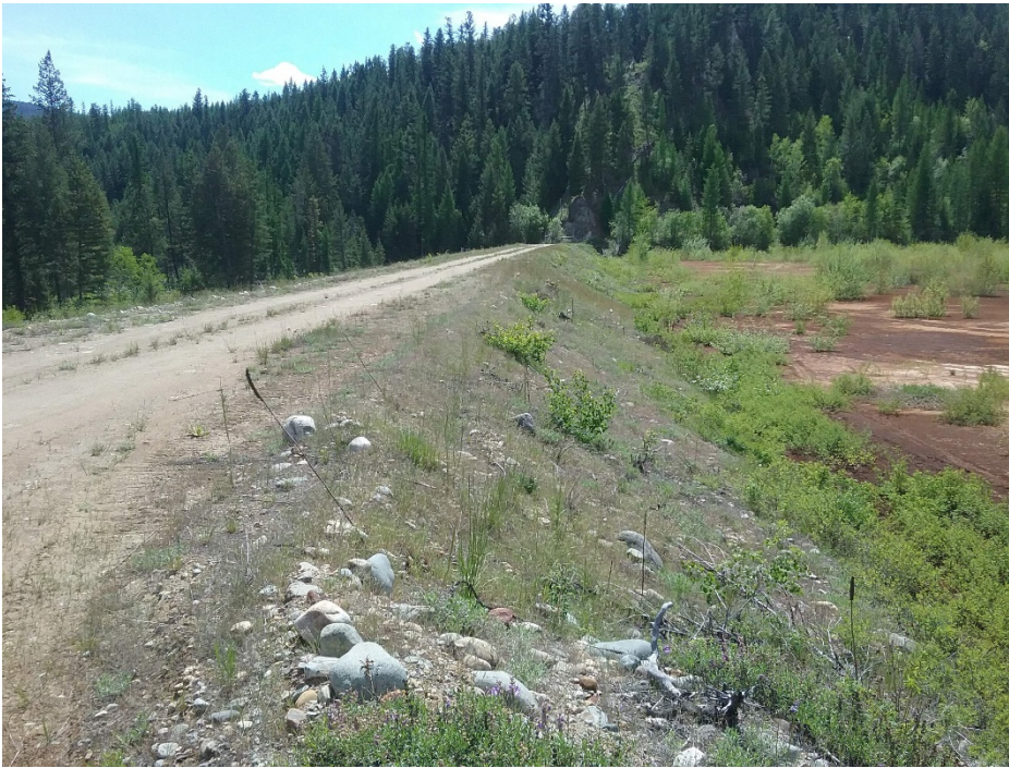
Photo 5.5 South Dike Upstream Slope and Crest (350)
