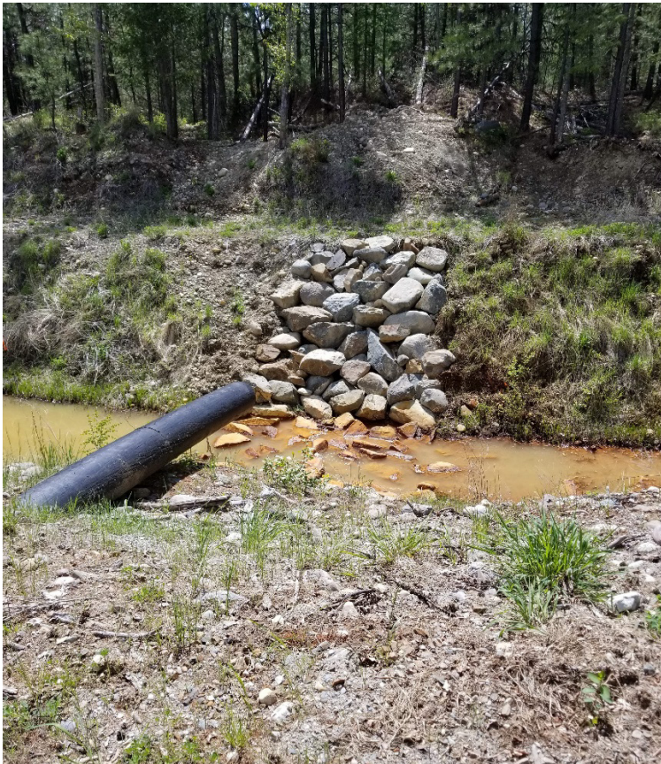
Photo 3.4 No. 3 Siliceous Dike Downstream Slope and Siliceous Spillway (149)
