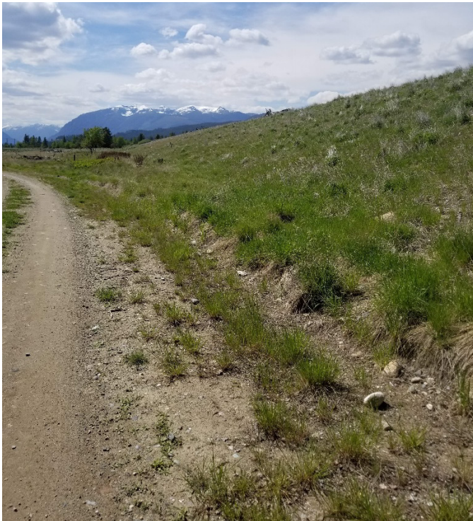
Photo 4.3 Animal Burrows at Toe of East Gypsum (171)
