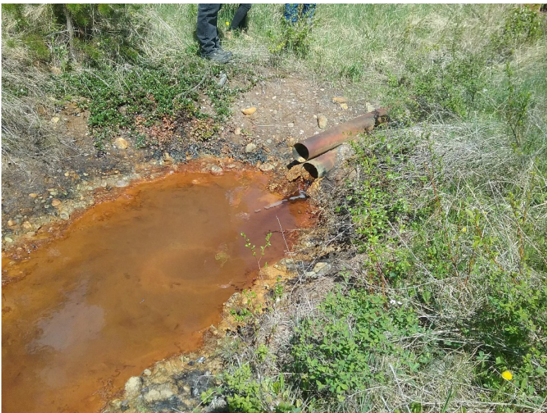
Photo 3.2 Historic Decant Downstream of No. 3 Siliceous Dike (286)
