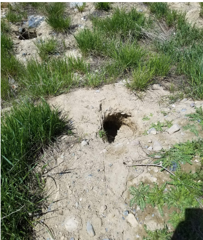
Photo 4.3 Animal Burrows at Toe of East Gypsum (171)
