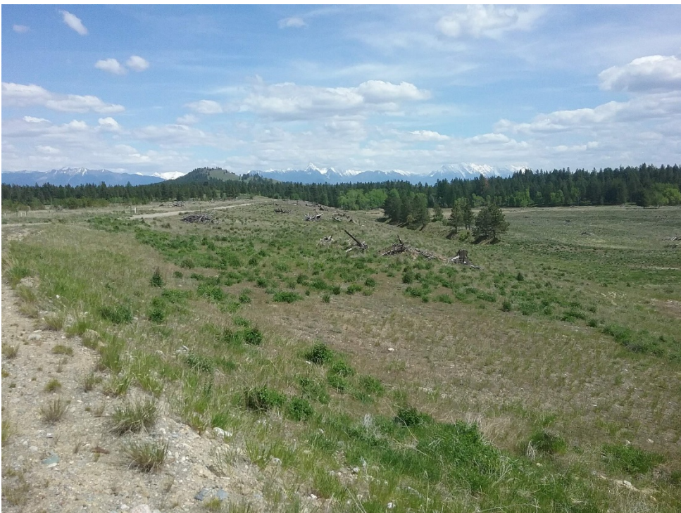
Photo 4.1 Crest and Downstream Slope of East Gypsum Dike (295)
