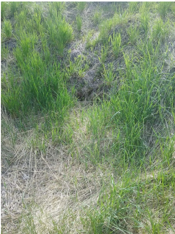
Photo 1.10 Animal Burrow on ARD North Dam (256)
