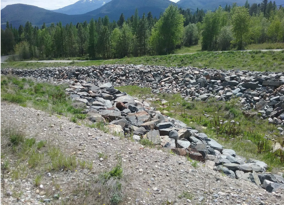
Photo 4.7 Emergency Spillway and Culvert Entrance (180)
