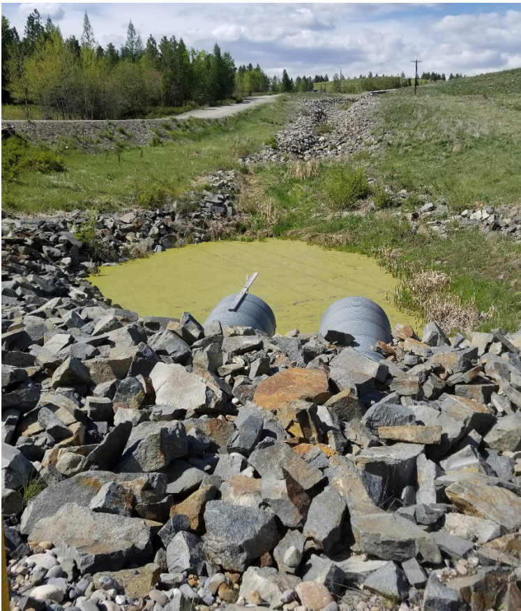
Photo 4.7 Emergency Spillway and Culvert Entrance (180)
