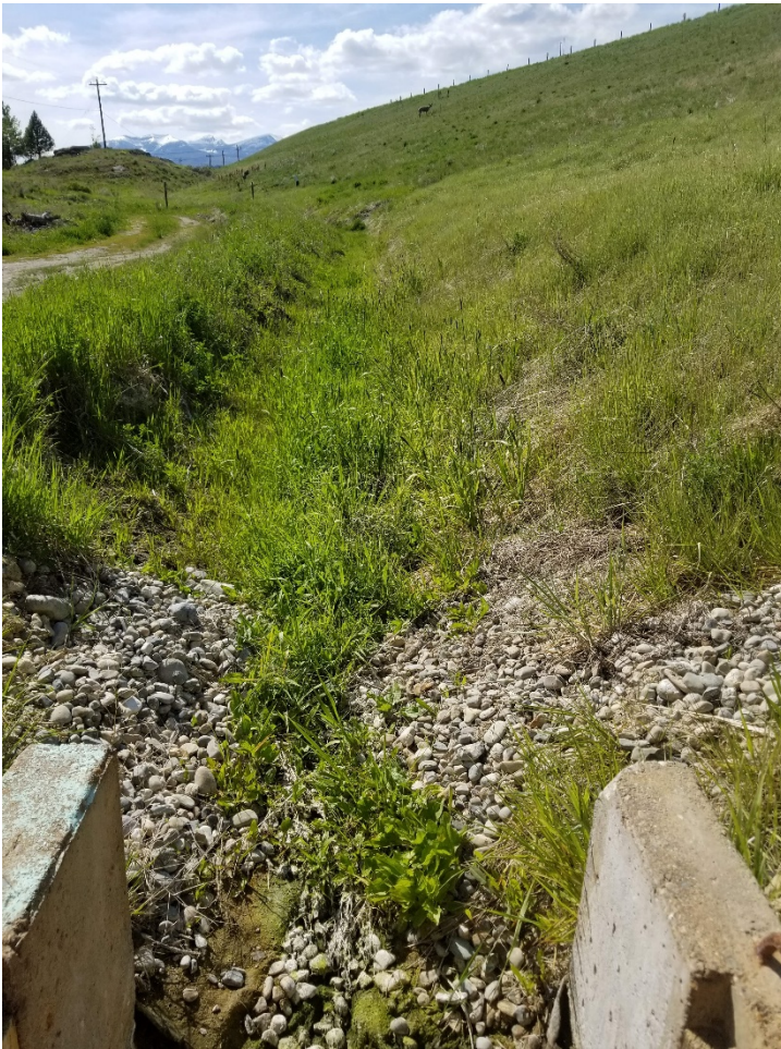
Photo 1.15 Weir 1 and Toe of ARD South Dam (186)
