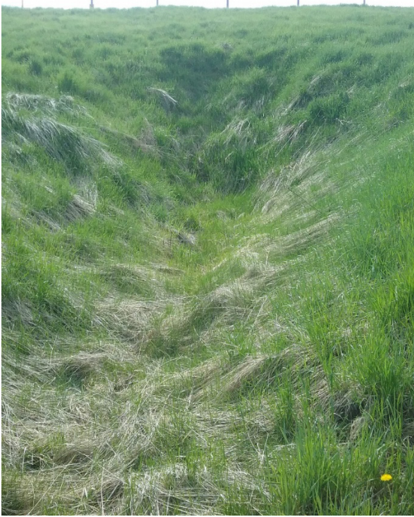
Photo 1.10 Animal Burrow on ARD North Dam (256)
