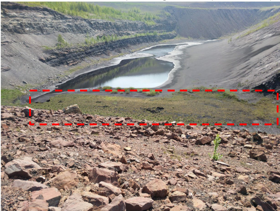
Photo I-7 Upstream slope and impoundment (general area where sinkholes are observed is shown in red box) – looking southeast (SNTD-2019-02)
