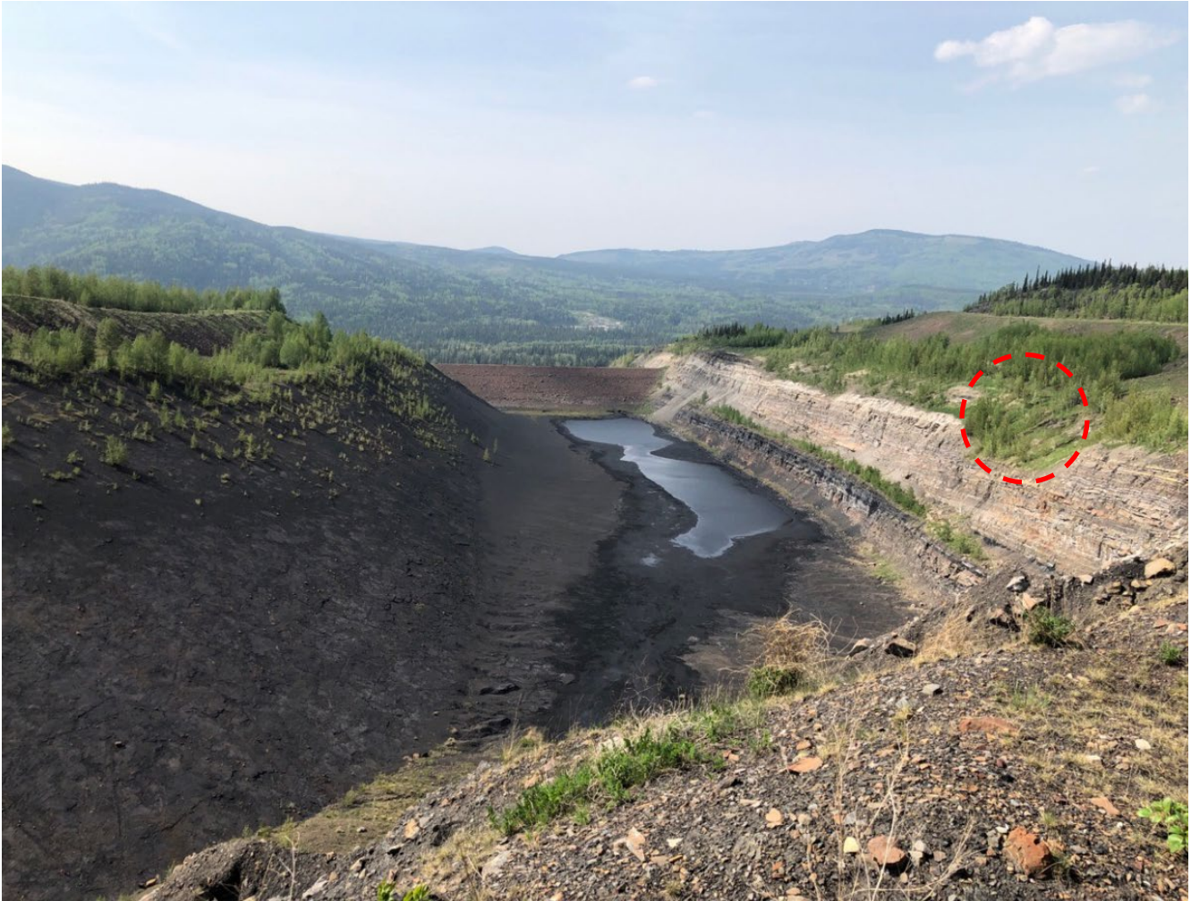
Photo I-16 Shikano North Tailings Dam – looking northwest. Historic slumping failure circled with red dash line (SNTD-2019-06)
