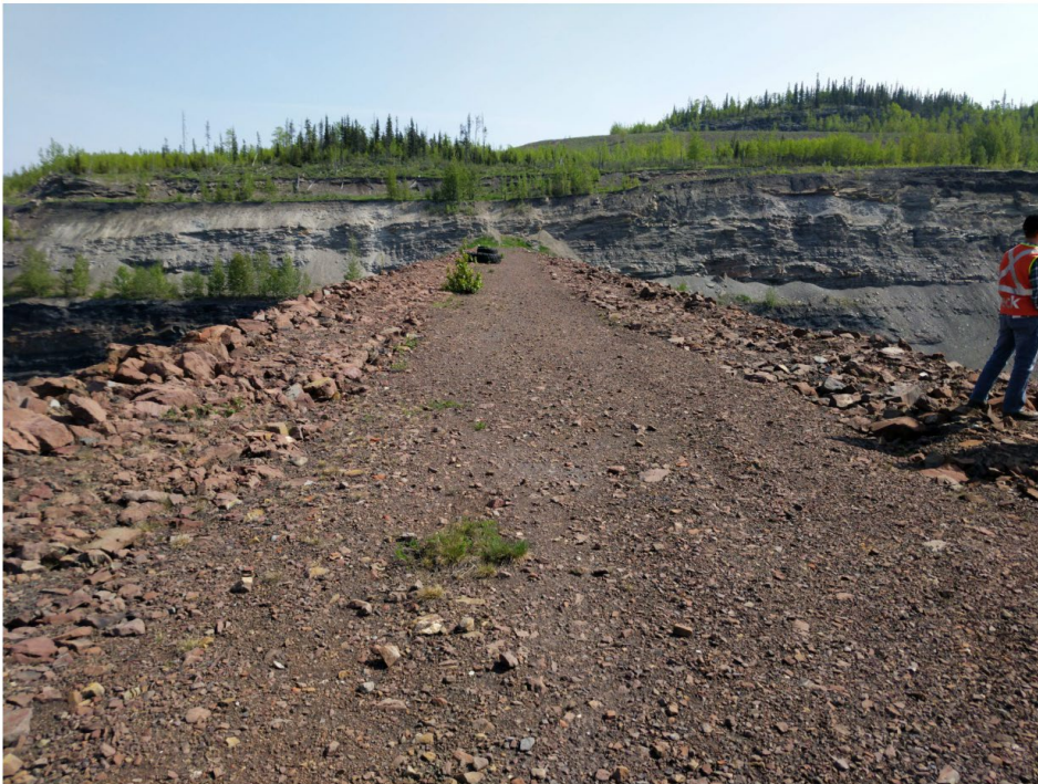
Photo I-2 Dam crest from left abutment – looking northeast (SNTD-2019-01)
