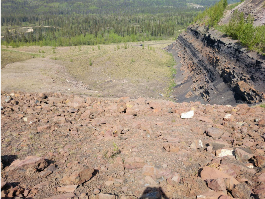
Photo I-8 Downstream slope – looking northwest (SNTD-2019-04)
