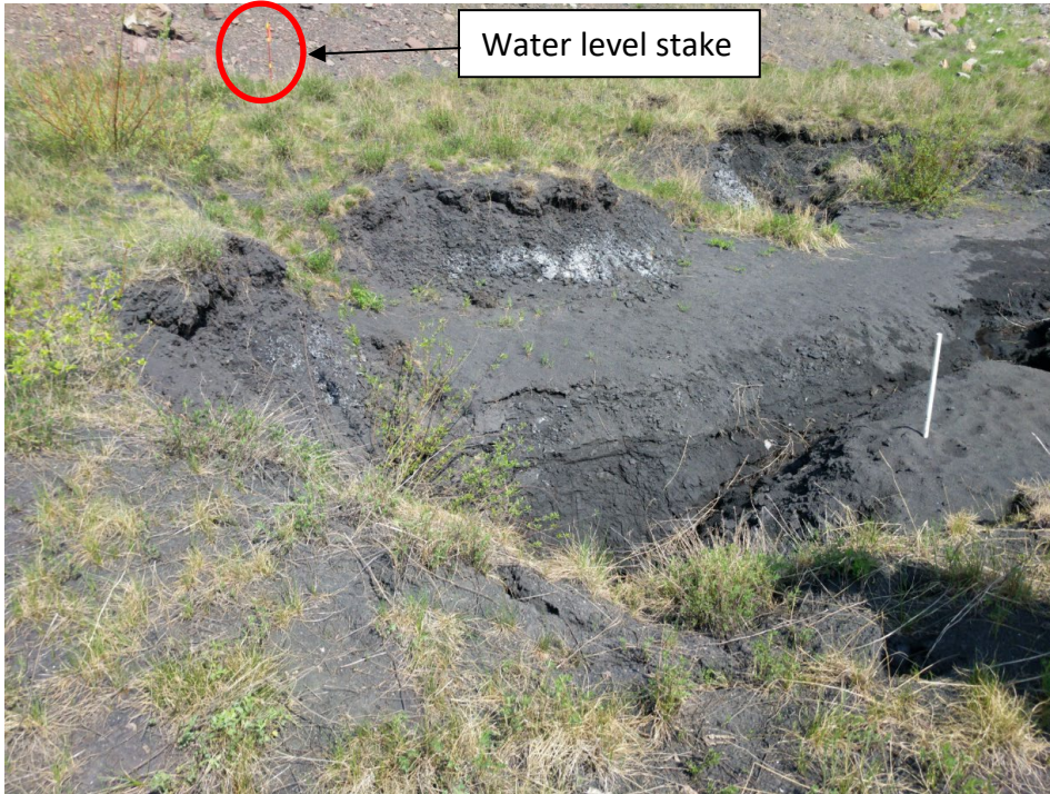
Photo I-10 Sinkhole 11, water level indicator visible in the background (SNTD-SINKHOLE-2019-11)
