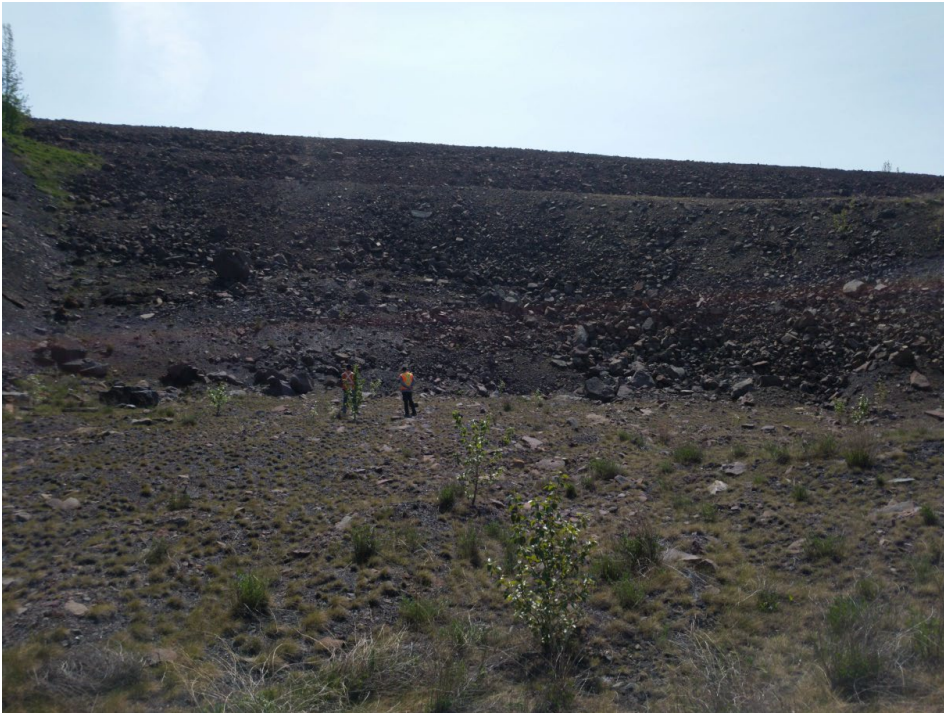
Photo I-4 Downstream slope – looking east (SNTD-2019-03)
