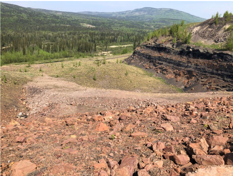
Photo I-3 Downstream slope – looking northwest (SNTD-2019-02)
