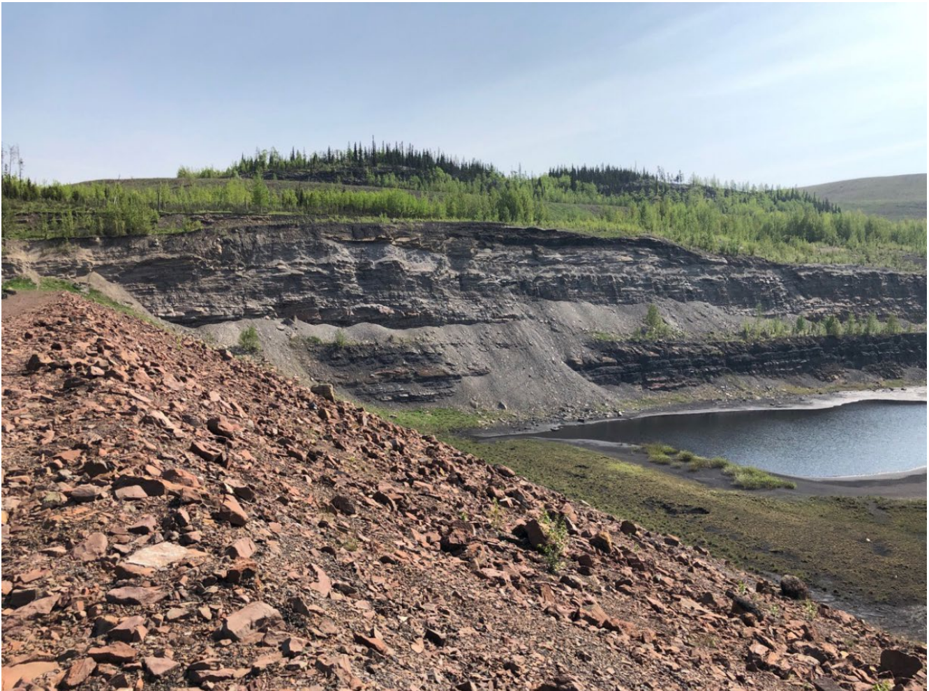
Photo I-1 Upstream slope from the left abutment with pit wall in the background – looking northeast (SNTD-2019-01)
