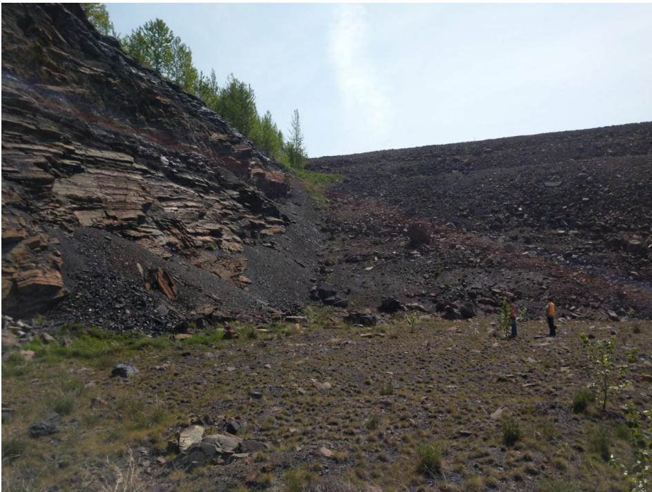
Photo I-5 Downstream right abutment – looking east (SNTD-2019-03)
