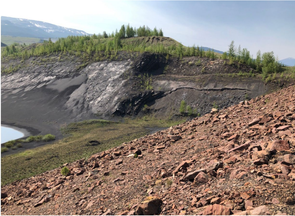
Photo I-6 Ravelling of shale slope upstream of the left abutment – looking southwest (SNTD-2019-04)
